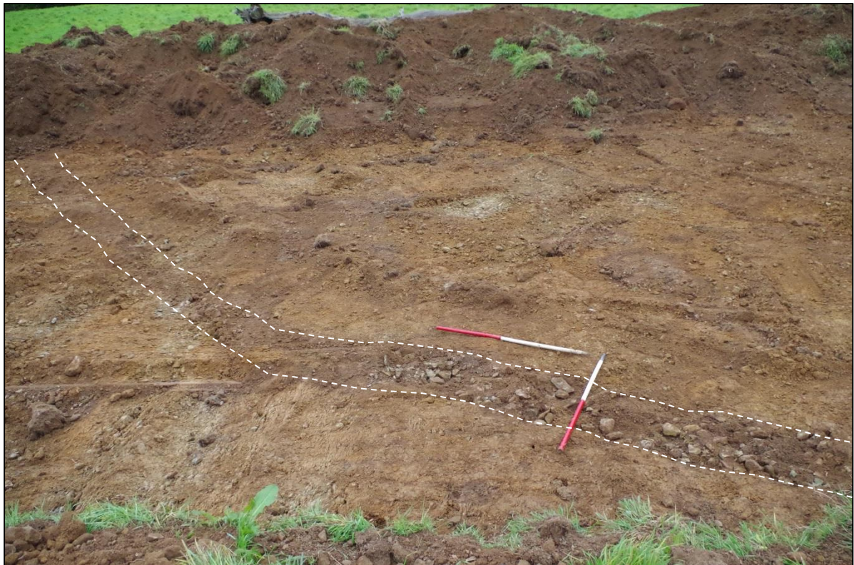
Figure 10. Land drain [14] looking west.
