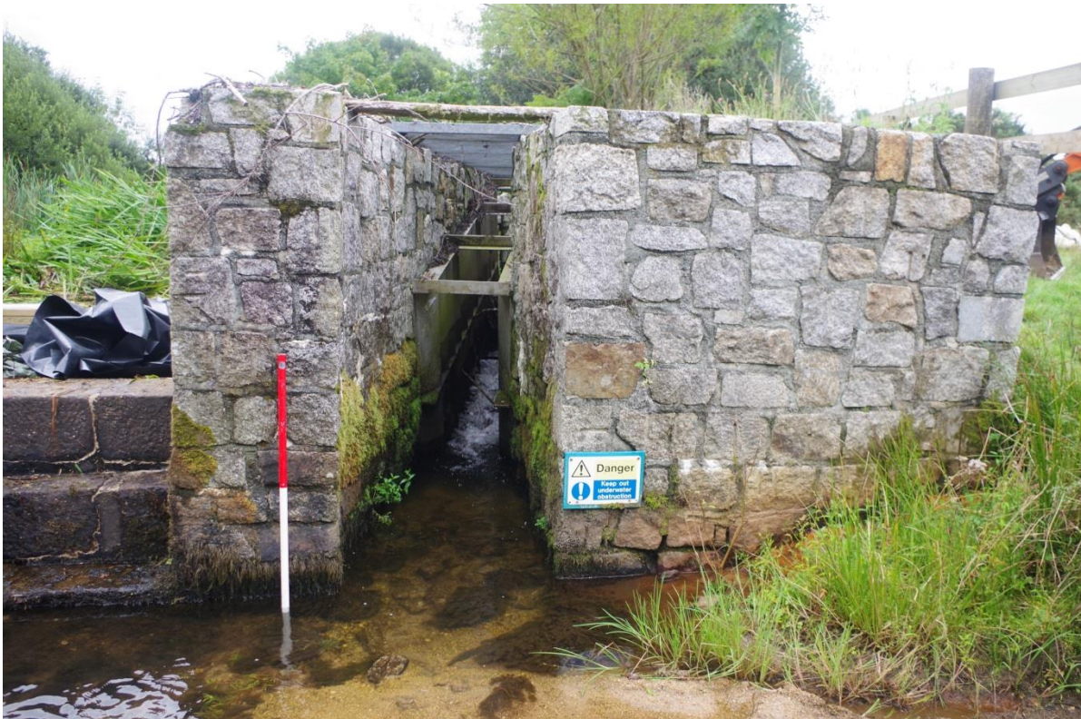
Fig 12 View of the fish pass looking east.
