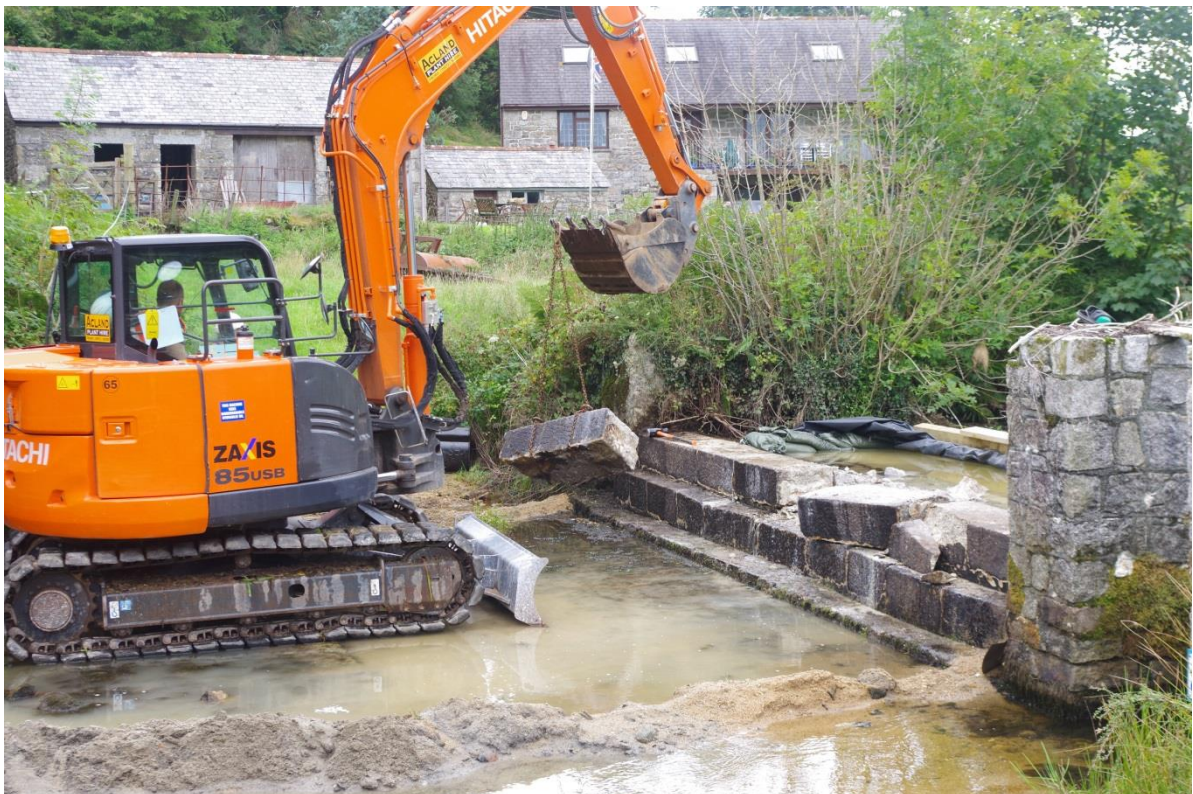
Fig 14 View of the weir during partial demolition looking north.
