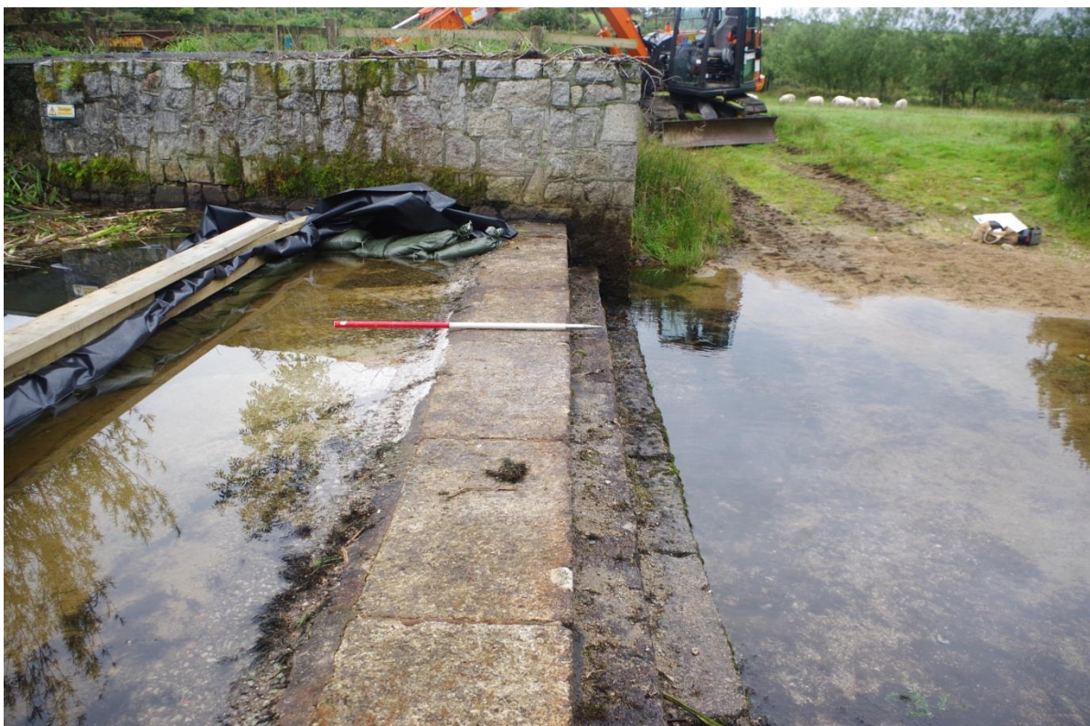
Fig 10 View of the weir and fish pass looking south.
