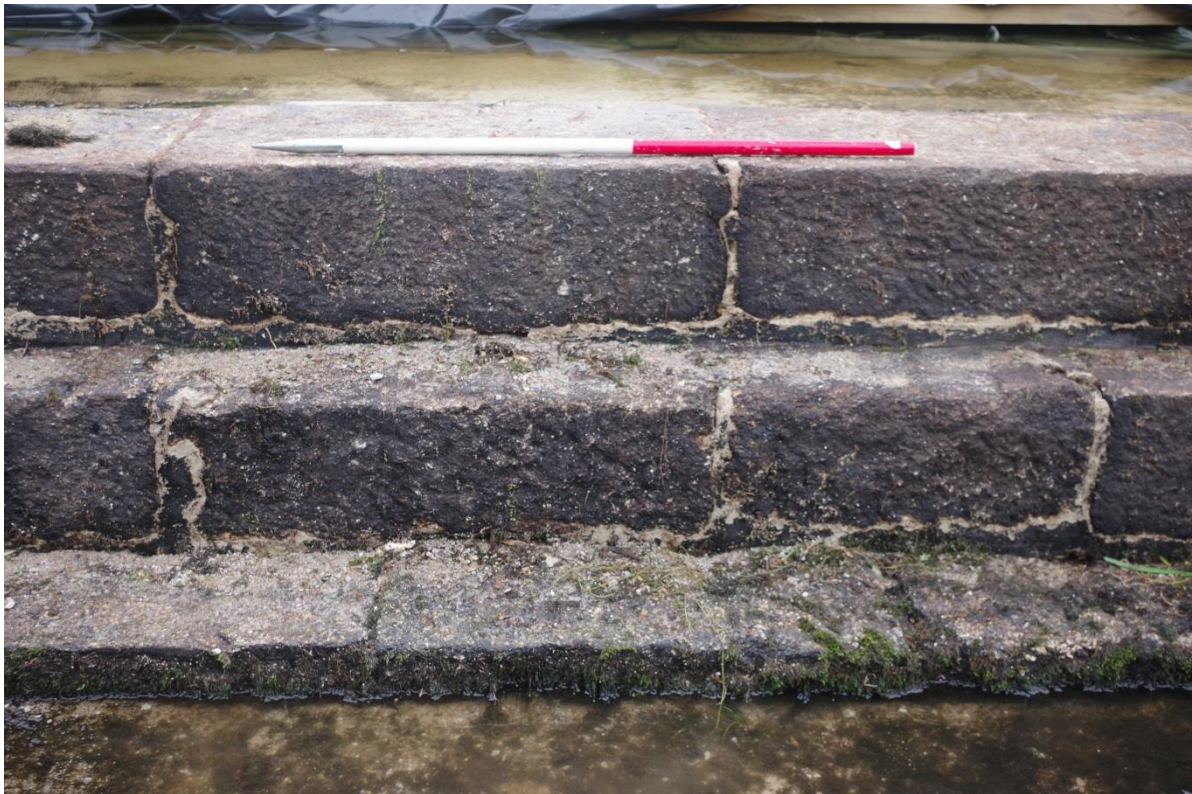
Fig 9 Detail of stepped, reused granite blocks.
