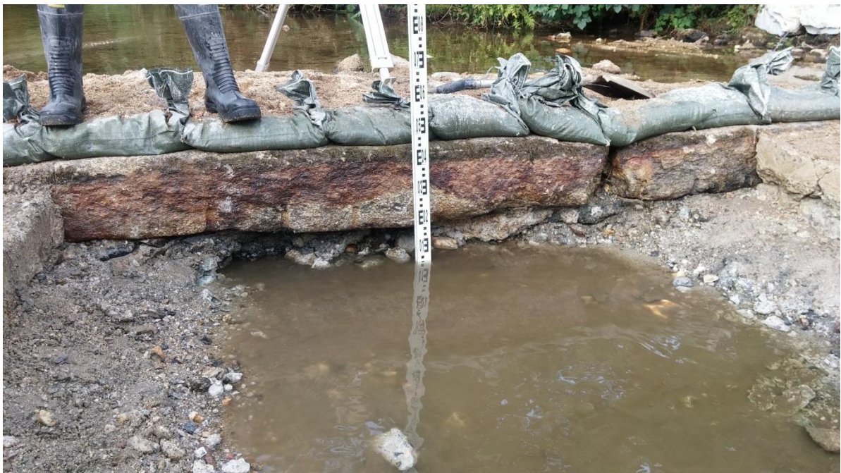
Fig 16 Reused granite edging blocks of ford with early/mid 19 th century drill marks.
