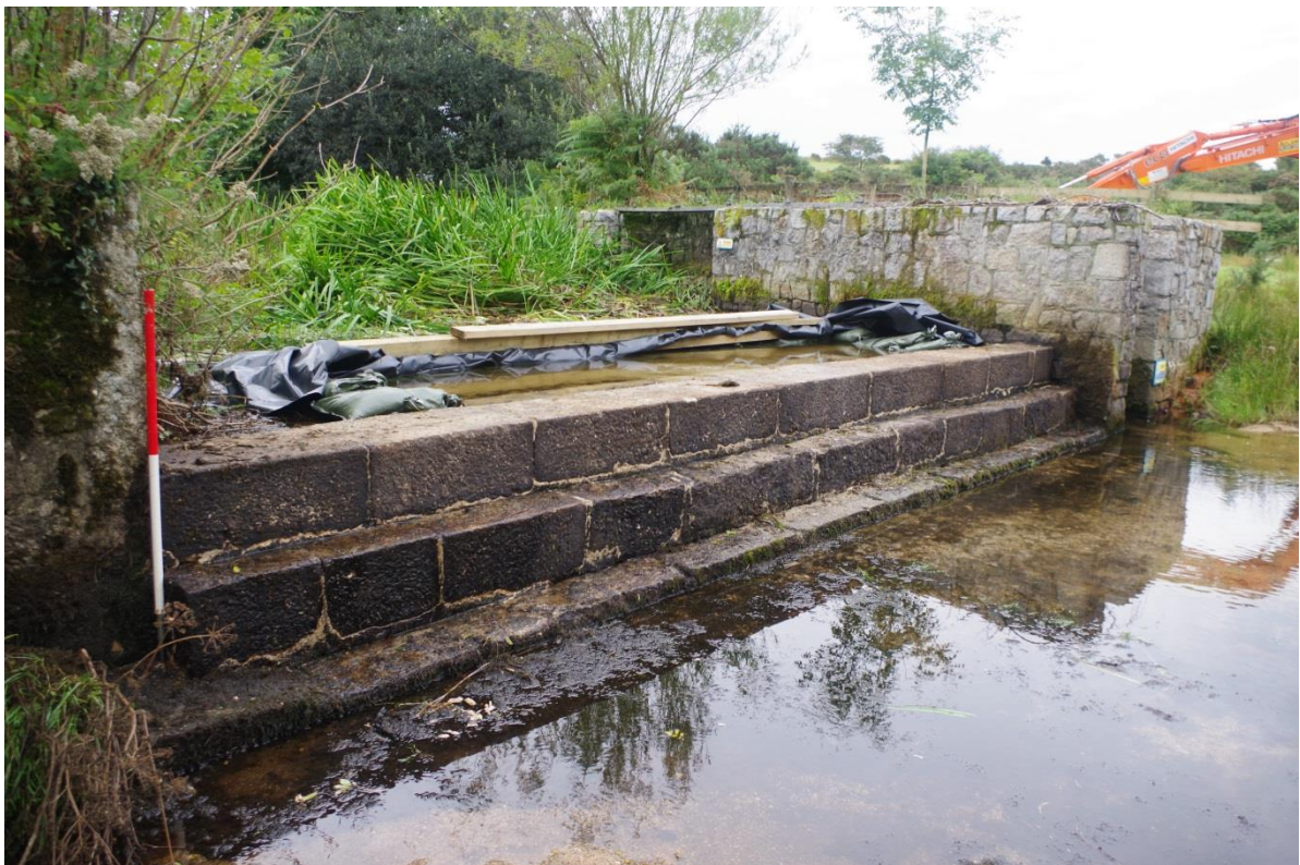
Fig 8 View of the weir and fish pass looking south-east.
