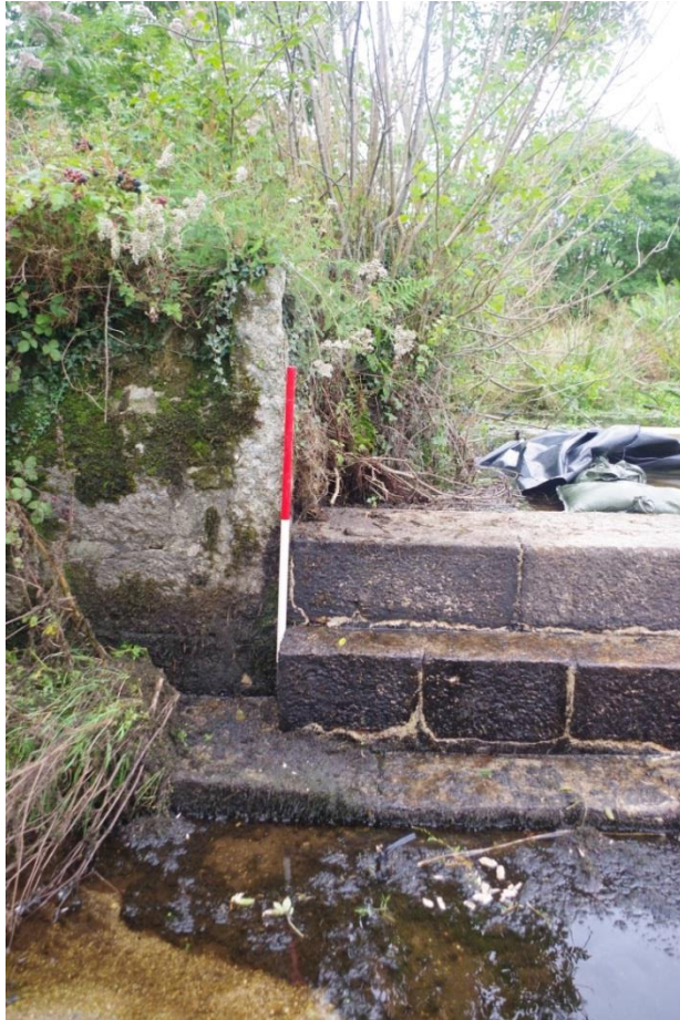
Fig 11 North end of the weir adjoining short length of wall.
