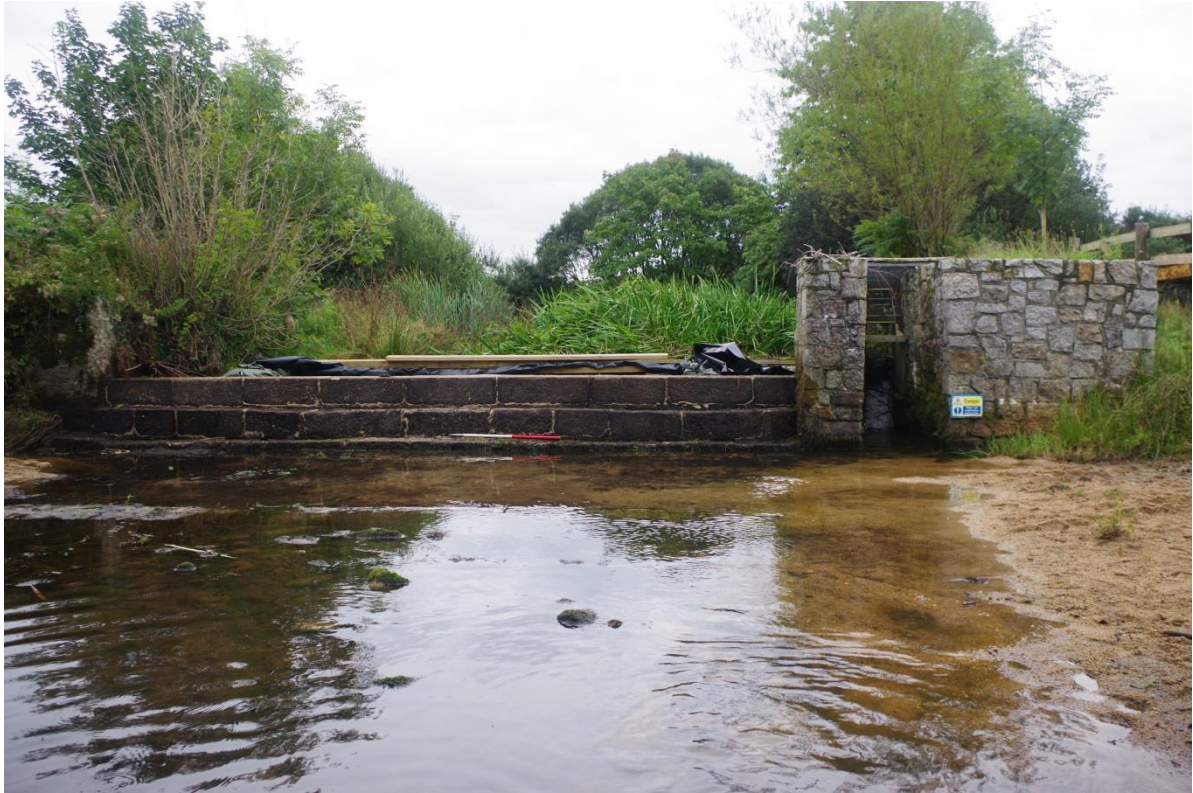
Fig 7 View of the weir and fish pass looking east.
