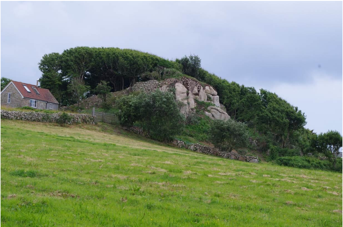
Fig 8.7 The keep of Ennor Castle, probably the only section of unaltered upstanding medieval masonry in Scilly, after vegetation clearance in June 2014 (photo: Cornwall Council).
