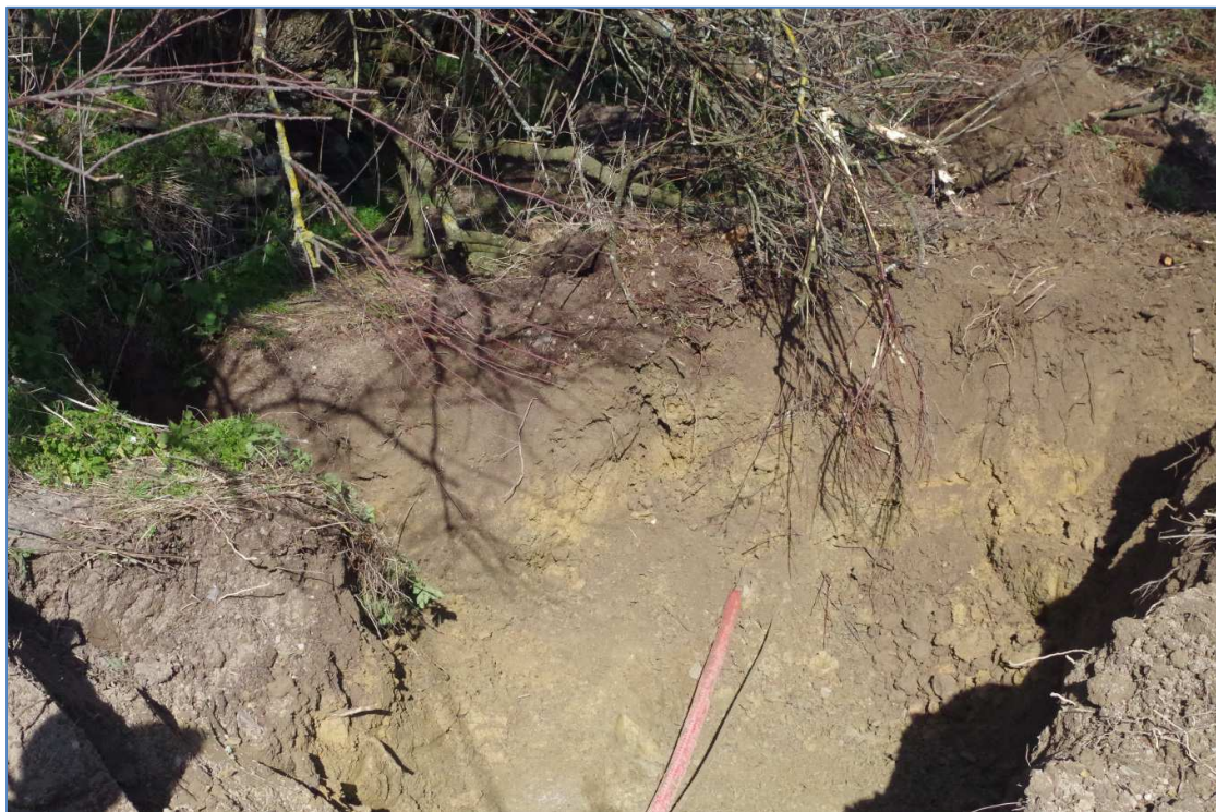
Fig 16 Cable pit in Field 7 showing sand at depth.
