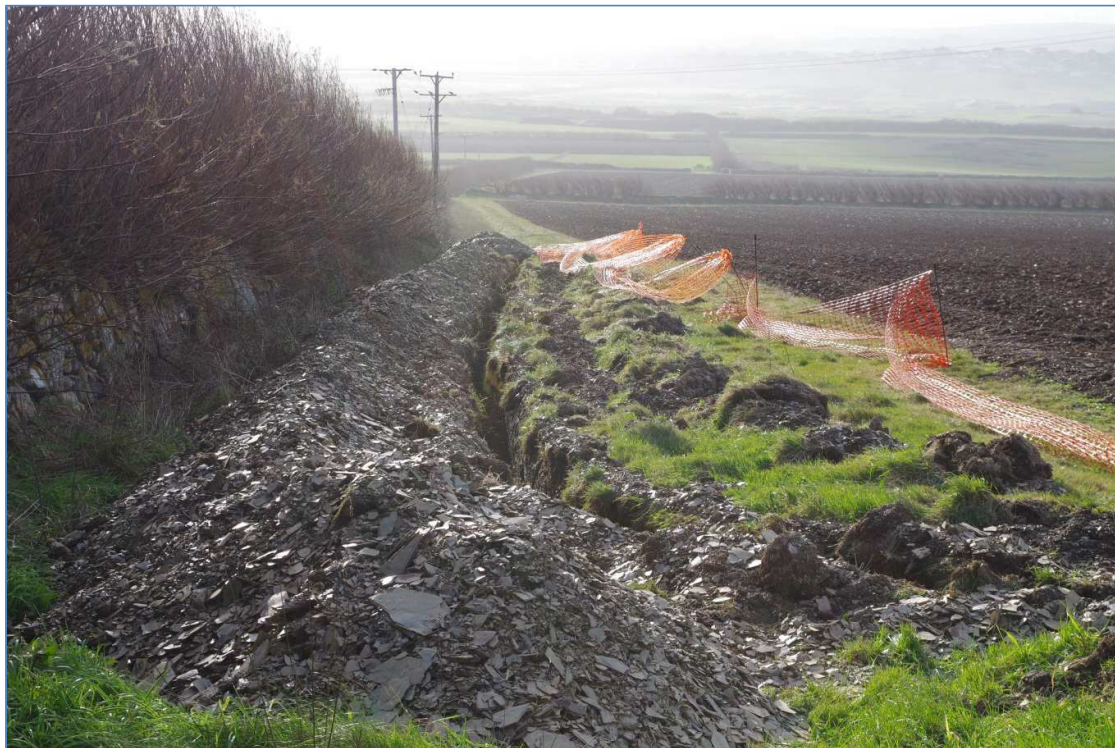
Fig 5 Trench in Field 1 looking southeast.
