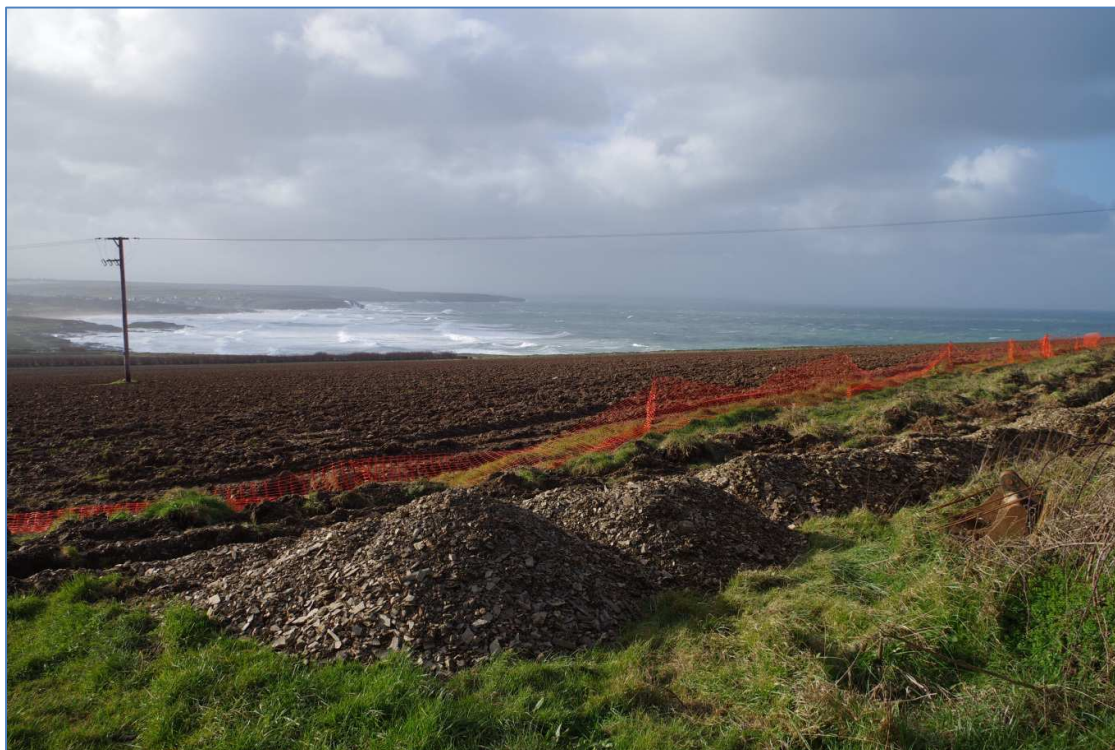
Fig 4 Trench along the north side of Field 1 looking southwest.
