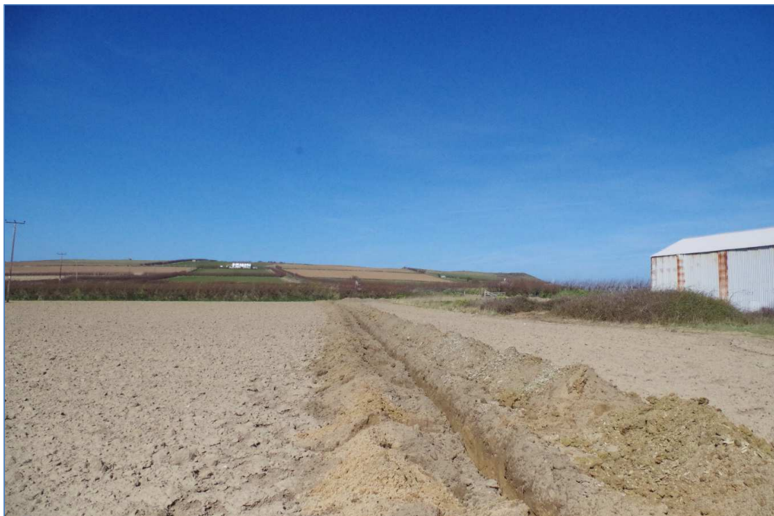
Fig 17 View along entire length of inspected pipeline, looking northwest.
