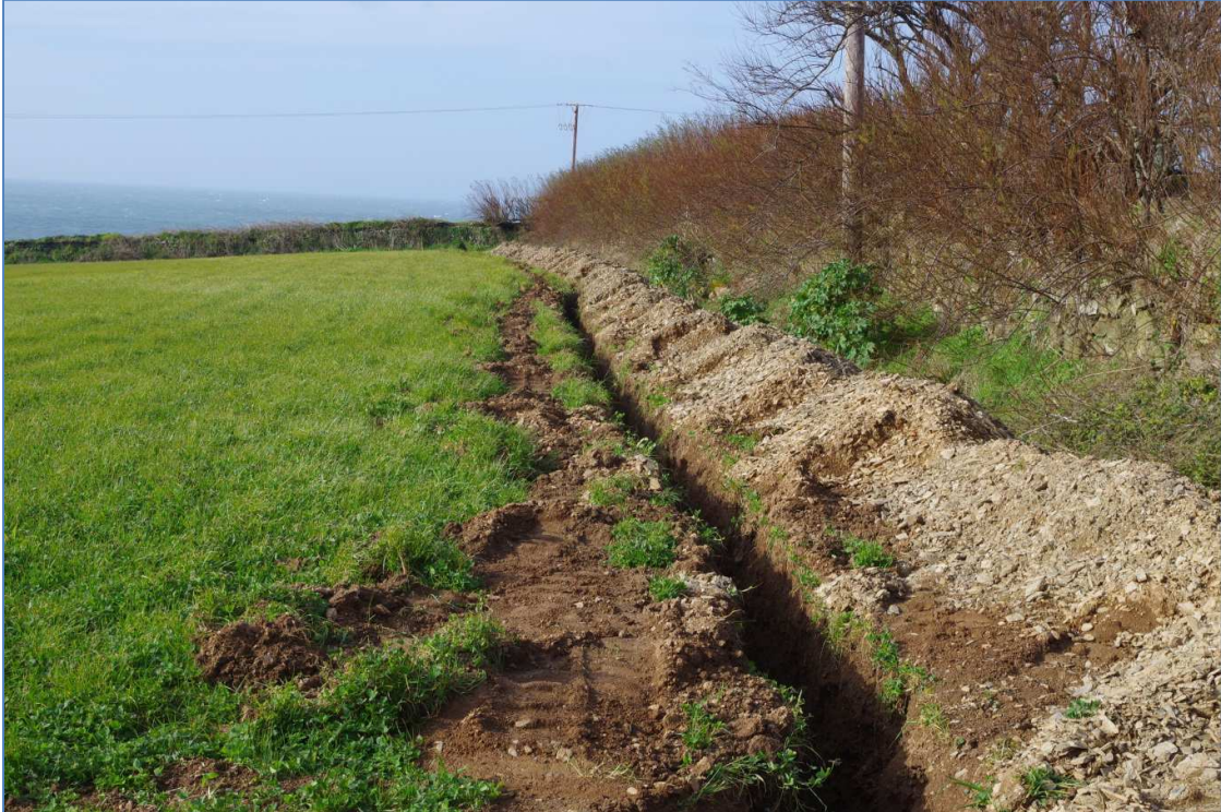
Fig 6 Trench across north side of Field 2 looking west.
