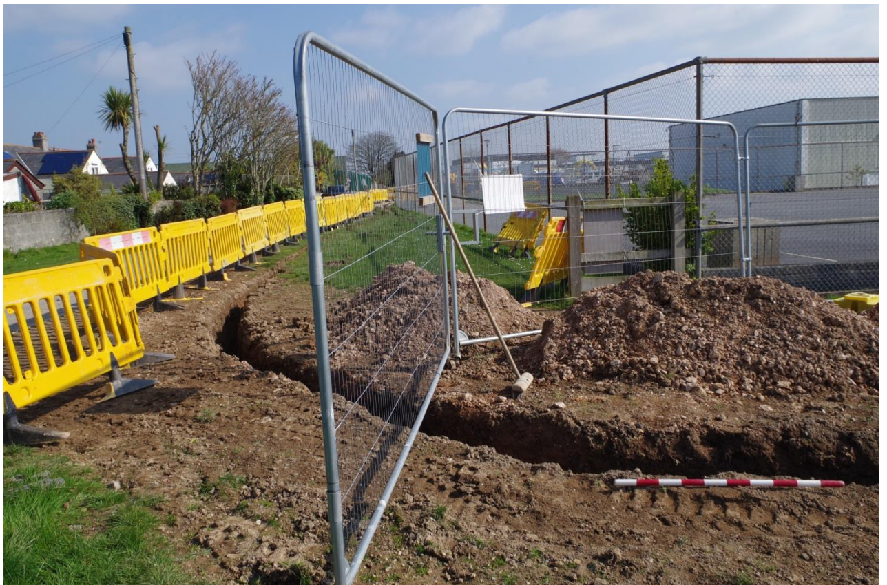
Fig 4 West corner of pipeline trench, looking NNE, with 1m scale.
