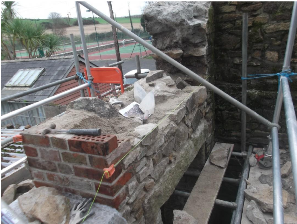
Fig 14. Reconstruction work in progress on the southern side of the upper floor wall opening.
