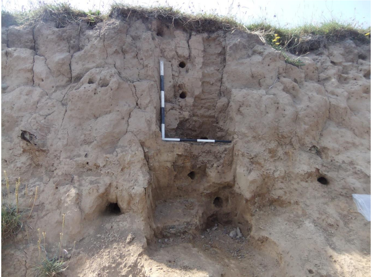
Fig 21 Cliff exposure following all sampling works, 50cm and 40cm scales, looking west.
