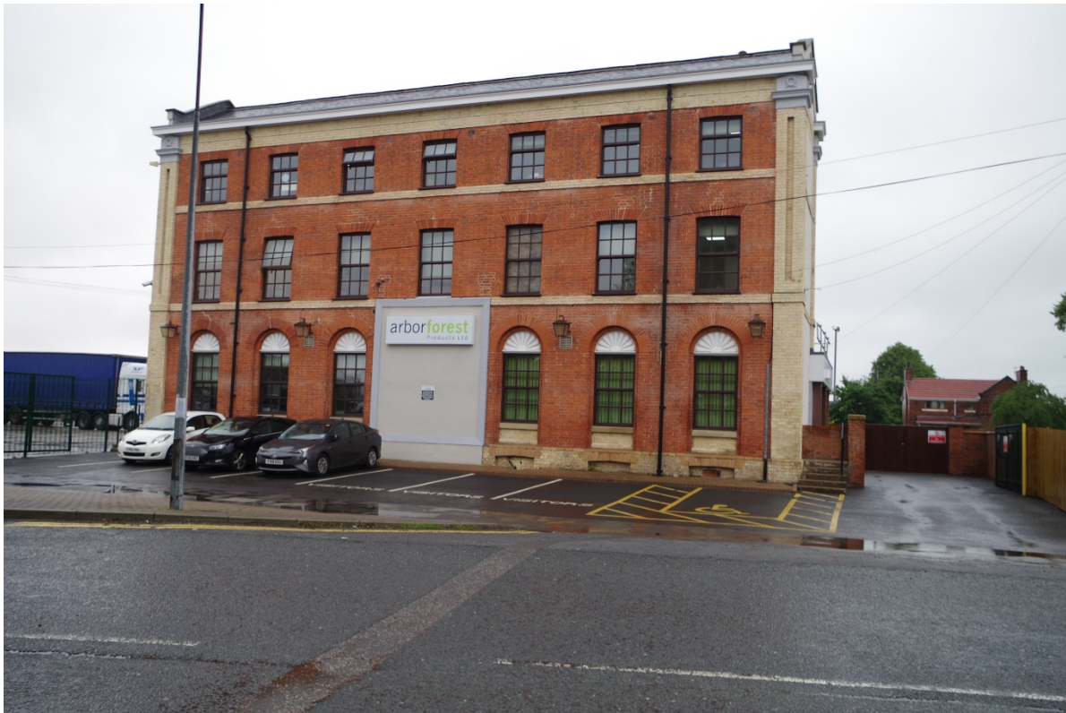
Figure 10.5 The Grade II Lincoln House Hotel, now dock offices, at New Holland, North Lincolnshire.
