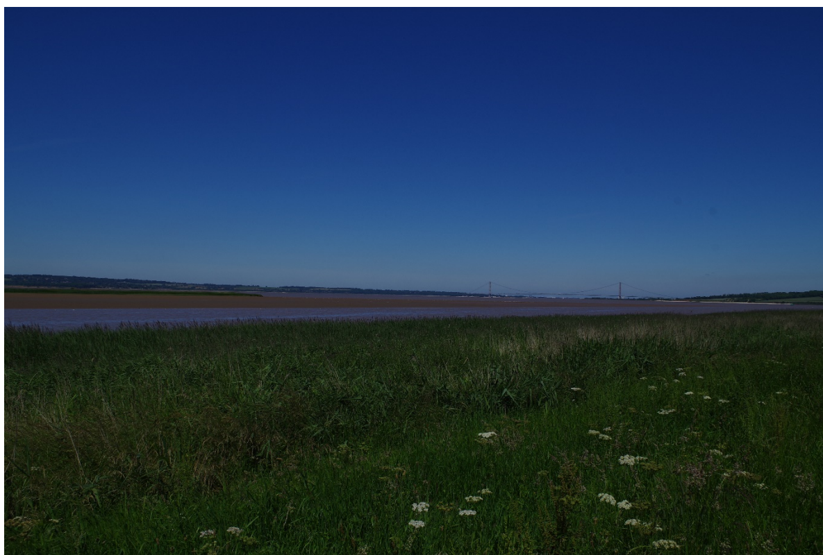
Figure 10.4 Looking across the South Channel to the eastern edge of Read’s Island from the flood defence bank near South Ferriby CEMEX plant. The area experiences high rates of coastal erosion and the flood defences here have recently been upgraded.
