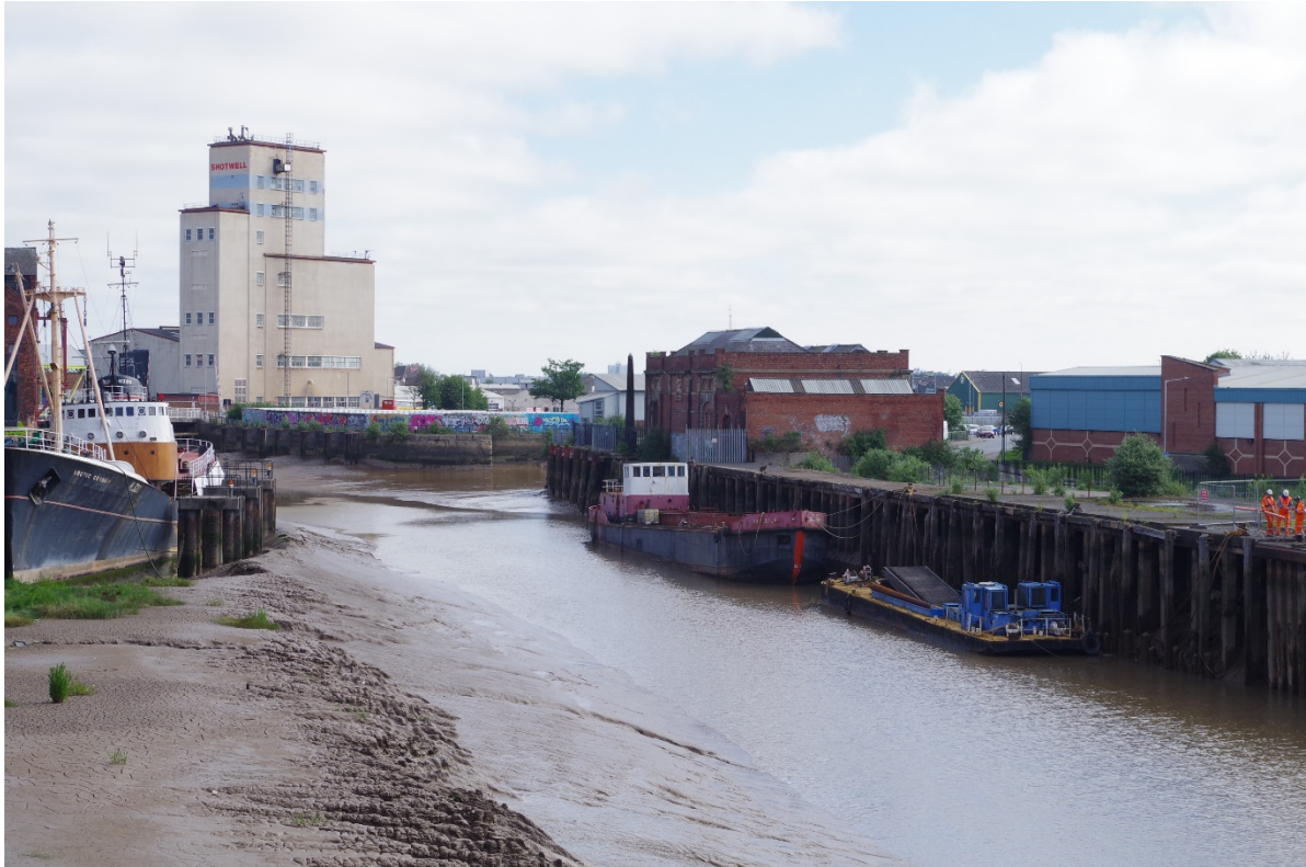
Figure 2.5 The River Hull. Looking from the Scale Lane footbridge up the river to the remaining mill at Clarence Street, Drypool, with the Arctic Corsair (former Hull based deep-sea trawler) (left) and the Grade II Listed former Trinity House buoy depot (NHLE 1197668) (right).
