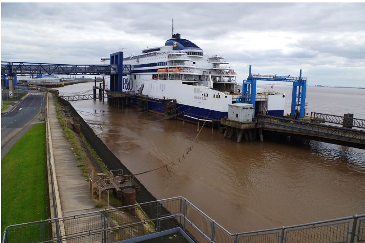
Figure 2.6 External Ro-Ro Ferry berth at King George Docks, Hull. (Photograph taken by CAU in 2015).
