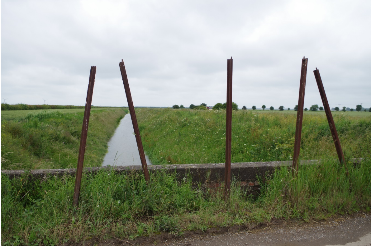
Figure 2.3 The drain at Salthaugh Clough, Near Stone Creek, Sunk Island.
