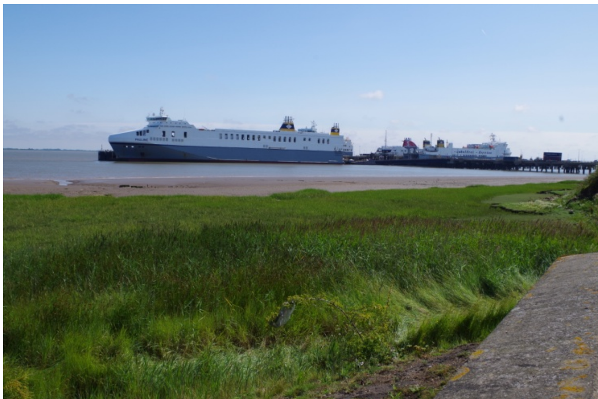
Figure 2.14 The Humber Sea Terminal. (Photograph taken by CAU in 2015).
