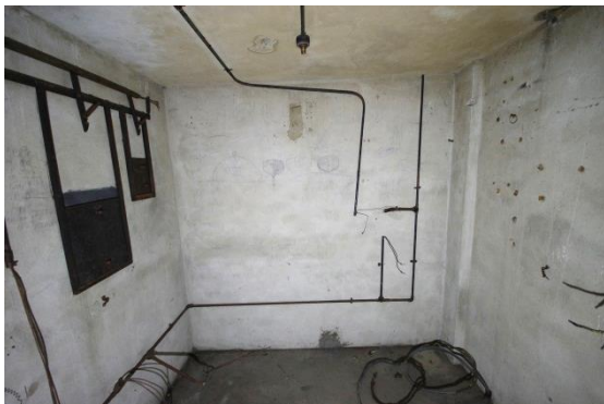
Fig 175 Room 25: Projection room looking east.
