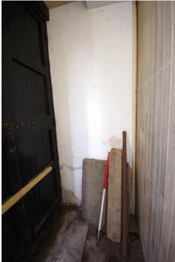
Fig 181 Room 26: Porch looking north.
