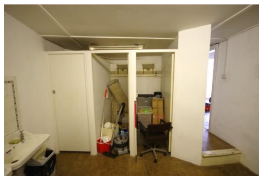
Fig 58 Room 4: Toilets (former ladies' toilets) looking south.
