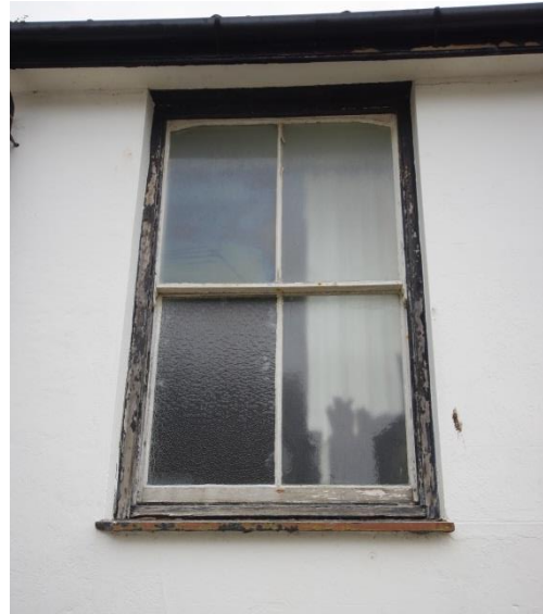
Fig 34 Four-paned sash (1911) in west elevation.
