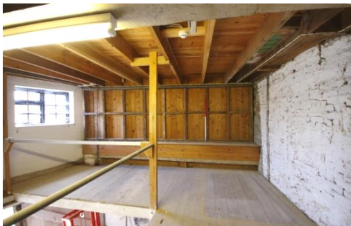
Fig 101 Room 11: Lower workshop (former store) looking south at mezzanine level.
