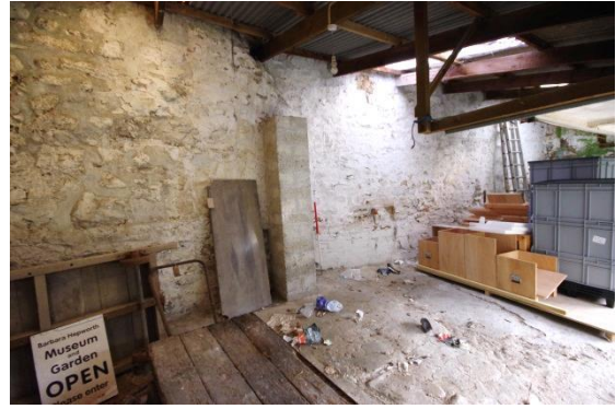
Fig 185 Room 27: Garage, north wall.
