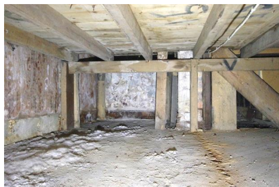
Fig 148 Room 21: Under stage looking east and showing skirting board.
