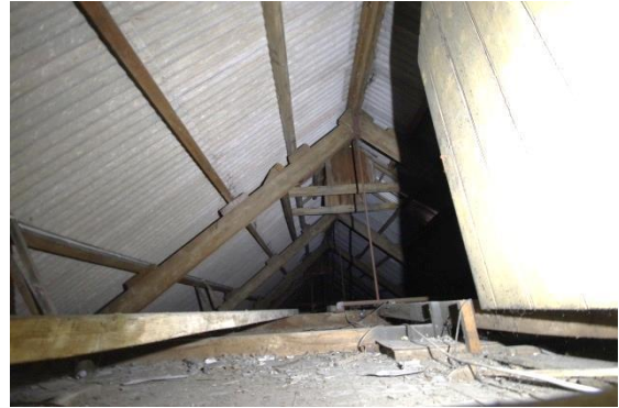
Fig 162 Room 23: Roof space above dancehall, north end looking south.
