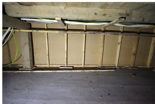
Fig 149 Room 21: Under stage looking south.
