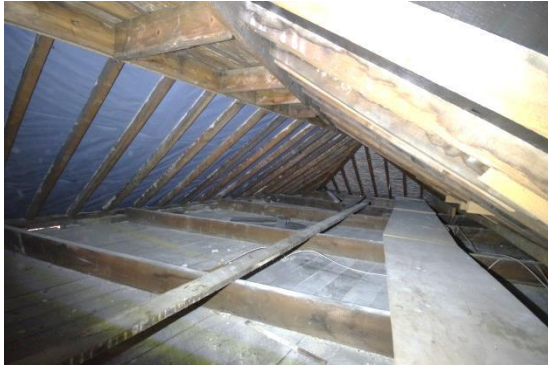
Fig 132 Room 15: Roof space above bar and canteen looking south.
