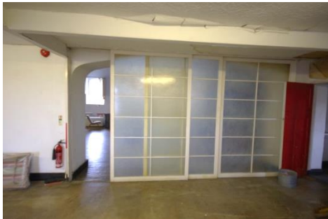
Fig 126 Room 14: Canteen area looking west to sliding doors.
