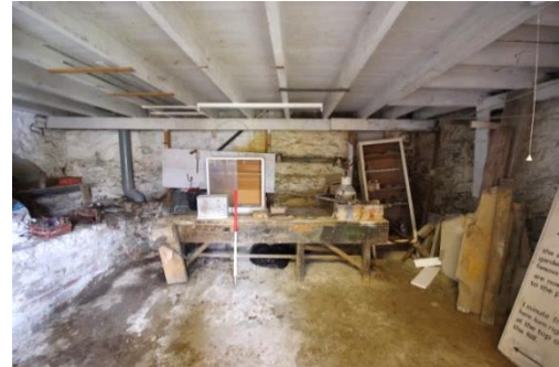
Fig 95 Room 11: Lower workshop (former store) looking north at ground floor level.
