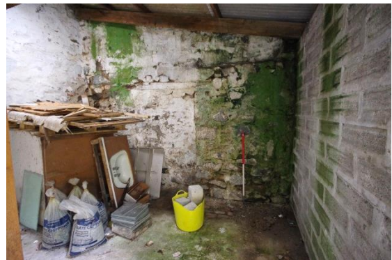
Fig 186 Room 27: Garage east wall.
