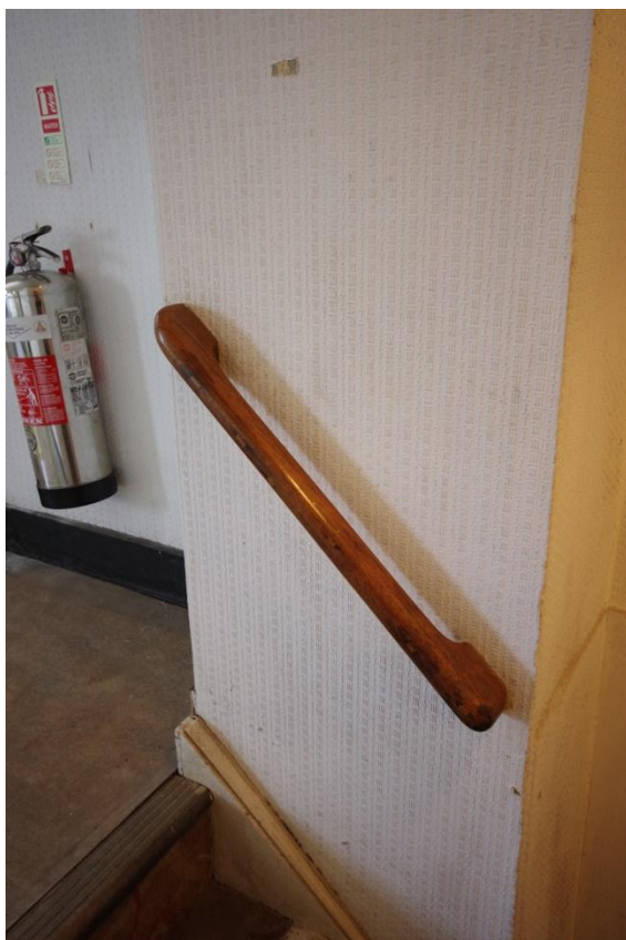
Fig 49 Room 2: Handrail at top of stairs.
