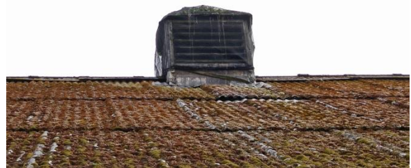
Fig 36 Detail of roof ventilator.
