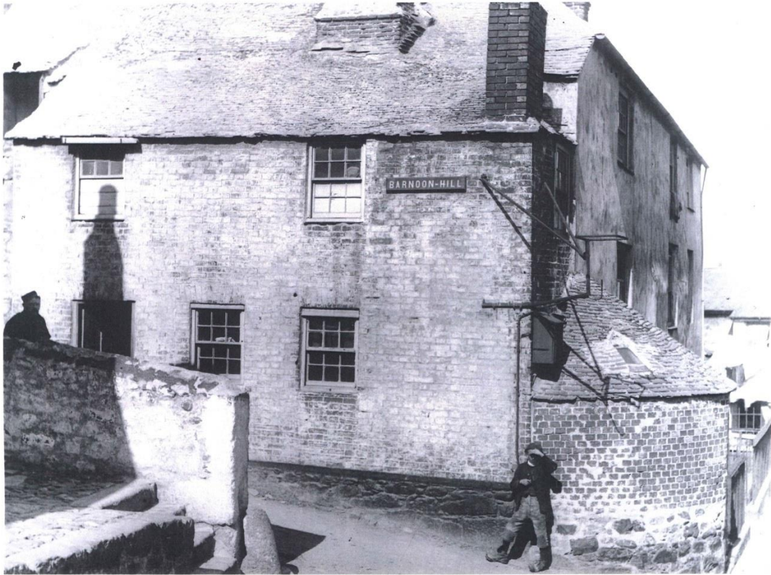
Fig 17 Photograph showing the brick workshop extension to the west with adjoining coal store and original frontage of the dwellings fronting Ayr Lane (Back Street) before 1898 (SIA REF: P13017).
