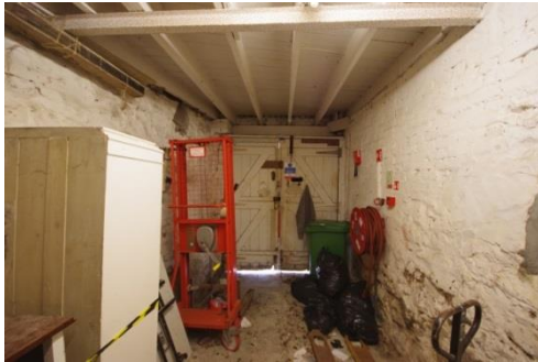
Fig 92 Room 10: Store looking south towards inserted double doors.
