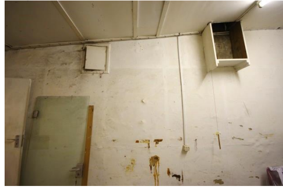
Fig 73 Room 6: Store looking west.
