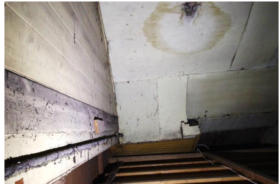
Fig 163 Room 23: Roof space above dancehall, above stage looking west.
