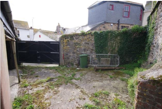
Fig 182 Room 27: Yard looking south.
