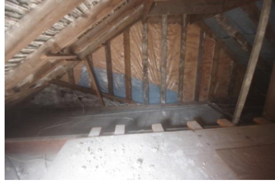
Fig 128 Room 15: Roof space above bar and canteen north end looking north.
