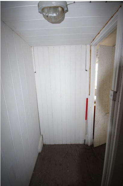
Fig 111 Room 12: Landing showing blocked entrance to truncated stairs.
