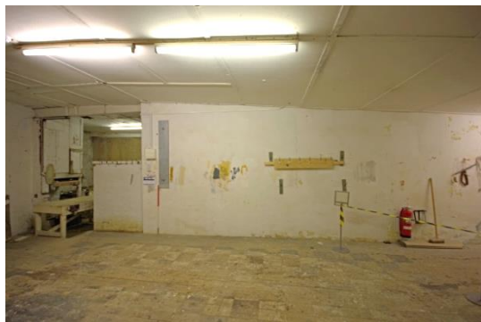
Fig 76 Room 7: Upper workshop looking east.
