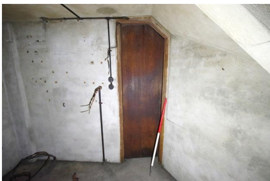
Fig 176 Room 25: Projection room looking south.
