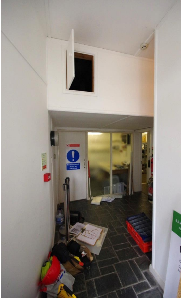
Fig 43 Room 1: Entrance lobby looking north.
