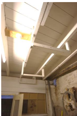
Fig 94 Room 10: Store ceiling with storage racks.
