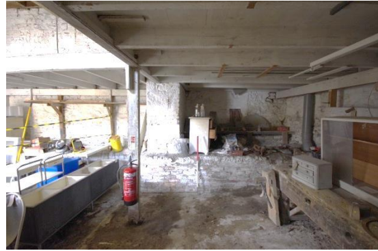
Fig 103 Room 11: Lower workshop (former store) looking west at north end of ground floor level.
