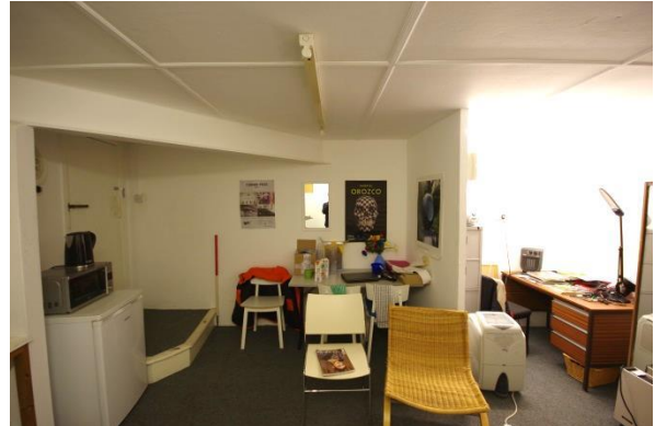
Fig 50 Room 3: Staff room (former men's toilets) looking north.
