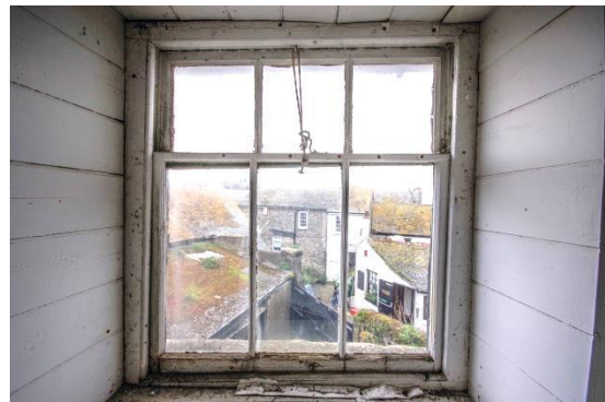
Fig 116 Room 13: Conservative room, 19 th century sash window.
