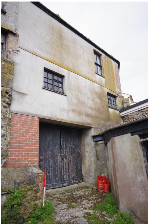
Fig 39 Central part of East elevation.
