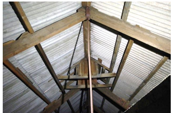
Fig 164 Room 23: Roof space above dancehall, north end looking south.
