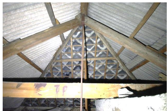
Fig 165 Room 23: Roof space above dancehall, south end looking south to hip.
