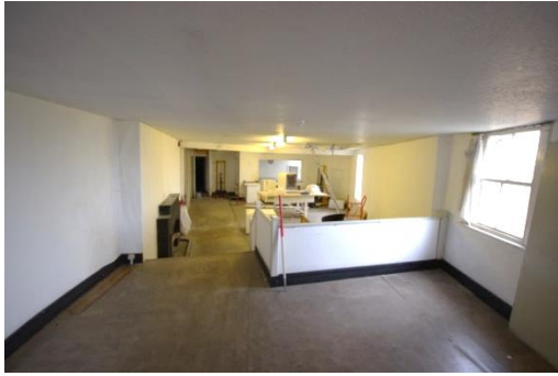
Fig 117 Room 14: Bar and canteen (former small hall) looking north.
