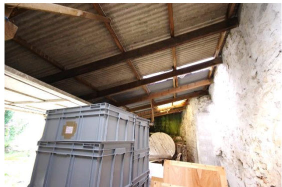
Fig 187 Room 27: Garage lean-to roof structure.
