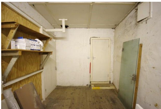
Fig 72 Room 6: Store looking south.
