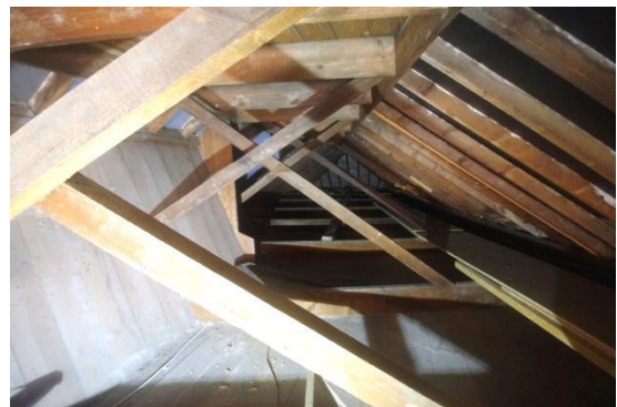
Fig 131 Room 15: Roof space above bar and canteen looking south.
