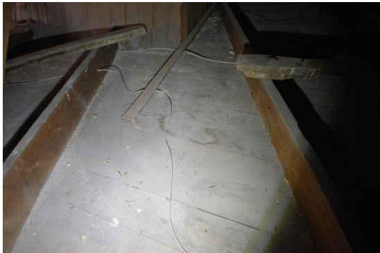
Fig 133 Room 15: Roof space above bar and canteen showing ceiling boards.
