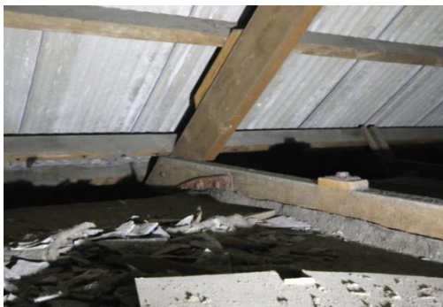
Fig 166 Room 23: Roof space above dancehall, south end showing iron straps.
