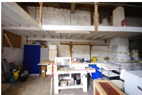
Fig 102 Room 11: Lower workshop (former store) looking west at south end of ground floor level.
