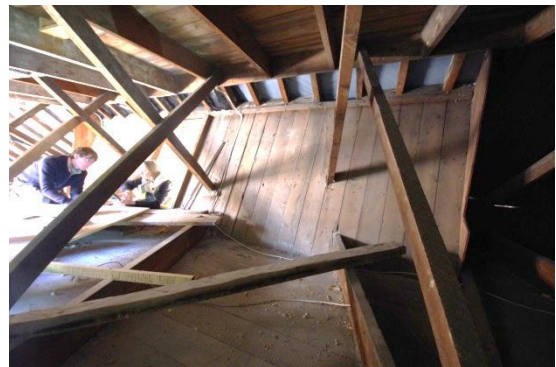
Fig 130 Room 15: Roof space above bar and canteen looking east.
