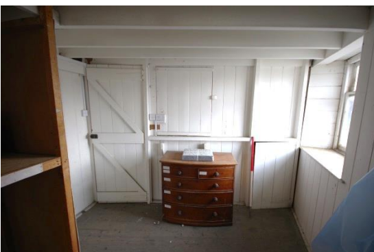
Fig 112 Room 13: Conservative room looking north.
