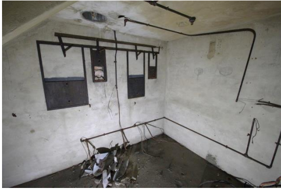
Fig 173 Room 25: Projection room looking north-east.
