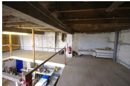
Fig 104 Room 11: Lower workshop (former store) looking west at mezzanine level.
