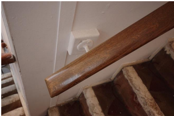
Fig 48 Room 2: Original handrail.
