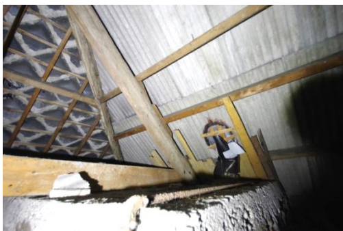
Fig 168 Room 23: Roof space above dancehall, area above Projection room.
