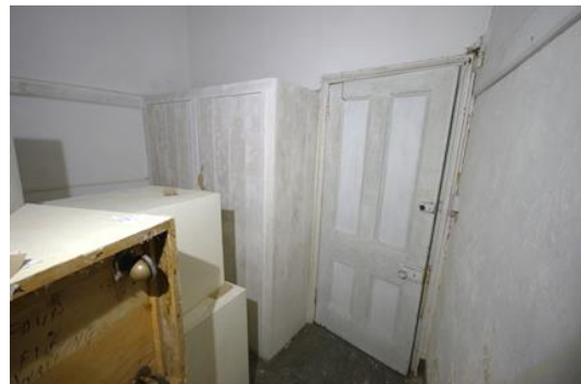
Fig 141 Room 19: Former dressing room/cloakroom looking south-west.
