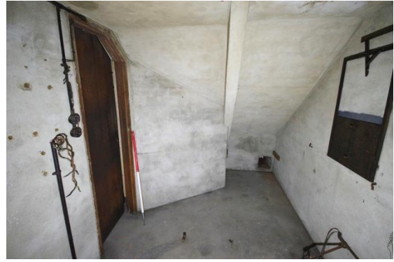
Fig 177 Room 25: Projection room looking west.
