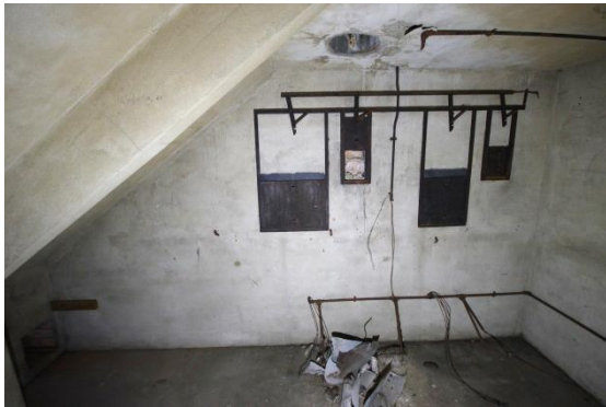
Fig 174 Room 25: Projection room looking north.
