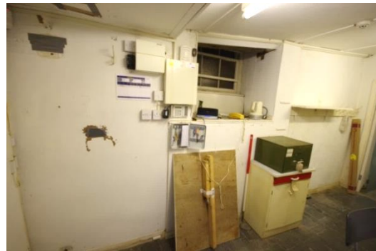
Fig 67 Room 5: Office (former box office and cloakroom) looking west.
