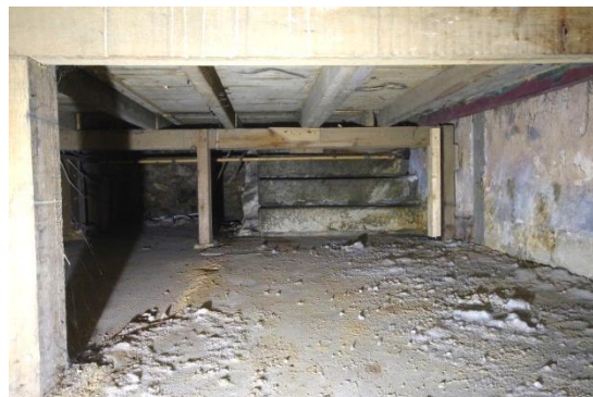
Fig 146 Room 21: Space beneath stage looking west towards granite steps.
