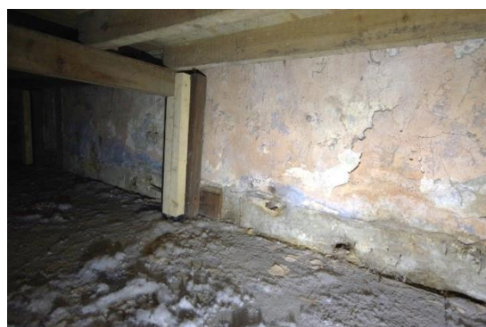
Fig 147 Room 21: North wall under stage showing removed skirting.
