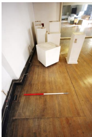
Fig 161 Room 22: Dancehall, blocked opening for former staircase to the south-east.
