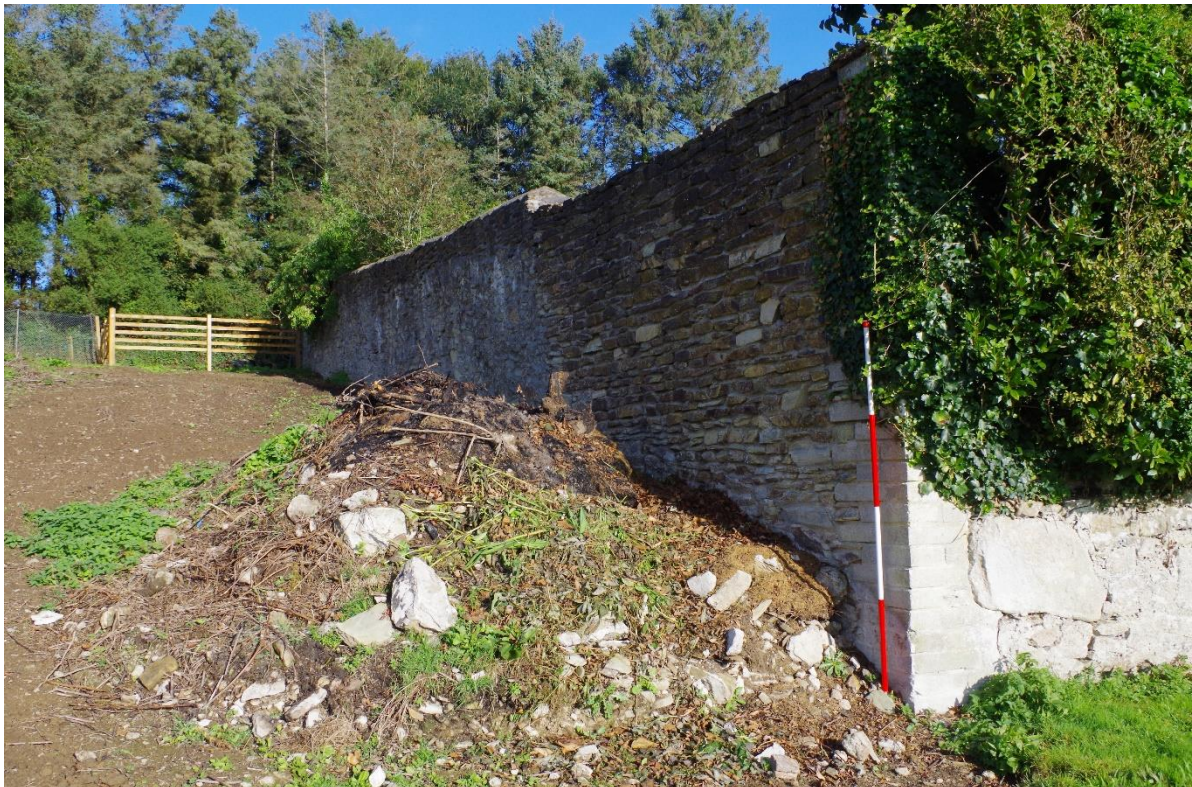
Fig 18 Boundary Wall of 187 Charlestown Road.
