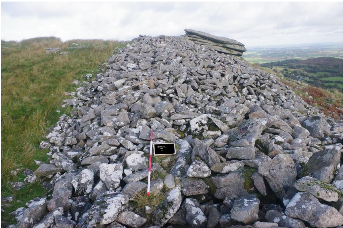
Fig 25 Feature 11 - possible exposed wall core, eastern rampart, southern enclosure.
