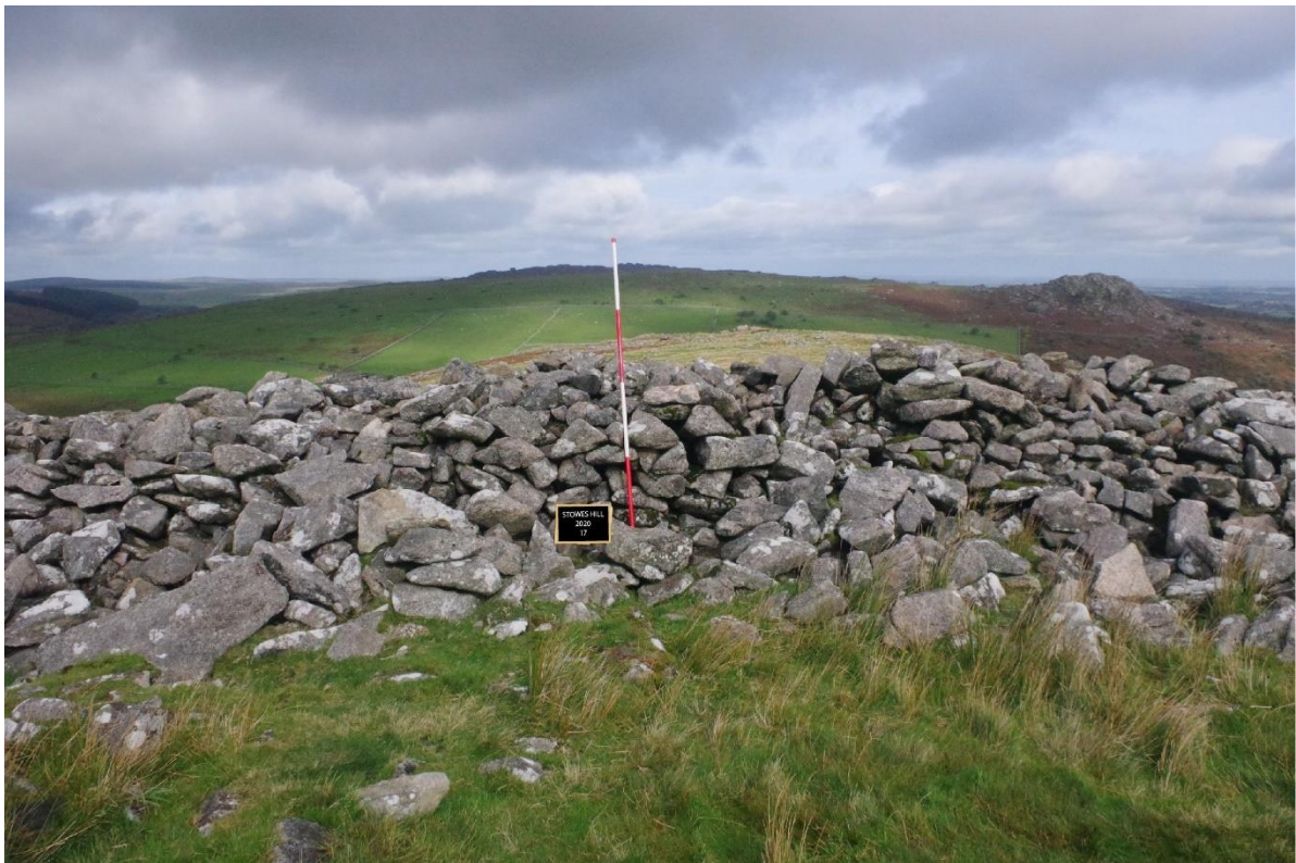
Fig 31 Feature 17 – exposed wall core, northern rampart, southern enclosure.
