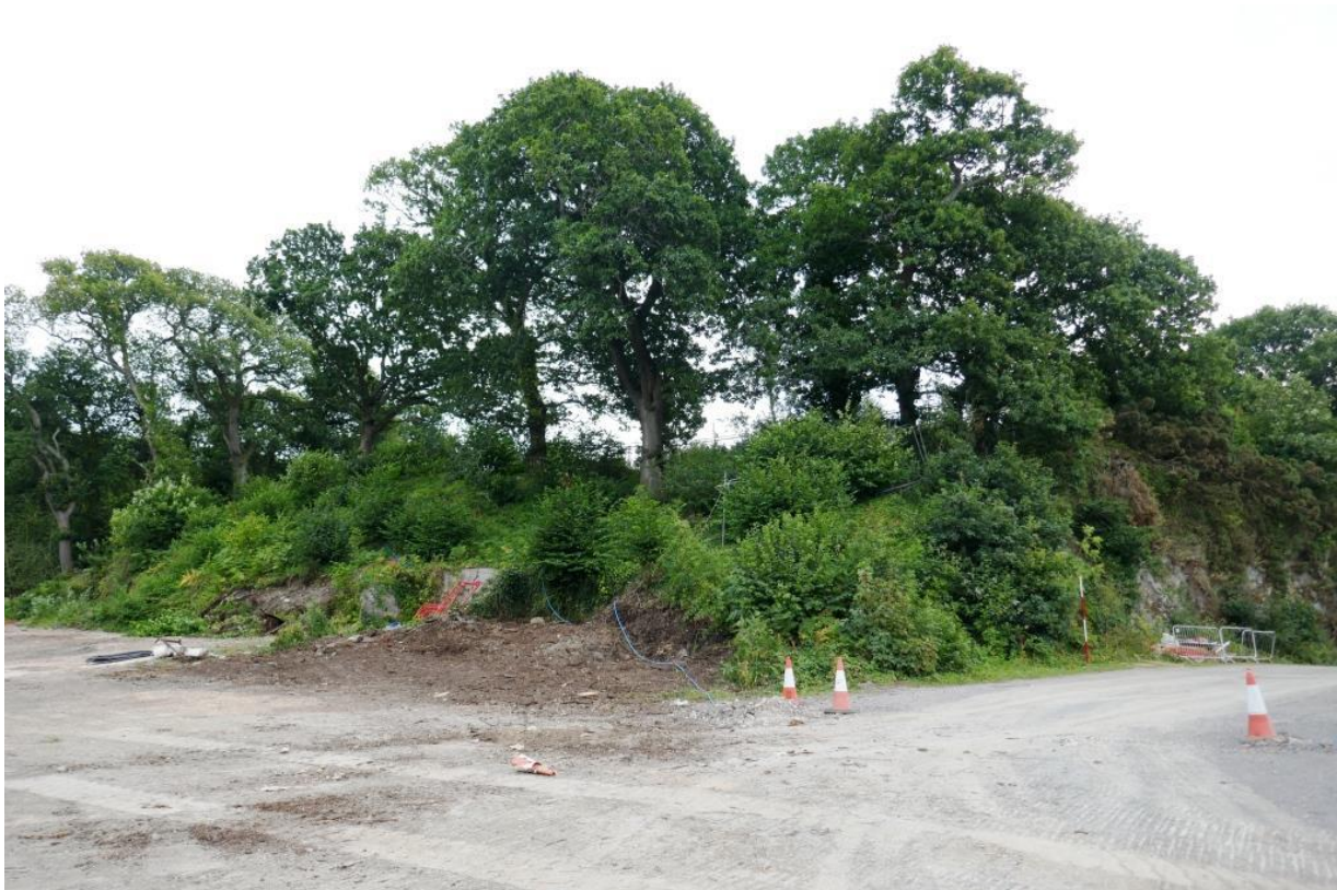
Fig 29 Old railway cutting west of new car park area (right) with trees on the ridge above mapped in 1895 and possibly indicated also in 1838 (2m scale).
