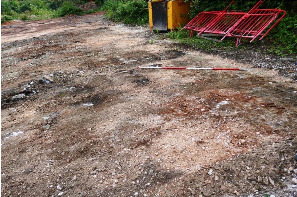
Fig 30 View from north west of south side of made ground stripped of gravel (112), showing infill (113), very stony clay with coal (2m scale).
