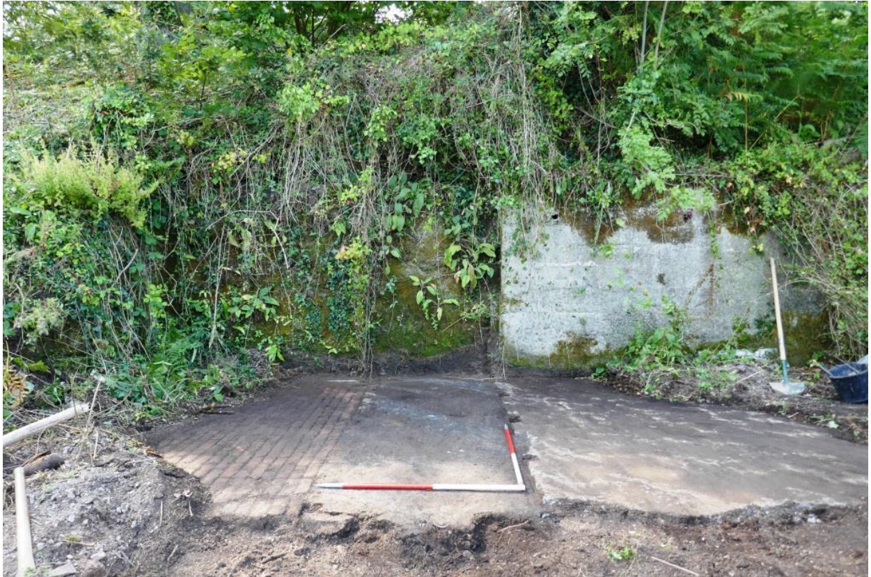
Fig 22 South east building 5, with floor features 103-107 partly exposed (1m scales). Removal of fill (101) and (102) was not all monitored as asbestos was present.
