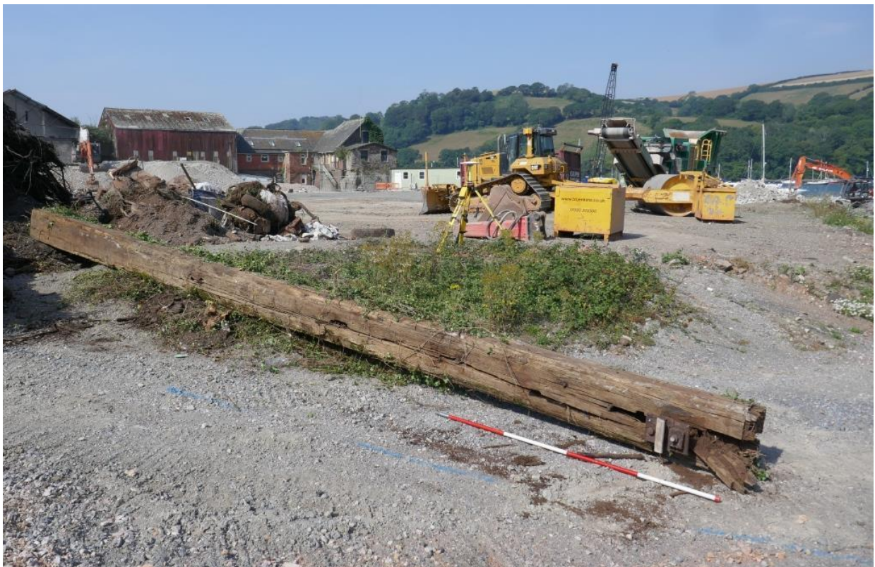
Fig 33 Large timber, possibly from crane, used to face modern creek infill (2m scale).
