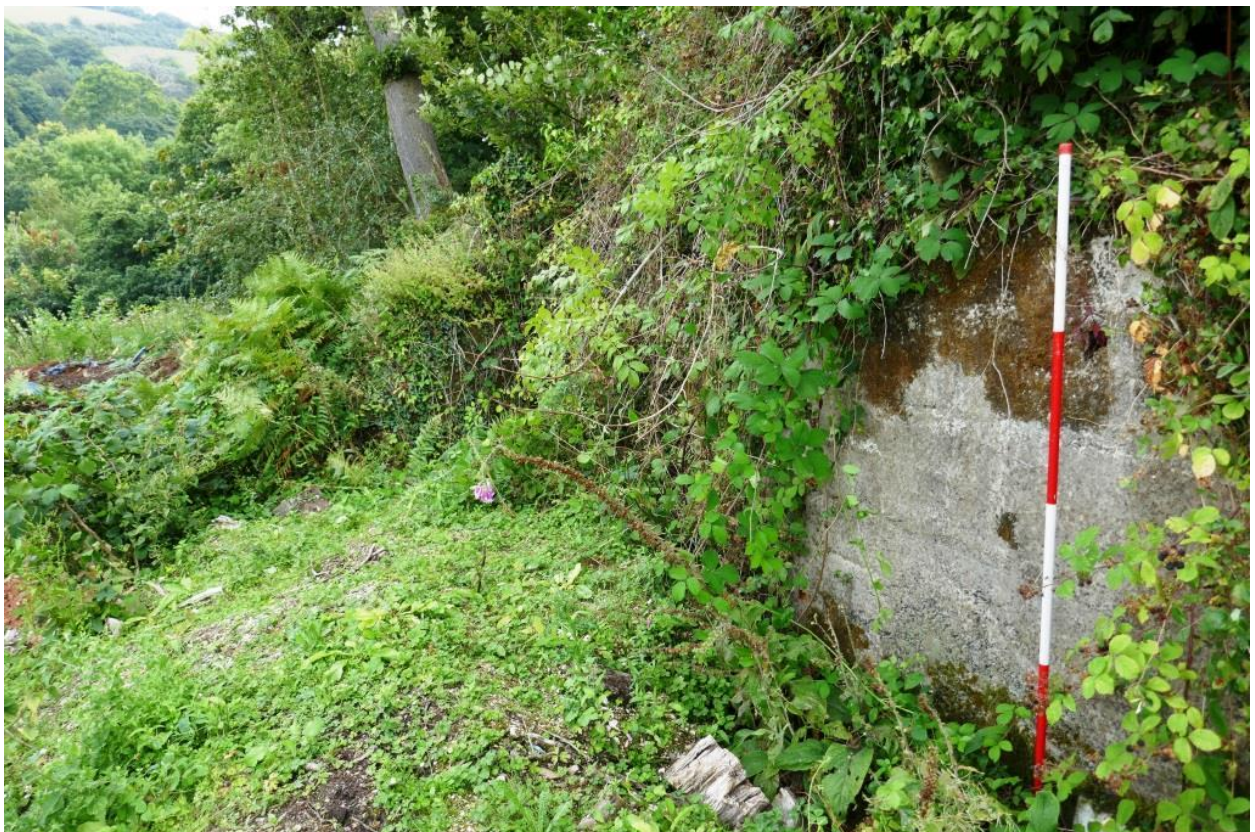
Fig 21 Building at site 5, looking east from centre prior to works, showing fill (101) (2m scale).
