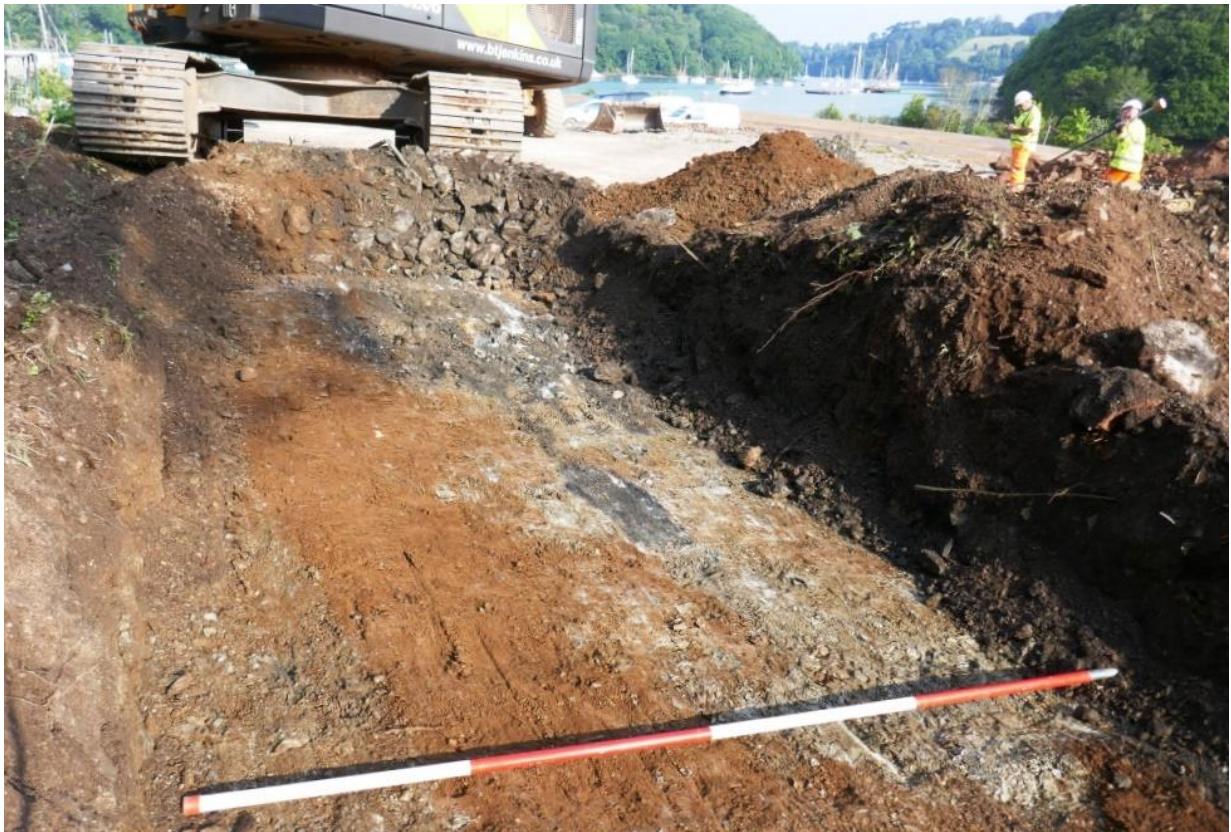
Fig 32 Stripping of modern fill on south east quarter of site in progress (looking north west). The base of the trench shows the thick stony coally pinkish layer (113), the most recent apart from the surface gravel, right; orangey clay (114), centre; and greyish stony layer (115), left; all spread successively into the creek (2m scale).
