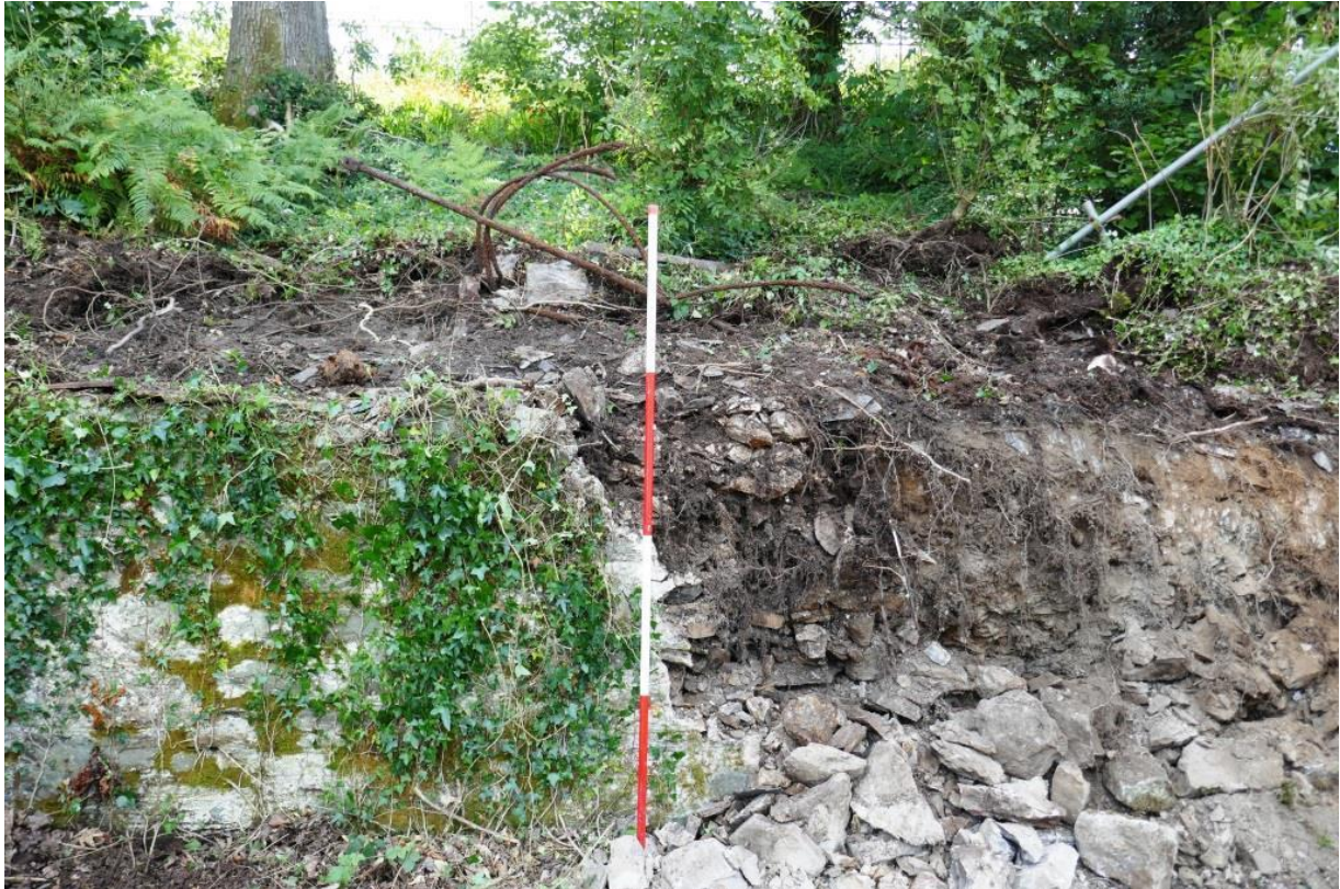
Fig 28 West part of south west building at site 7 during removal of its south wall where the building platform had been cut into the bedrock and the space between wall and cut later filled with debris dumped down the scarp including asbestos (2m scale).
