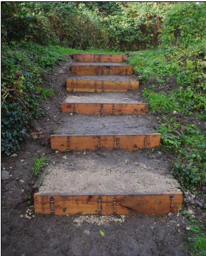
Fig 9 A-7, completed installation of steps.
