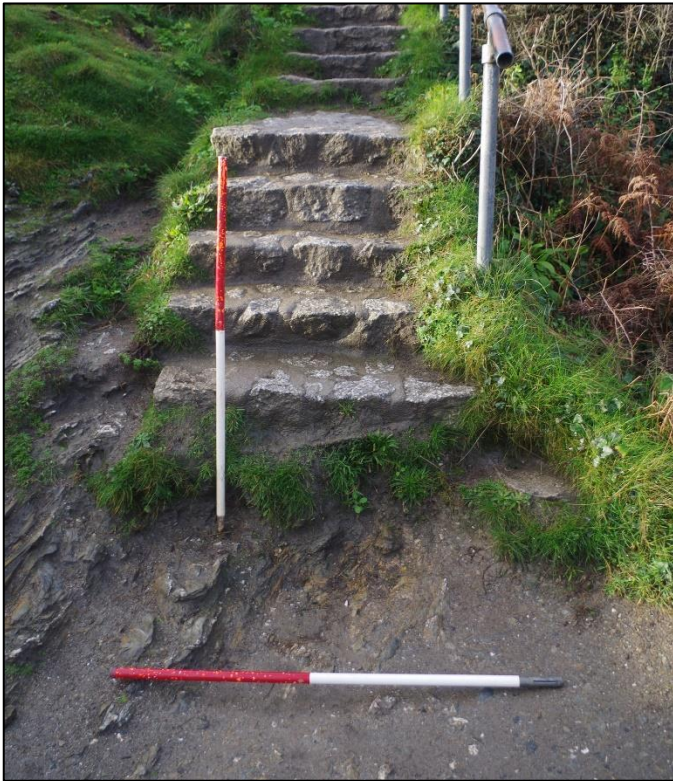
Fig 6 A-3, pre groundworks.
