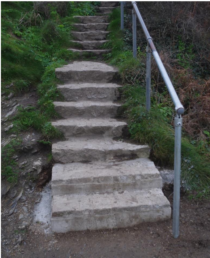
Fig 7 A-3, completed installation of steps.
