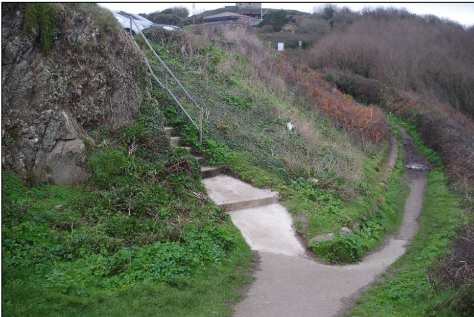
Fig 3 A-1 post installation of steps.
