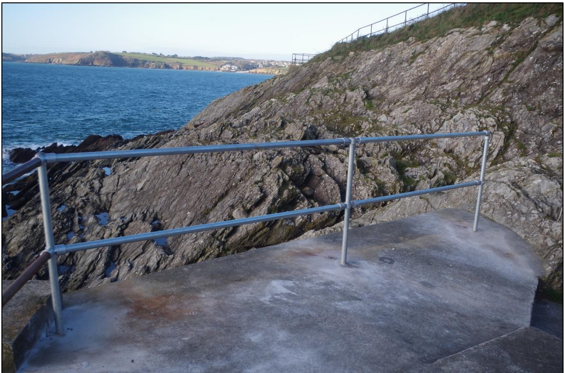
Fig 5 A-2, completed installation of steps.
