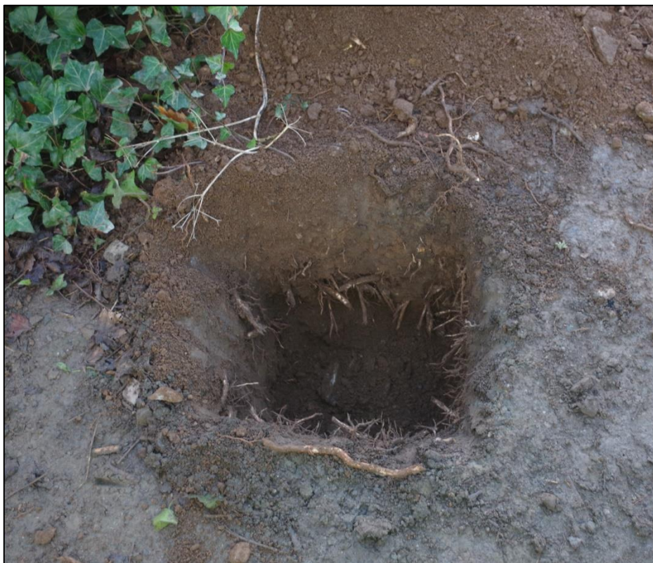
Fig 11 A-8, post hole for timber fencing.
