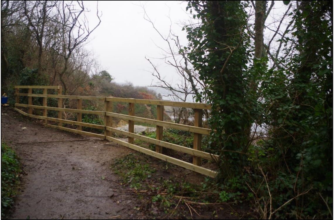
Fig 12 A-8, completed timber fencing.
