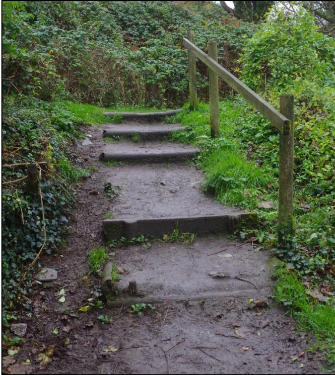
Fig 8, A-7, pre groundworks.
