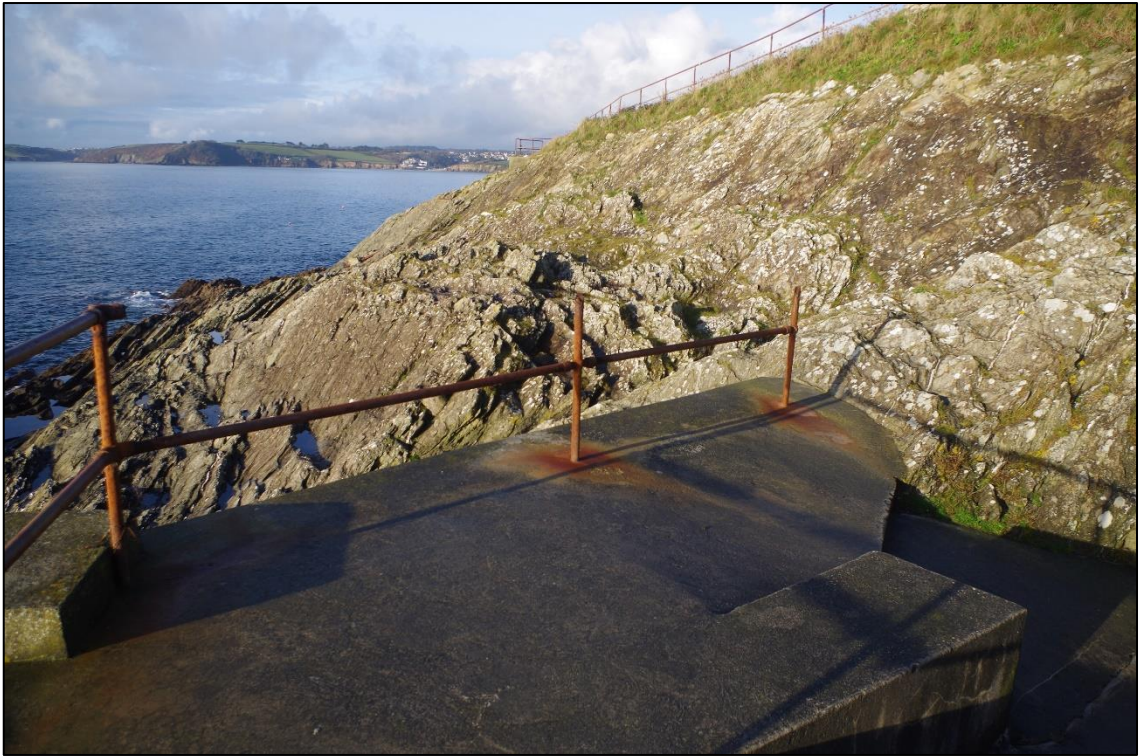
Fig 4 A-2, pre groundworks.
