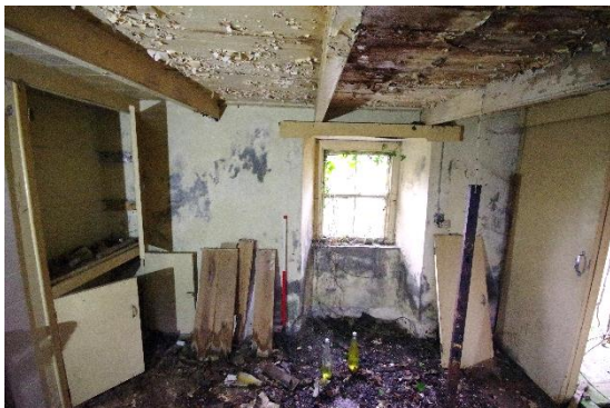
Fig 25 Room 4 south wall.
