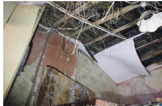
Fig 28 Room 8 east wall.
