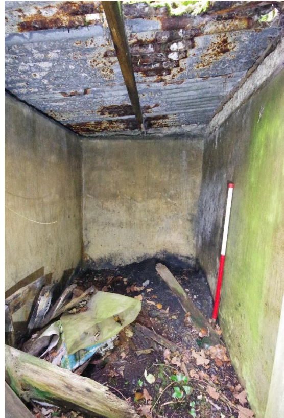
Fig 36 Room 7 lean-to looking east.
