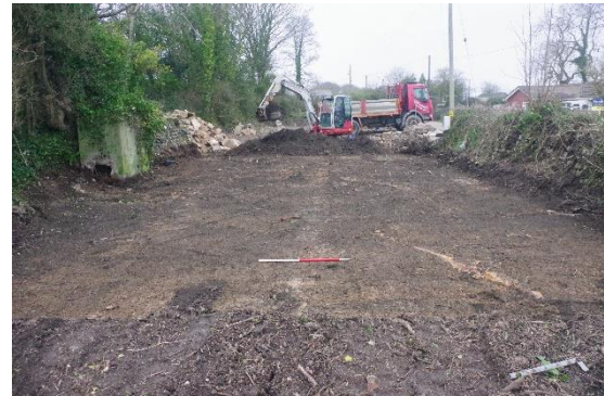
Fig 51 Topsoil stripped area to the south of the house, looking north.
