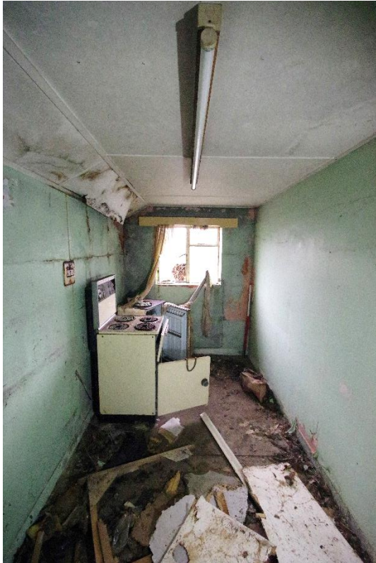
Fig 34 Room 6 looking south.
