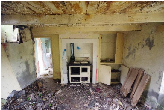
Fig 24 Room 4 east wall.
