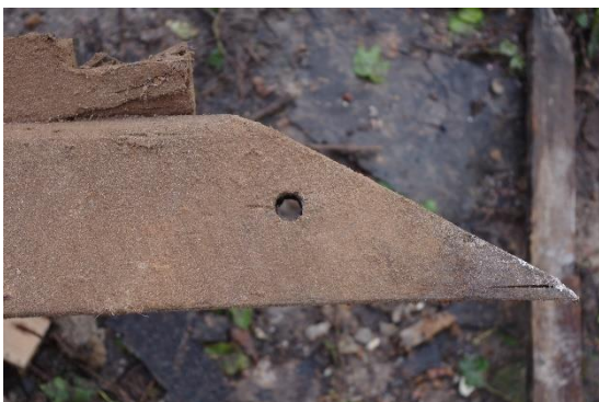
Fig 45 Pegged hole at base of principal rafter.
