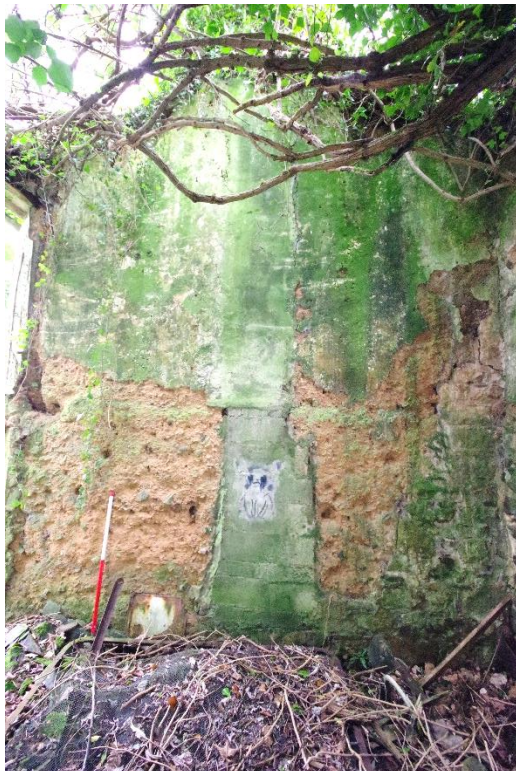
Fig 16 Room 1 east wall. Showing inserted concrete flue.
