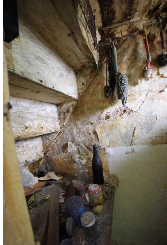
Fig 32 Room 5 west wall and underside of phase 2 staircase.
