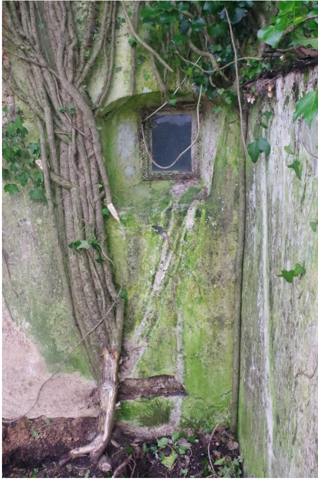
Fig 13 Blocked phase 1 back door opening.
