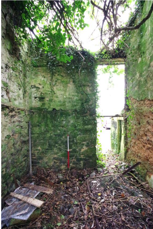
Fig 15 Room 1 north wall.
