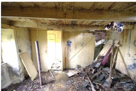
Fig 26 Room 4 west wall showing phase 2 and 3 matchboard panelling for the staircase.
