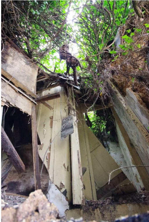
Fig 30 Room 8 west wall.
