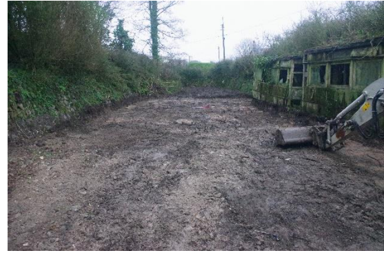
Fig 50 Topsoil stripped area to the north of the house, looking north.
