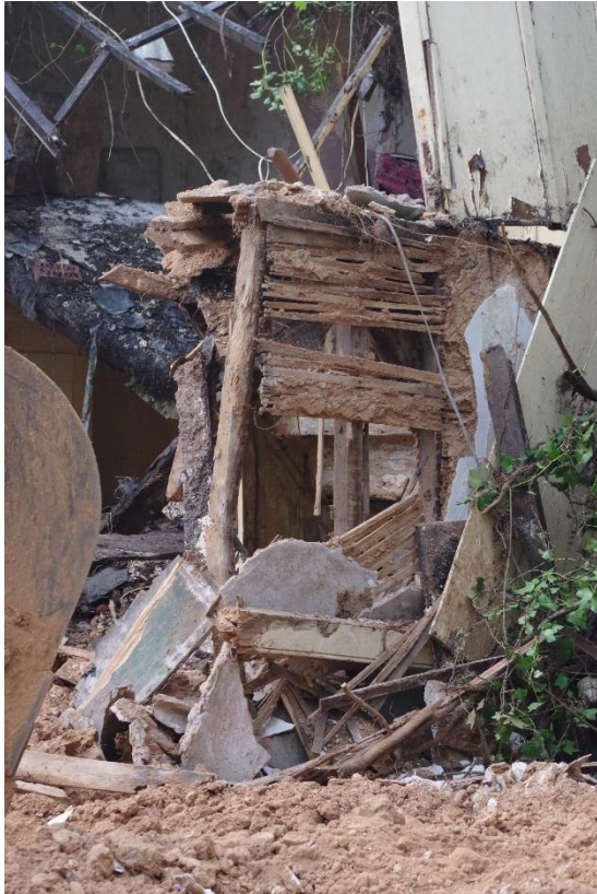
Fig 43 Lath and earth plaster partition wall between rooms 2 and 5 showing position of blocked door opening.
