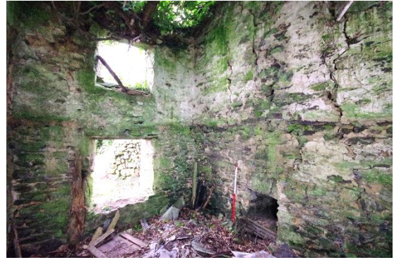
Fig 17 Room 1 south and west walls.
