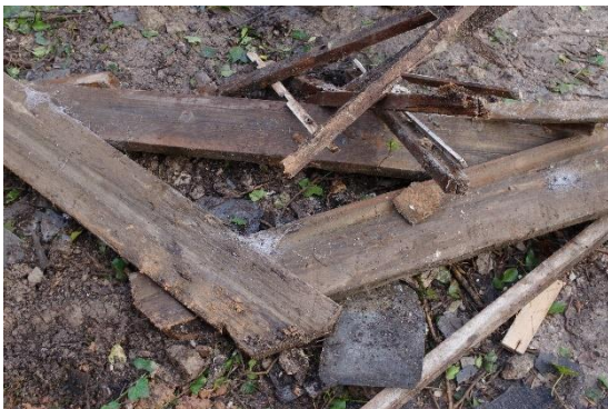
Fig 44 Phase 1 lap-jointed collar roof truss.
