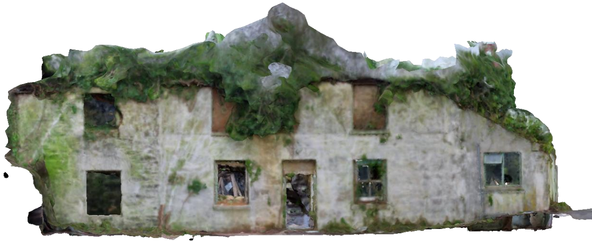
Fig 57 Orthophoto of south (front) elevation.
