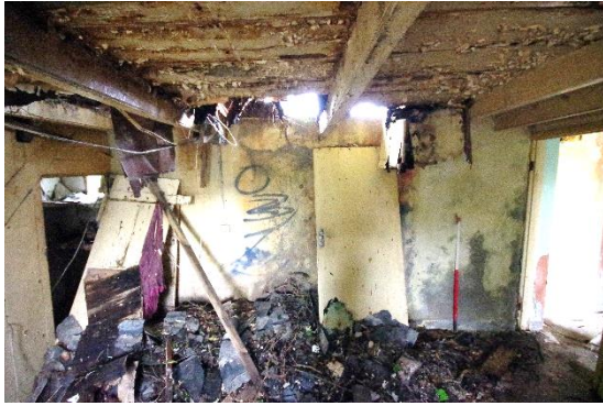
Fig 23 Room 4 north wall.
