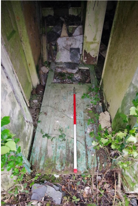
Fig 9 Detached early-mid 20th century front door in south elevation.
