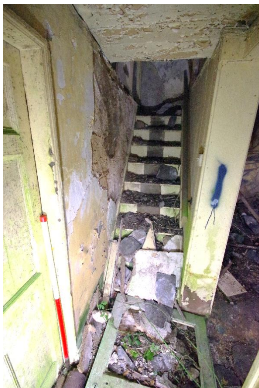
Fig 20 Room 3 staircase looking north from entrance hallway (former cross passage).
