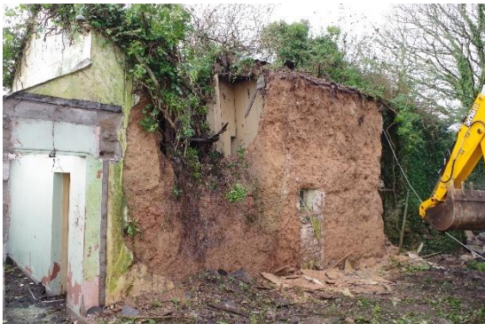
Fig 40 North elevation of phase 1 house stripped of render.
