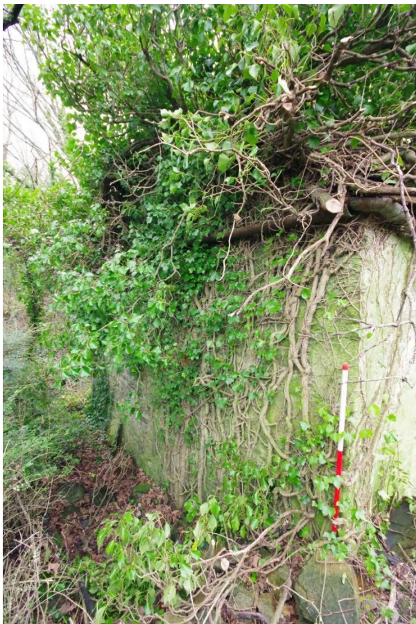
Fig 10 West elevation of western phase 2 extension, showing iron/steel guttering.
