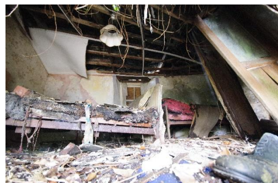
Fig 29 Room 8 south wall.
