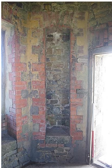
Fig 29 Interior north east wall with blind window.
