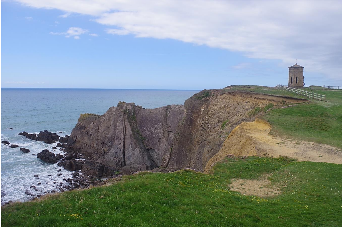
Fig 10 Storm tower looking north east.
