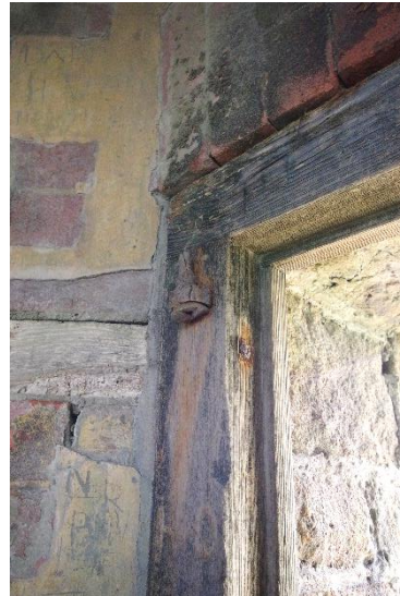
Fig 43 Detail of iron pintle on door frame.
