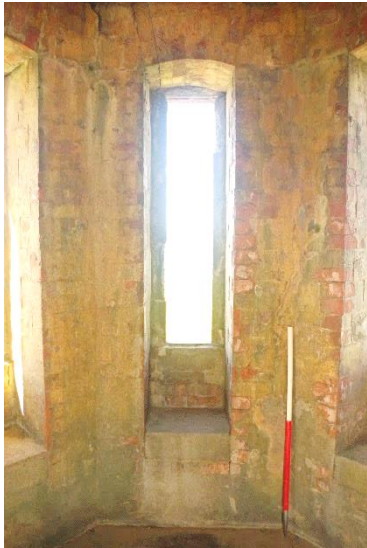
Fig 33 Interior west wall.
