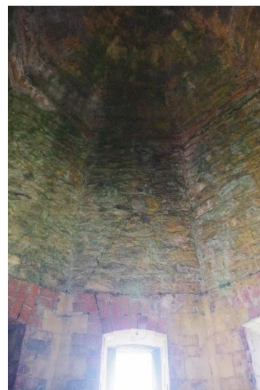
Fig 38 Interior south wall above window.
