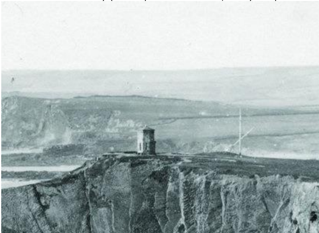
Fig 8 Cropped photograph of the first Storm Tower, taken between 1850-1879 by local photographer Harry Thorn, © Thorn and Thorn. It shows the tower without a plinth at the base or a cross on the roof but does show the signalling flagstaff close by.
