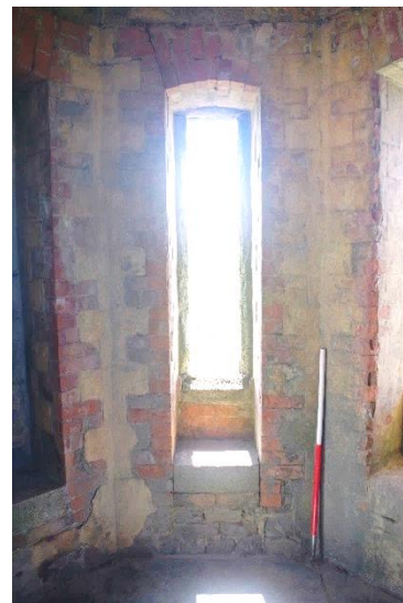
Fig 37 Interior south wall.
