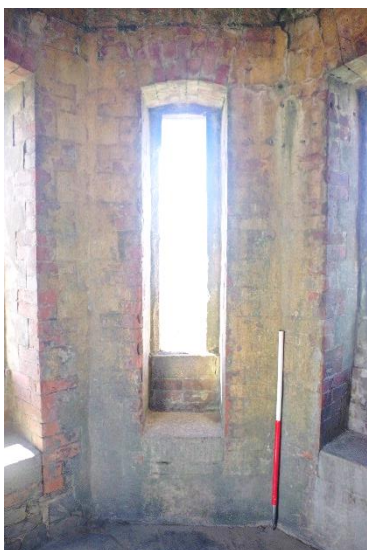
Fig 35 Interior south west wall.
