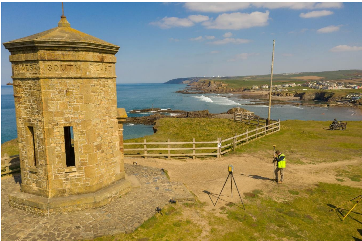
Fig 11 Storm tower during measured survey looking north (supplied by Mark Trewin).
