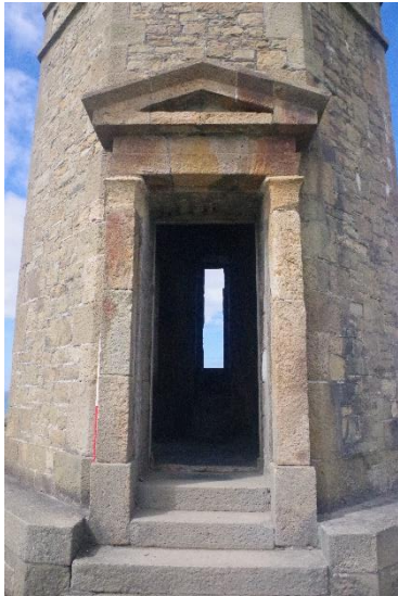
Fig 15 Detail of doorway in east elevation.
