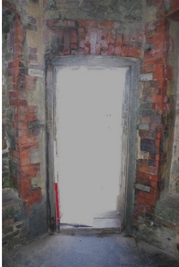
Fig 27 Interior east wall and door frame.
