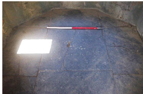
Fig 25 Interior slate flagstone floor looking west.
