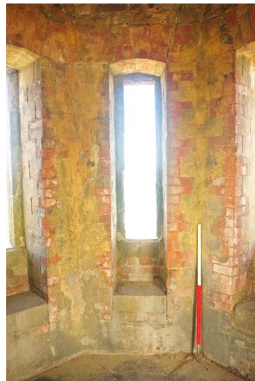
Fig 32 Interior north west wall.
