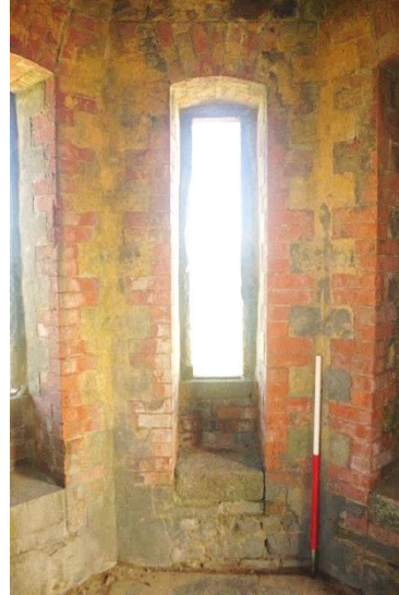
Fig 30 Interior north wall.
