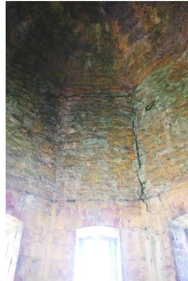
Fig 36 Interior south west wall above window.
