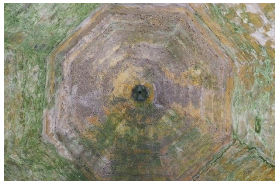
Fig 26 Interior shuttered concrete domed ceiling.
