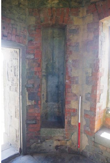
Fig 39 Interior south east wall.
