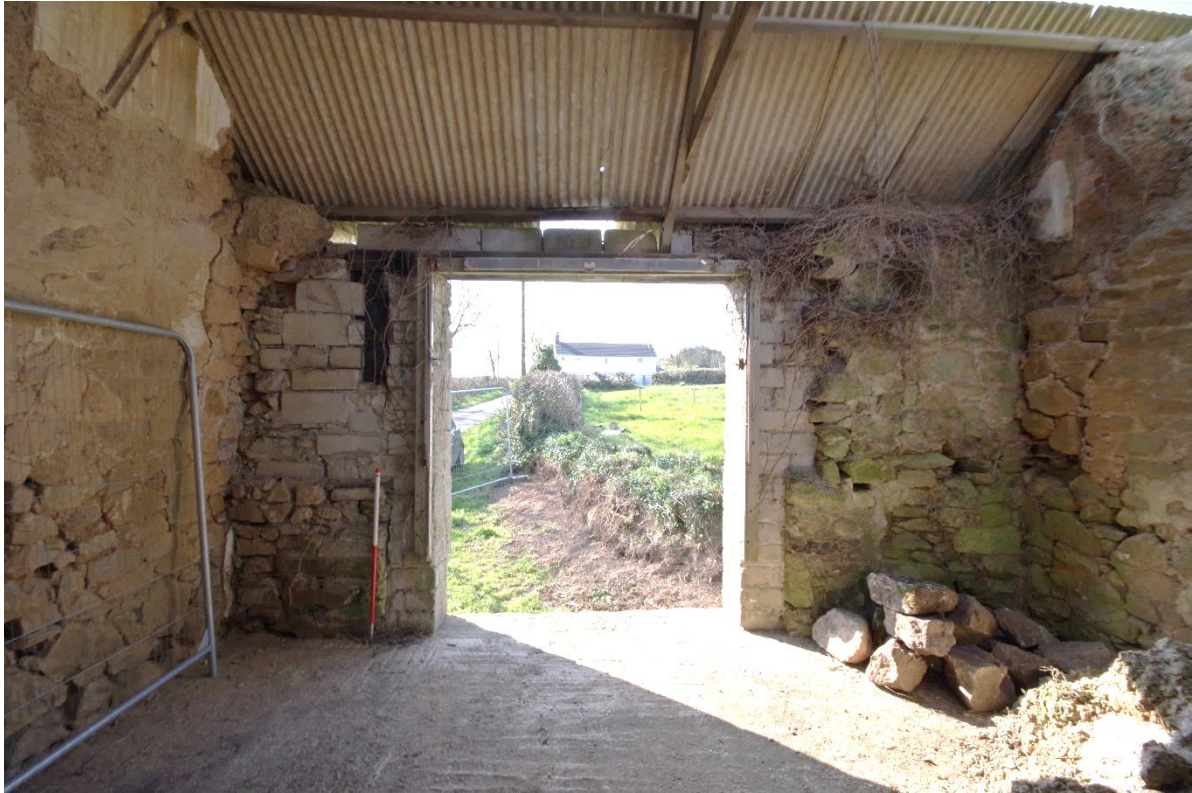
Fig 9 Interior south wall.
