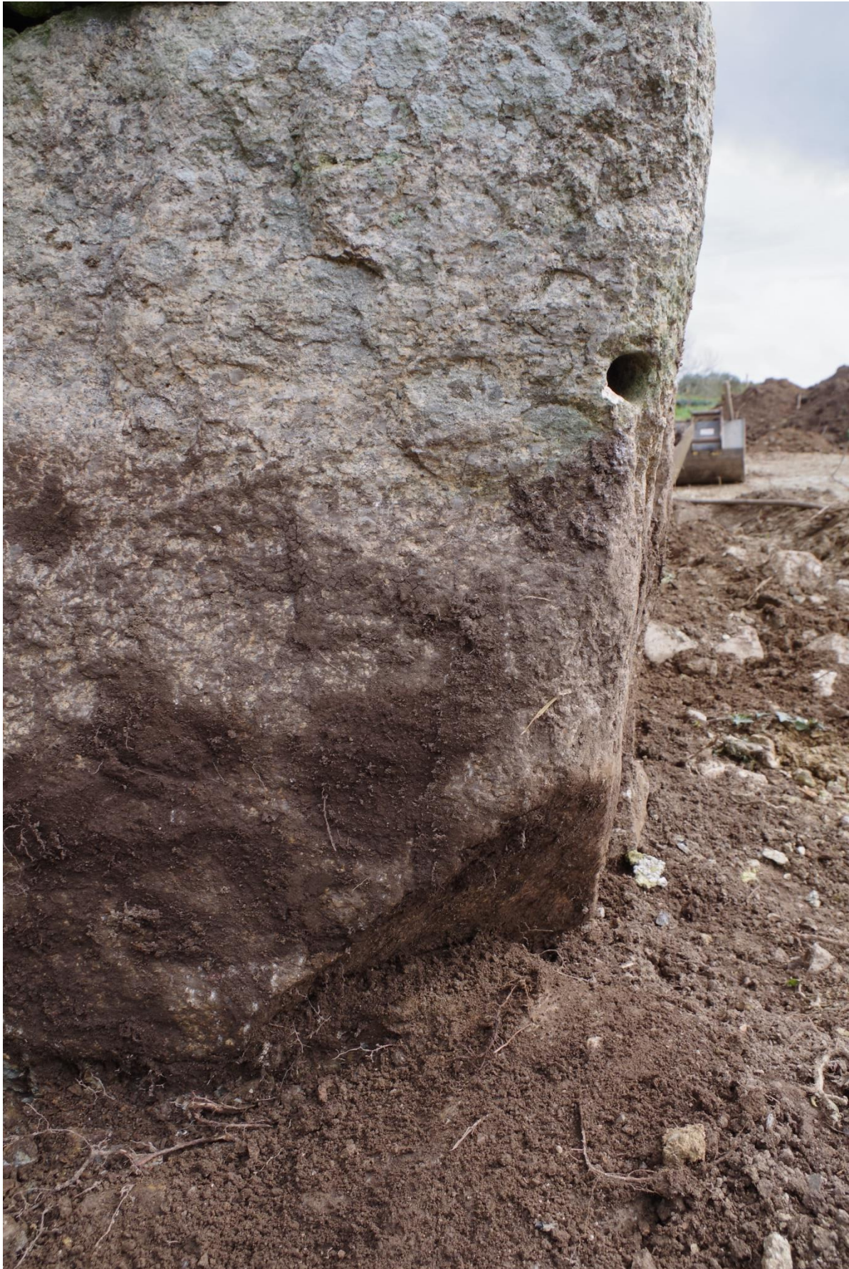
Fig 34 Reused chamfered stone to northwest corner
