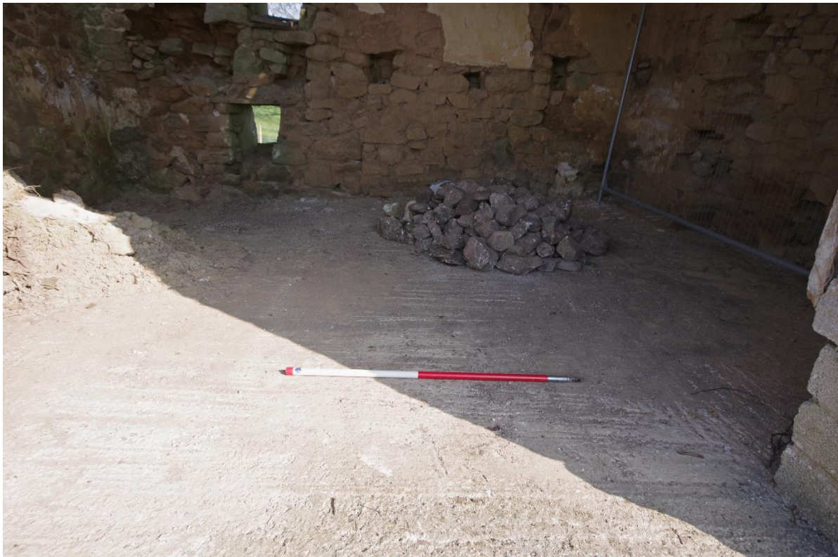
Fig 12 Modern raised concrete floor.
