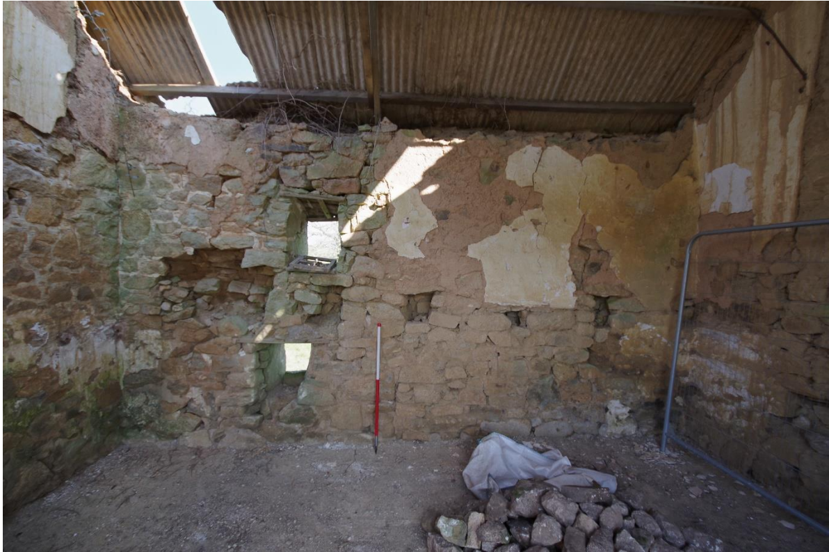
Fig 7 Interior north wall.
