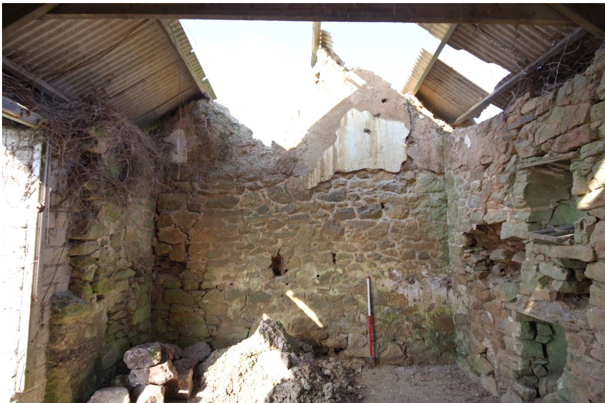
Fig 10 Interior west wall.
