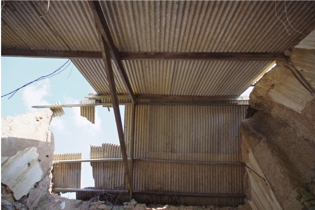
Fig 11 Modern roof structure and corrugated covering.
