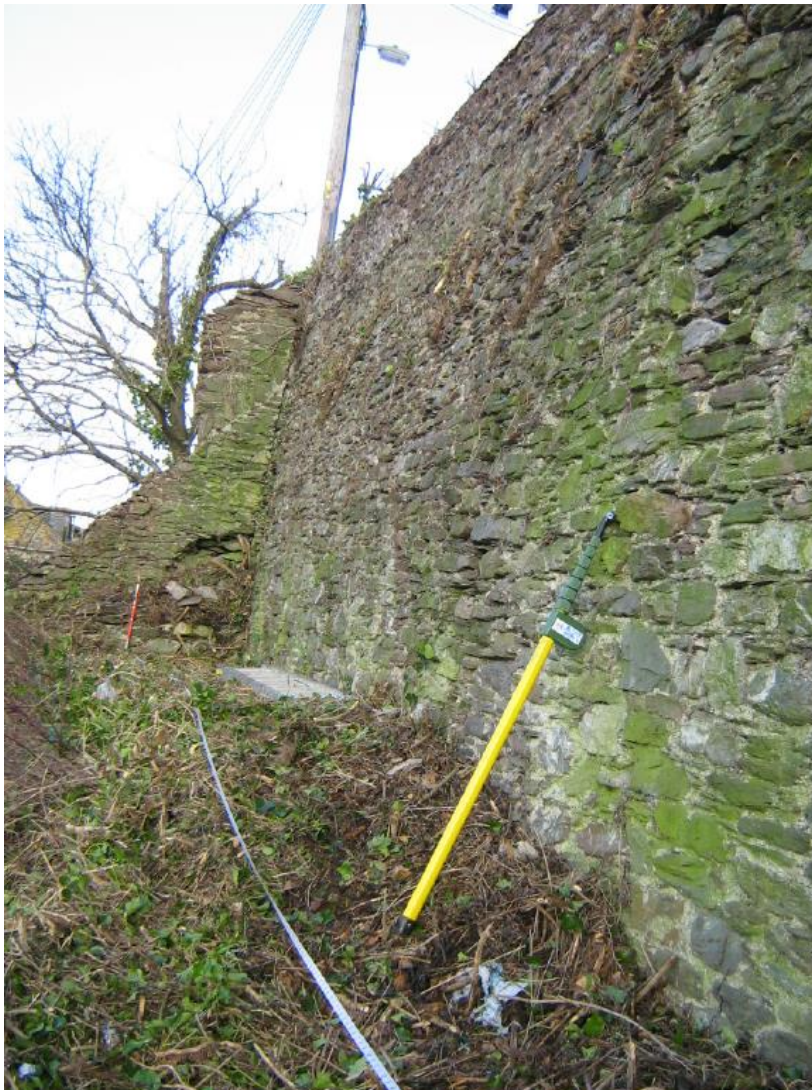
Fig 31 Section F west elevation in 2008 showing buttress (The Design & Maintenance Consultancy).
