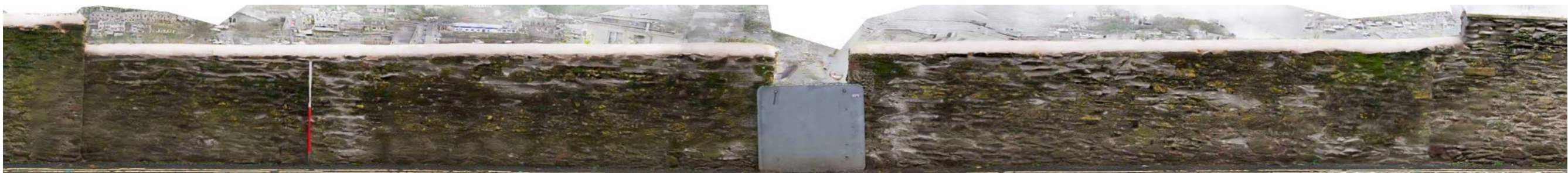
Fig 75 Orthophoto of Section H east elevation.
