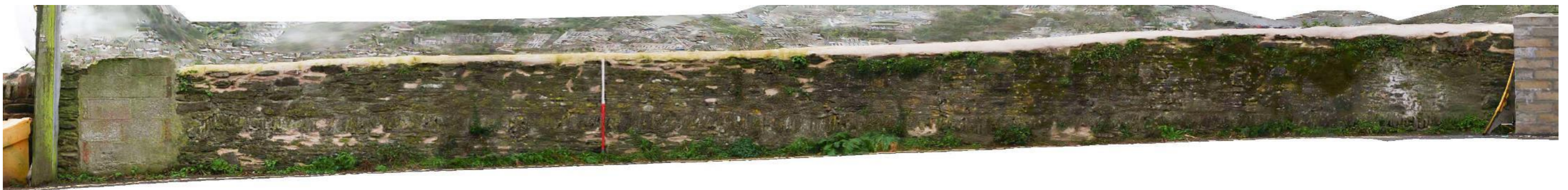
Fig 71 Orthophoto of Section C east elevation.
