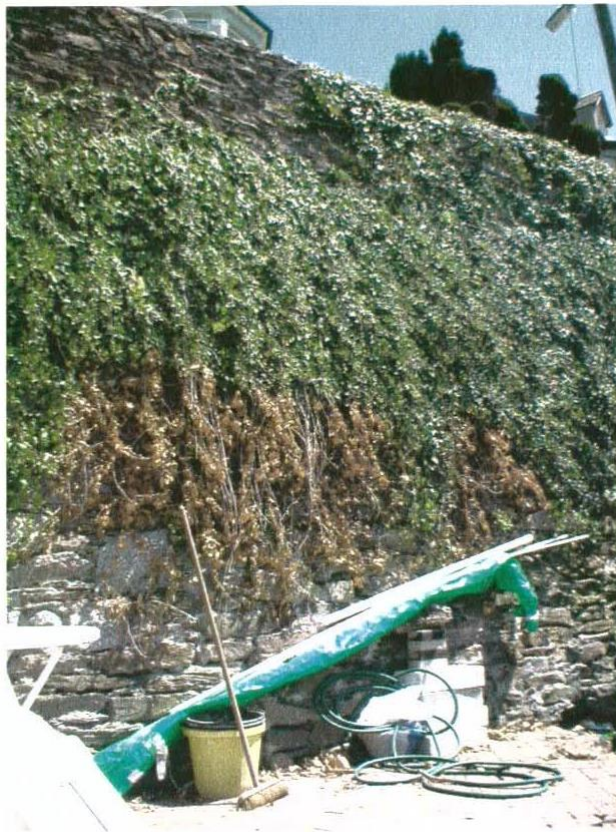
Fig 55 Section N west elevation in 2003 (The Design & Maintenance Consultancy 2003d).
