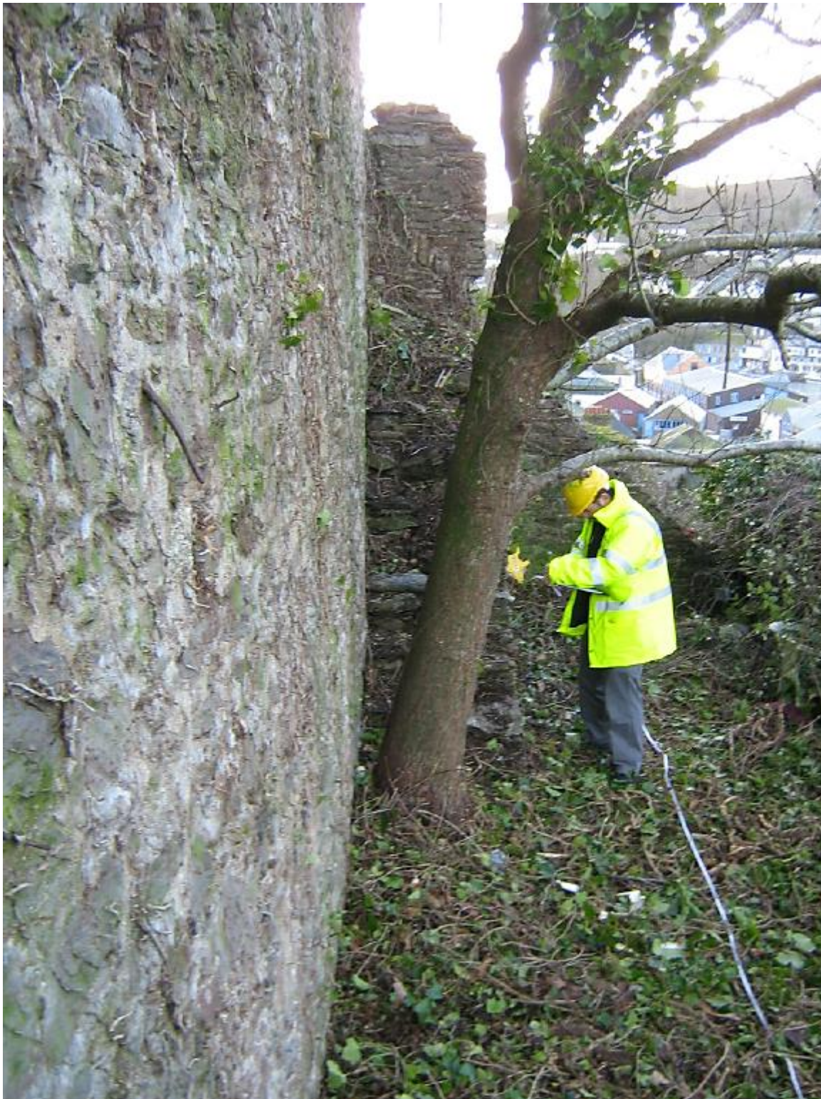
Fig 36 Section G west elevation showing steps in 2008 (The Design & Maintenance Consultancy).
