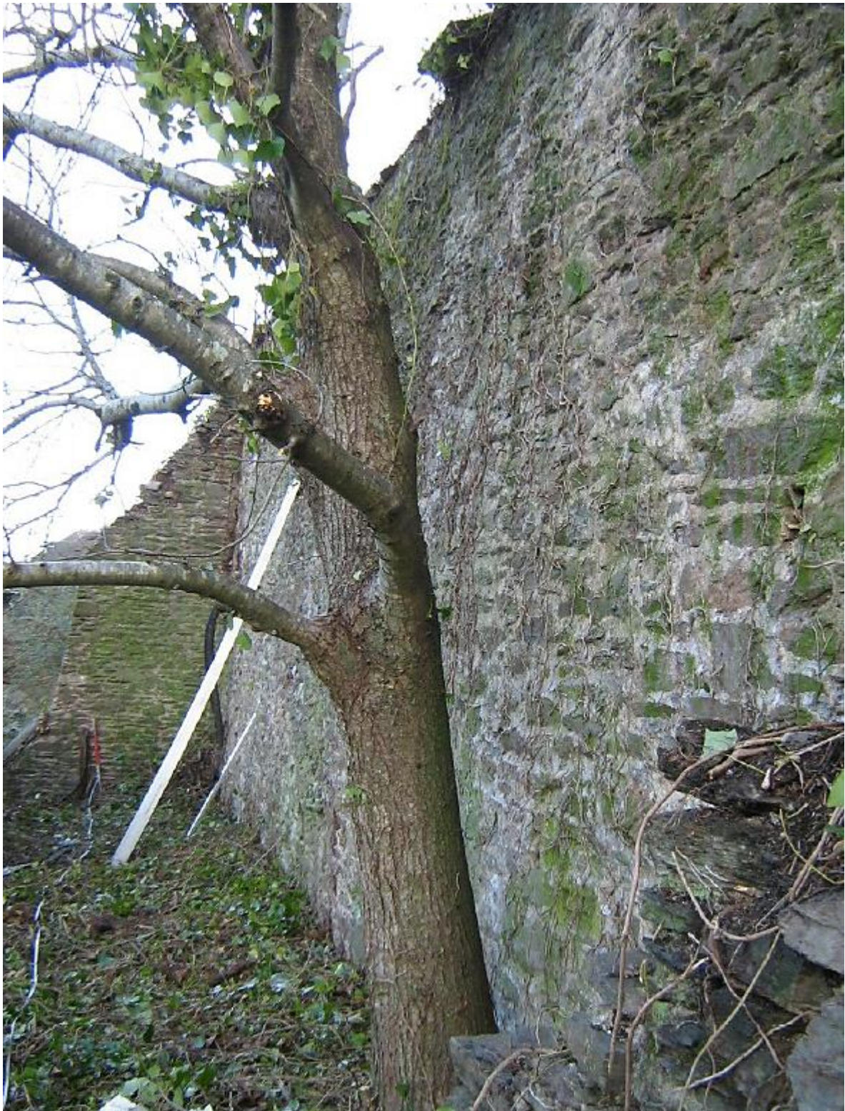
Fig 35 Section G west elevation in 2008 showing buttress (The Design & Maintenance Consultancy).
