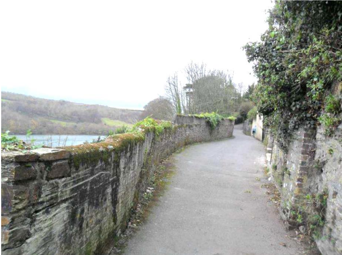
Fig 65 Section T east elevation in 2011 prior to demolition (Total Access 2011).
