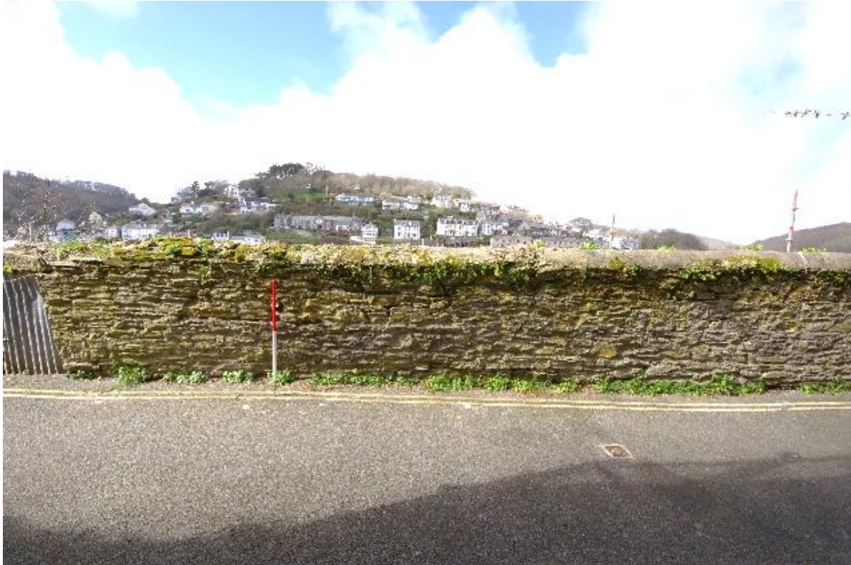
Fig 28 Section F east elevation in March 2021 prior to demolition.
