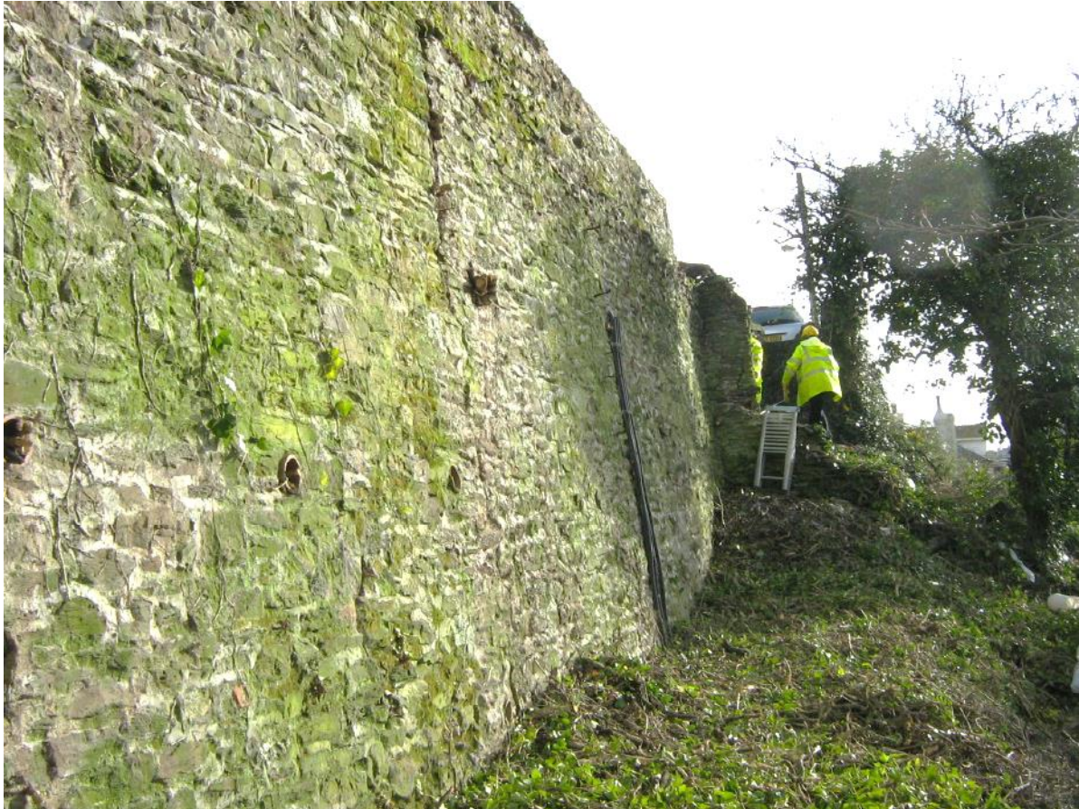
Fig 24 Section E west elevation in 2008 (The Design & Maintenance Consultancy).
