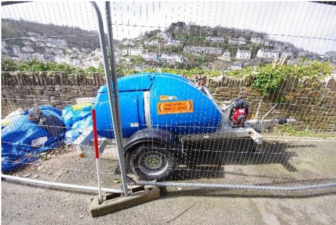
Fig 12 Section B east elevation in March 2021. No proposed works.
