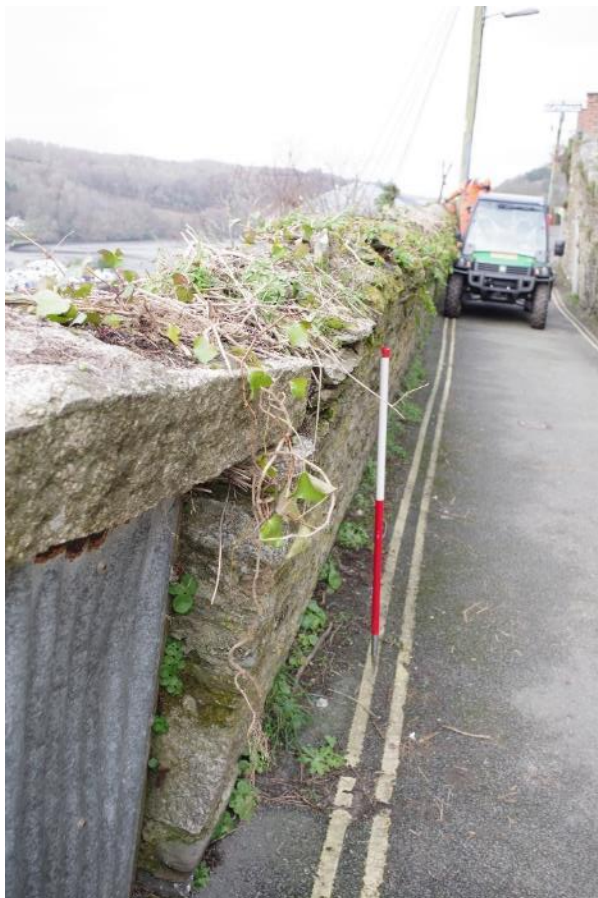
Fig 27 Section F in March 2021 prior to demolition,
