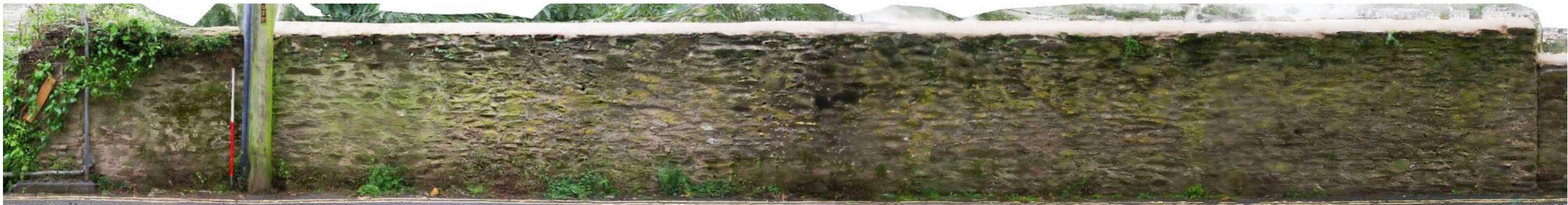
Fig 74 Orthophoto of Section G east elevation.
