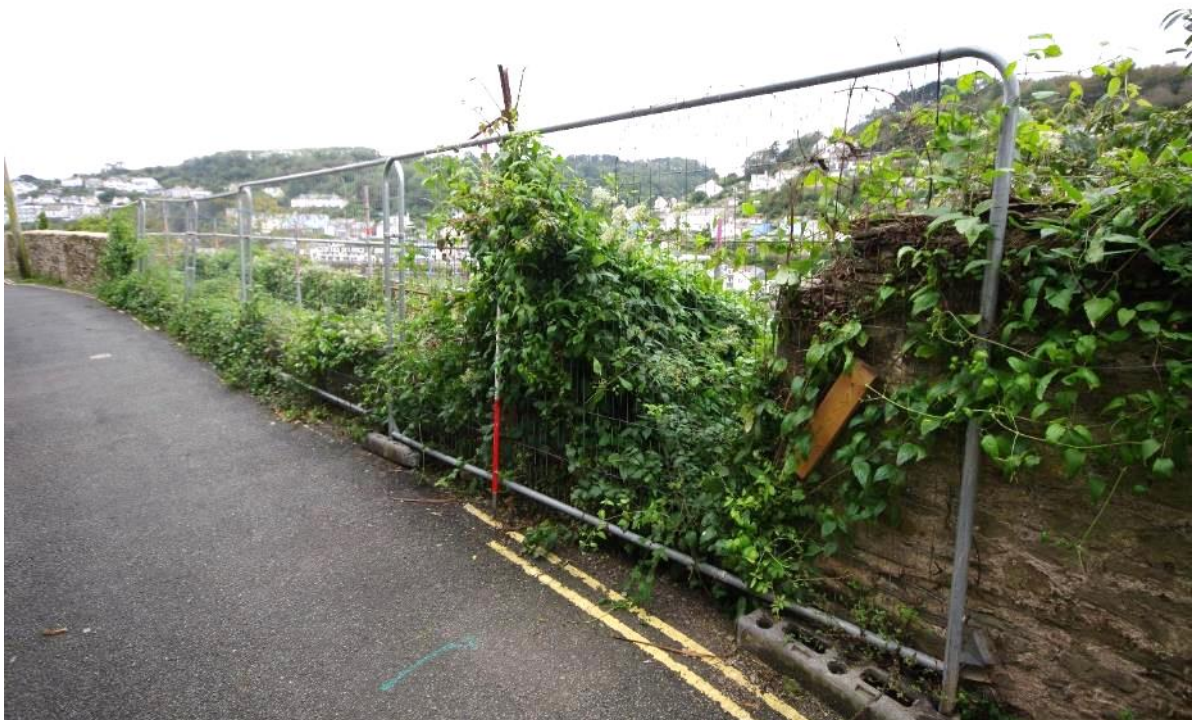
Fig 25 Section F east elevation (parapet wall now demolished).
