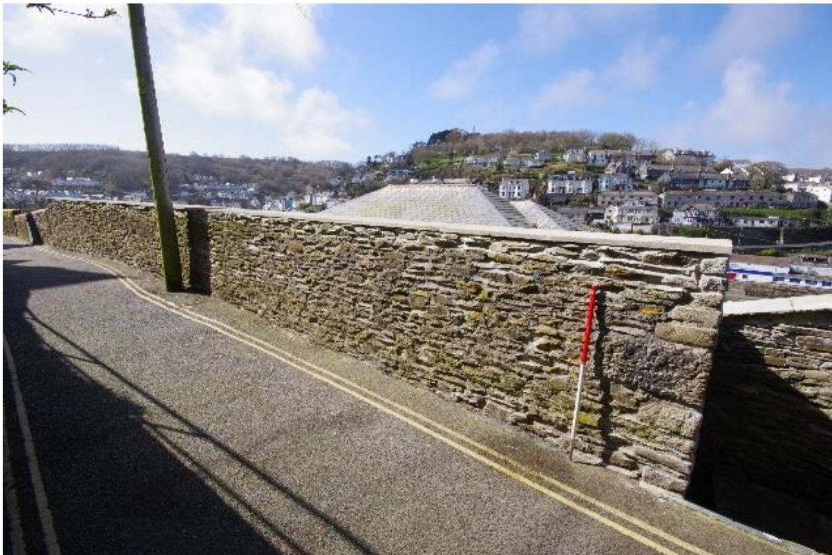
Fig 40 Section I east elevation in March 2021. No proposed works.
