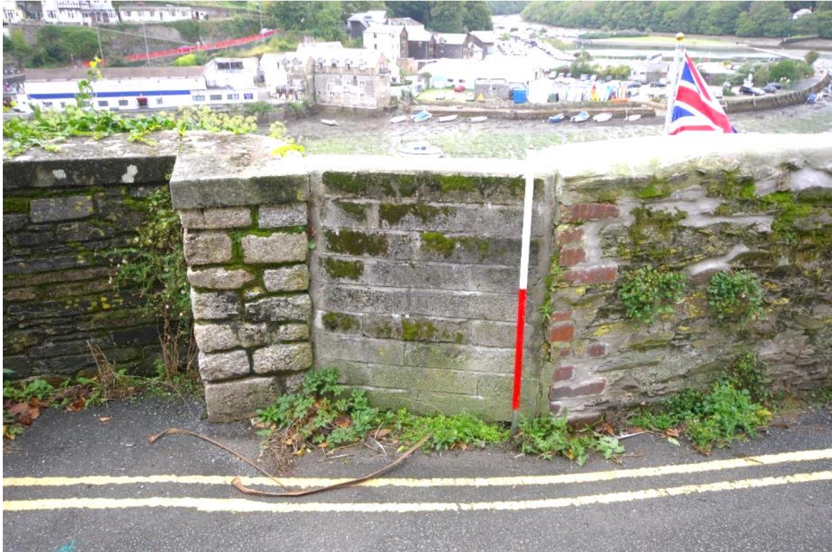
Fig 43 Section K blocked opening at south end.
