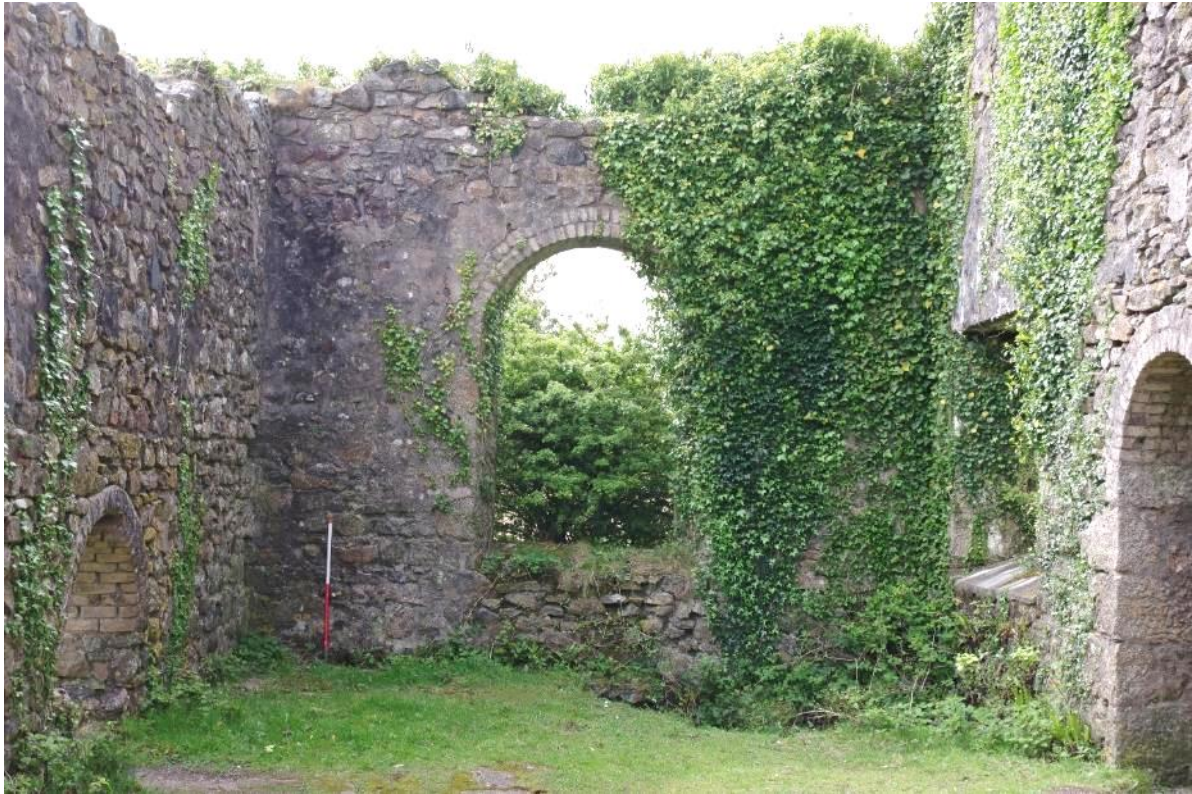
Fig 48 Room 4 south wall.
