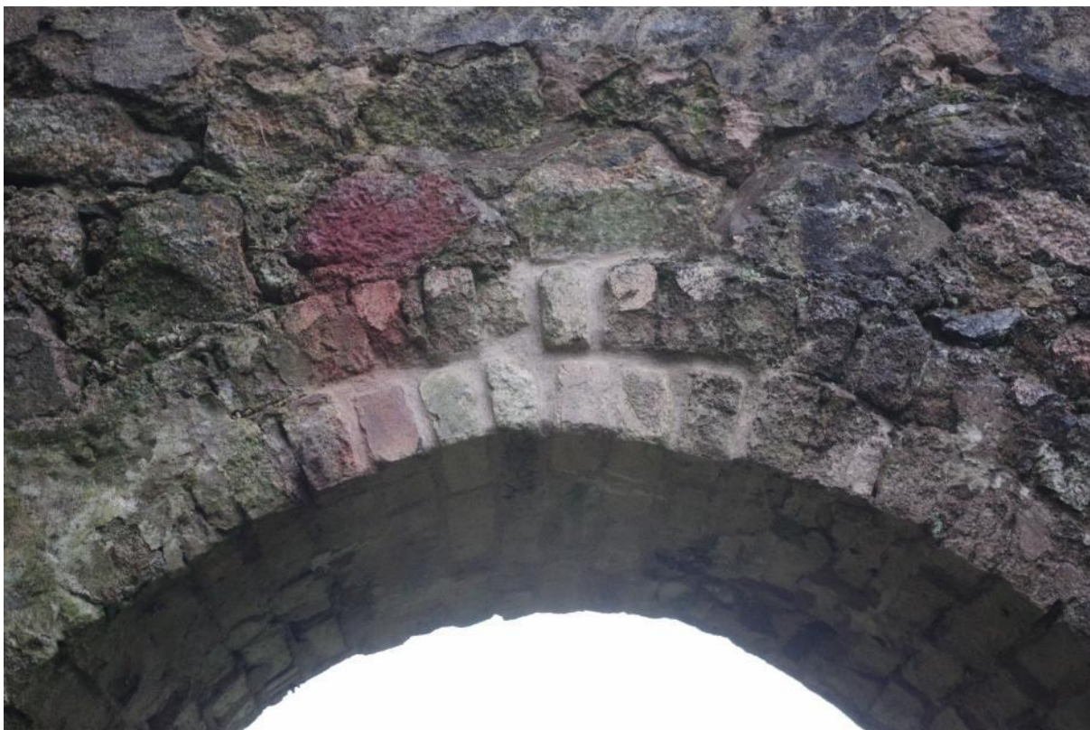
Fig 81 Room 9 south wall following repair of the window arch.
