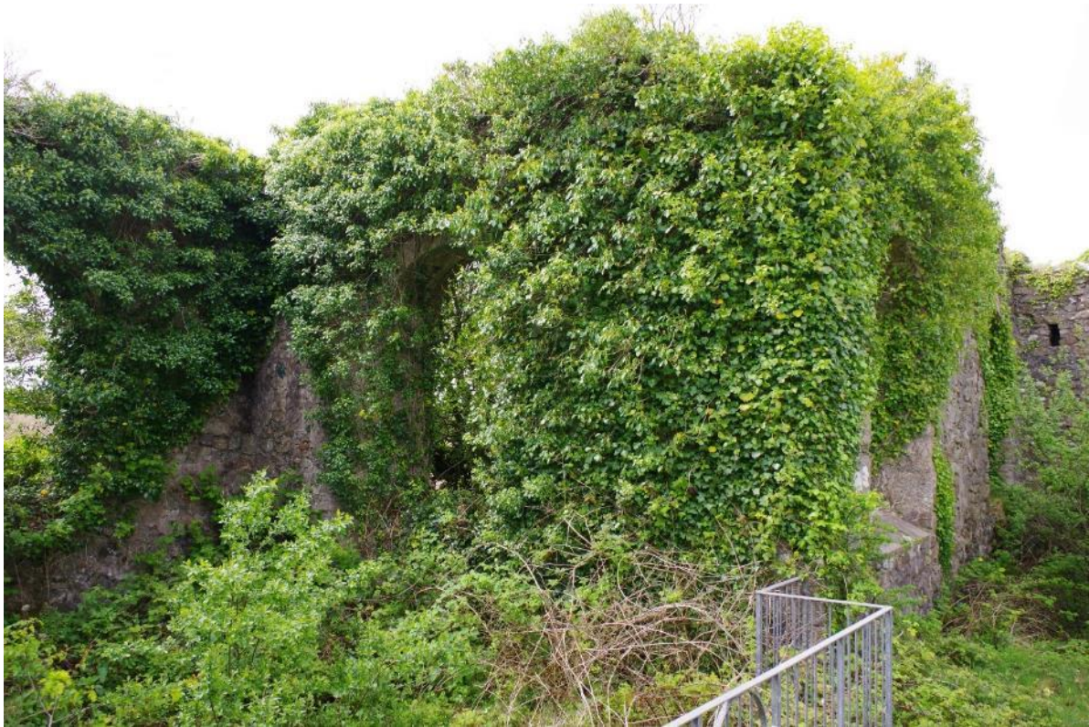
Fig 66 Room 6 west wall.
