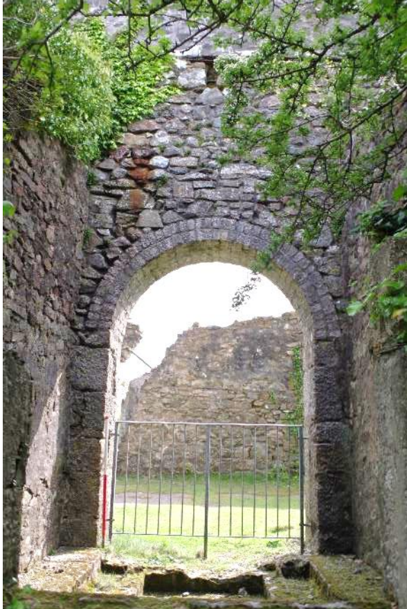
Fig 31 Room 2 east wall.
