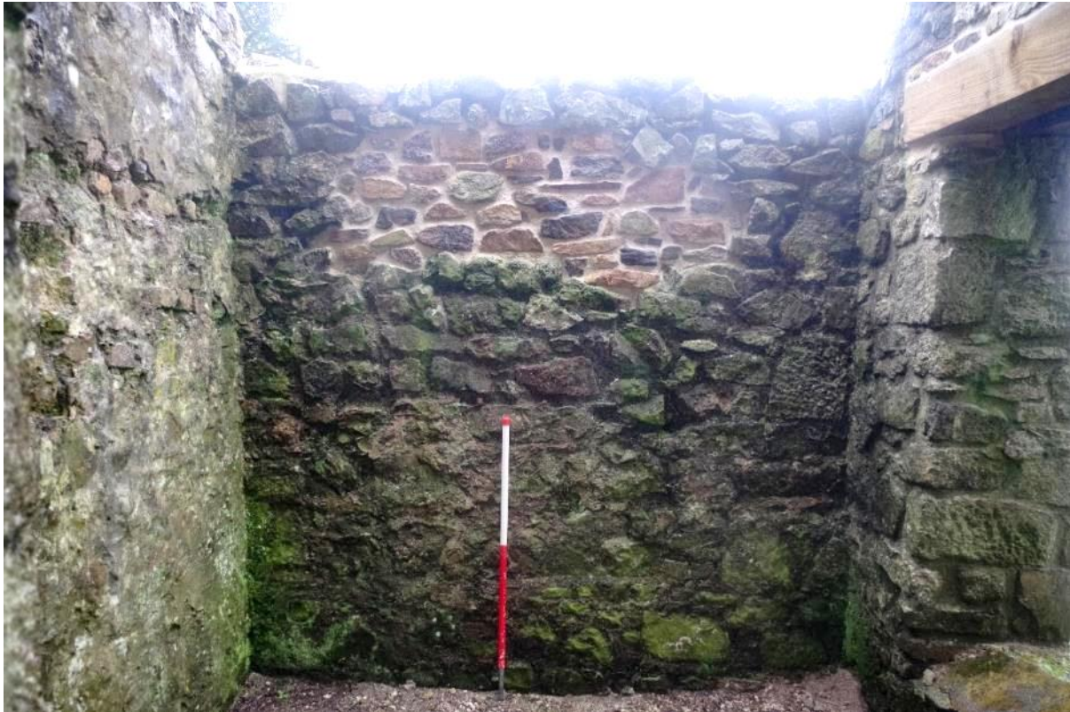
Fig 40 Room 3 west wall following masonry repairs.
