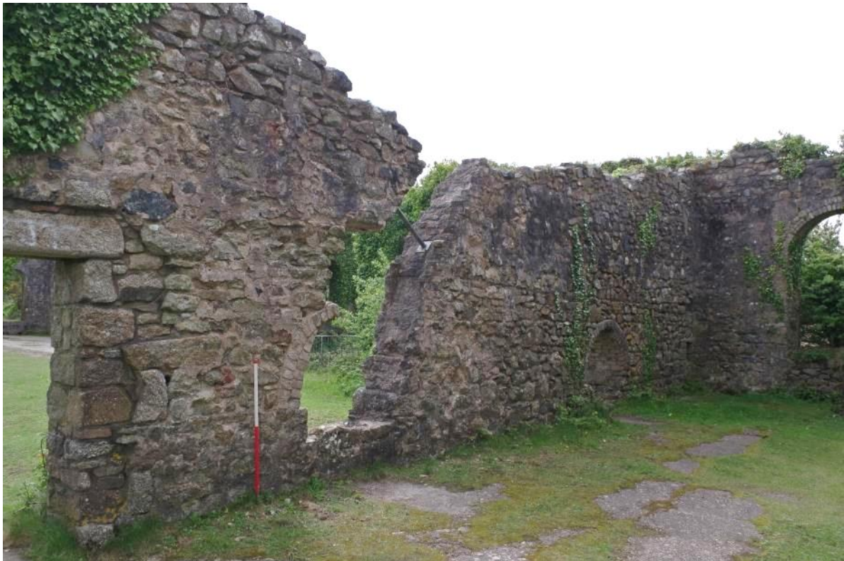
Fig 43 Room 4 east wall looking southeast.
