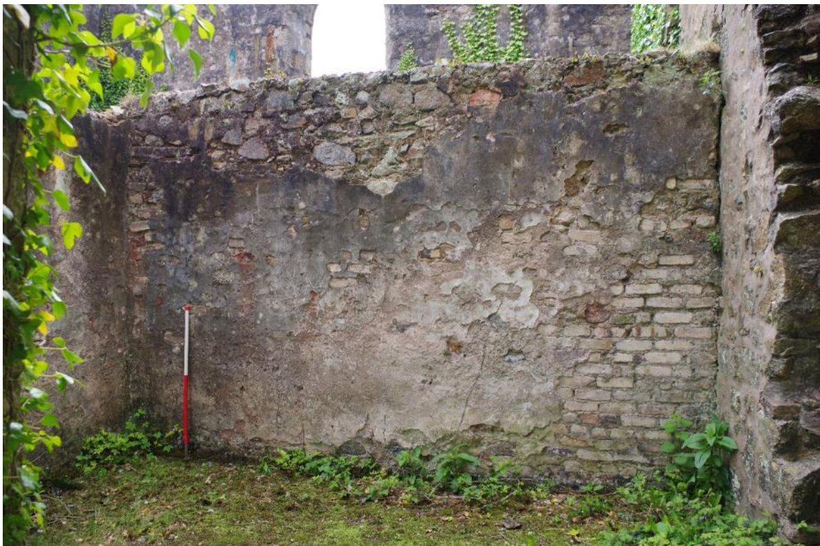
Fig 75 Room 8 south wall.
