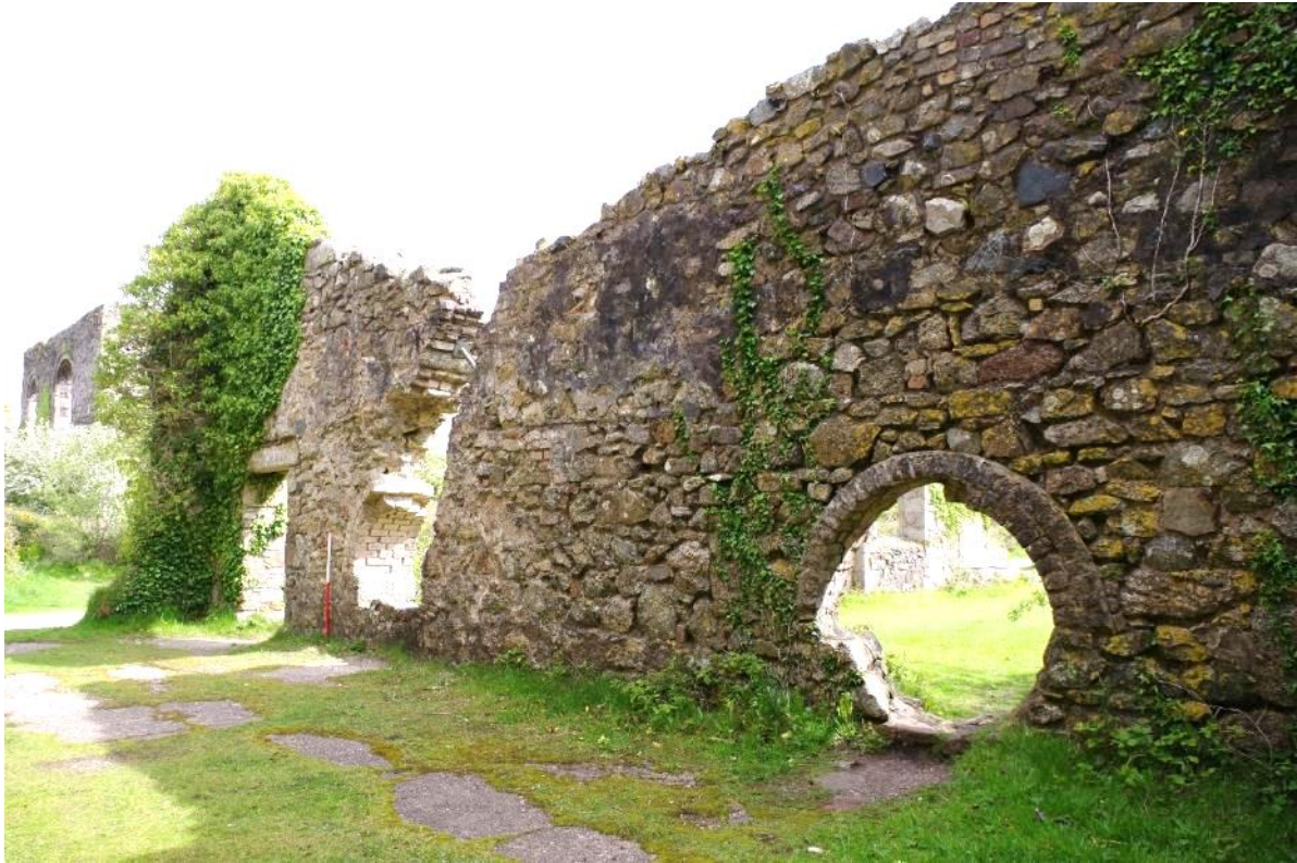
Fig 42 Room 4 east wall looking northeast.
