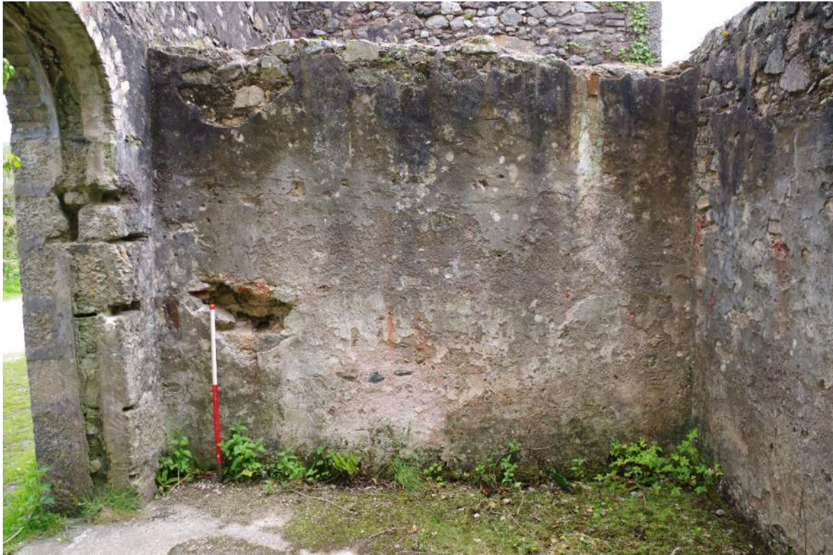
Fig 74 Room 8 east wall.
