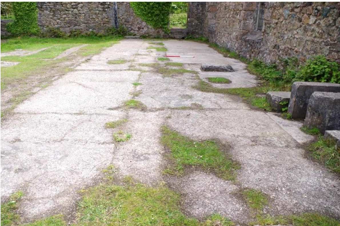
Fig 61 Room 5 inserted phase 3 concrete floor in southeast quarter of the room, looking east.
