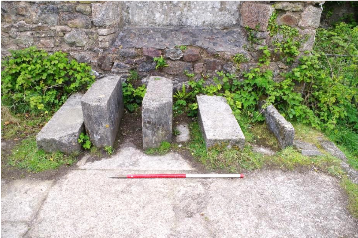
Fig 62 Room 5, phase 3 concrete machine base against south wall.
