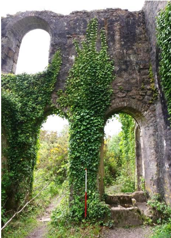
Fig 70 Rooms 7 and 10 south wall.
