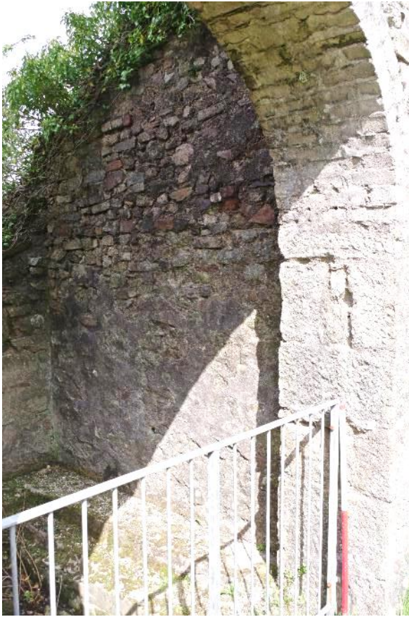
Fig 30 Room 2 north wall.
