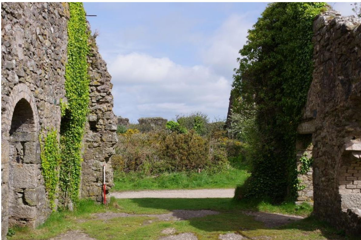
Fig 41 Room 4 remains of north wall (now mostly missing).
