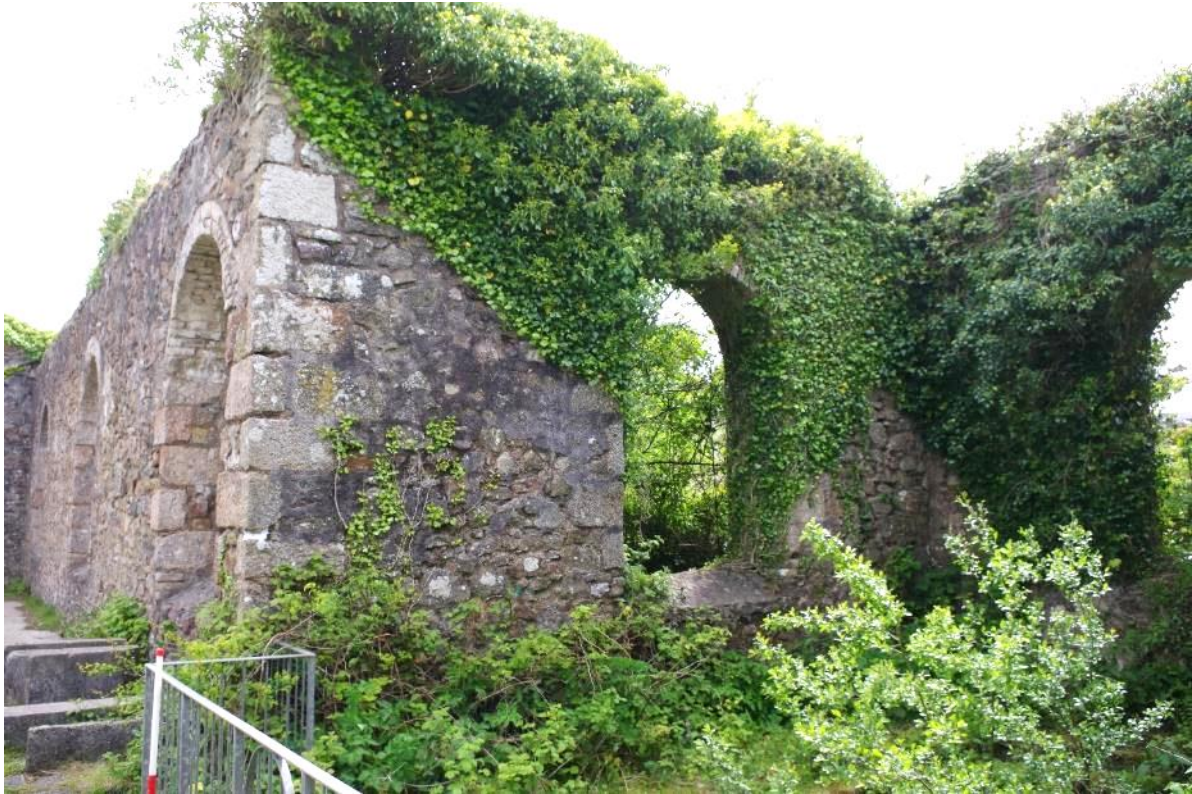
Fig 64 Room 6 east wall.
