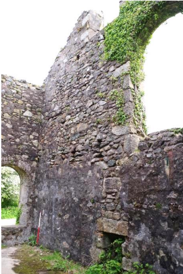
Fig 78 Room 9 east wall looking northeast, with room 10 at first floor level.
