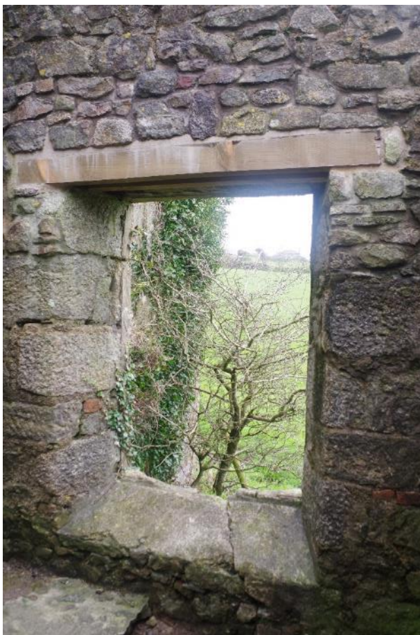
Fig 27 Room 1 south wall following replacement of lintel.
