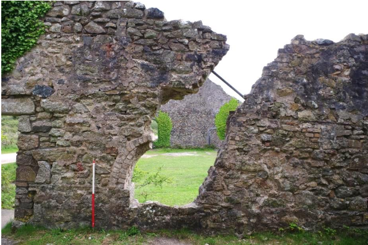
Fig 44 Room 4 east wall, northern steam pipe opening before repairs.
