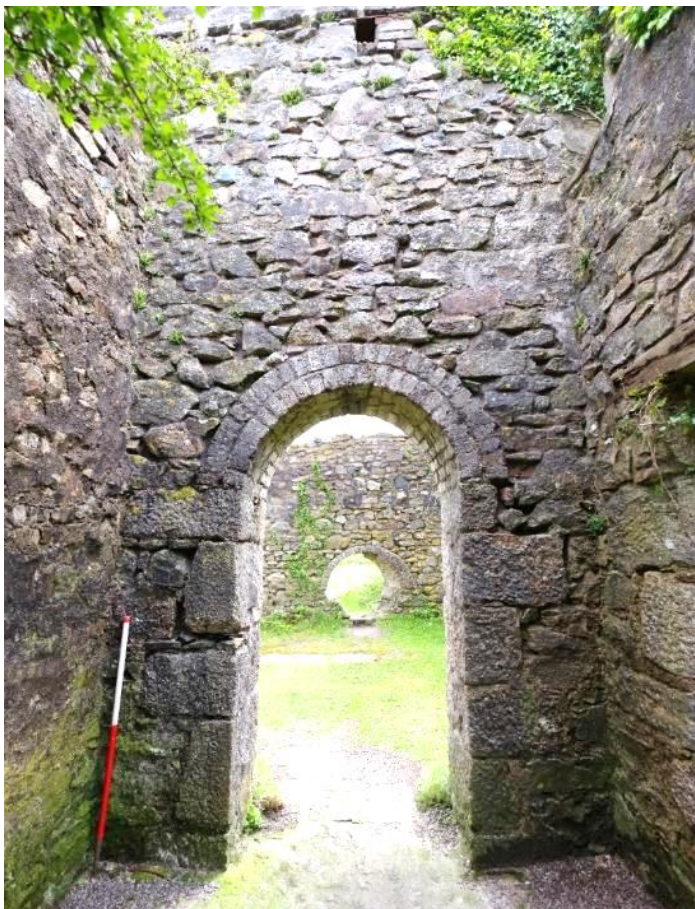
Fig 25 Room 1 east wall.
