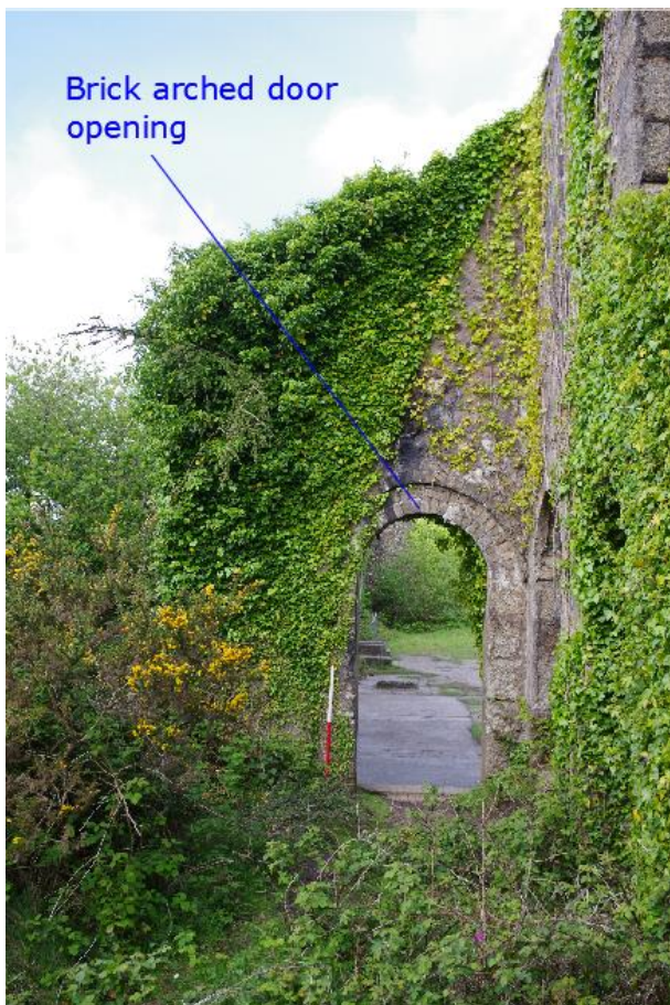
Fig 17 East elevation of main dry where it protrudes to the south.
