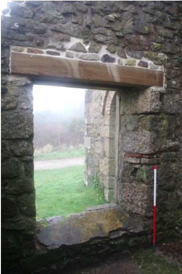
Fig 36 Room 3 north wall following insertion of new lintel and repairs.
