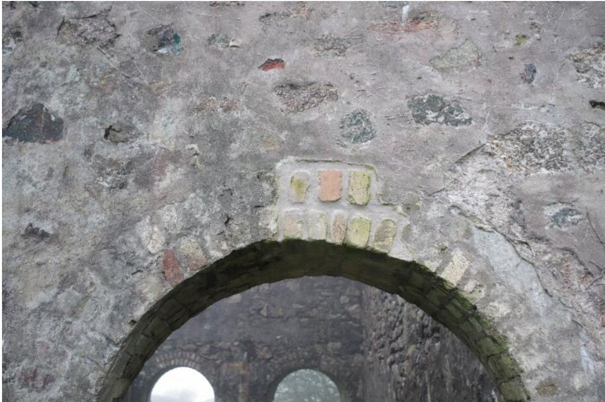
Fig 82 South exterior elevation of the window arch of room 9 following repair.
