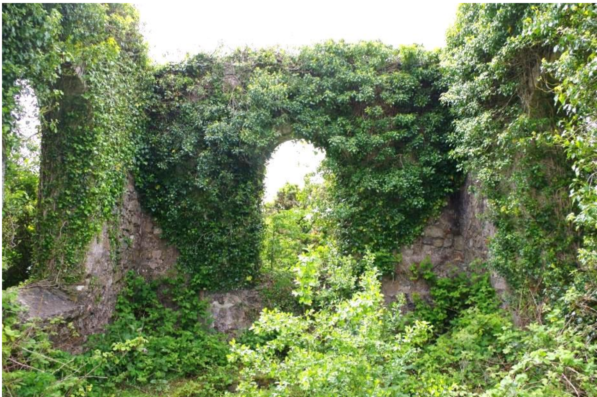
Fig 65 Room 6 south wall.
