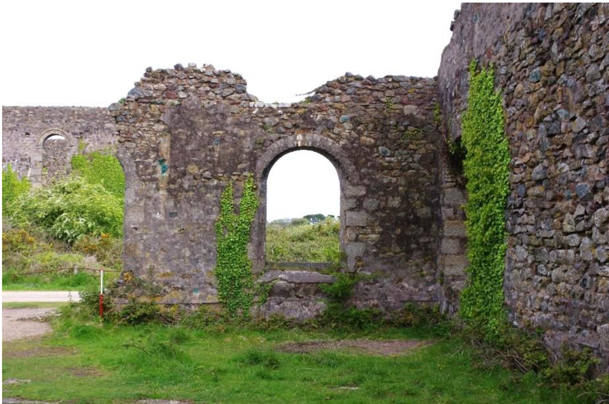
Fig 53 Room 5 north wall, extant section at east end.
