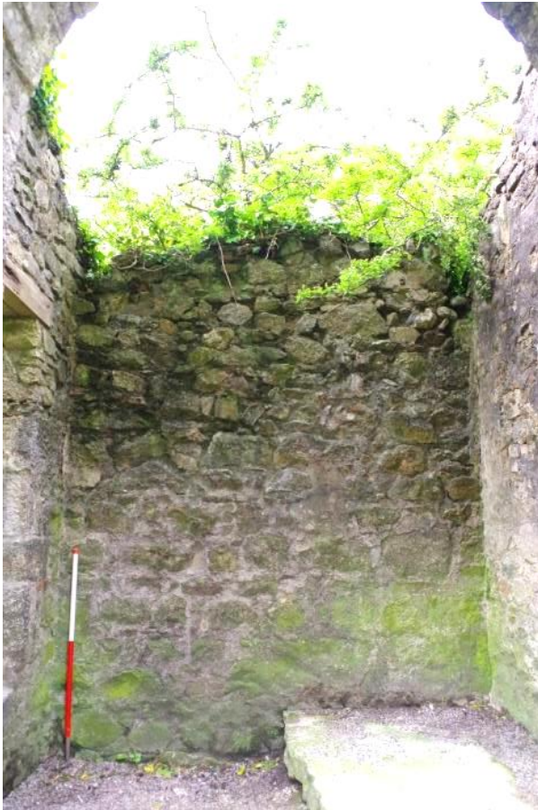
Fig 28 Room 1 west wall.
