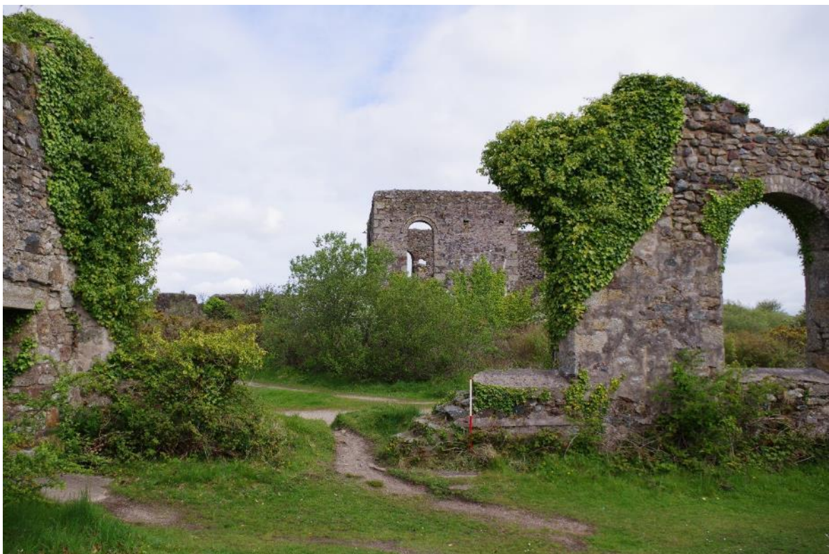
Fig 51 Room 5 north wall, missing section at west end.
