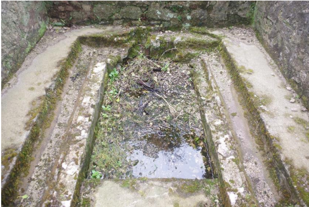
Fig 34 Room 2 cement rendered bath looking west.
