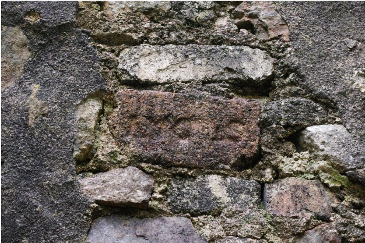
Fig 24 Room 1, St Day brick in the north wall.
