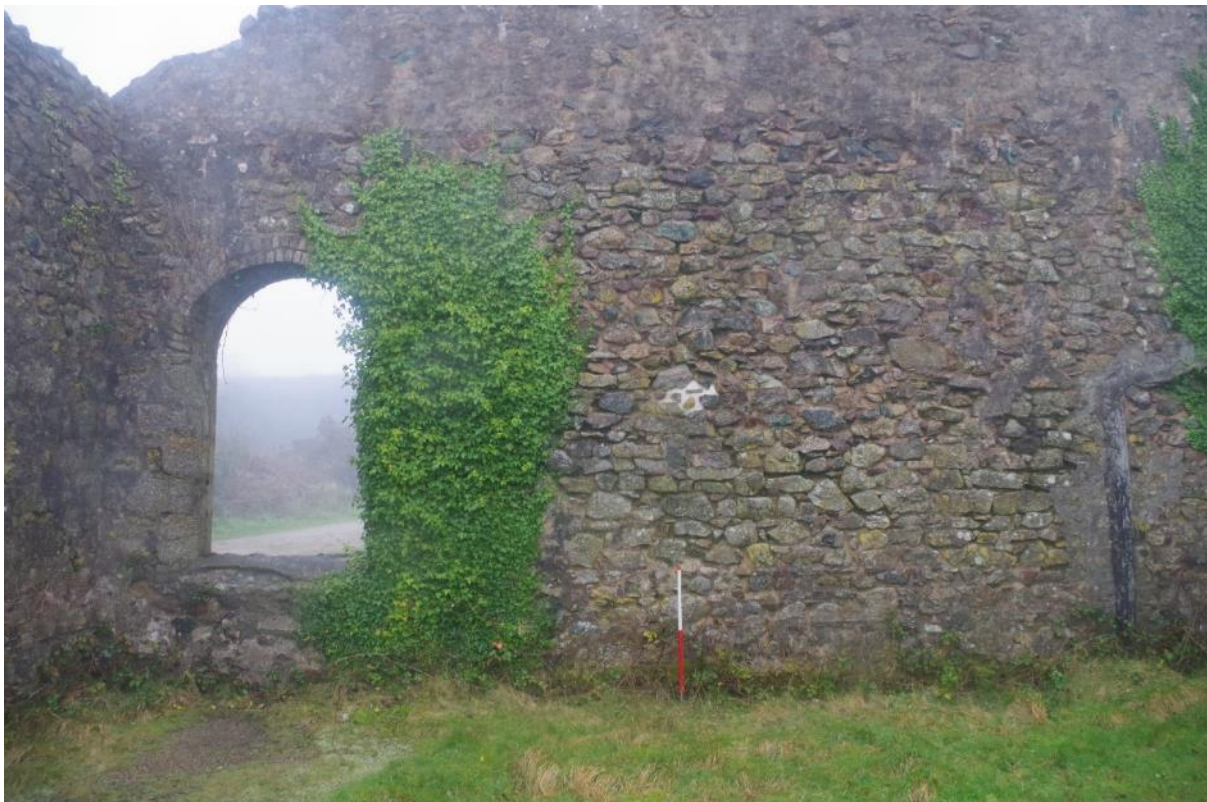
Fig 55 Room 5 east wall following repairs, showing small patch repair.
