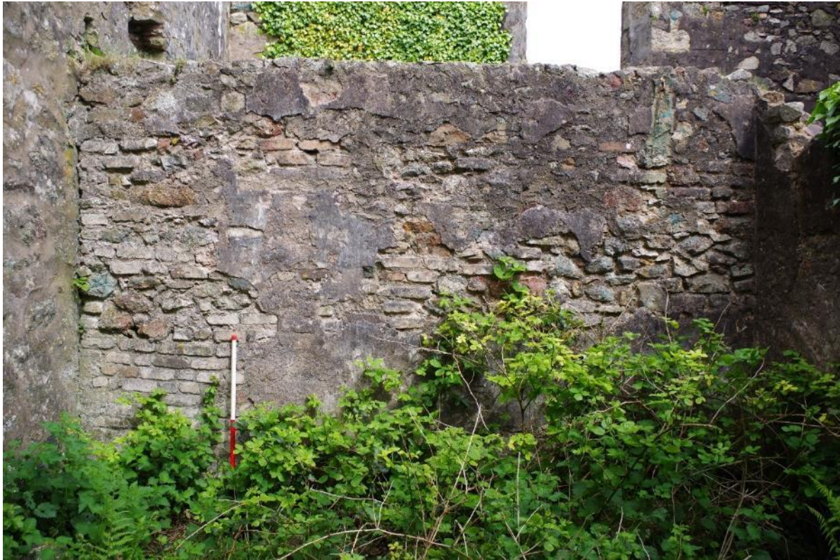
Fig 68 Room 7 north wall.
