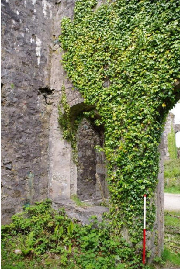
Fig 73 Room 8 north wall (west half) with room 10 at first floor level.
