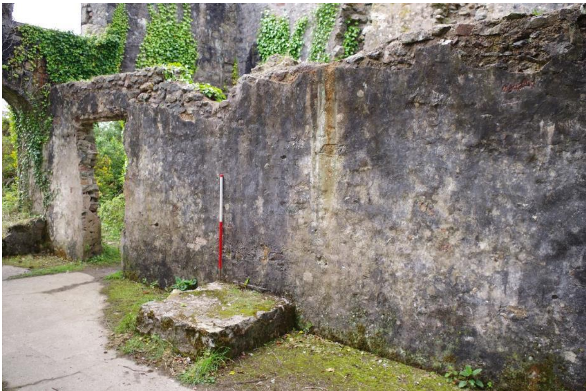
Fig 83 Room 9 west wall.
