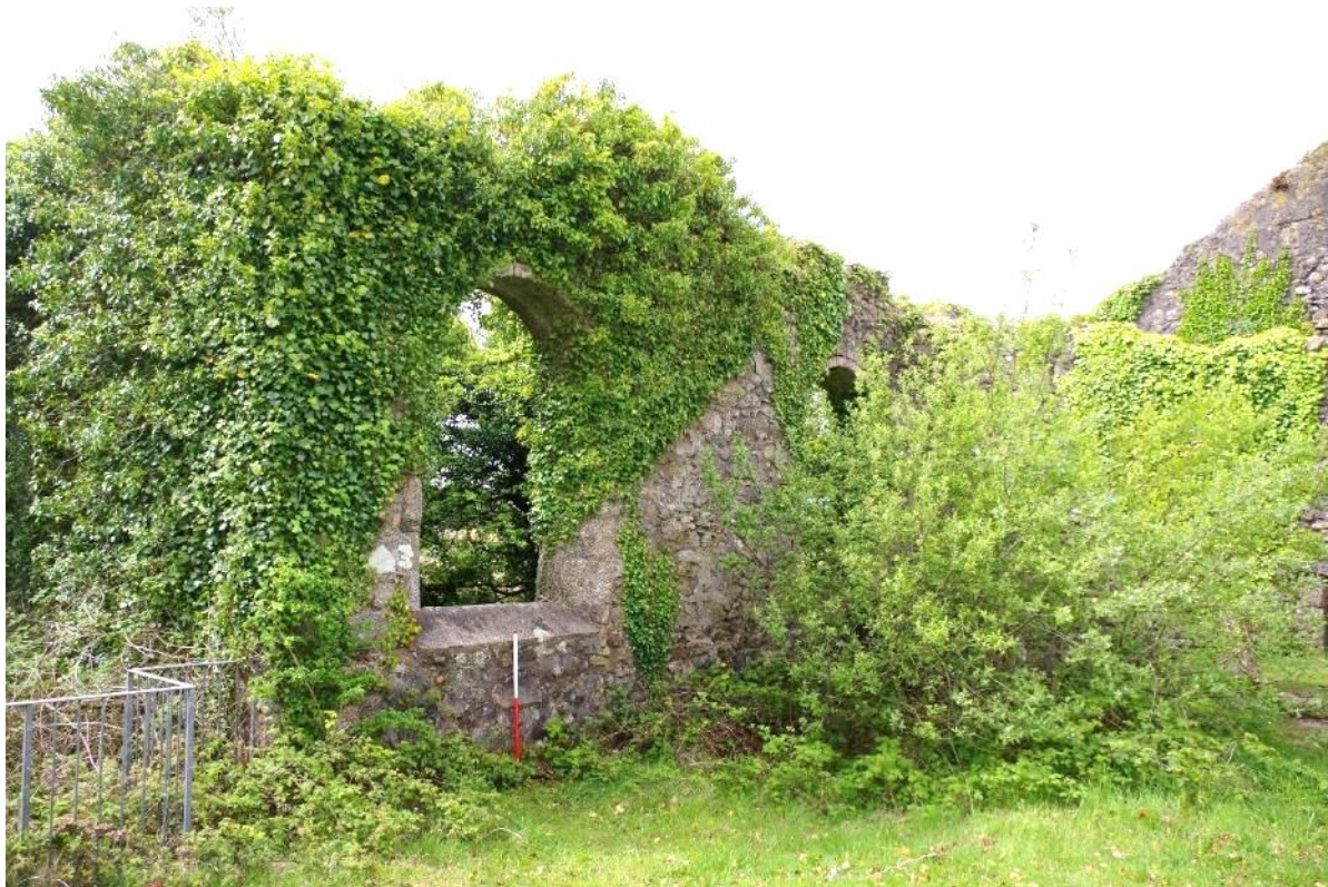
Fig 57 Room 5 south wall, western half.
