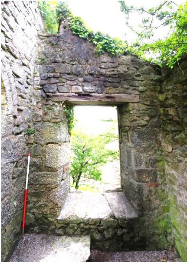
Fig 26 Room 1 south wall.
