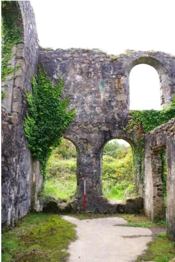
Fig 80 Room 9 south wall before repairs, with room 10 at first floor level.
