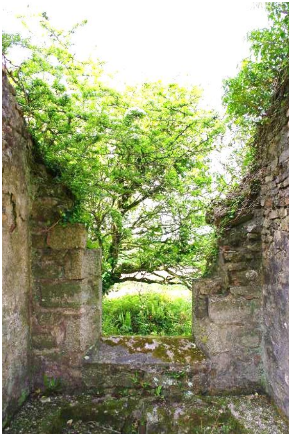
Fig 33 Room 2 west wall.
