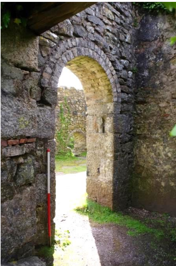
Fig 37 Room 3 east wall.
