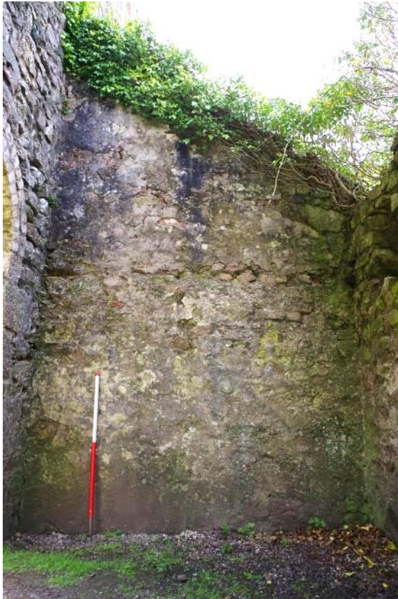
Fig 38 Room 3 south wall.
