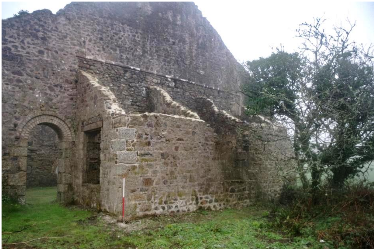
Fig 21 West elevation following vegetation clearance and repair work.
