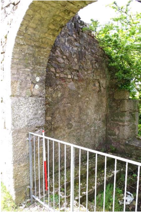
Fig 32 Room 2 south wall.
