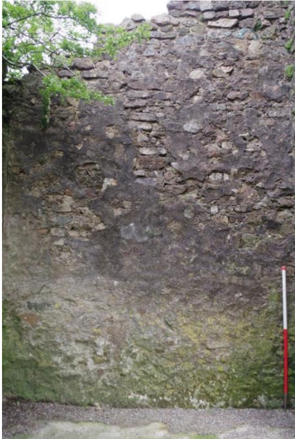
Fig 23 Room 1 north wall.
