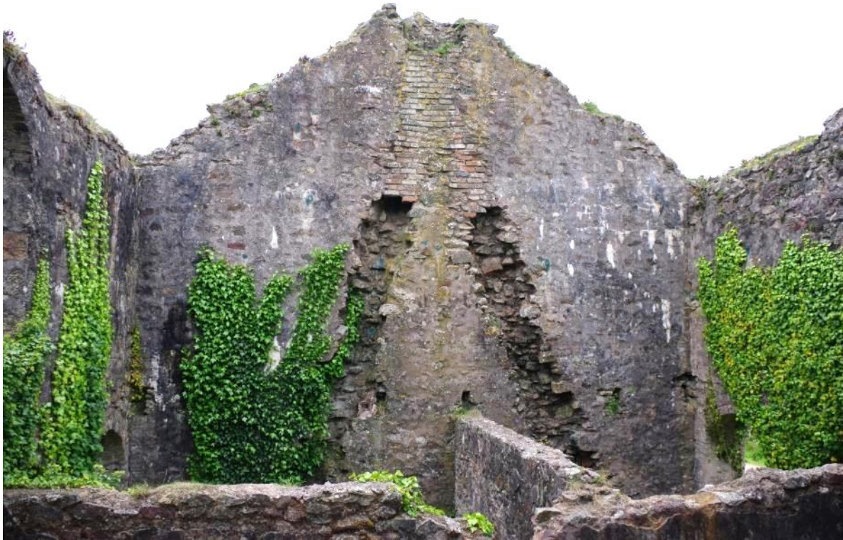
Fig 84 Room 10 before the repair of the flues in the west wall.
