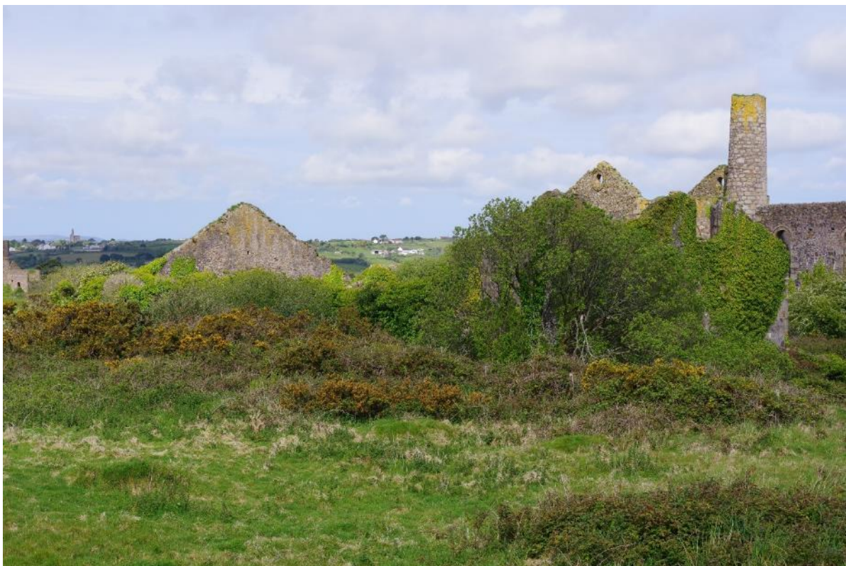
Fig 19 South elevation which is mainly inaccessible and heavily overgrown.
