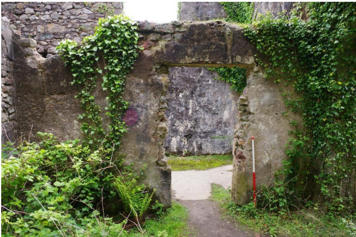
Fig 69 Room 7 east wall.
