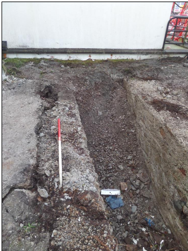
Fig 22 Looking along the leat towards the former Cowlins Mill, looking south.
