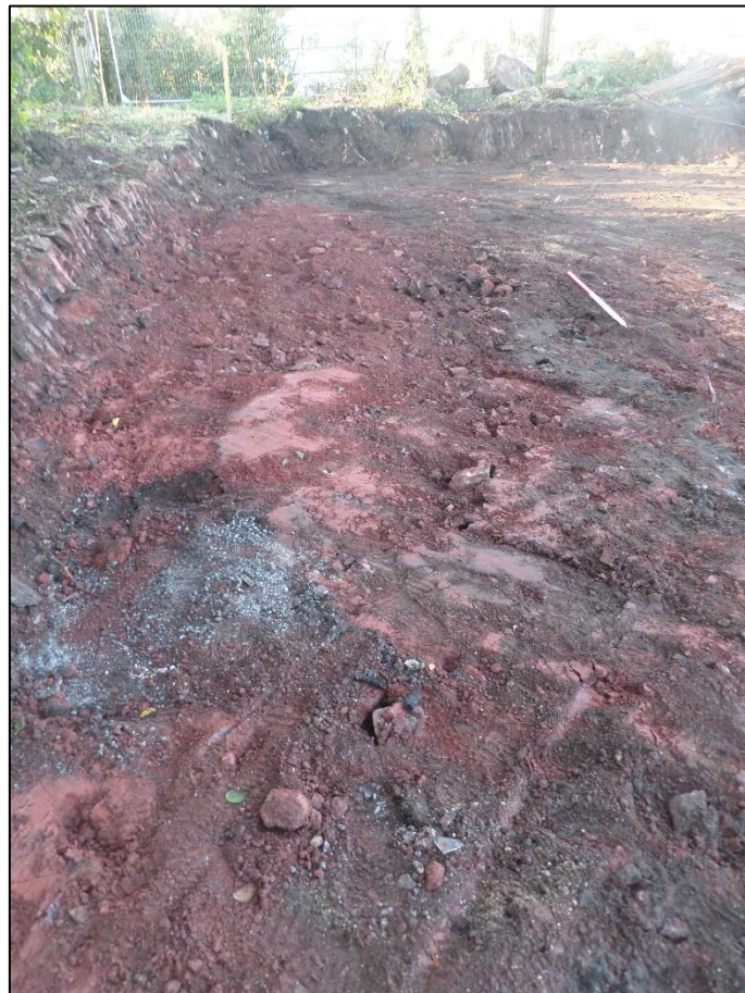
Fig 10 General shot of southwestern section of the excavated area, looking southwest.
