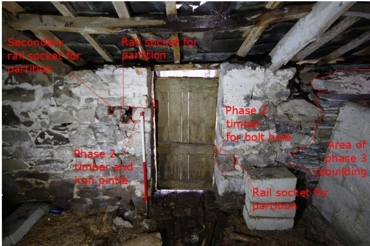
Fig 27 Northwest wall of the piggery showing door B.
