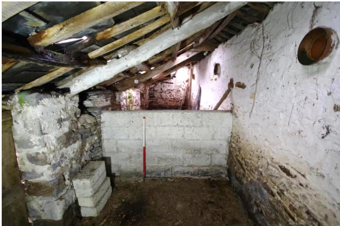
Fig 28 Inserted 20th century partition wall inside the piggery, looking northeast.
