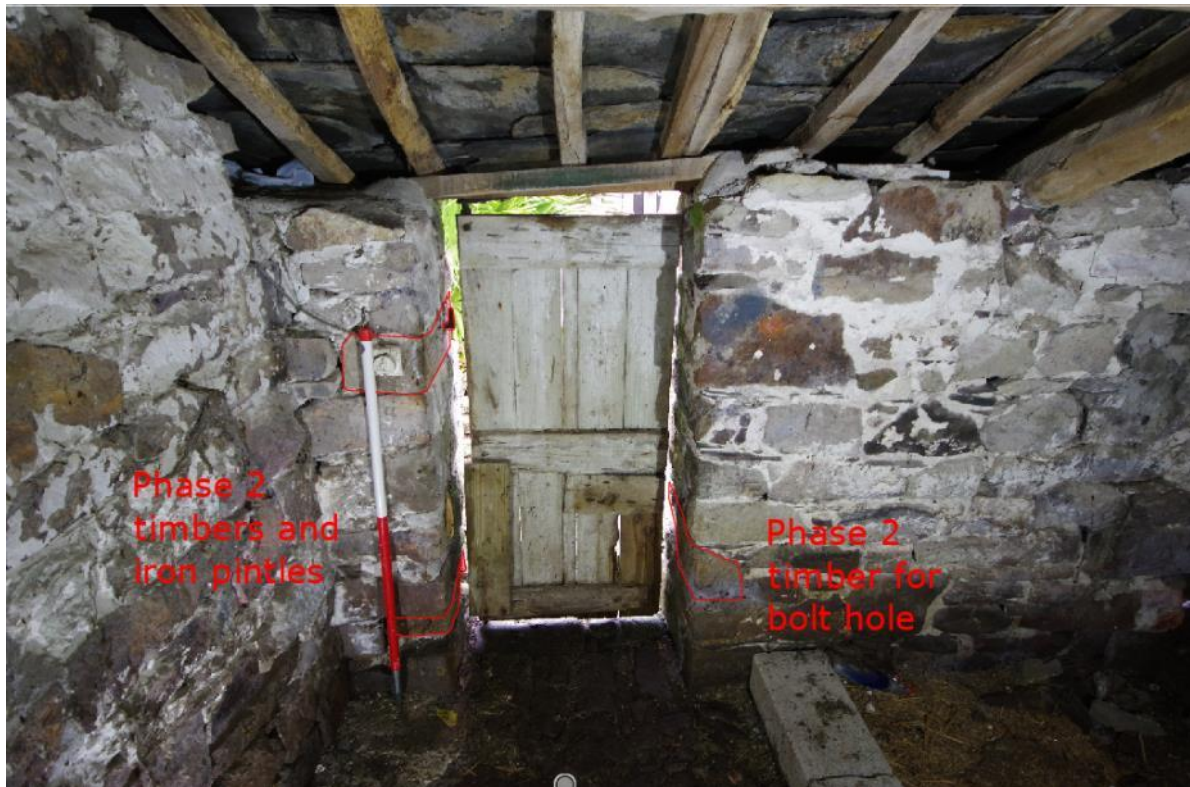
Fig 25 Northwest wall of the piggery, showing door A.
