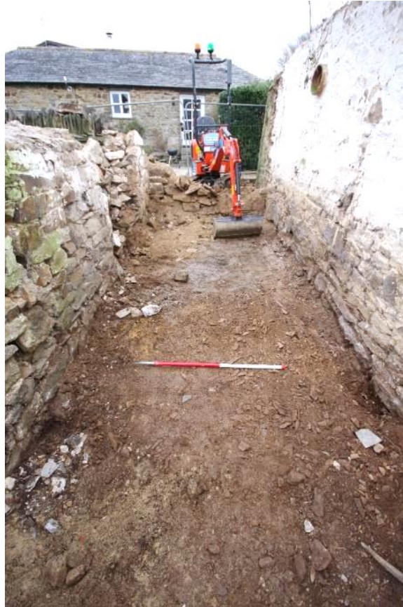
Fig 45 View looking northeast following the removal of the floor.
