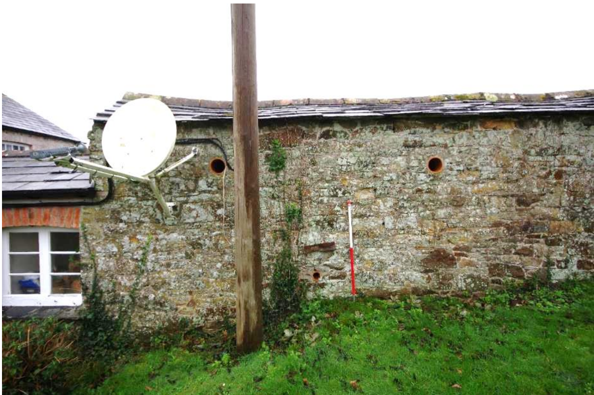
Fig 22 Southwest end of the southeast elevation.
