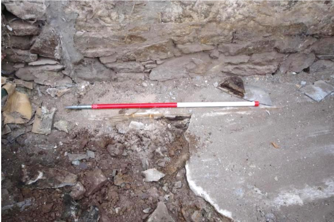
Fig 43 The timber revealed embedded in the lime screed (102).
