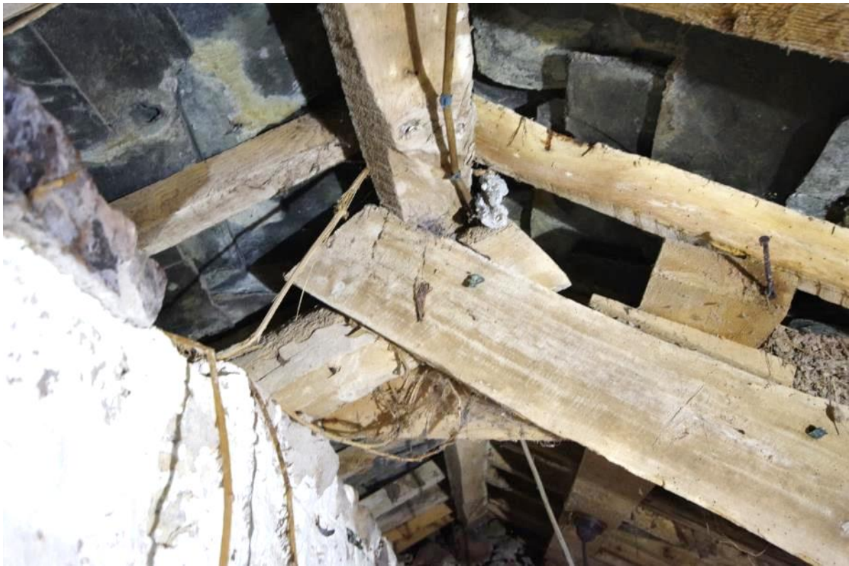
Fig 38 Example of the small collar trusses.
