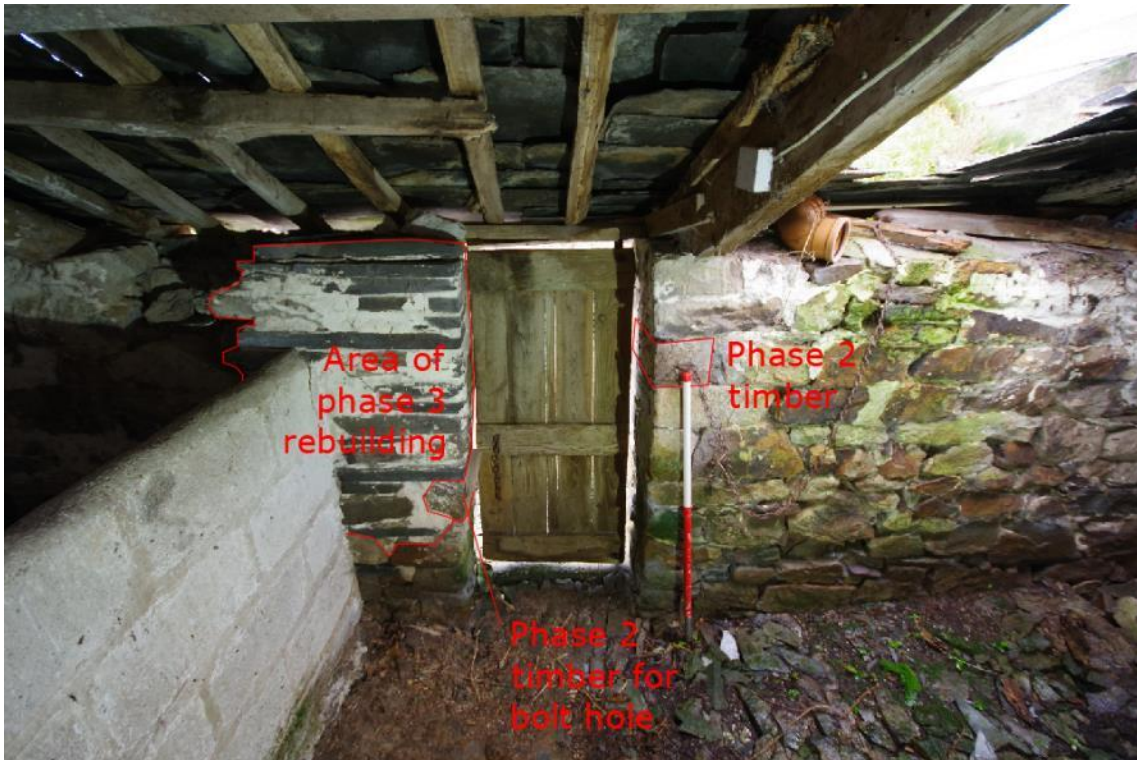
Fig 30 Northwest wall of the piggery showing door C.
