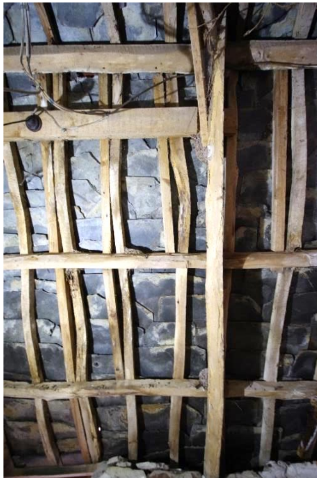
Fig 39 Roof structure at the southwest end of the building.
