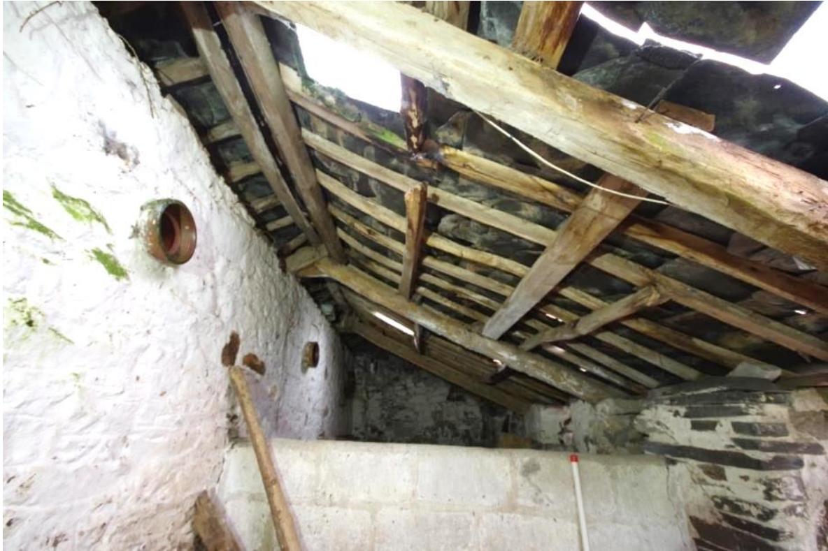
Fig 40 The roof structure looking southwest.
