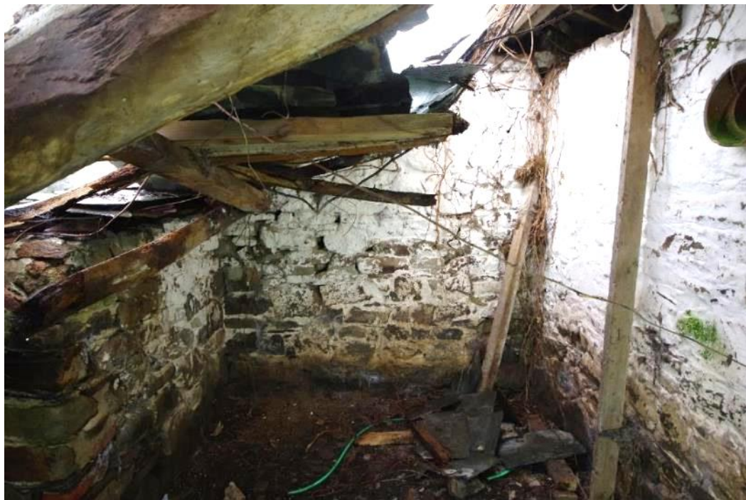
Fig 32 Northeast wall of the piggery.
