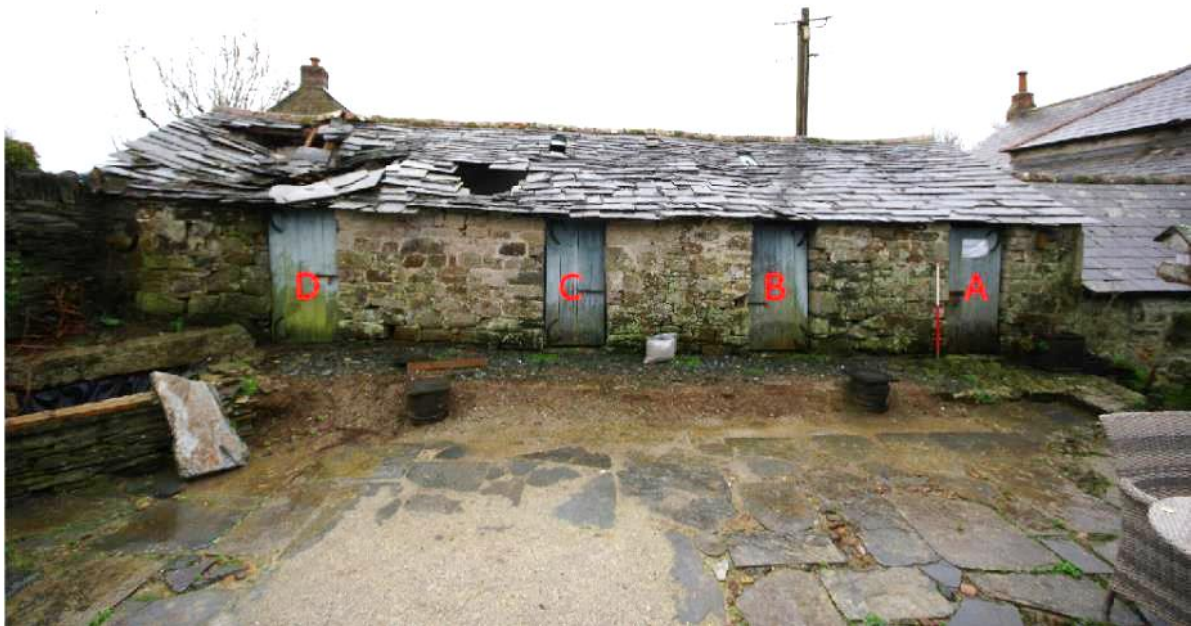
Fig 10 Northwest elevation showing location of doors A-D.
