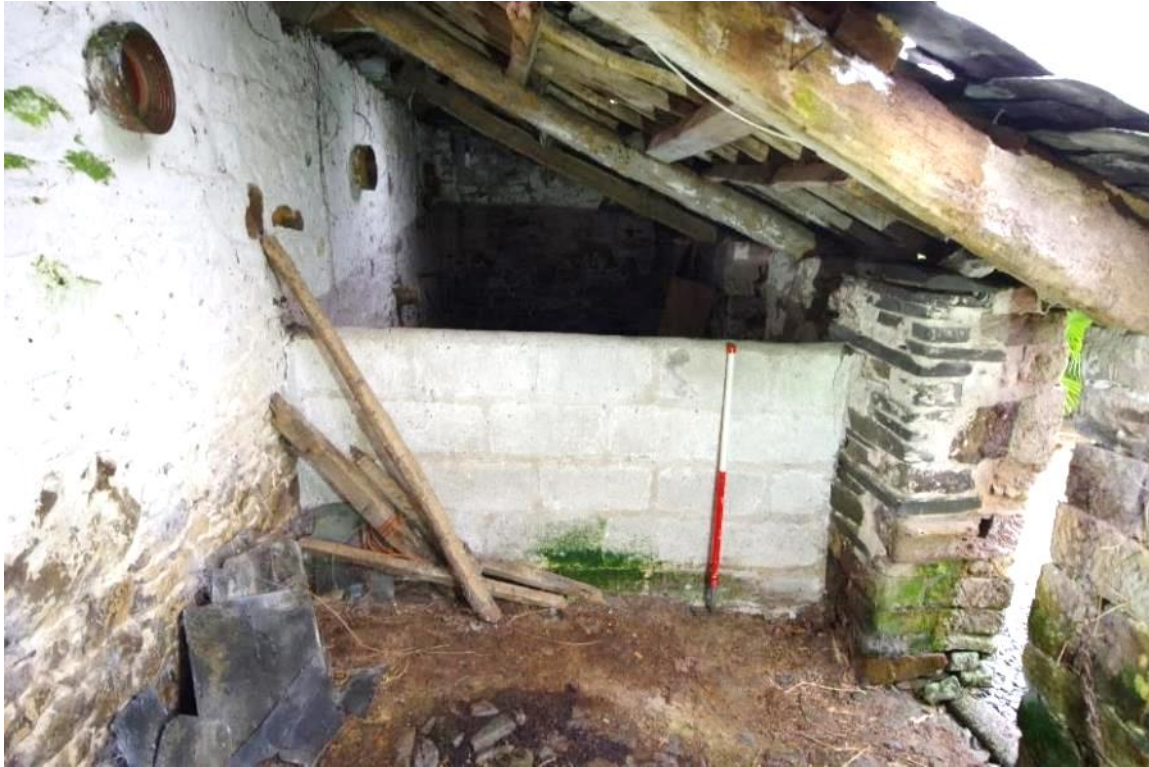
Fig 29 Inserted 20th century partition inside the piggery, looking southwest.
