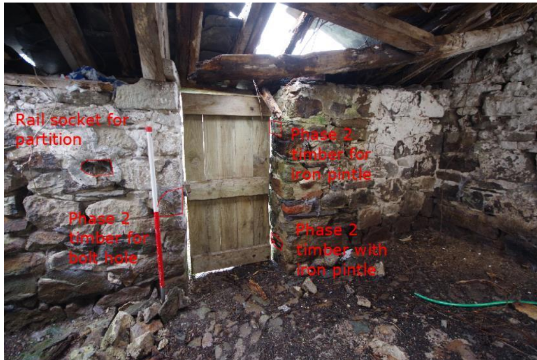
Fig 31 Northwest wall of the piggery showing door D.
