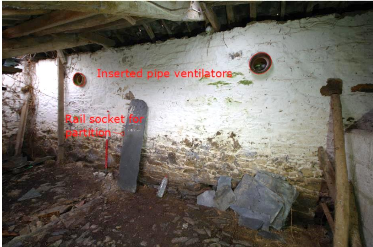
Fig 33 Southeast wall of the piggery, northeast end.
