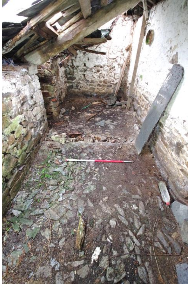
Fig 37 The floors of pens C and D looking northeast.
