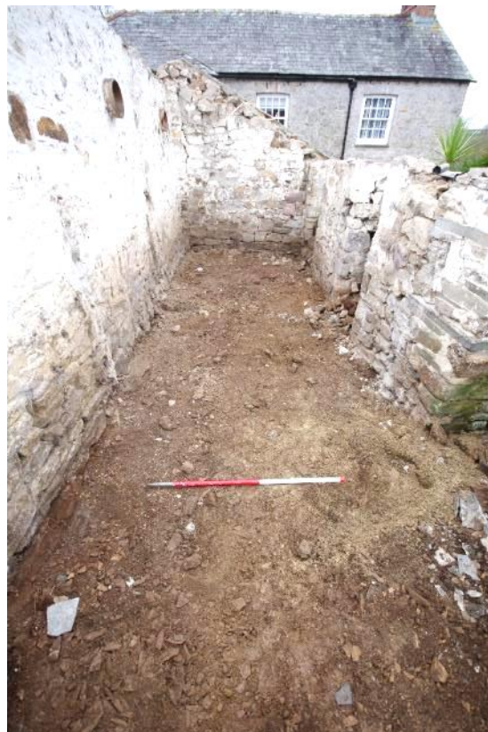
Fig 46 View looking southwest following the removal of the floor.
