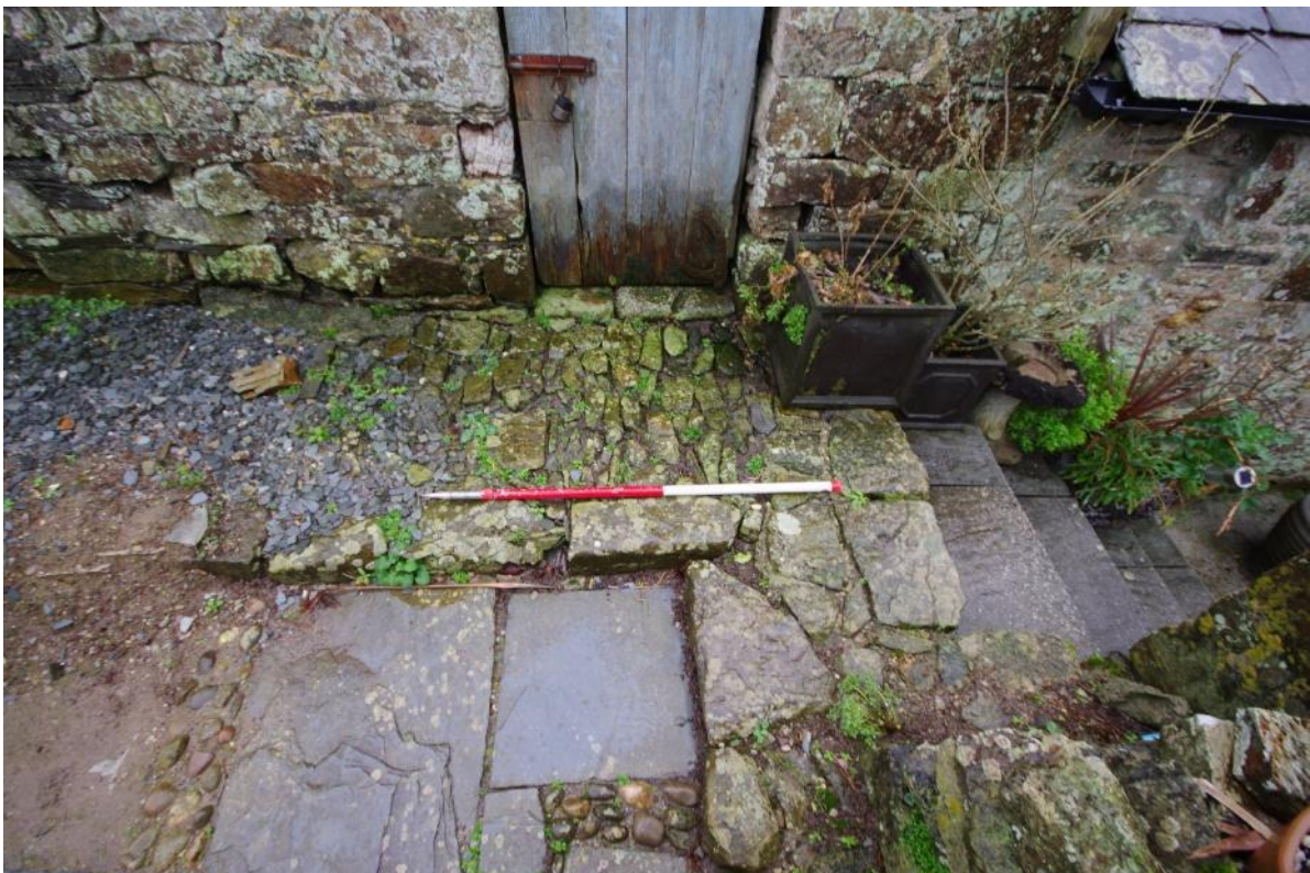
Fig 11 Stone setts outside Door A.
