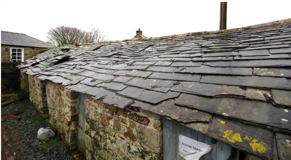
Fig 24 Roof looking east.
