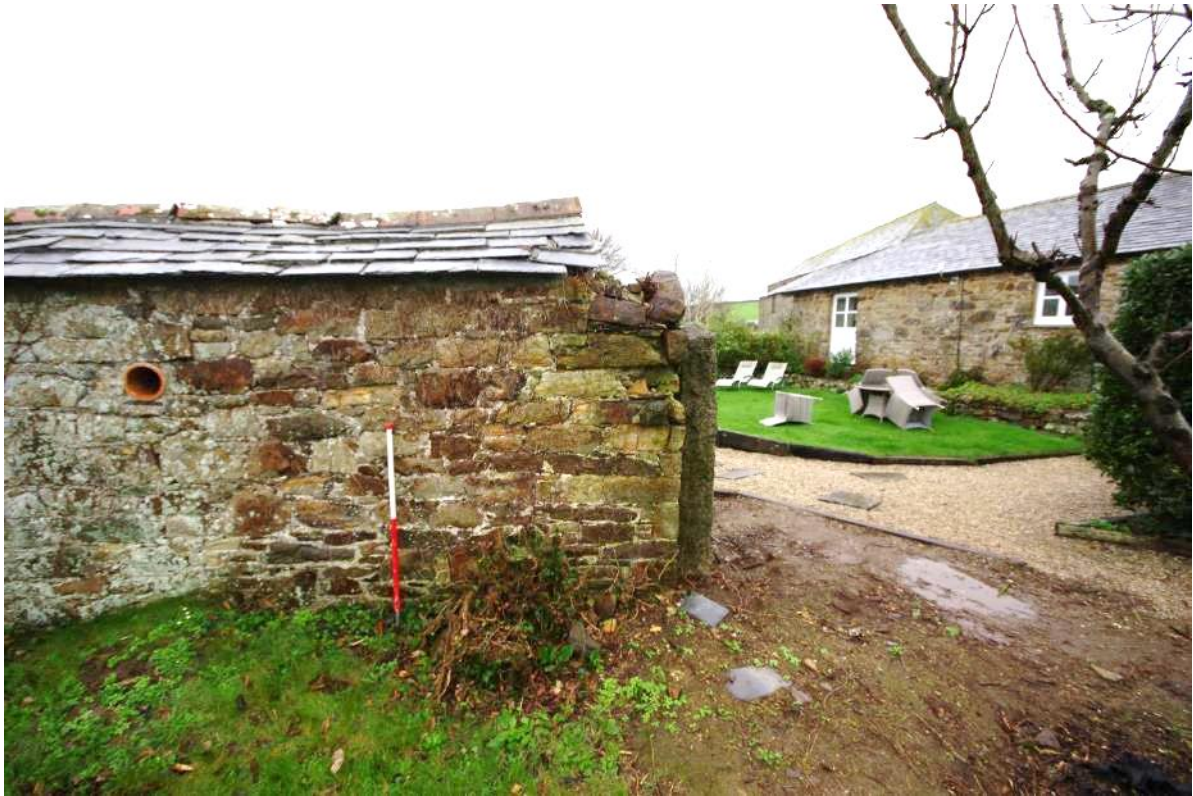
Fig 19 Northeast end of the southeast elevation.
