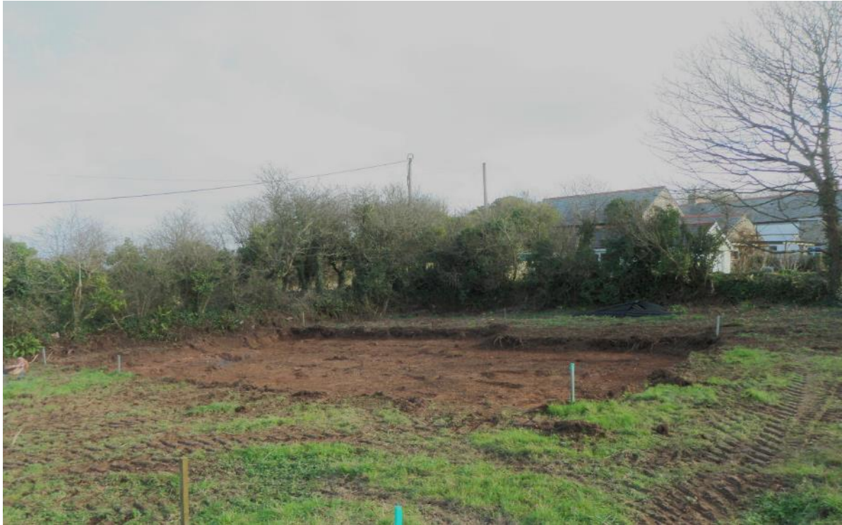
Fig 8: Looking southeast across the stripped House 1 footprint.
