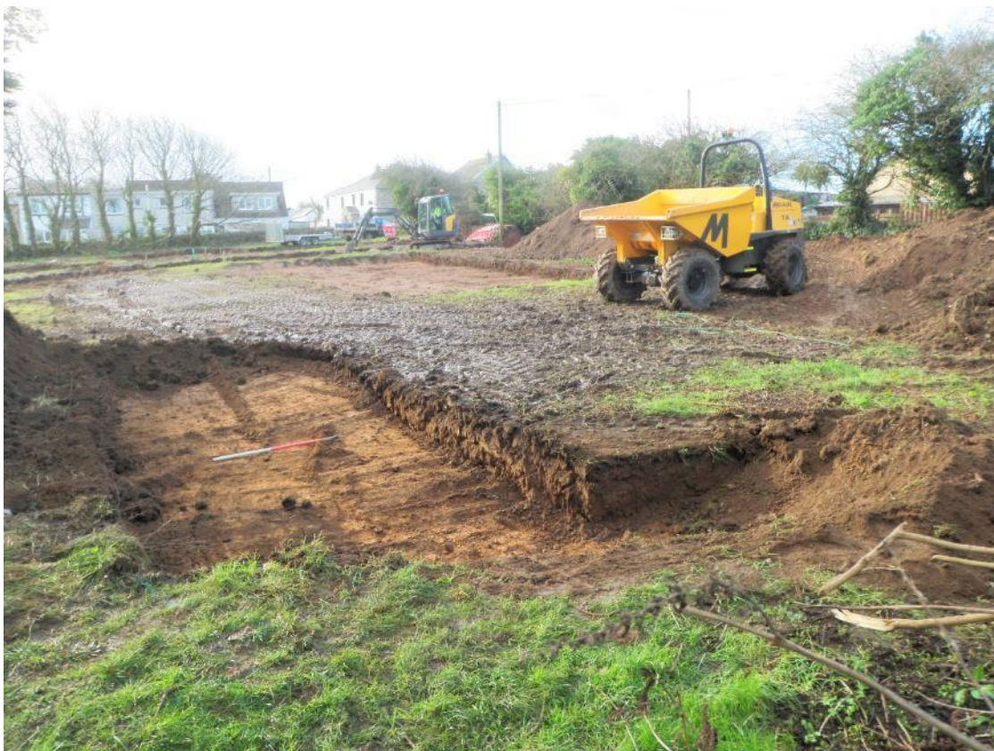
Fig 17: Looking south across the combined sewage treatment area during excavation.
