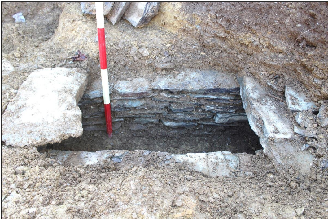
Fig 20 North facing side of culvert 124, looking south.
