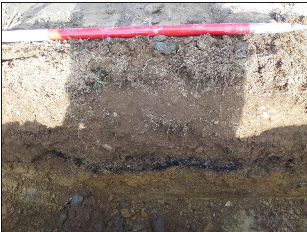
Fig 50 Tarmac layer in lower section of Trench 7, looking north.
