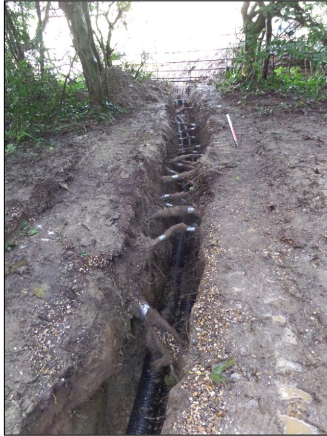
Fig 43 Trench 6, vac-ex section, post-ex, looking south.
