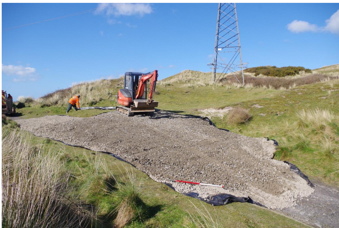
Fig 35 Full extent of temporary surfacing by pylon.
