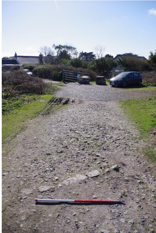
Fig 32 Looking southeast along the track showing remains of drain in foreground.
