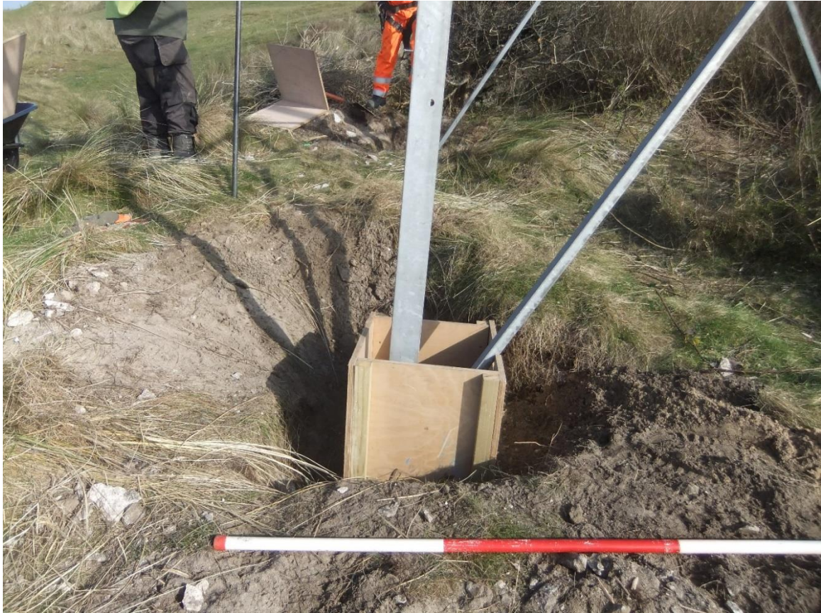
Fig 38 Southwest leg of the new pylon.
