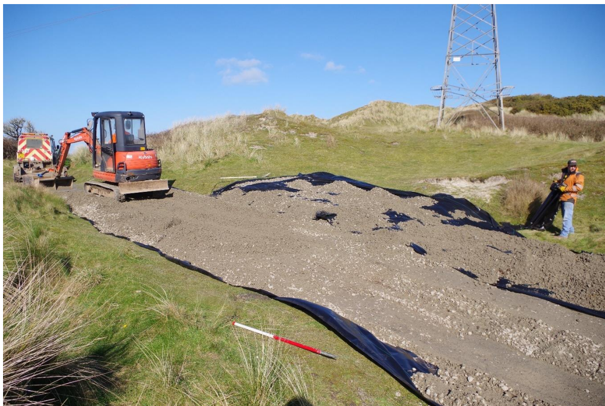
Fig 34 Extended temporary surface next to the pylon.
