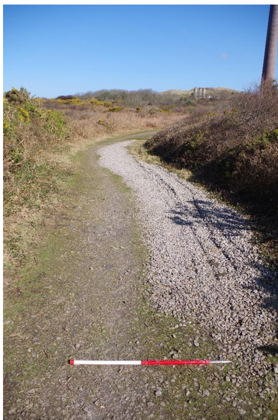
Fig 25 Looking northeast along the track towards the chimney.
