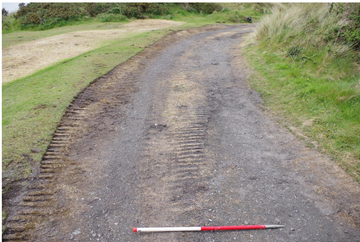
Fig 42 Bend in track before pylon after works looking west.
