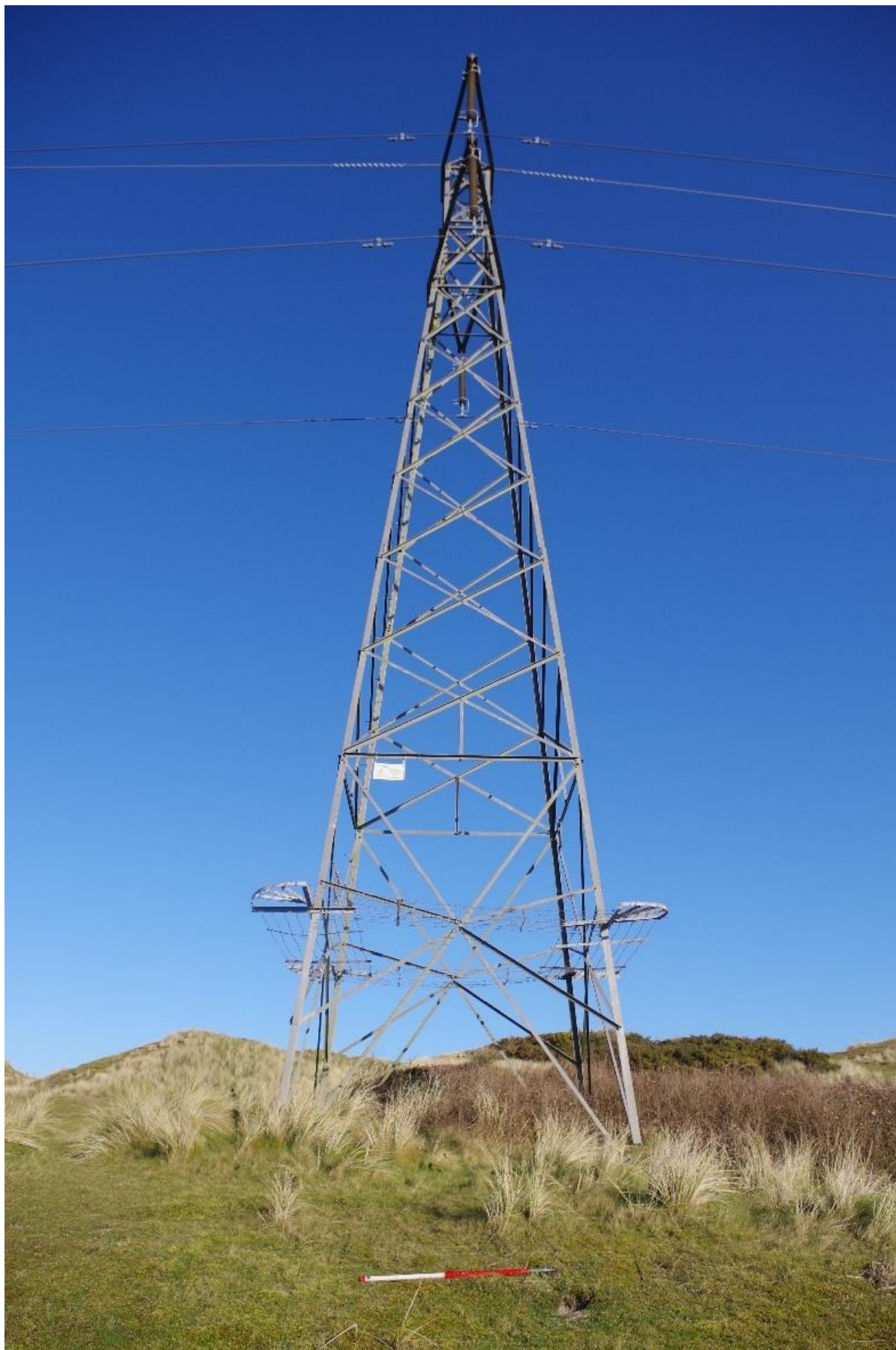
Fig 7 The pylon prior to removal looking north.
