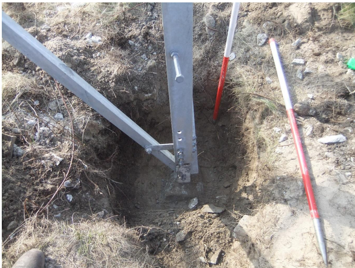
Fig 37 Northwest leg of the new pylon.
