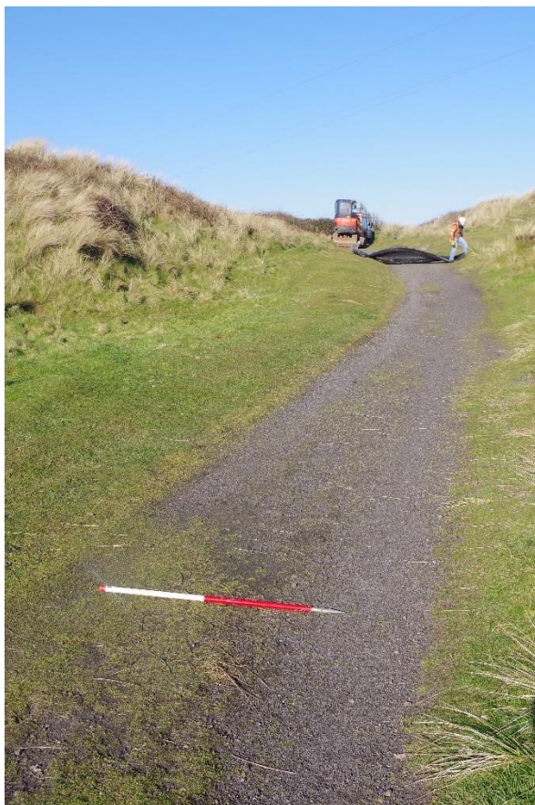
Fig 10 Track in front of the pylon looking west.
