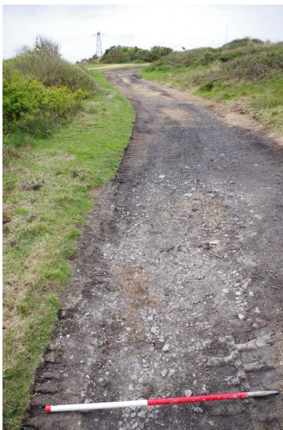
Fig 41 Area of small temporary surface after removal looking west.
