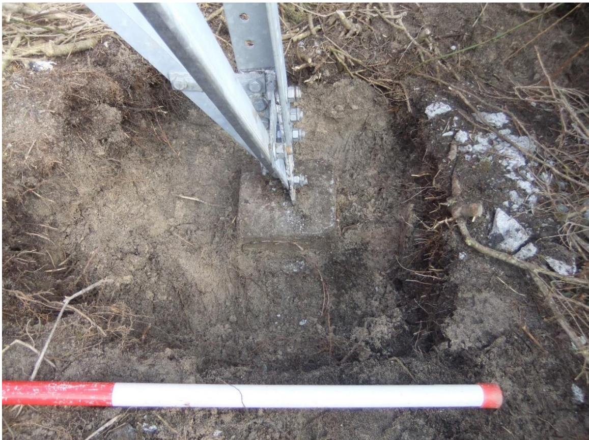
Fig 39 Northeast leg of the new pylon.
