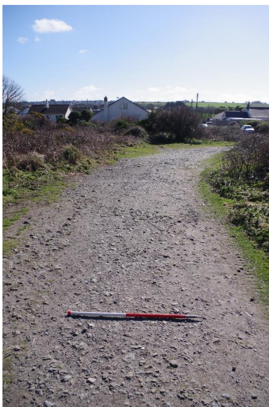
Fig 31 Looking southeast along the track.
