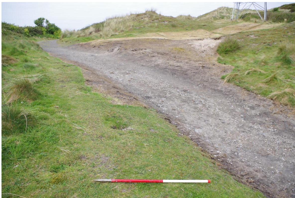
Fig 43 Area in front of pylon after removal of temporary surface.
