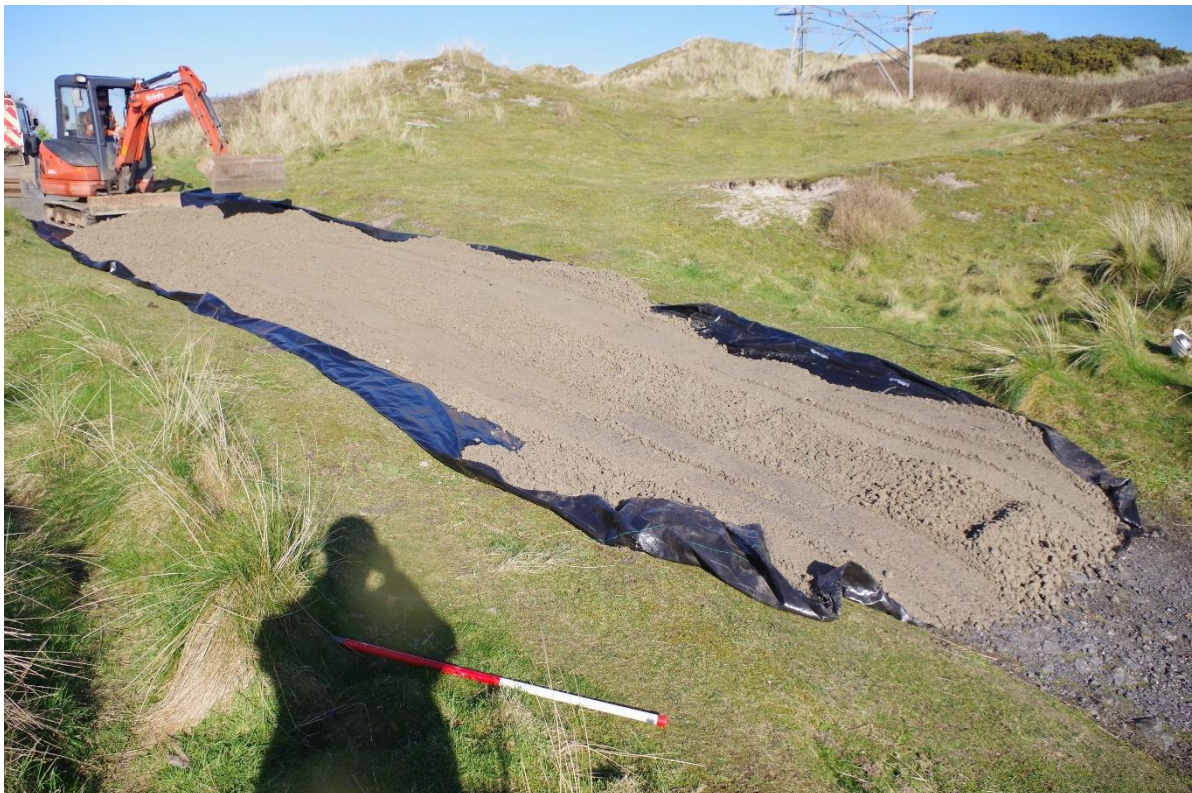
Fig 33 First stretch of temporary surface.
