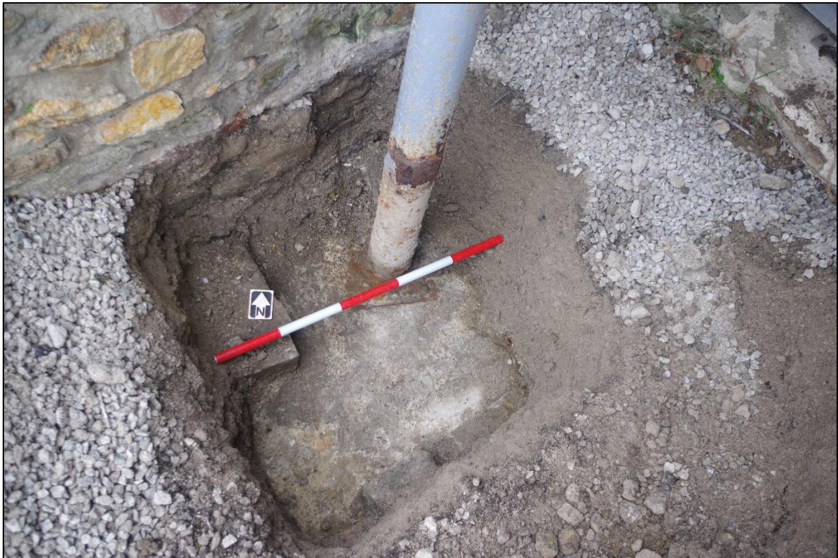
Fig 12 TP-1 (showing lime floor at base).
