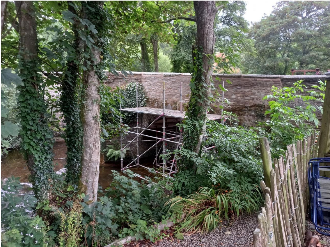
Fig 37 West elevation of new parapet and spandrel wall following reconstruction.
