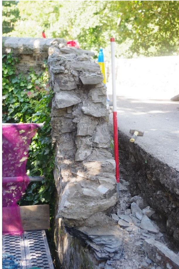
Fig 29 (36) South facing section of parapet wall.
