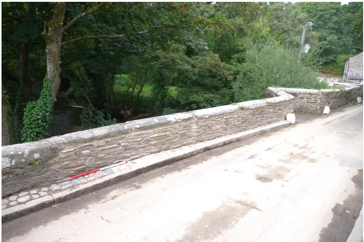
Fig 34 (41) East elevation of new parapet wall following reconstruction looking north west.
