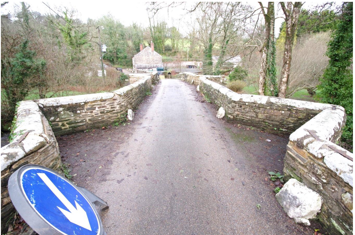
Fig 12 (27) Looking north along the bridge.
