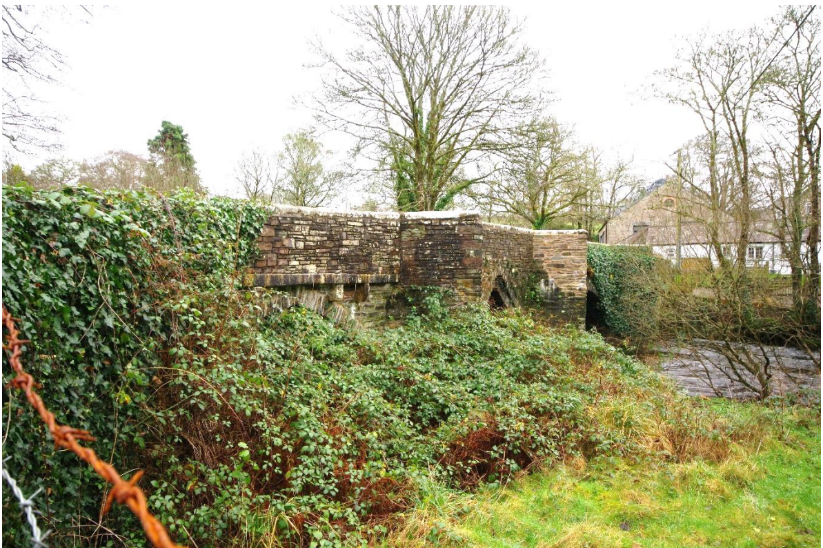
Fig 14 (35) The west elevation of the bridge looking south.
