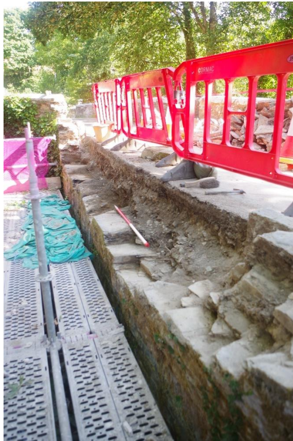
Fig 32 (39) Area of removed walling looking north.
