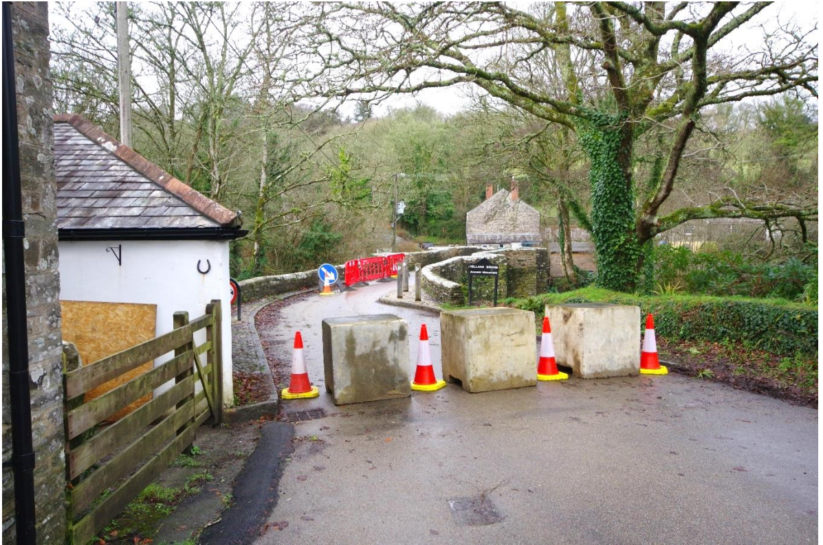
Fig 11 (19) The southern approach to the bridge looking north.
