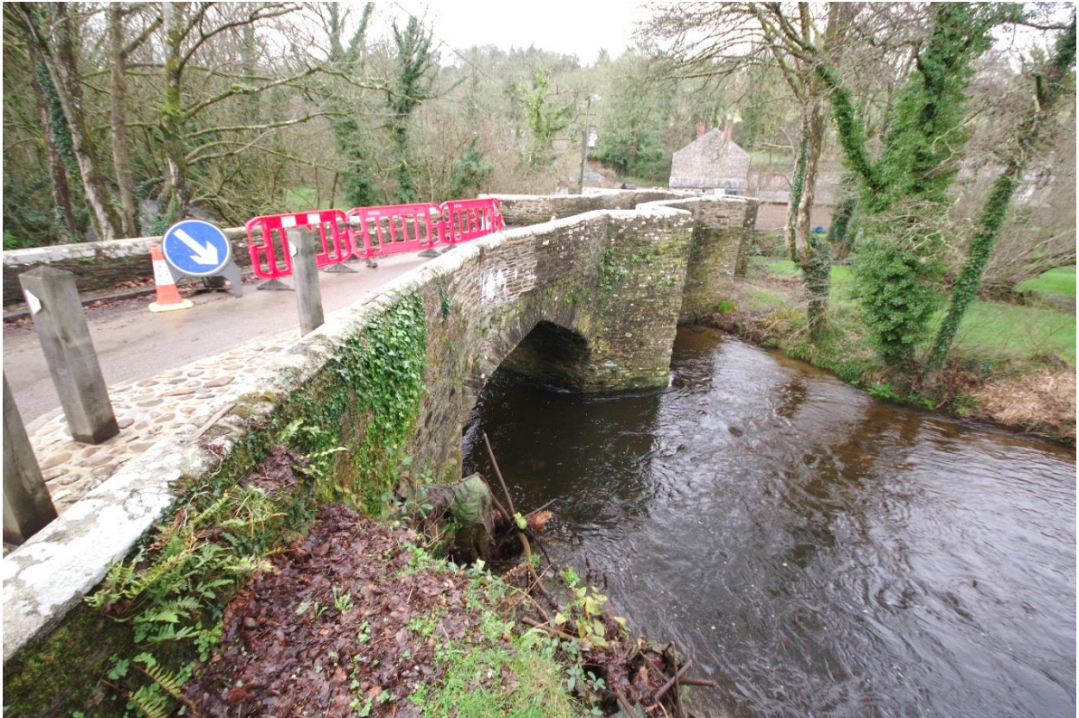
Fig 15 (34) East elevation of the bridge looking north.
