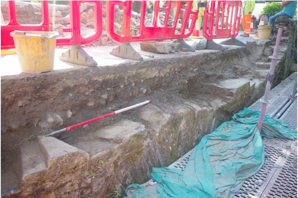
Fig 31 (38) West facing section exposed beneath the road surface, also showing the top of the arch and spandrel walls.
