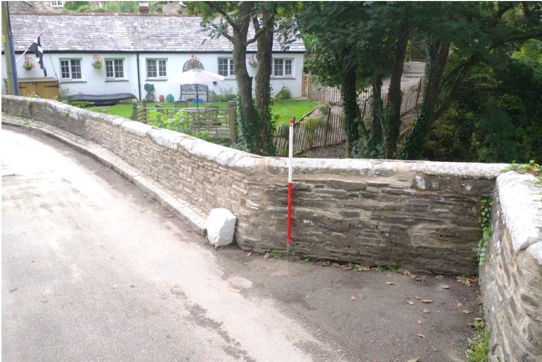
Fig 35 (42) East elevation of new parapet wall following reconstruction looking south west.
