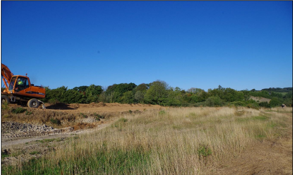
Fig 4 Looking south-west across the site area prior to excavation.
