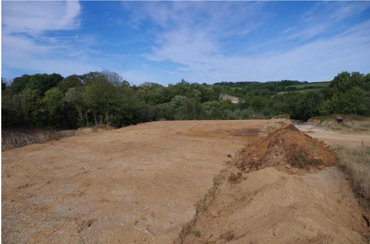
Fig 6 Stripping of the western section of the site, looking west.
