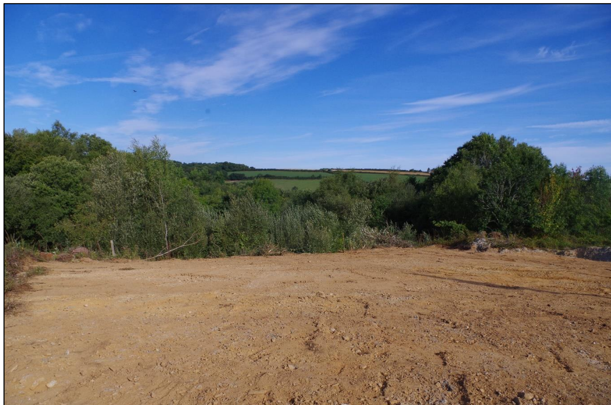
Fig 7 Stripping of the western section of the site, looking west.
