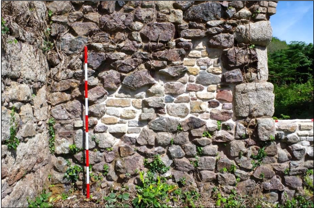
Fig 65 Interior south-west wall of boiler house following patch repairs.
