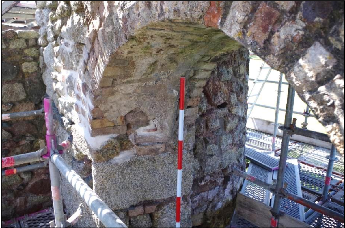
Fig 57 Interior south-west engine house wall following patch repair to arch.
