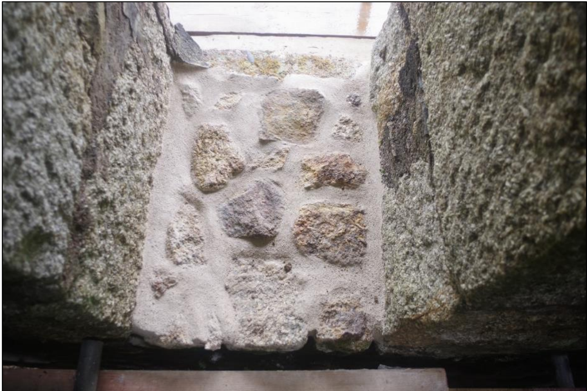
Fig 105 Interior south-west wall, small patch repair to window sill.
