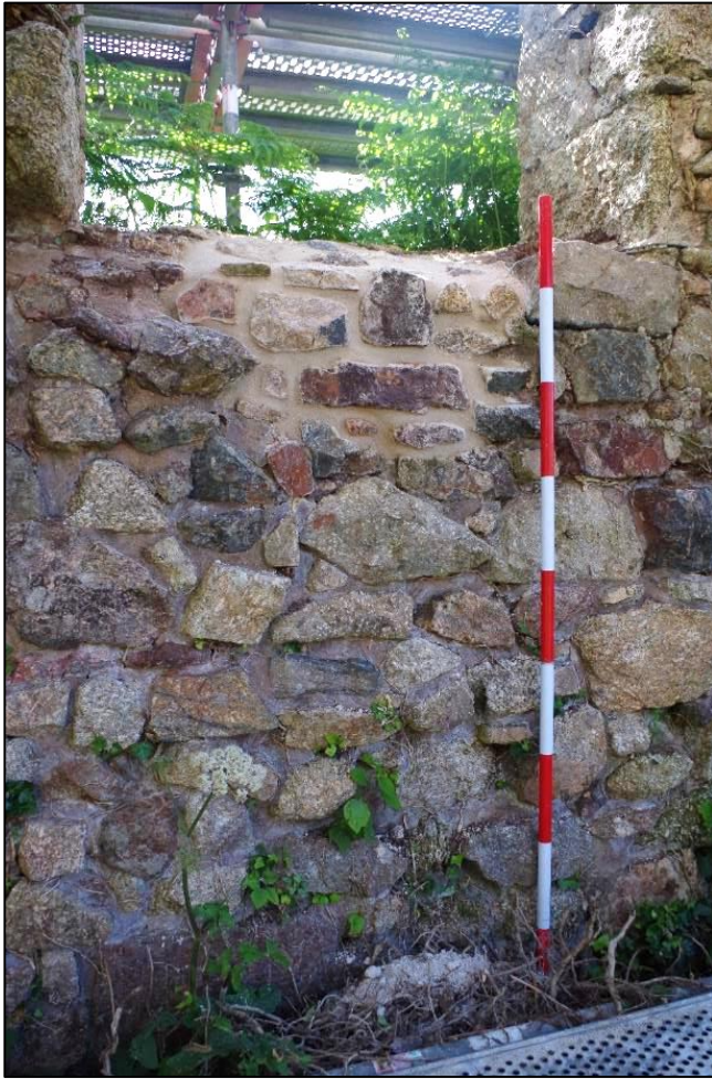
Fig 47 Interior south-east wall of the boiler house following patch repair.
