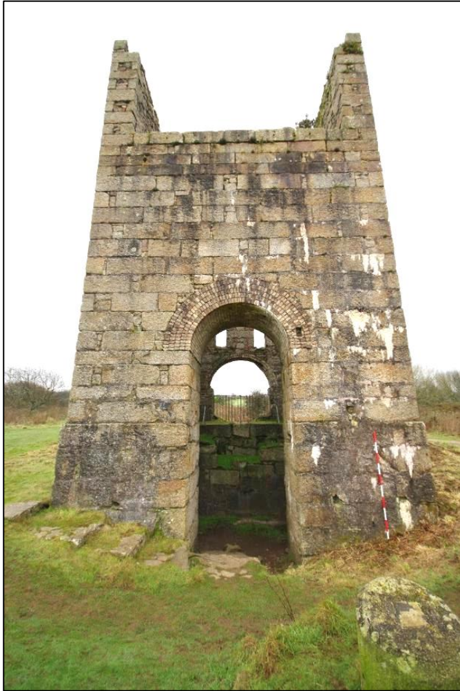
Fig 81 North-west elevation, bob wall.
