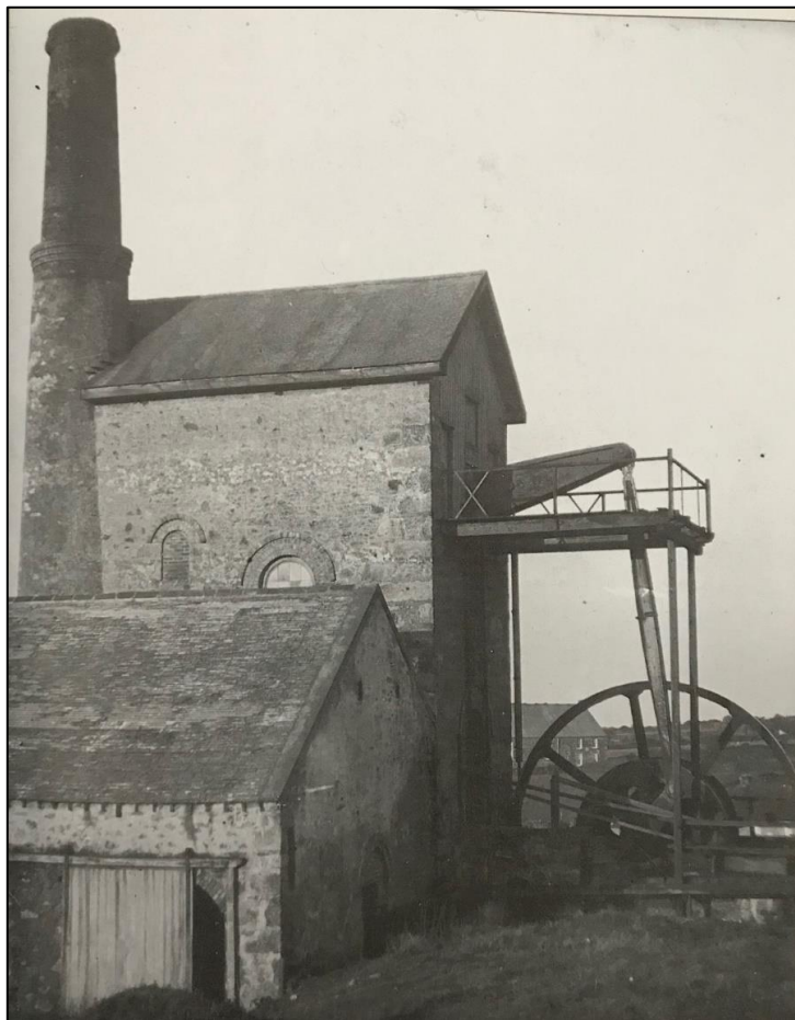
Fig 8 Pascoe's winding engine house c1880 photograph (Trounson and Bullen 1999).
