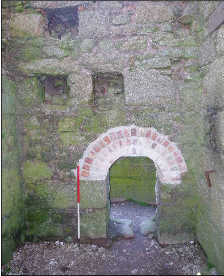
Fig 25 Interior north-west cataract pit wall following reconstruction of brick arch.
