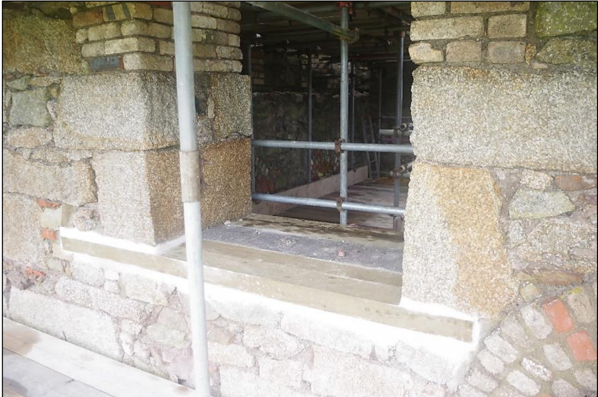
Fig 79 Exterior north-east elevation, repairs to main girder slot sill.
