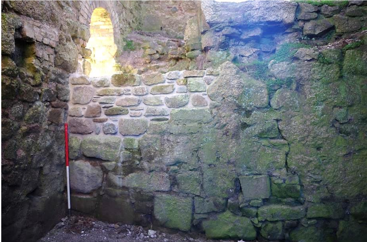
Fig 69 Interior cylinder bed following remedial works.
