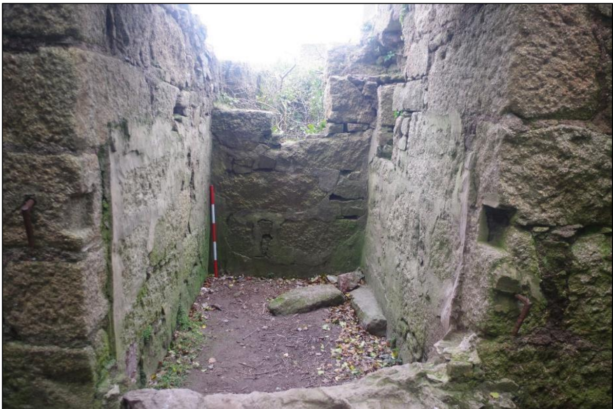
Fig 18 Interior looking north-east into condenser pit before remedial works.
