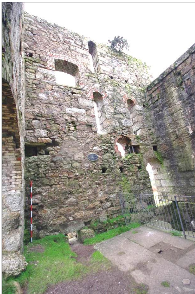
Fig 100 Interior south-west wall before remedial works.
