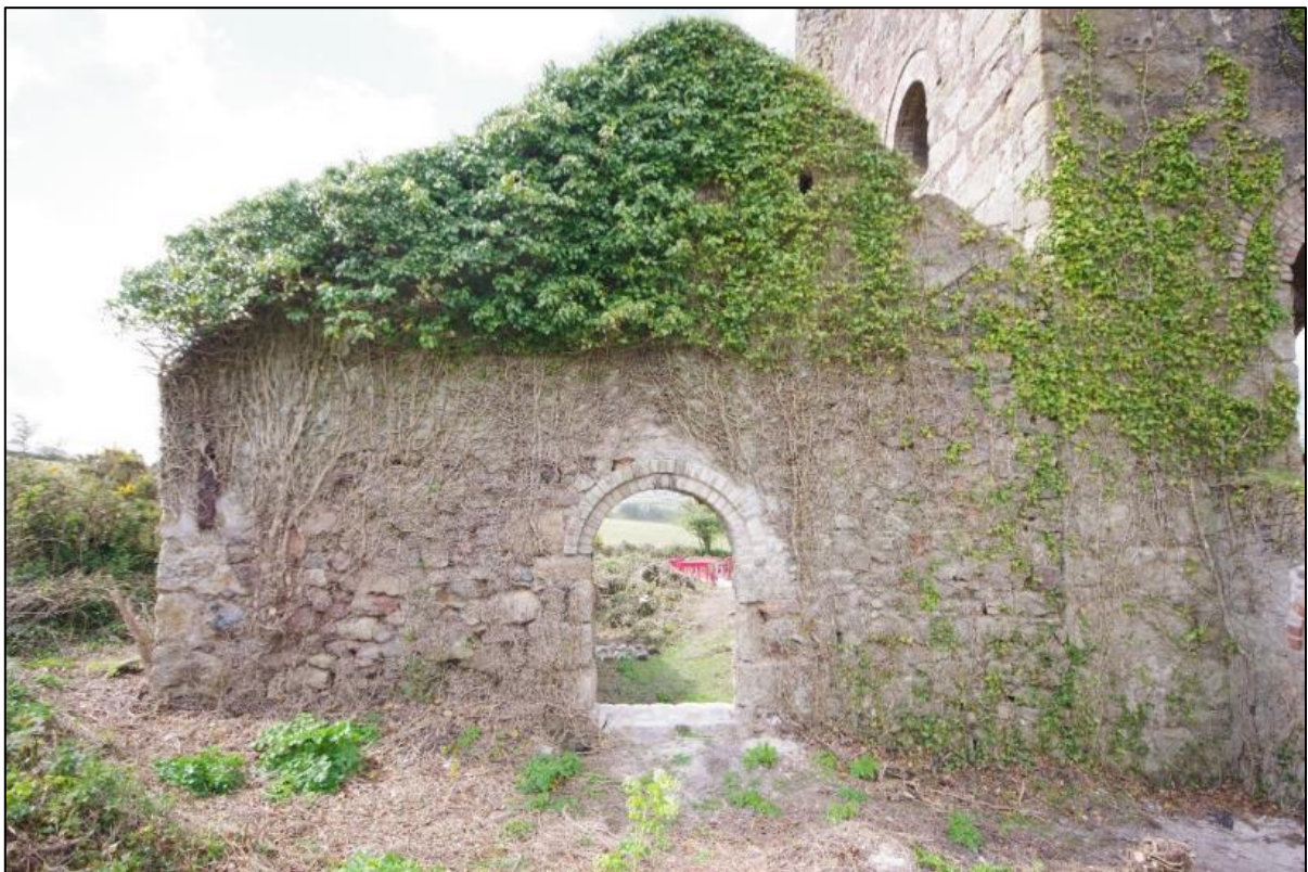
Fig 16 North-east elevation following vegetation clearance and repair work to the arch over the boiler house window opening.
