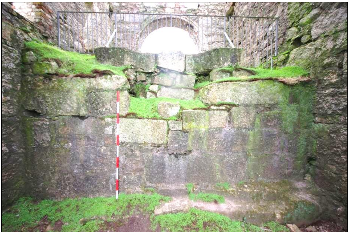
Fig 96 South-east wall of cataract pit (cylinder bed).
