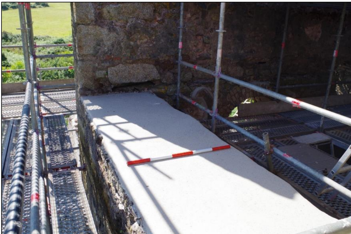
Fig 20 Top of bob wall following lime mortar capping.
