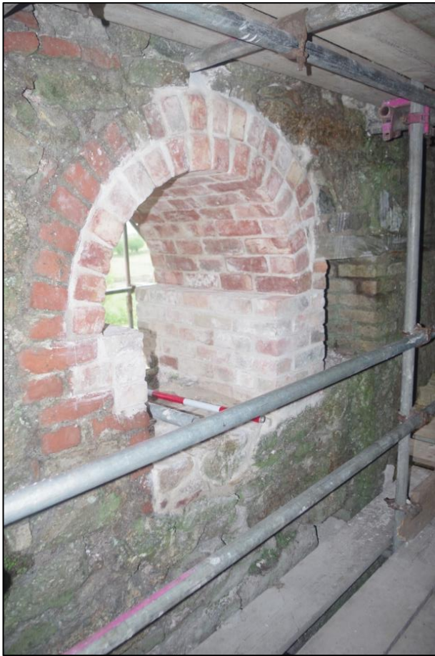
Fig 103 Interior south-west wall, reconstruction of arch.
