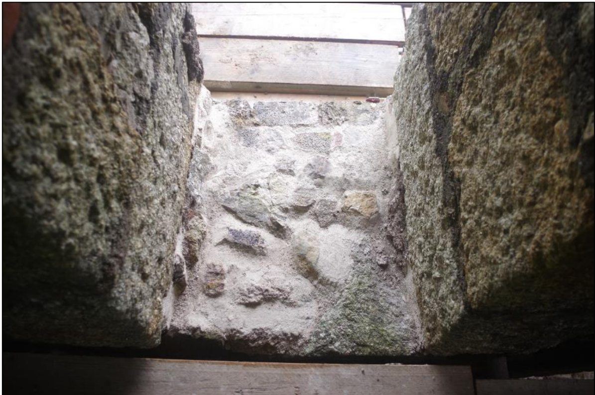
Fig 104 Interior south-west wall, small patch repair to window sill.
