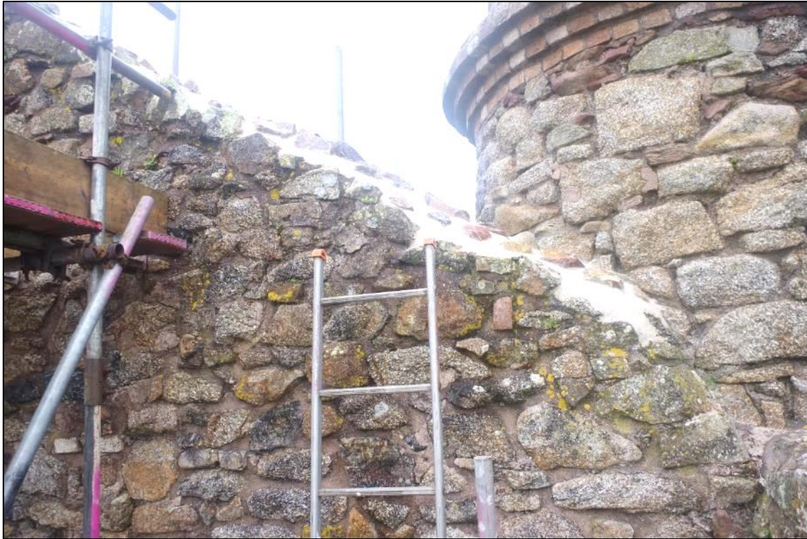
Fig 91 Interior south-east gable wall following capping.
