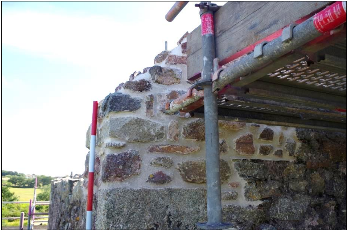
Fig 55 South-west gable end wall of engine house following patch repair.
