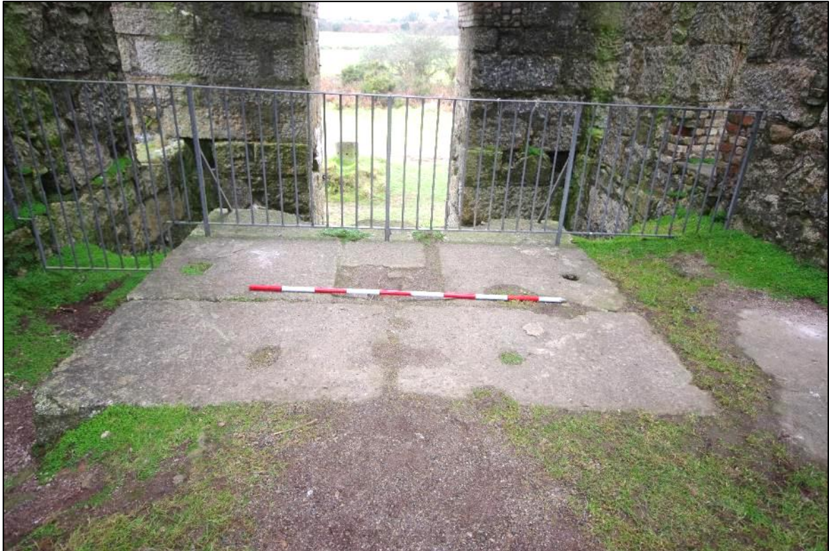
Fig 109 Cylinder bed with 1990s metal safety railings.
