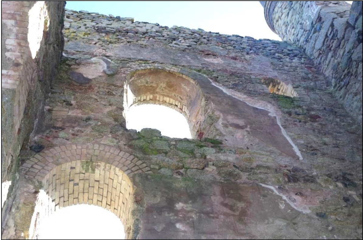
Fig 39 Interior south-east wall following patch repairs.
