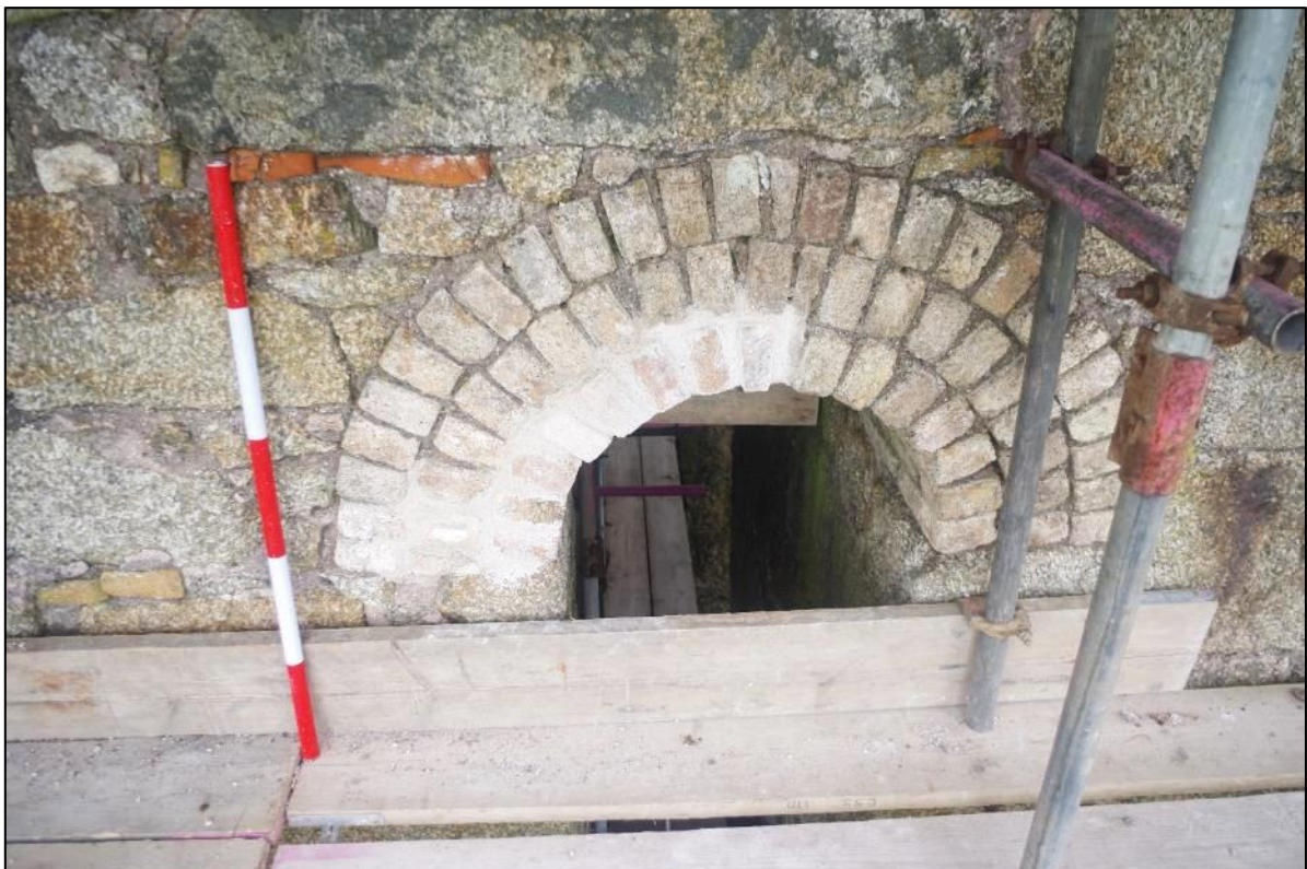
Fig 80 Exterior north-east elevation, repairs to window arch.
