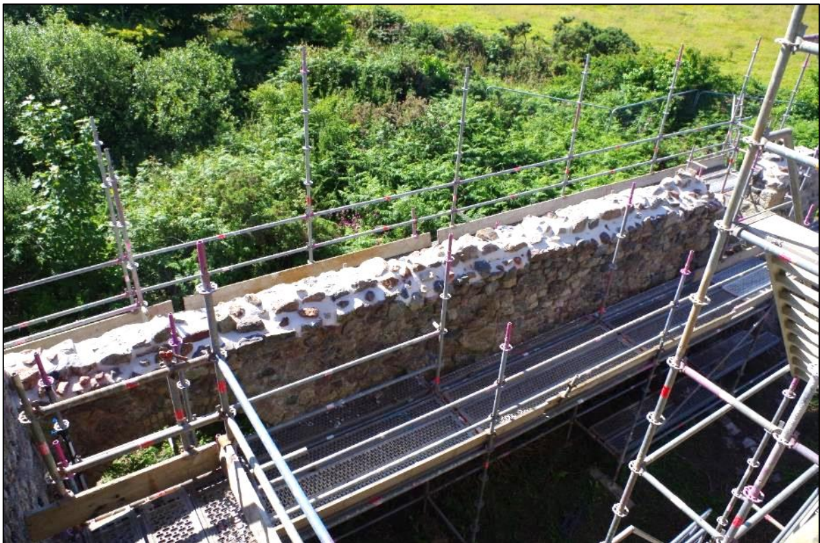
Fig 44 South-east wall of the boiler house following lime mortar capping.
