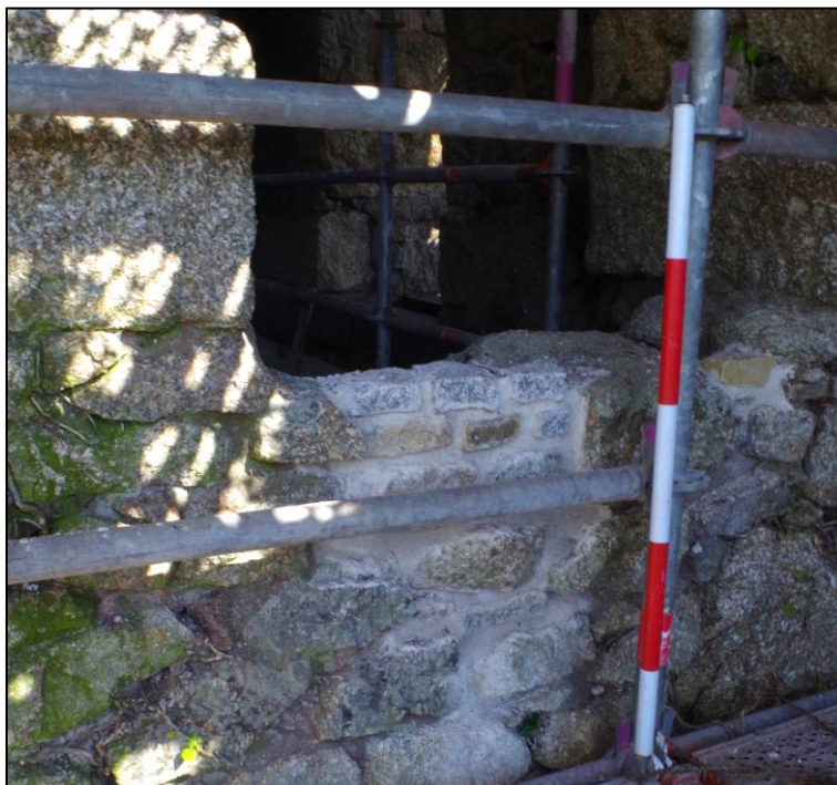
Fig 32 South-east elevation following patch repairs.
