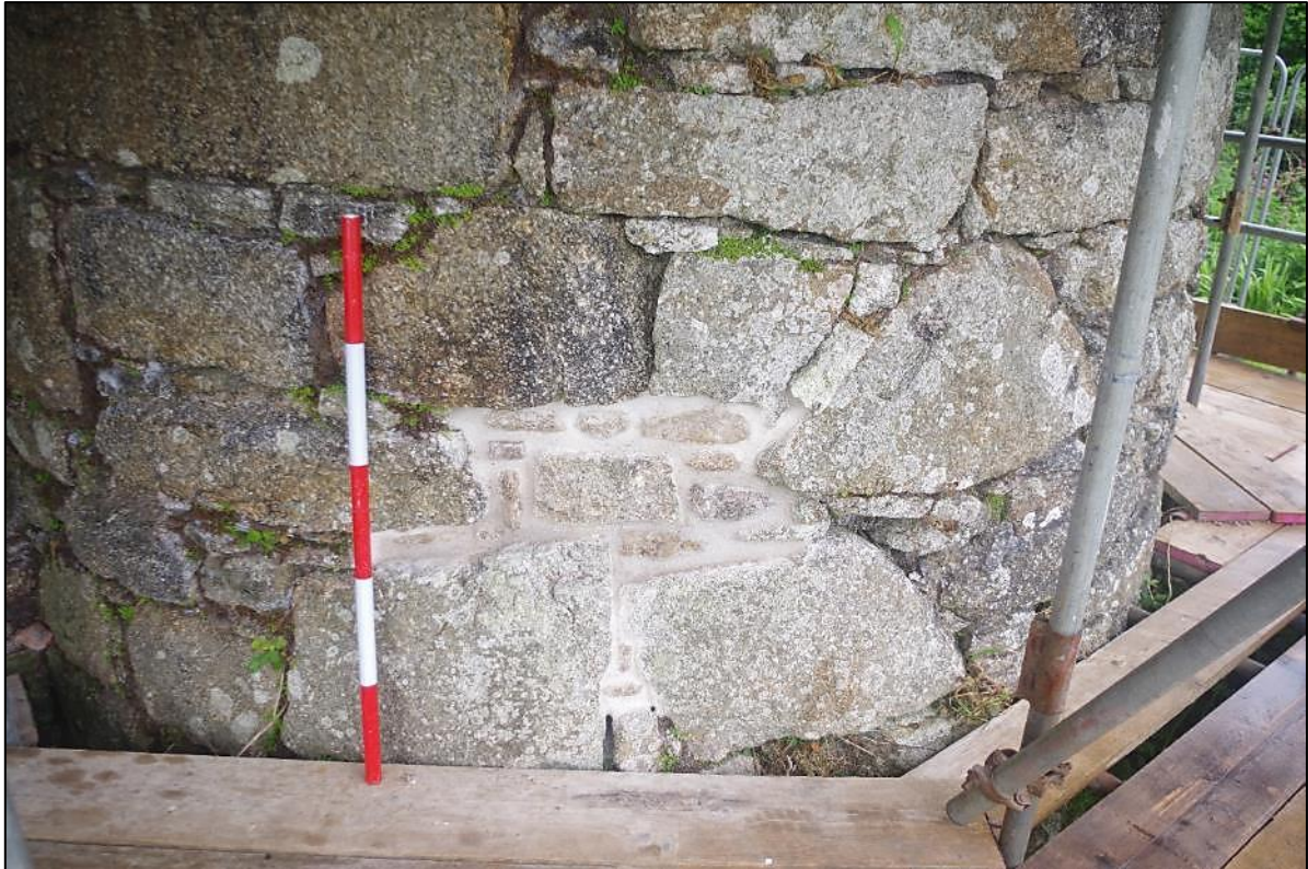
Fig 99 Small patch repair to chimney stack.
