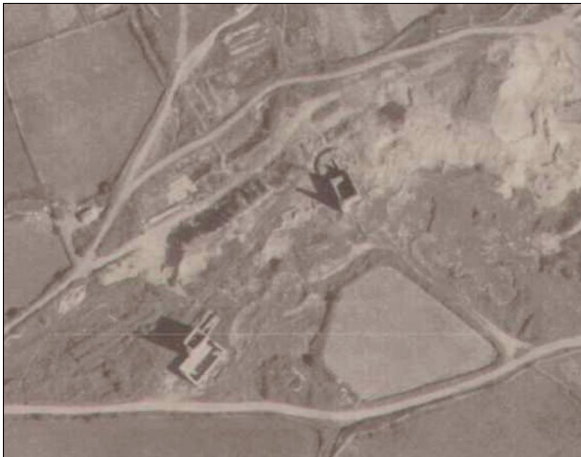
Fig 6 RAF aerial photograph taken in 1946 showing the roofless buildings.
