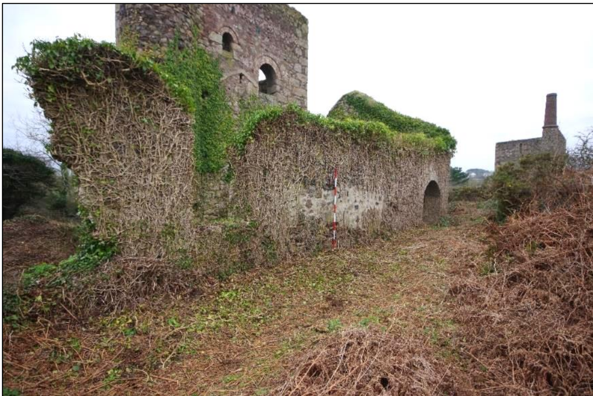
Fig 34 South-east elevation of the boiler house before remedial works.
