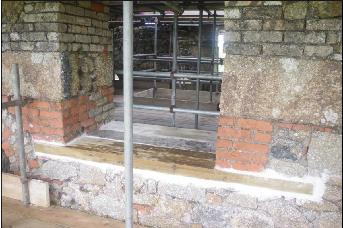
Fig 107 South-west elevation, replacement sill of main girder slot.
