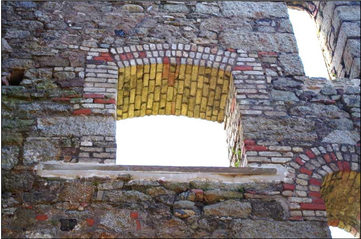
Fig 101 Interior south-west wall, replacement sill of main girder slot opening.
