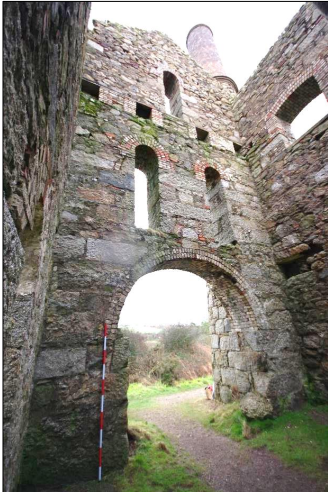
Fig 87 Interior south-east wall and cylinder arch before remedial works.
