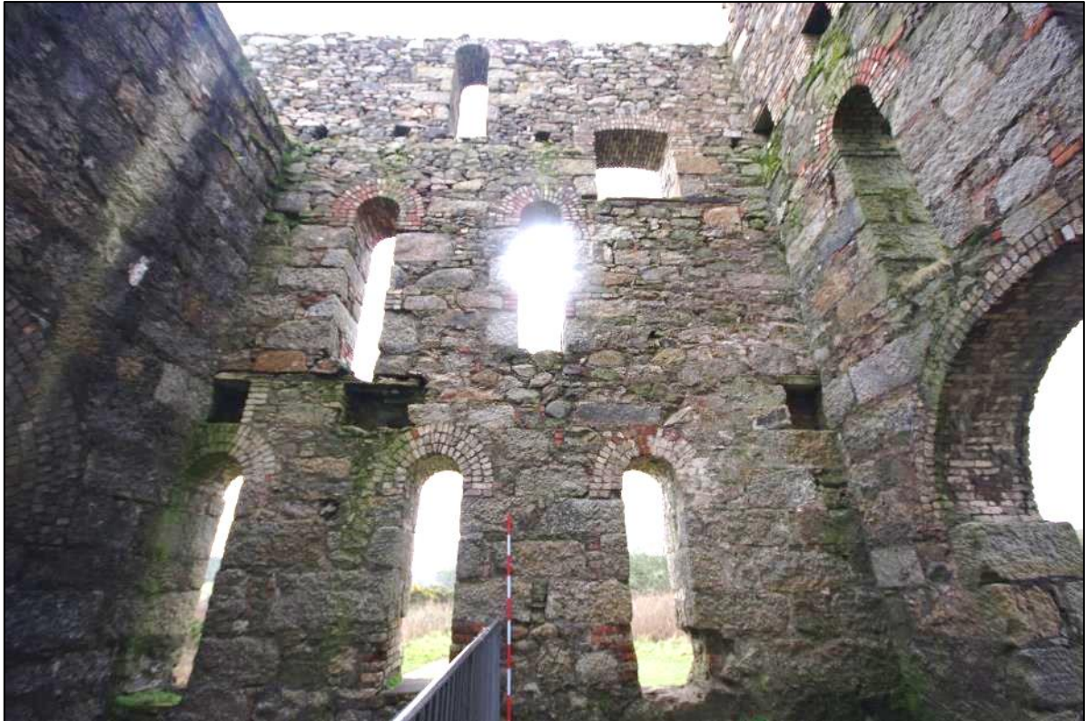
Fig 73 Interior north-east wall before remedial works.
