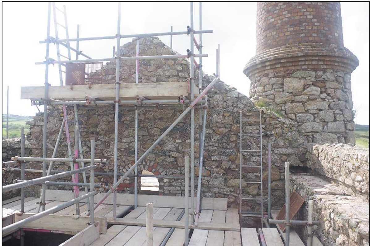
Fig 52 Interior south-west engine house wall before remedial works.
