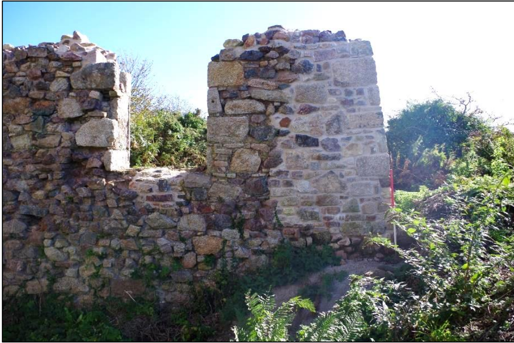
Fig 49 Interior south-east wall of the boiler house following patch repairs.
