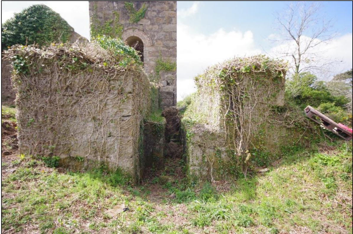
Fig 15 North-east elevation following vegetation clearance.
