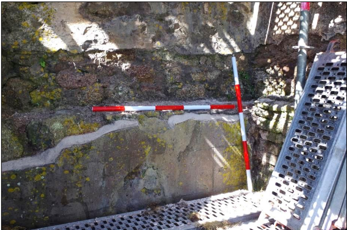
Fig 58 Interior south-west wall following small patch repair to incised plaster.
