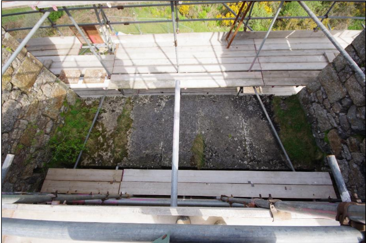
Fig 19 Top of bob wall before remedial works.
