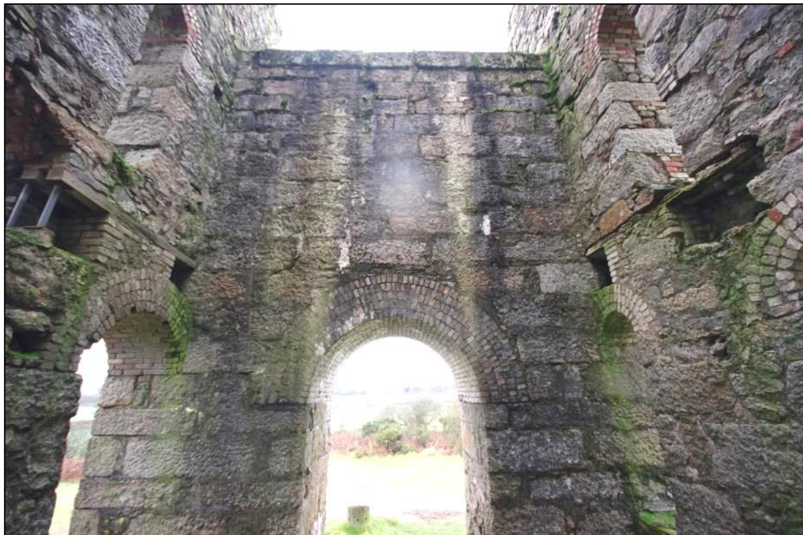
Fig 82 Interior north-west bob wall.
