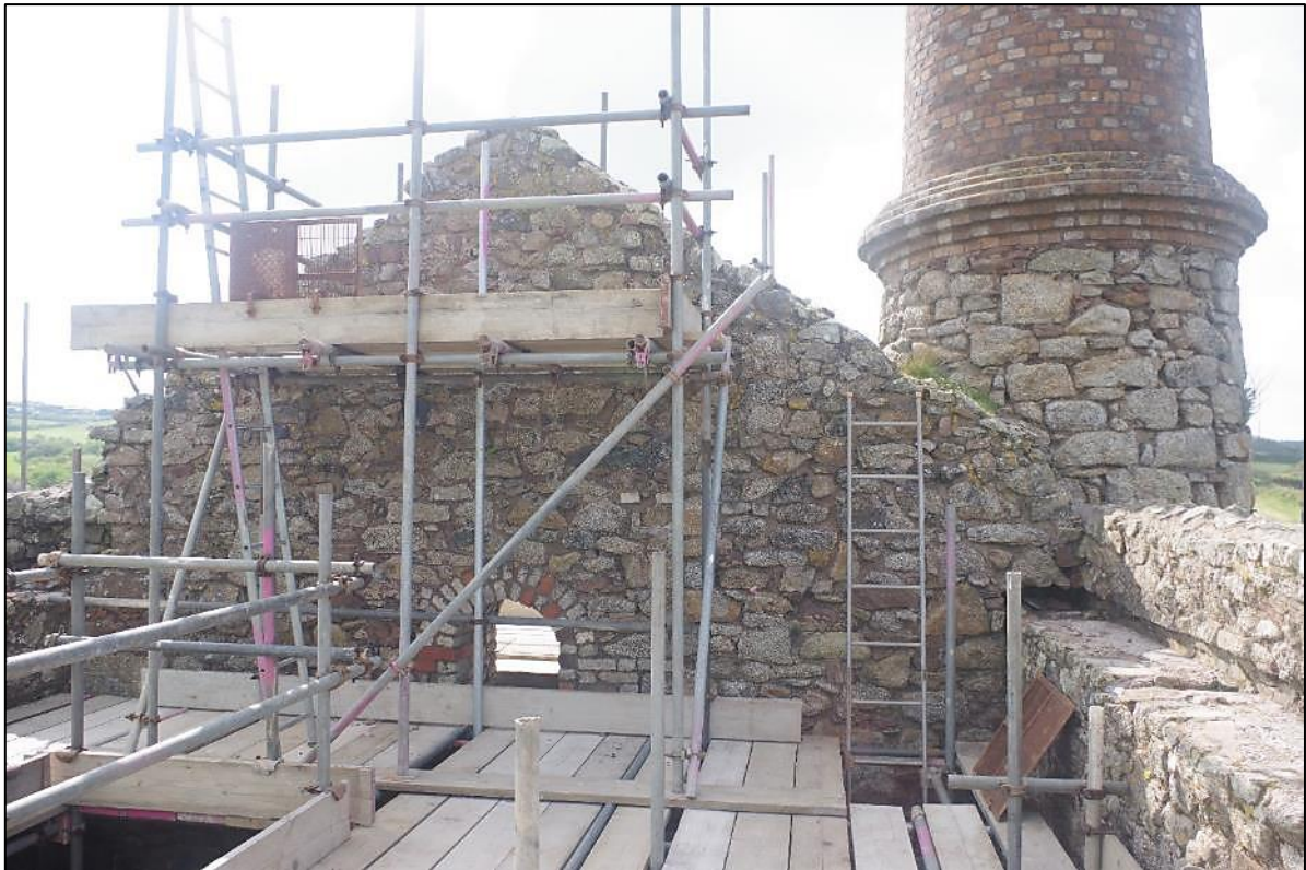
Fig 89 Interior south-east gable end before remedial works.
