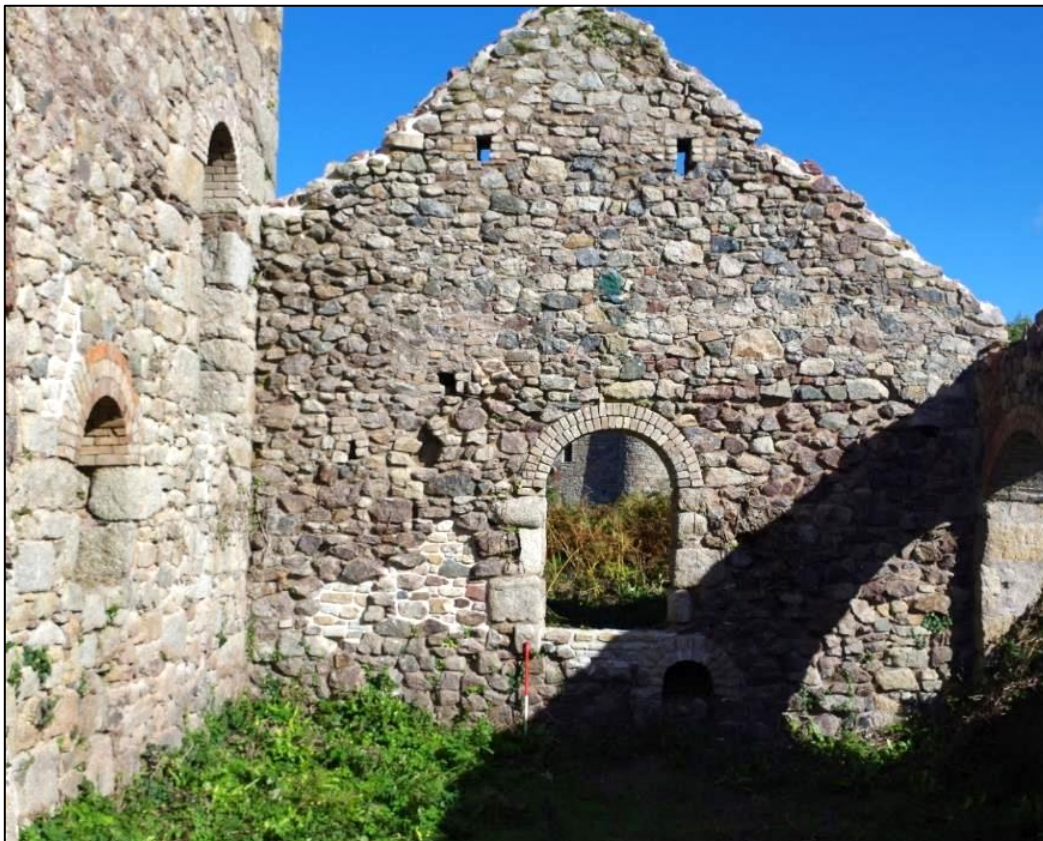
Fig 60 Interior south-west wall of boiler house following patch repairs.
