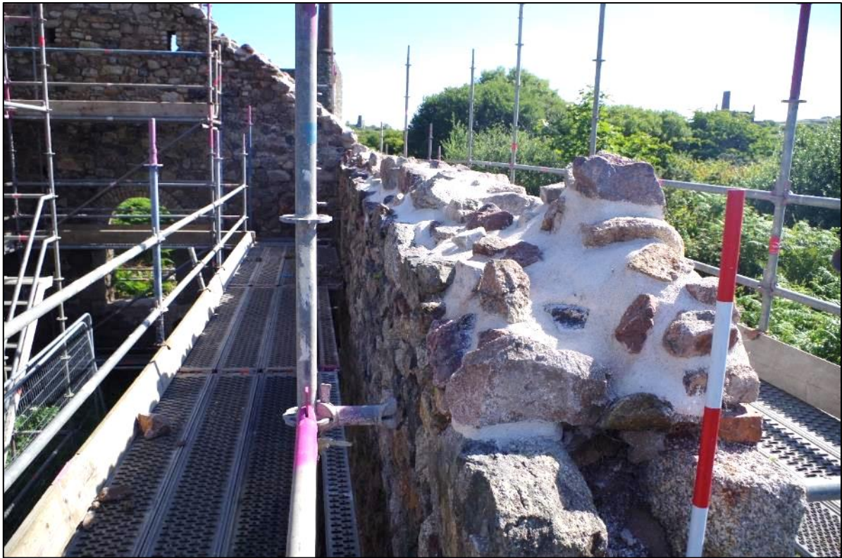
Fig 45 South-east wall of the boiler house following lime mortar capping.
