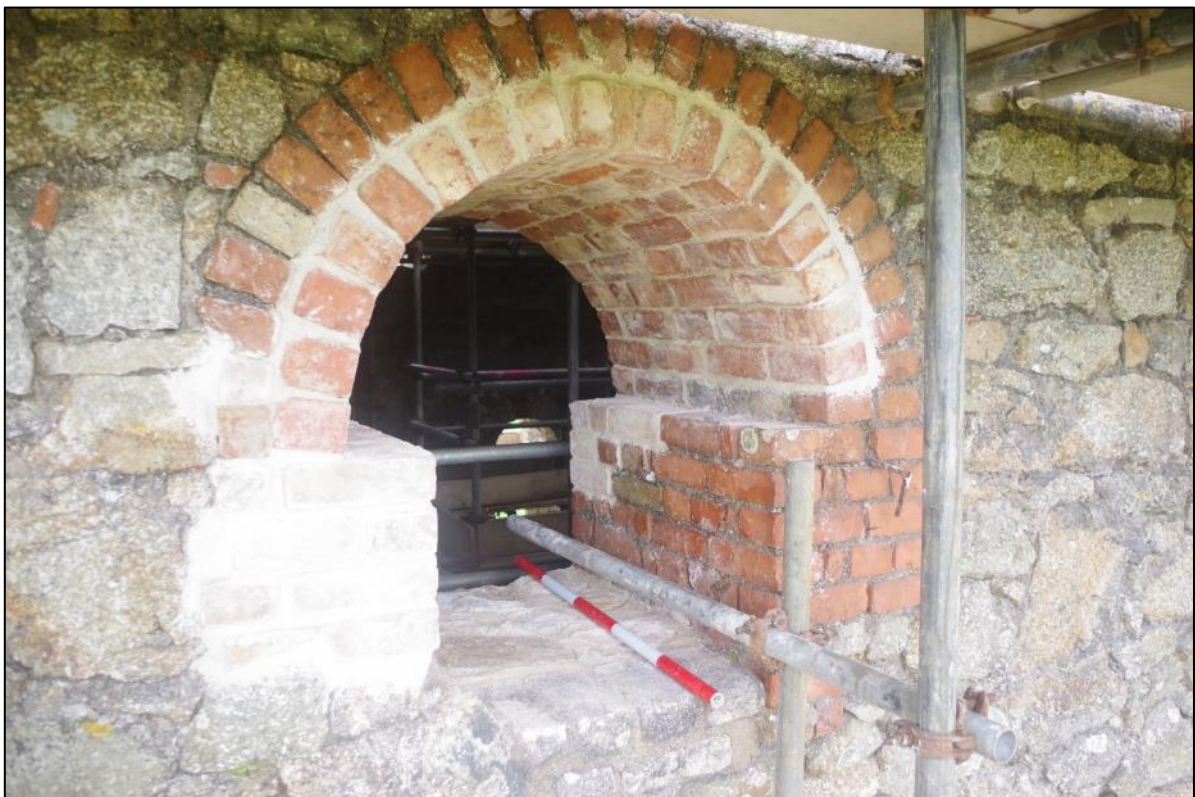
Fig 106 South-west elevation, view of arch reconstruction.
