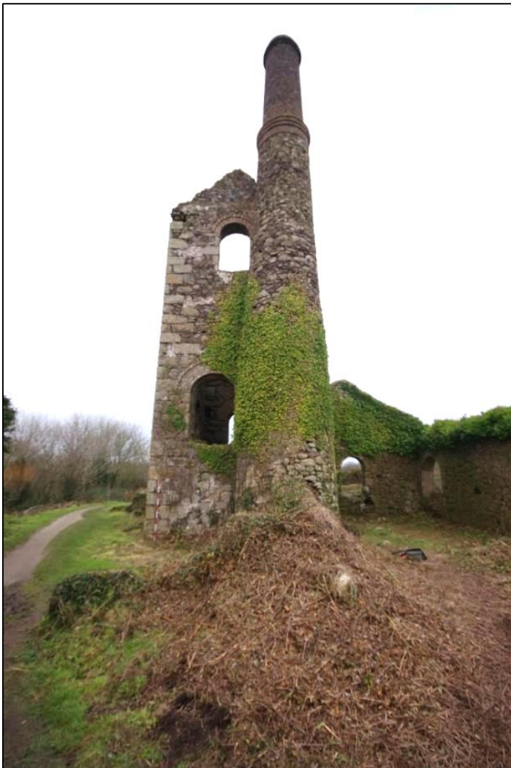
Fig 50 South-west elevation of the engine house before remedial works.
