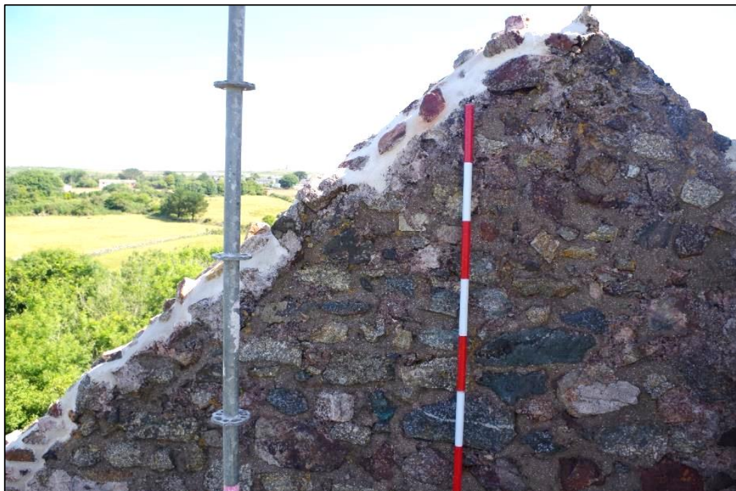
Fig 54 South-west engine house wall following gable end capping.
