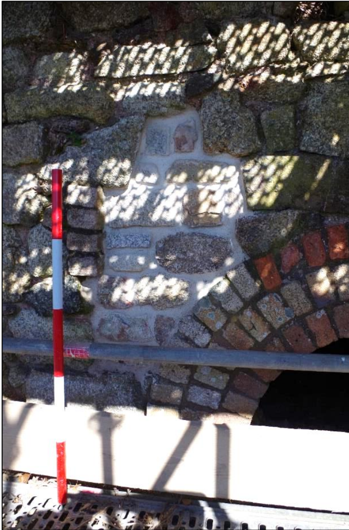
Fig 31 South-east elevation following patch repairs.
