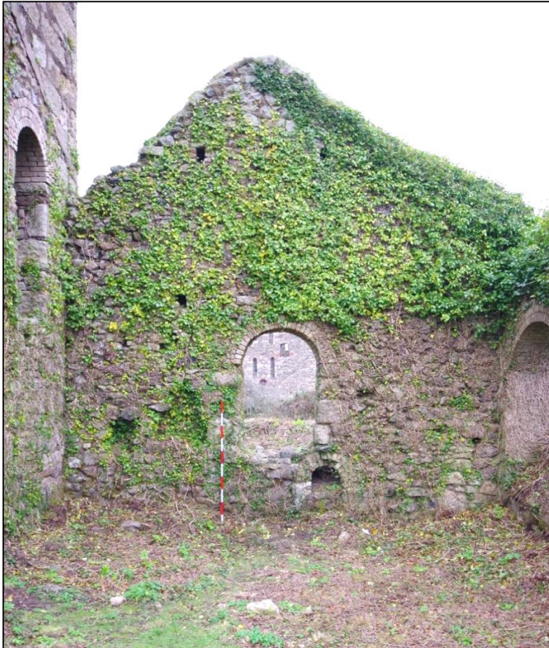
Fig 59 Interior south-west wall of boiler house before remedial works.
