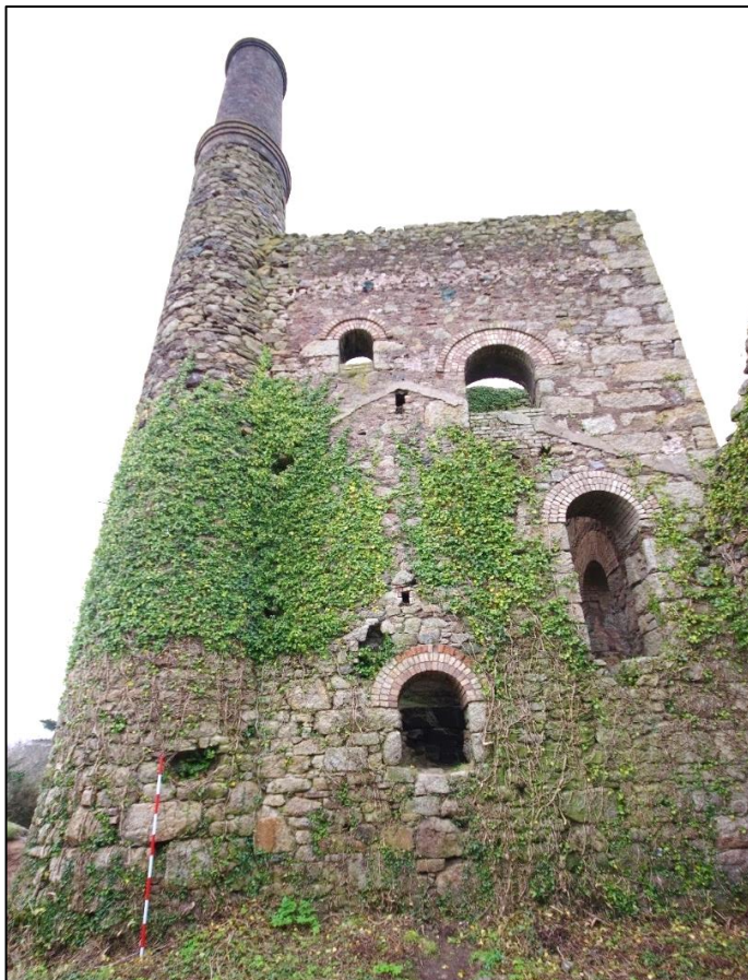
Fig 28 South-east elevation of engine house before remedial works.
