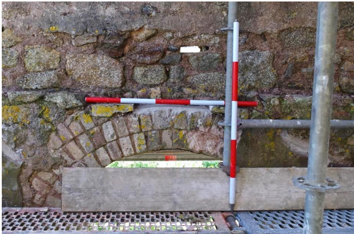
Fig 40 Interior south-east wall following patch repairs.
