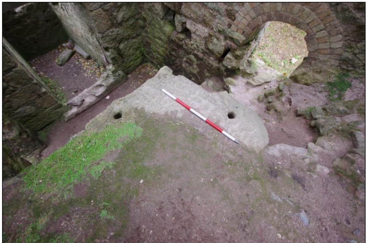
Fig 70 Top of Cylinder bed before repair works showing bolt tunnels.
