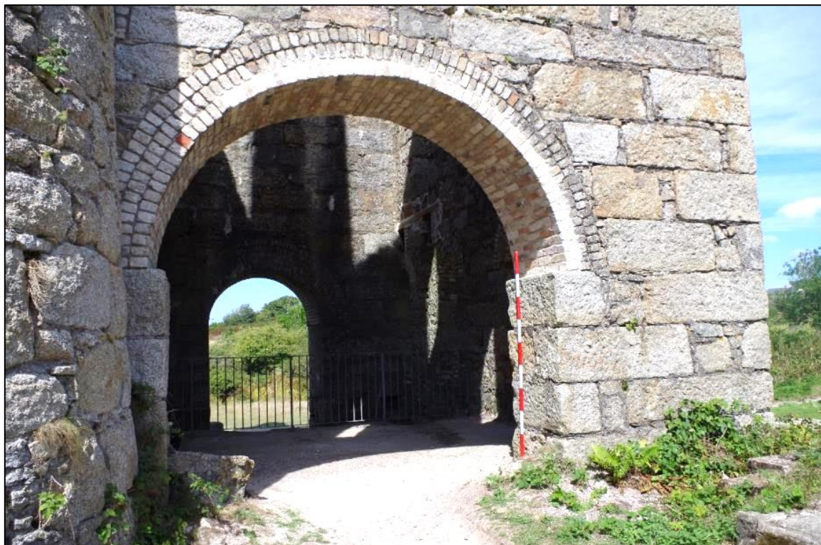
Fig 86 South-east elevation following reconstruction of the lower course of cylinder arch.
