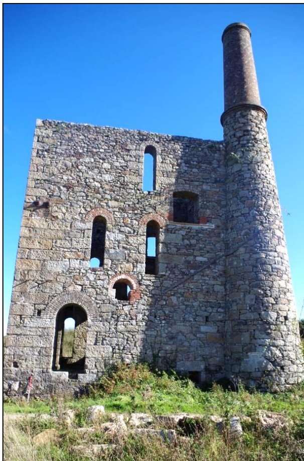
Fig 98 South-west elevation following remedial works.
