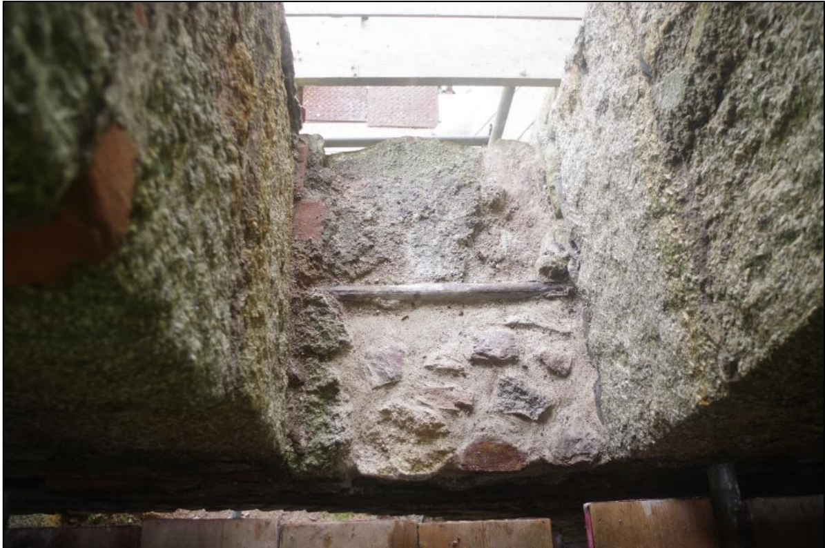
Fig 95 Interior south-east gable wall following small patch repair to window sill.
