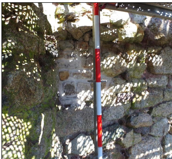
Fig 30 South-east elevation following patch repairs.
