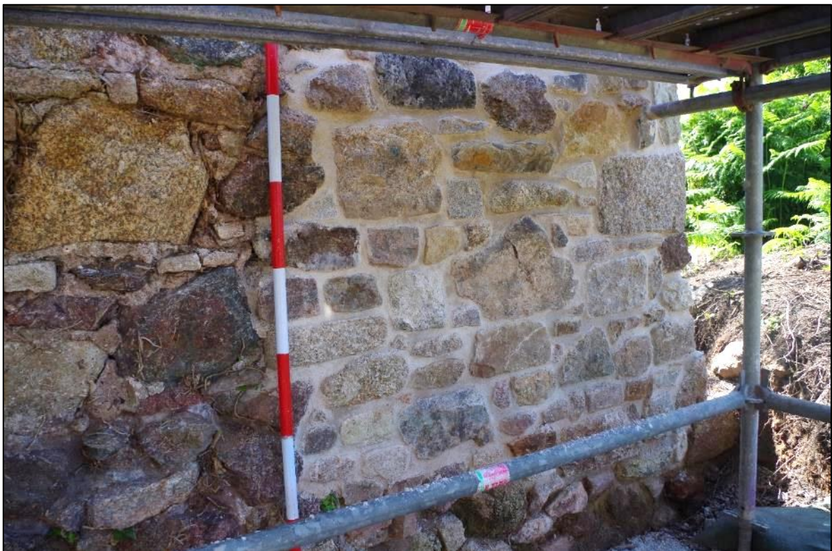
Fig 48 Interior south-east wall of the boiler house following patch repair.
