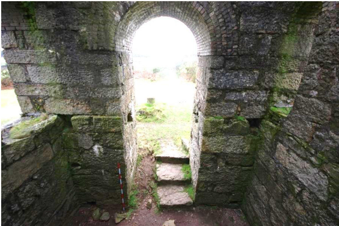
Fig 83 Interior north-west bob wall.
