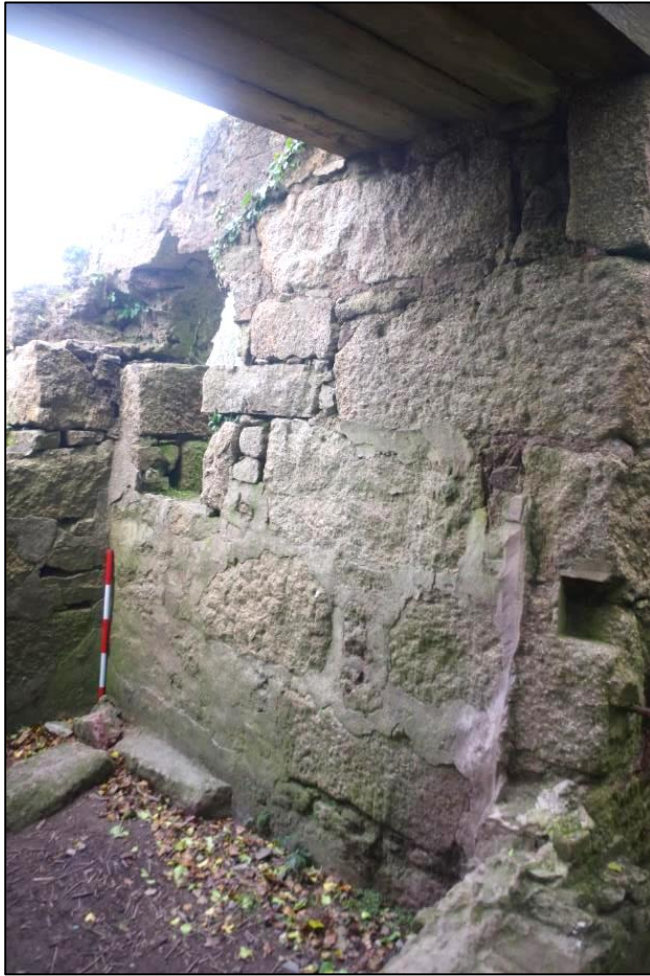
Fig 41 Interior south-east wall of the condenser pit before remedial works.
