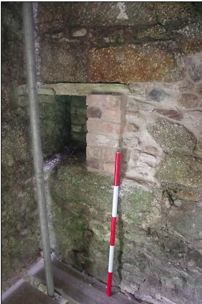
Fig 102 Interior south-west wall, repair to joist socket.
