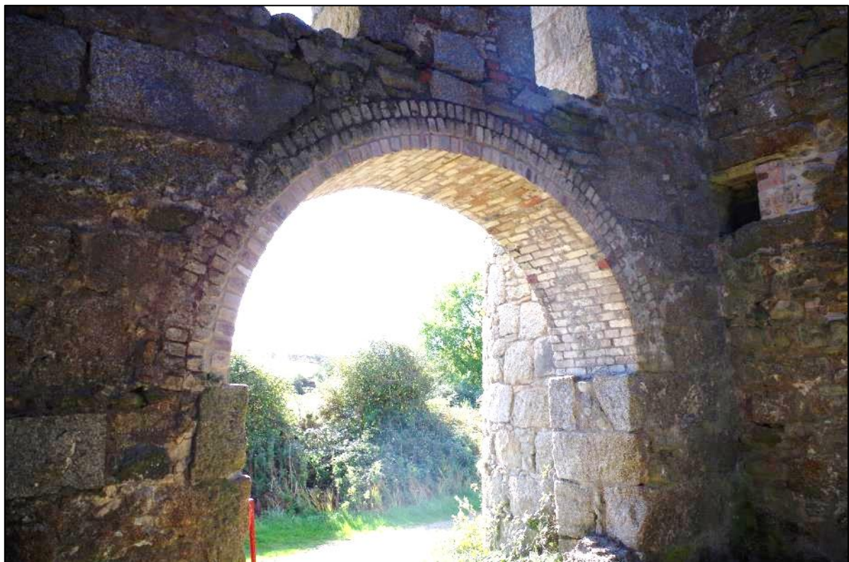
Fig 88 Interior south-east cylinder arch following repairs.
