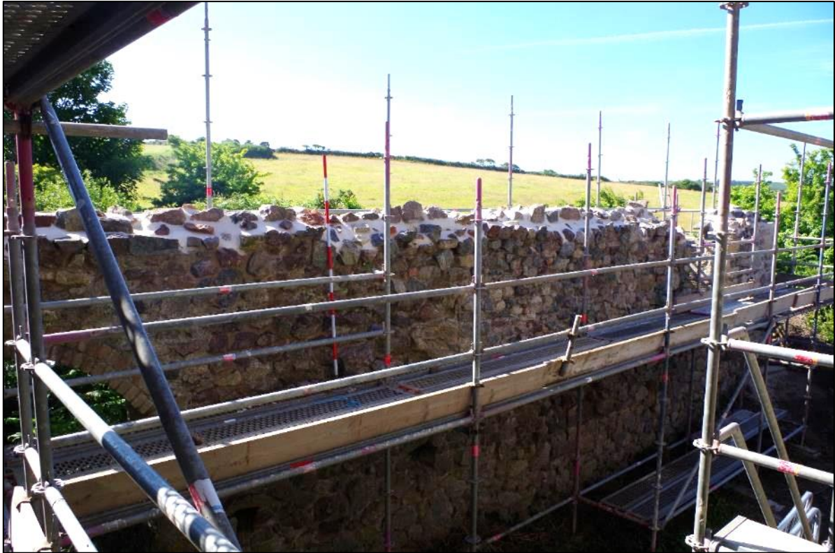
Fig 43 South-east wall of the boiler house following lime mortar capping.
