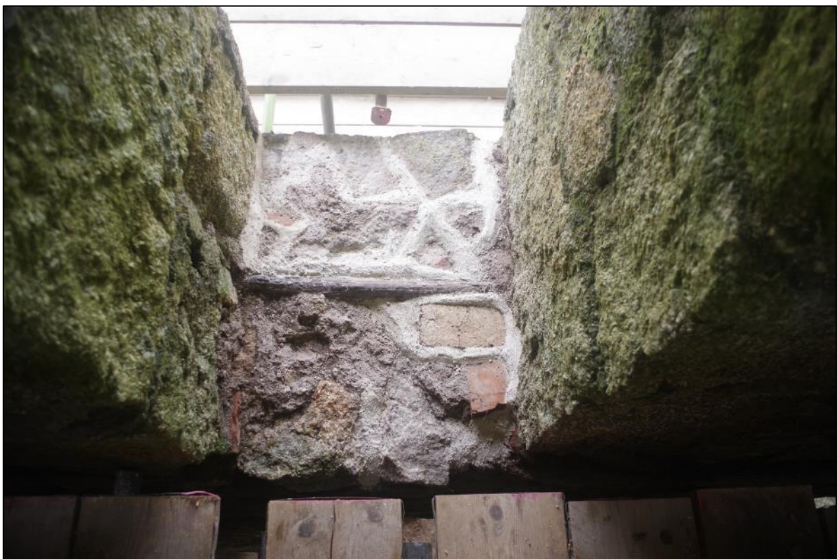
Fig 94 Interior south-east gable wall following small patch repair to window sill.
