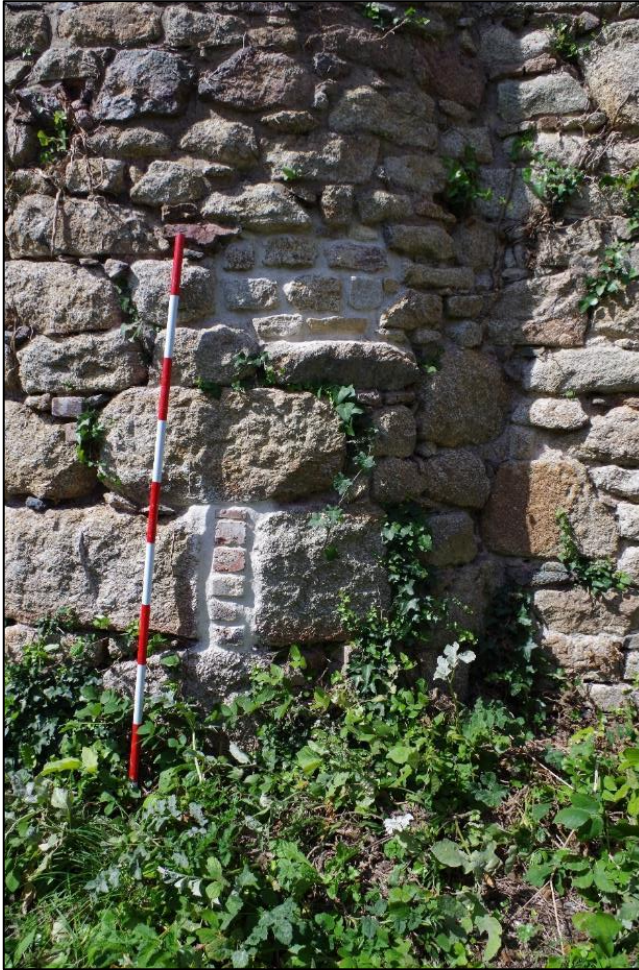
Fig 33 South-east elevation following patch repairs to chimney stack.
