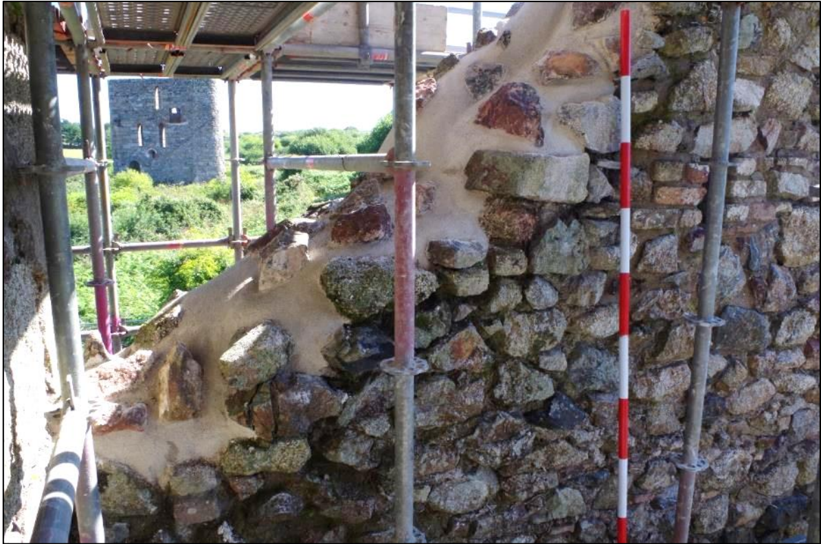
Fig 61 Interior south-west wall of boiler house following repairs to gable end.
