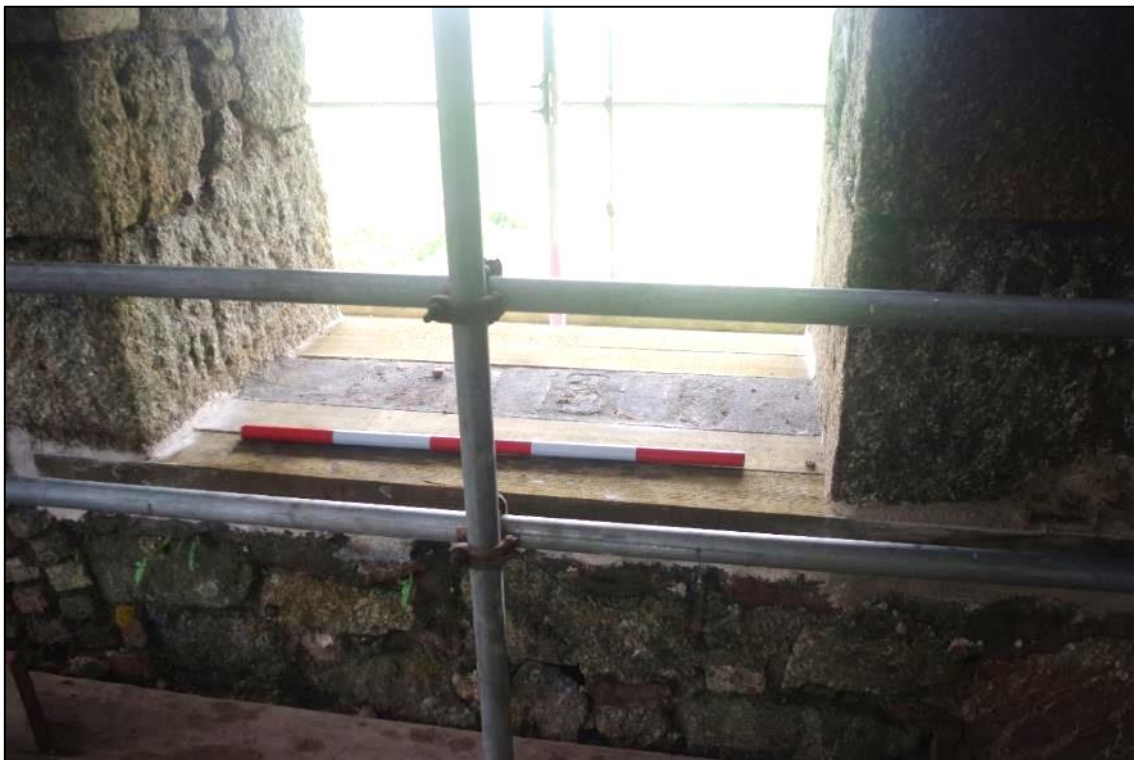
Fig 78 Interior north-east wall, repairs to main girder slot sill.
