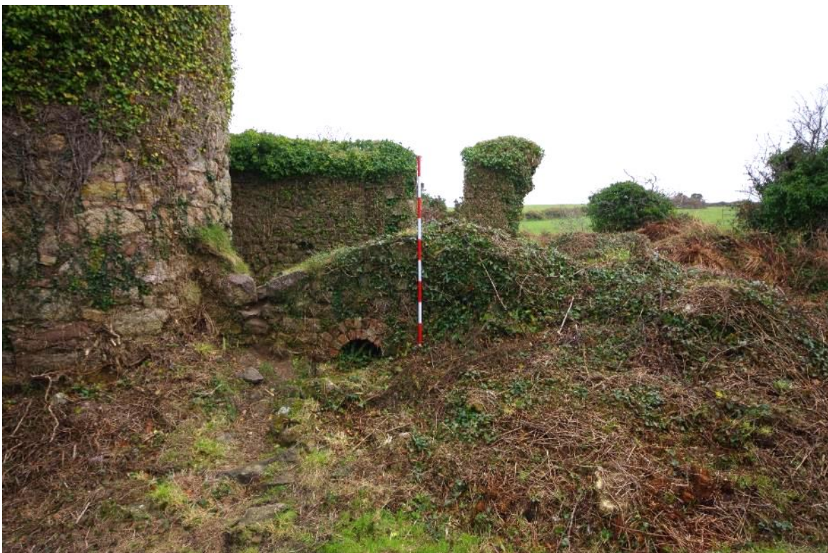
Fig 22 North-west elevation of remains of boiler house wall before remedial works.
