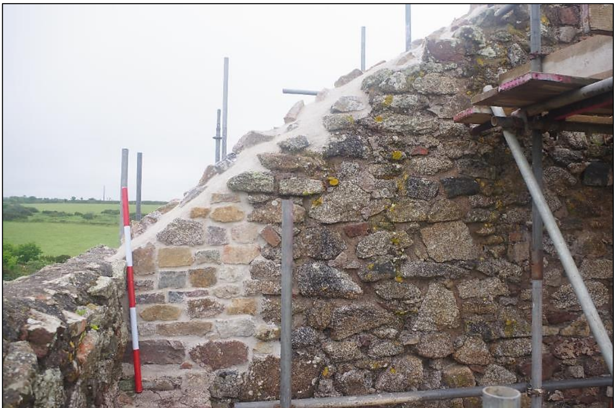
Fig 90 Interior south-east gable wall following patch repair and capping.
