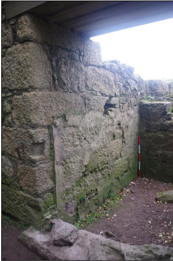
Fig 27 North-west wall of condenser pit.
