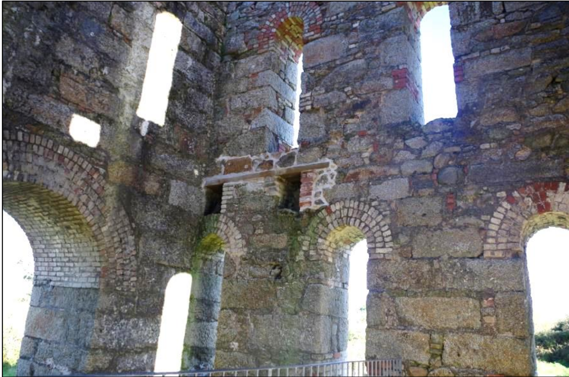
Fig 77 Interior north-east wall following remedial works.
