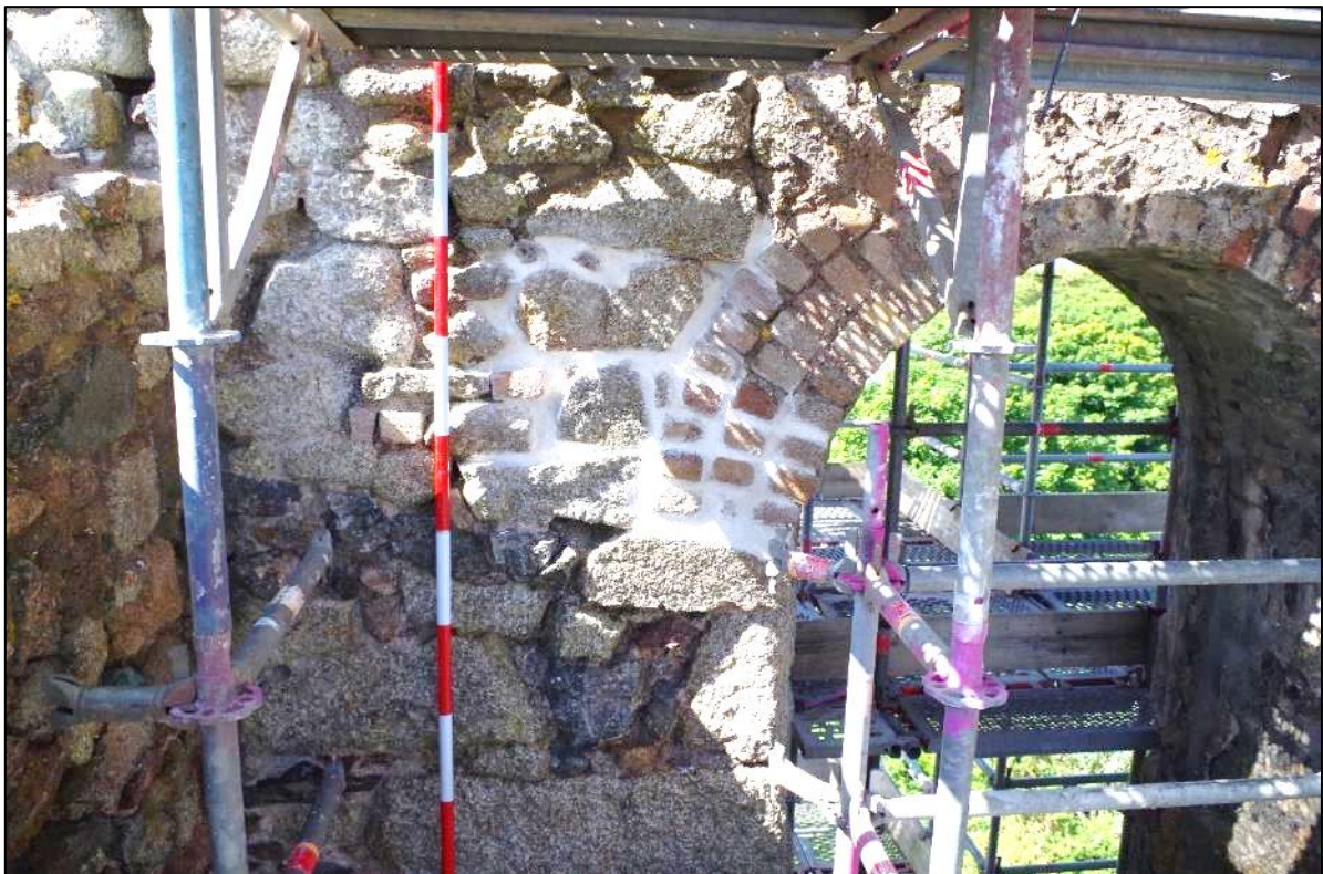
Fig 56 Interior south-west engine house wall following patch repairs.
