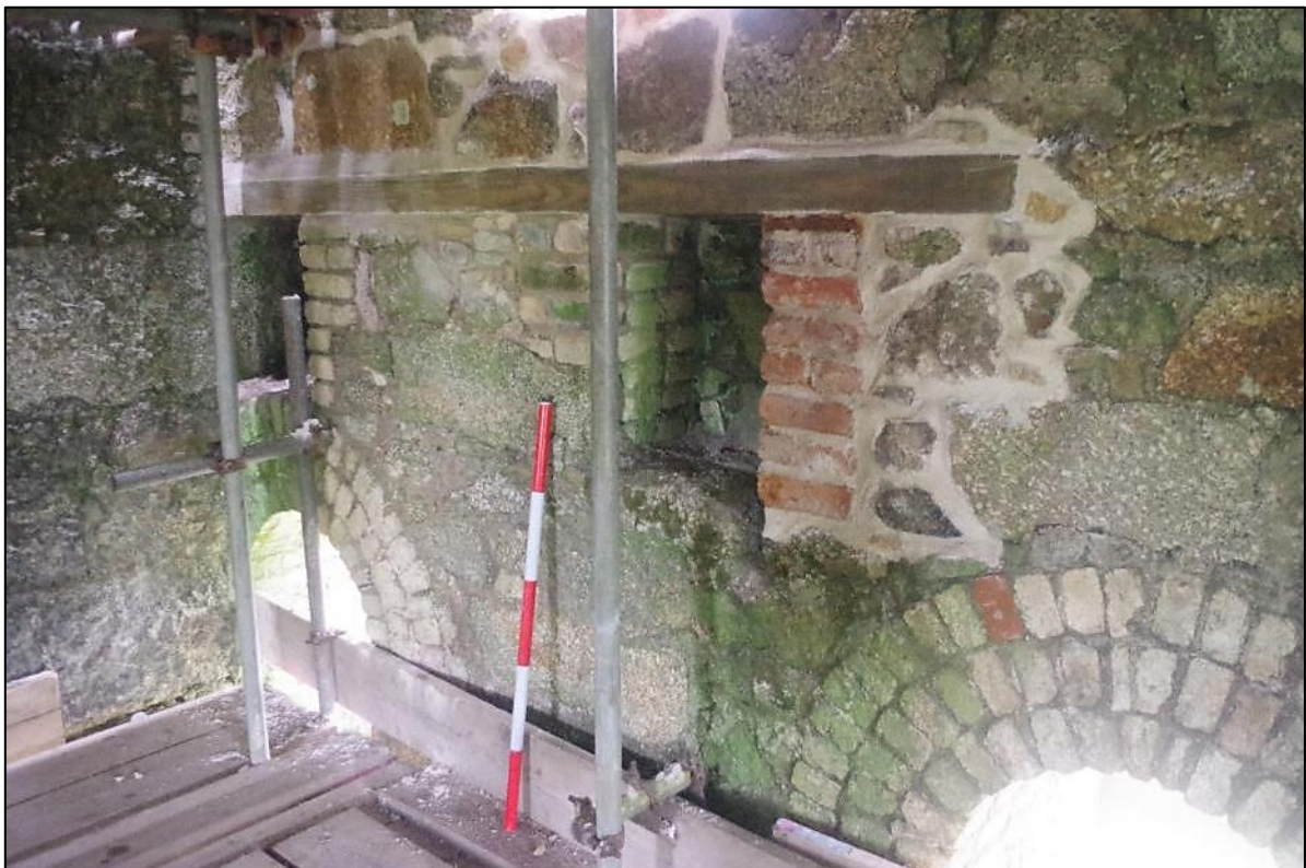
Fig 76 Interior north-east wall, jost sockets and lintel following remedial works.
