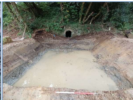
Fig 83 Excavated area below Toad Hall Culvert, looking west.
