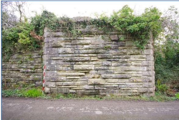
Fig 44 RRB05 Reen Rose Bridge east abutment, looking east.
