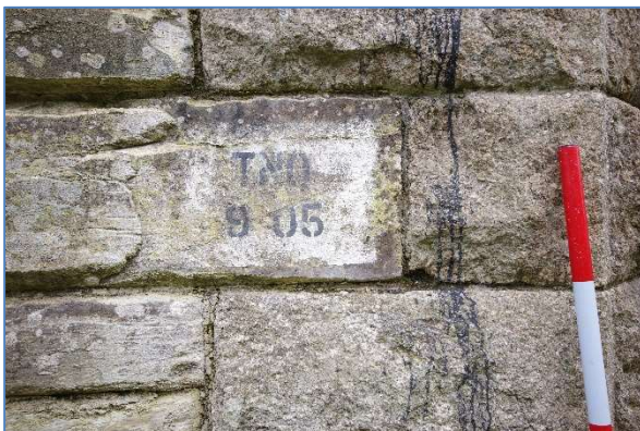
Fig 46 RRB07 Reen Rose Bridge east abutment, railway sign, looking east.
