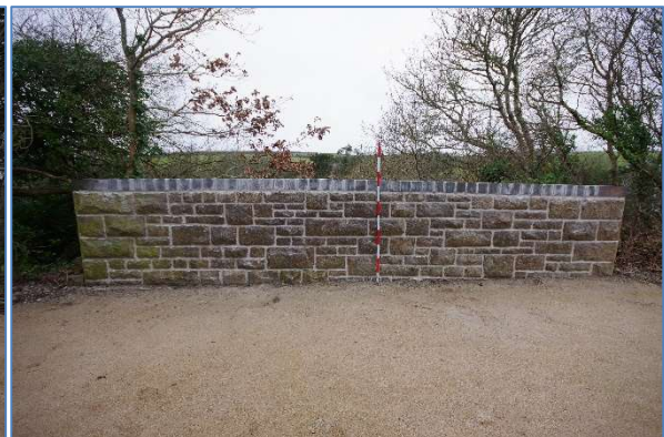
Fig 39 LHB17 Lighthouse Bridge northern parapet wall, repointed, looking north.
