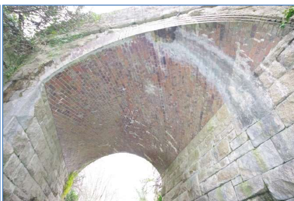
Fig 31 LHB07 Lighthouse Bridge, underside brick bridge span, looking east.
