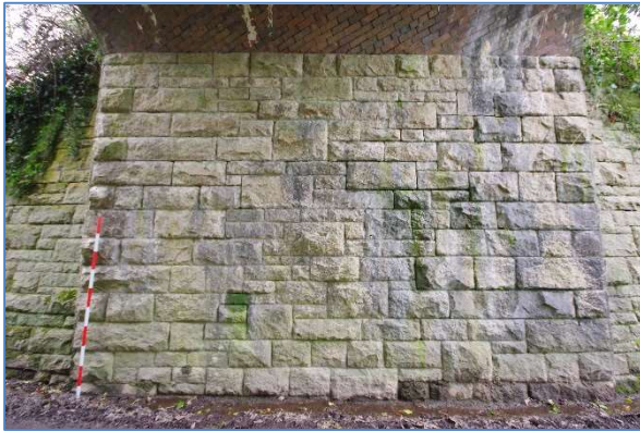
Fig 36 LHB13 Lighthouse Bridge northern abutment, looking north.
