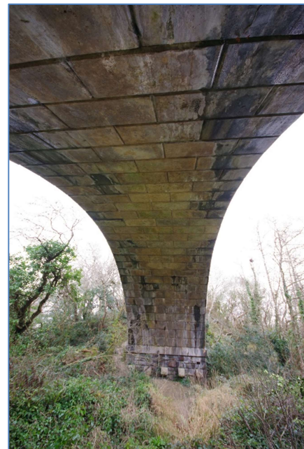
Fig 24 COV54 Cocks Viaduct, eastern arch span, looking east.
