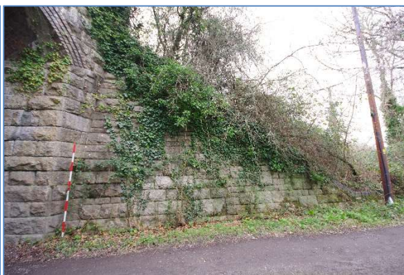
Fig 33 LHB09 Lighthouse Bridge southern abutment, west side retaining wall looking south.
