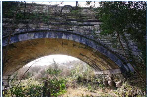
Fig 16 COV38 Western arch of Cocks Viaduct, looking south.
