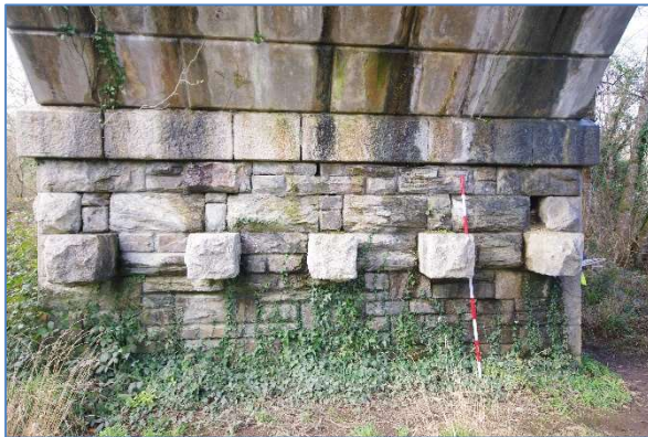
Fig 15 COV36 West central arch, west side, with granite corbels and openings above, looking west.
