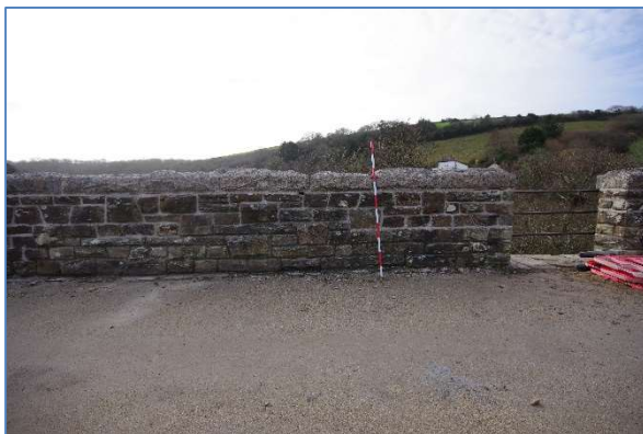
Fig 11 COV11 Cocks Viaduct southern parapet and recess, looking south.
