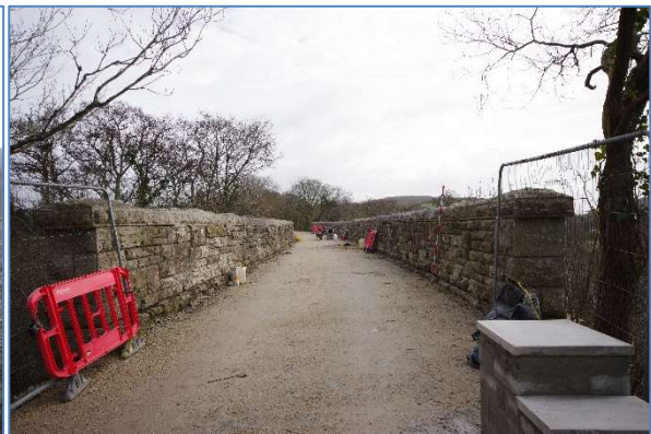
Fig 10 COV09 Long shot along Cocks Viaduct, looking east.
