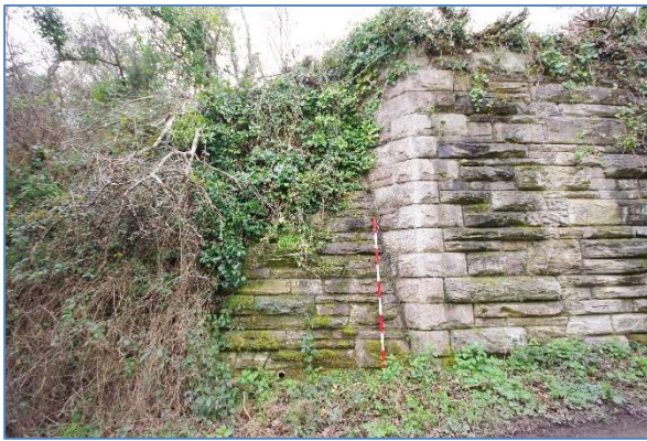
Fig 50 RRB11 Reen Rose Bridge west abutment, south retaining wall, looking west.
