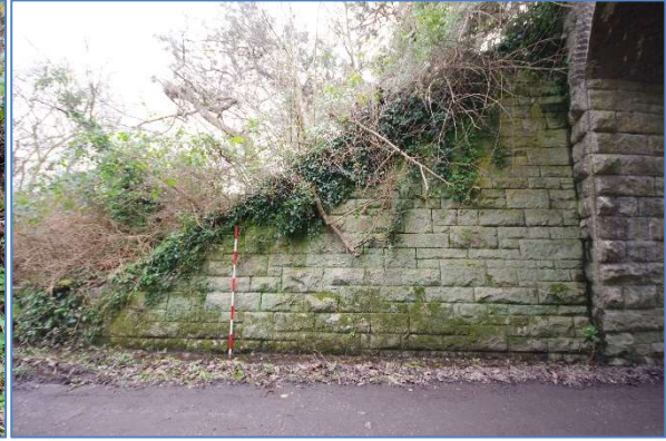
Fig 35 LHB12 Lighthouse Bridge northern abutment, west side retaining wall, looking north.
