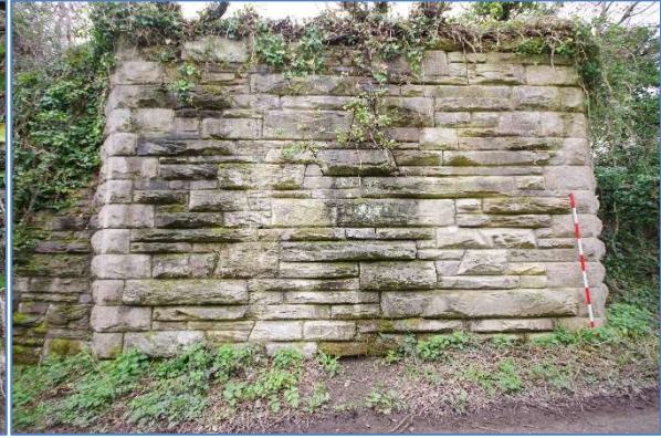
Fig 49 RRB10 Reen Rose Bridge west abutment, looking west.
