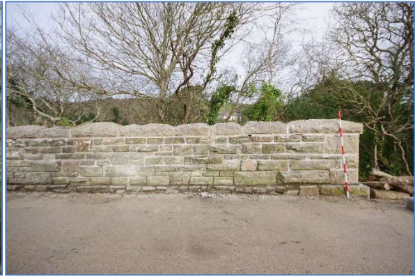
Fig 8 COV03 Cocks Viaduct northern parapet wall, east end, looking north.
