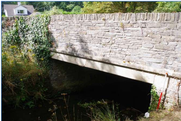
Fig 57 East elevation of the current bridge at Cocks Hill, looking west.
