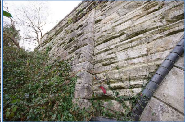
Fig 20 COV45 Cocks Viaduct west end of south elevation, looking northwest.
