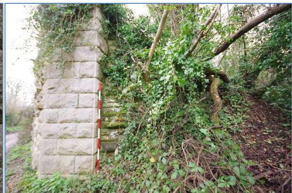
Fig 47 RRB08 Reen Rose Bridge west abutment, north retaining wall, looking south.
