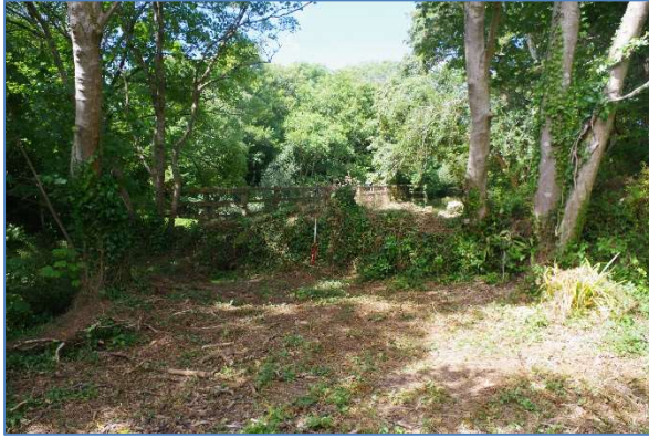
Fig 69 Southeast elevation of the boundary wall overlying the leat (left of shot), looking northwest.
