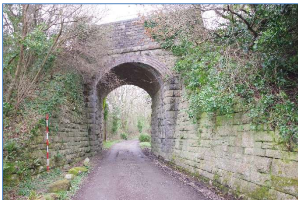
Fig 28 LHB02 Lighthouse Bridge from the east, looking west.
