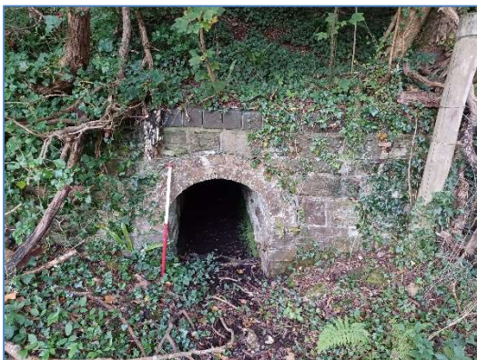
Fig 82 Toad Hall Culvert, looking west.
