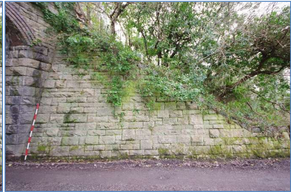
Fig 37 LHB14 Lighthouse Bridge northern abutment, east side retaining wall, looking north.
