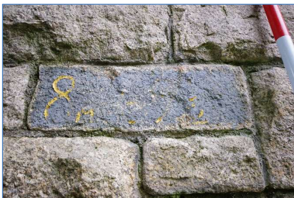
Fig 32 LHB08 Lighthouse Bridge southern abutment railway sign, looking south.
