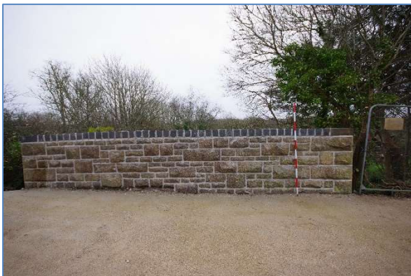
Fig 38 LHB16 Lighthouse Bridge southern parapet wall, repointed, looking south.
