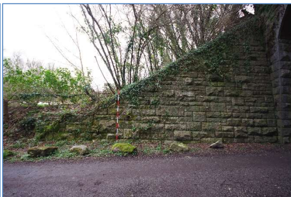
Fig 29 LHB04 Lighthouse Bridge southern abutment, east side retaining wall, looking south.
