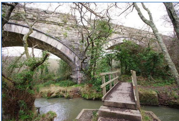
Fig 23 COV53 Cocks Viaduct, south elevation, eastern arch, looking northeast.
