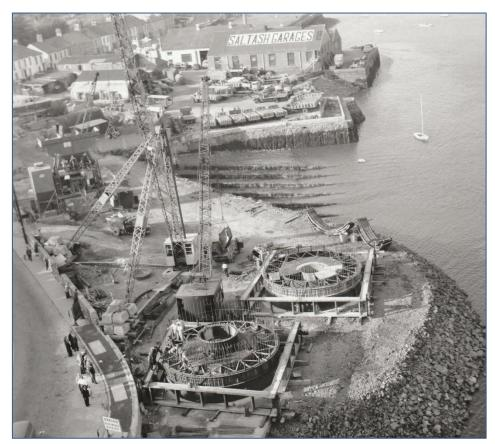
Fig 7 Construction of bridge piers for the Tamar Bridge c1959. Aggregate was laid across the foreshore and quay to provide stable access for machinery.
