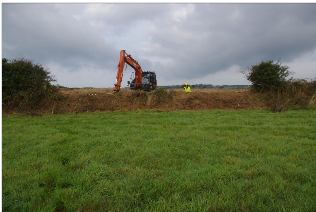
Figure 21 HE-03-03. Pre-excavation photograph of east-facing elevation of hedge-break. 1m scale.
