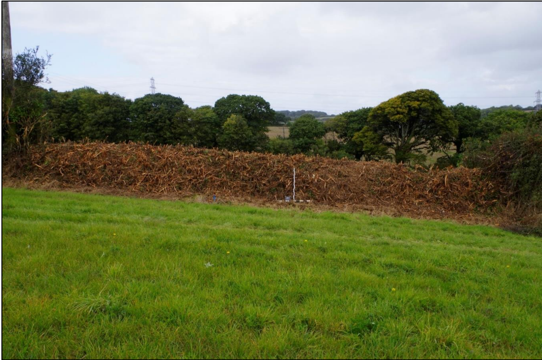
Figure 66 HE-08-08. Pre-excitation photograph of south-facing elevation in area of hedge-break. 1m scale.
