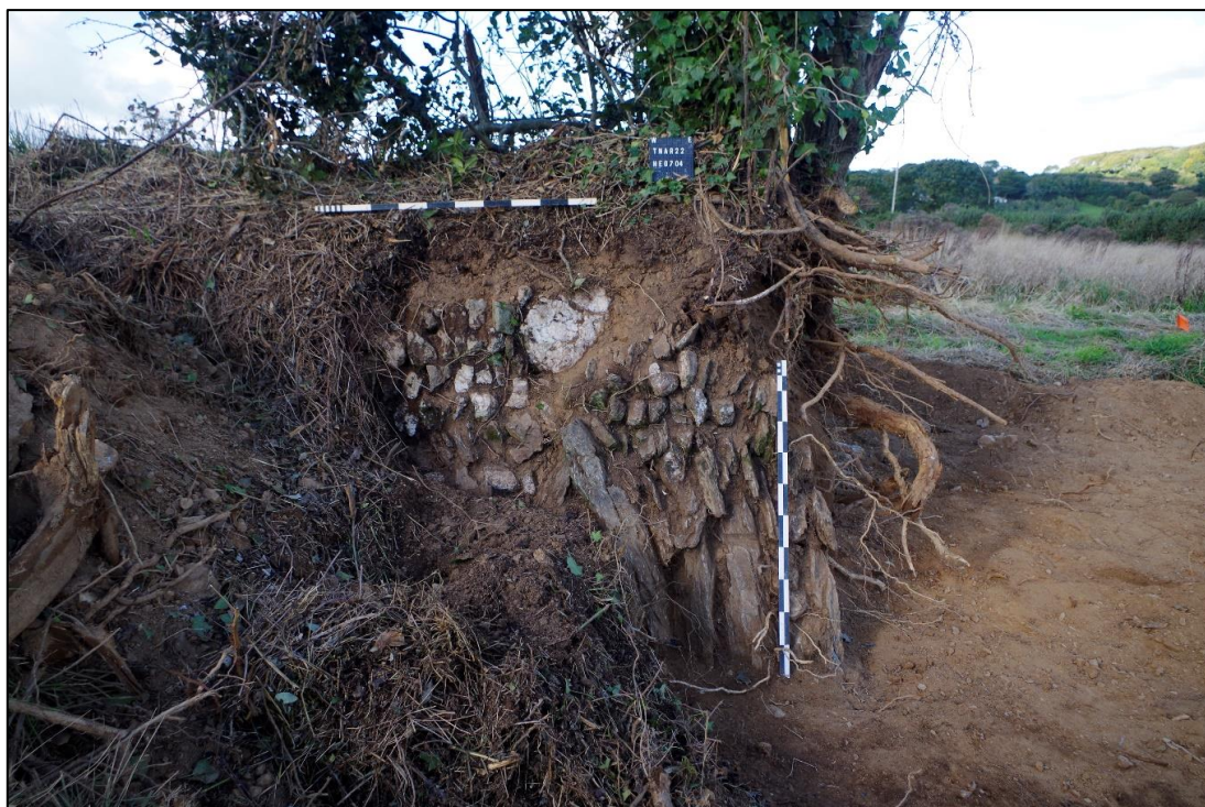
Figure 55 HE-07-04. Post-excavation photograph of south-facing elevation immediately west of hedge-break, showing two possible phases of construction. 1m scale.
