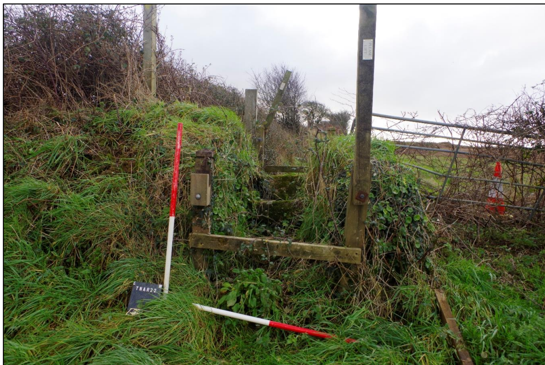
Figure 77 Historic stone stile between fields 2 and 3. Pre-excavation photograph looking south across stile. 1m scale.
