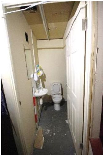
Fig 109 G25 looking north west.
