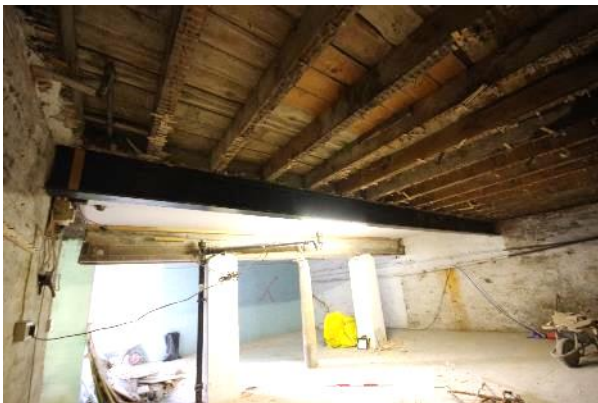
Fig 108 G24 looking west showing walls and ceiling.
