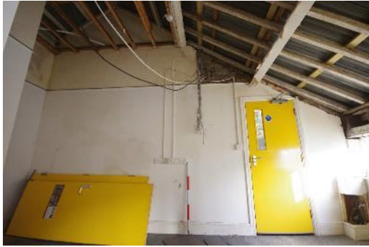
Fig 158 F9 north east wall.
