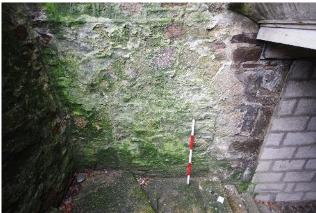
Fig 118 Blocked arched door opening in north east wall of market house taken from steps next to Wheal Peevor purser's office.
