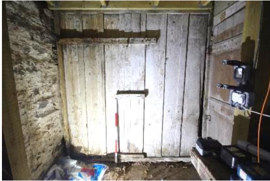
Fig 100 G21 north east wall.
