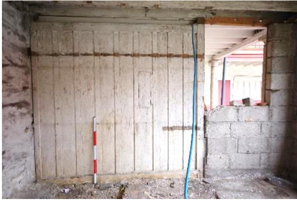
Fig 80 G12 south west wall during watching brief showing original plank and muntin wall.
