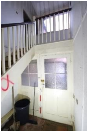
Fig 92 G18 north east wall.
