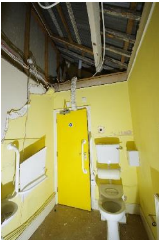
Fig 163 F13 looking south west.
