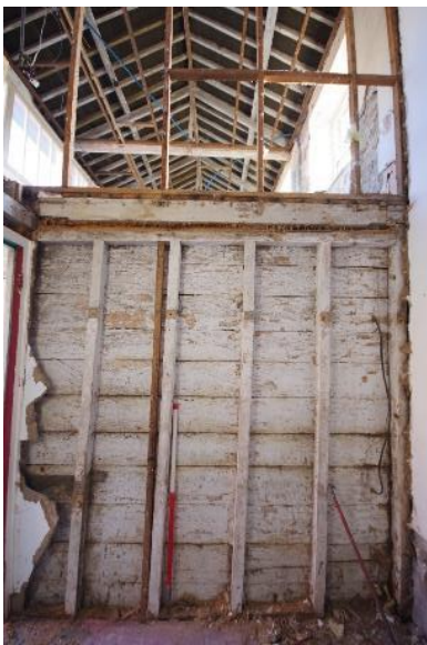
Fig 95 G18 during watching brief, south east wall with removed boarding.
