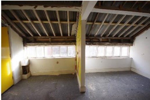
Fig 159 F9 and F10 south east wall.
