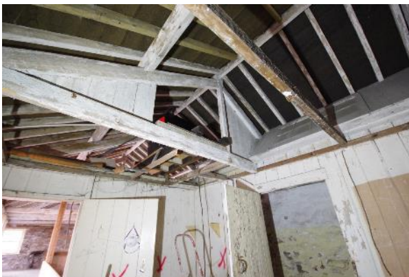
Fig 142 F5 roof structure after removal of the ceiling, looking south east.
