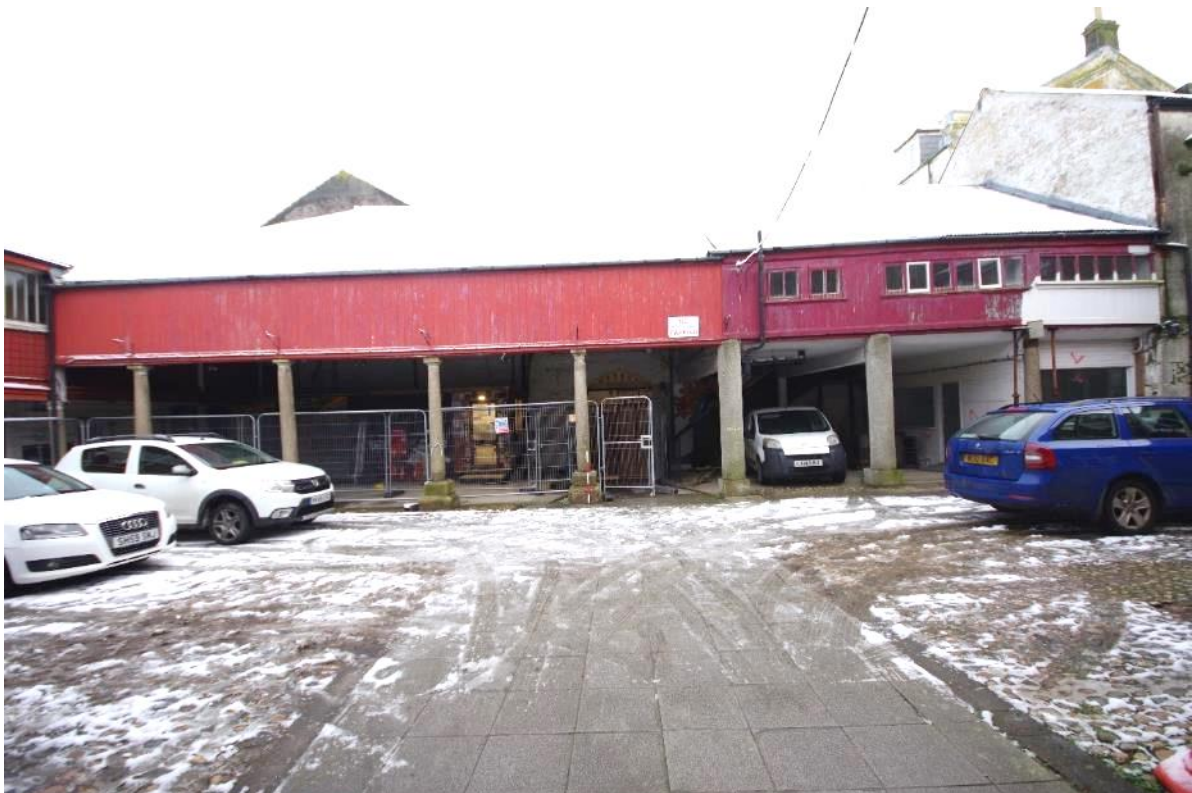
Fig 52 Exterior south east elevation of the covered market area.
