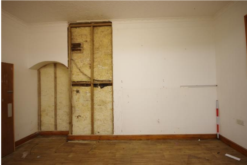
Fig 61 G1 north east wall.
