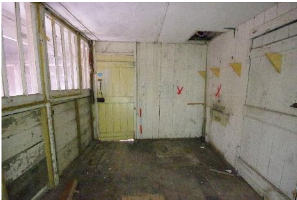
Fig 141 F5 south east wall.
