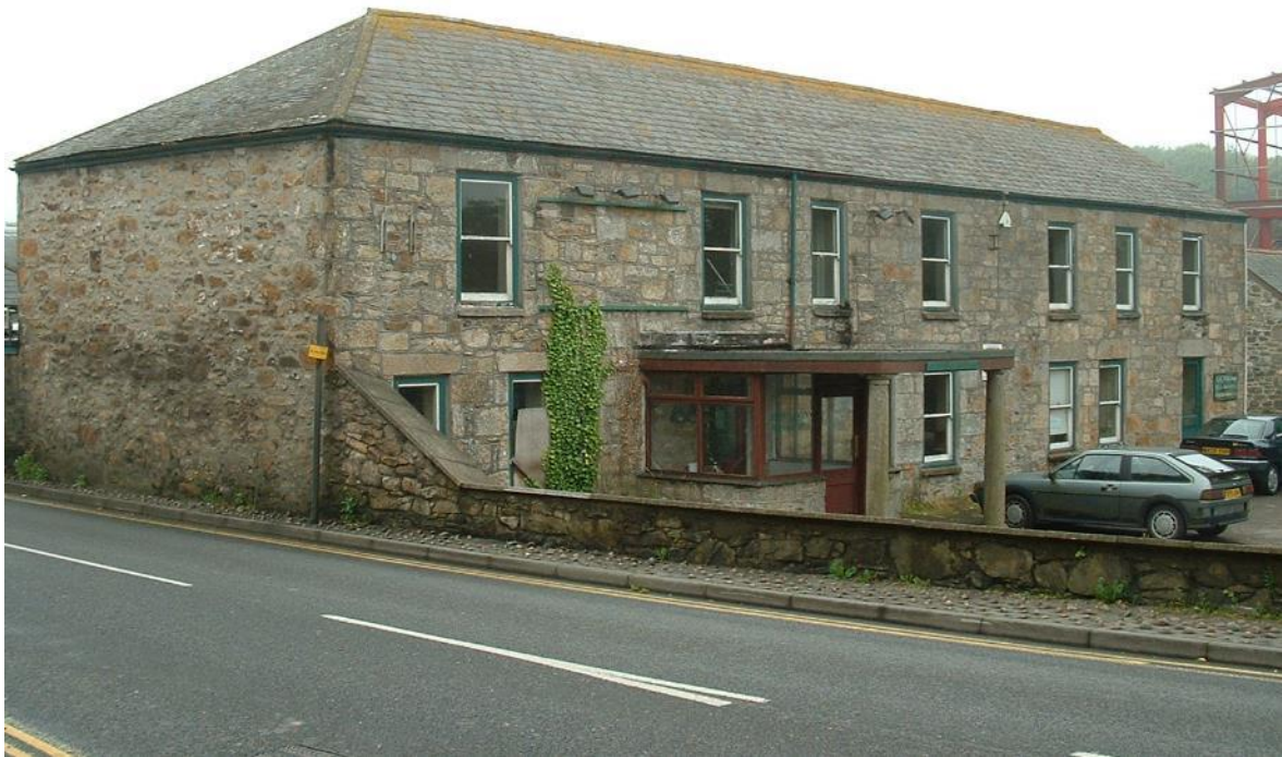
Fig 28 Chymbbla House to the north of Kresen Kernow (former 19th century safety fuse works owned by Alfred Lanyon) taken in 2005, showing two granite Tuscan columns taken from the market in the c1930s and reused in the portico.
