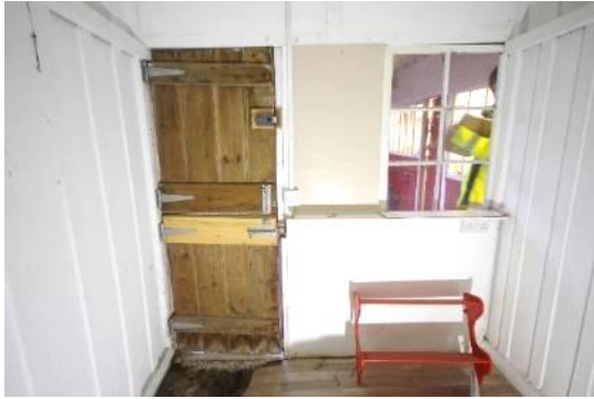
Fig 86 G15 north east wall.
