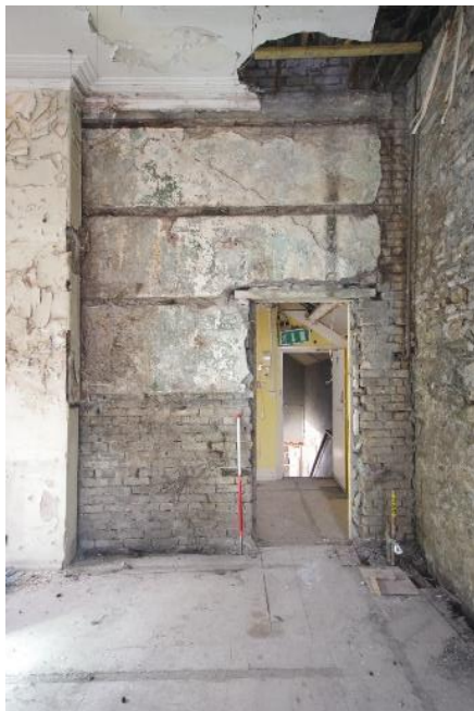
Fig 156 F8 south west wall with all finishes removed.
