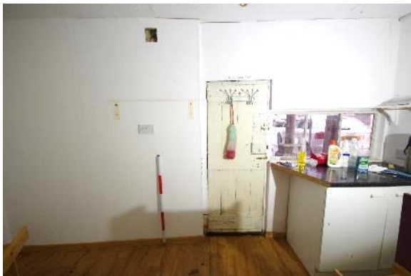
Fig 97 G19 north east wall.
