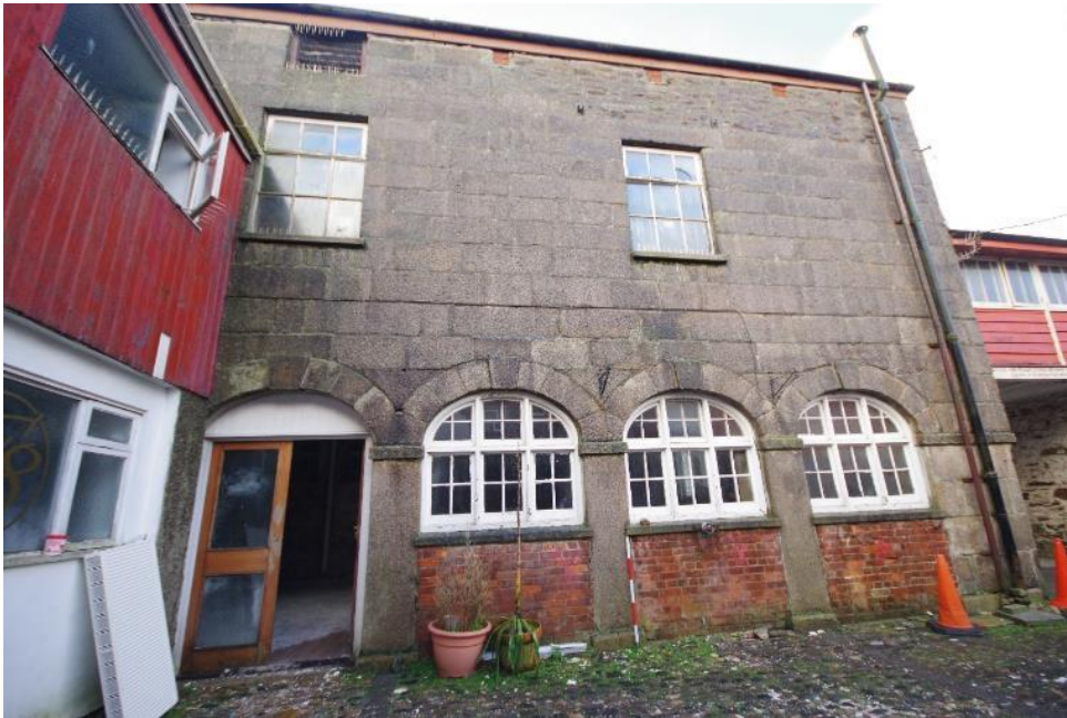
Fig 45 North west elevation of the market house.
