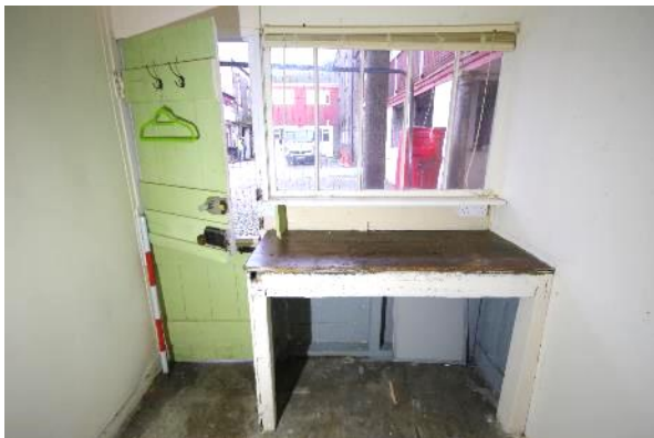
Fig 88 G16 north east wall.
