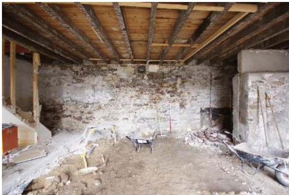
Fig 111 G26 North east wall following demolition of rooms.
