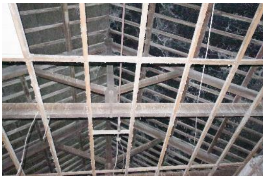
Fig 130 F1 market house roof structure.
