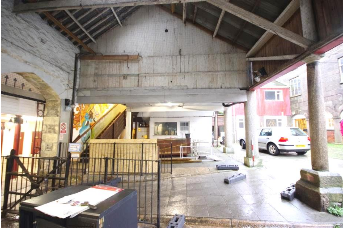
Fig 55 South west elevation of the Mining Exchange extension and area below.
