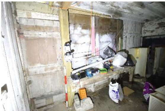
Fig 101 G21 south east wall.
