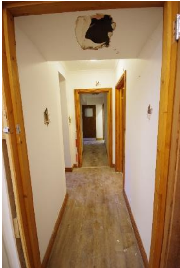
Fig 72 G7 looking north west.
