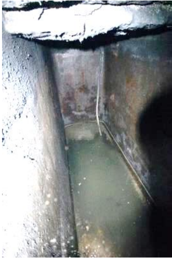
Fig 124 G30 Interior looking north west.
