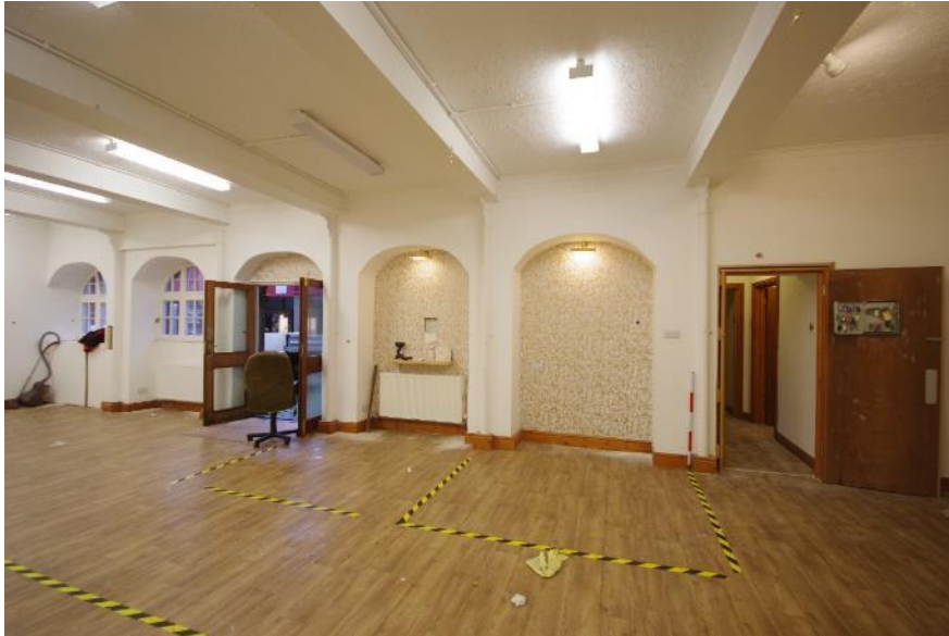
Fig 59 G1 north west (front) wall.
