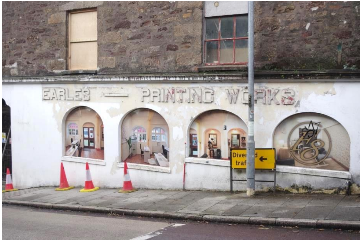
Fig 39 South east elevation of the market house showing Earles printing works sign.
