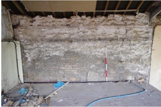
Fig 133 F2 south east wall.
