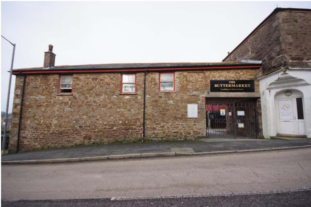
Fig 40 South east elevation of the south east range.
