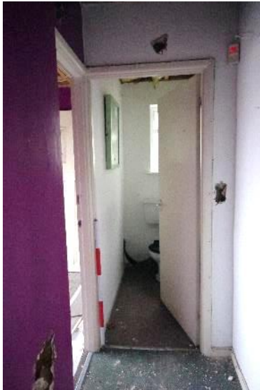
Fig 184 F20 looking through to F23.
