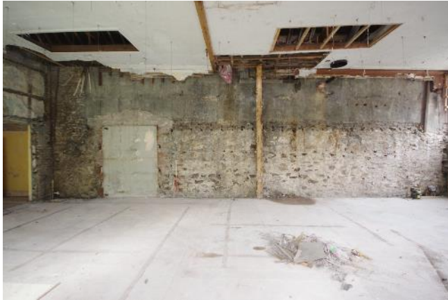
Fig 154 F8 north west wall with all finishes removed.
