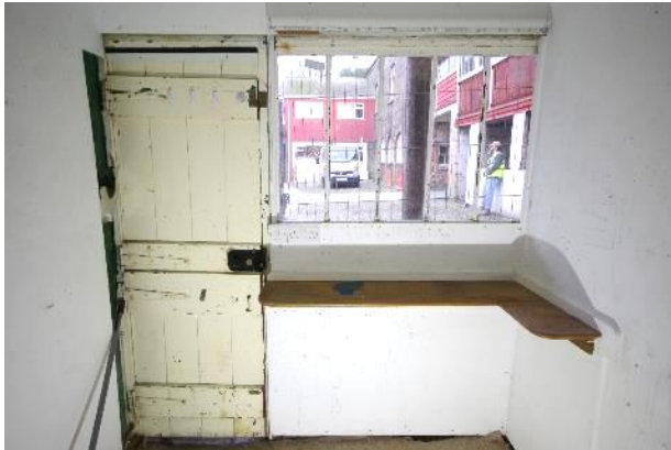
Fig 89 G17 north east wall.
