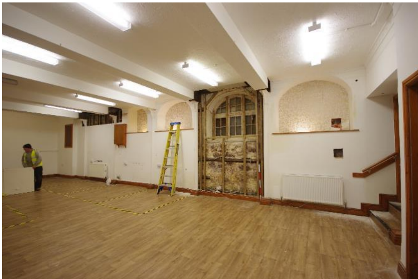
Fig 62 G1 south east wall.
