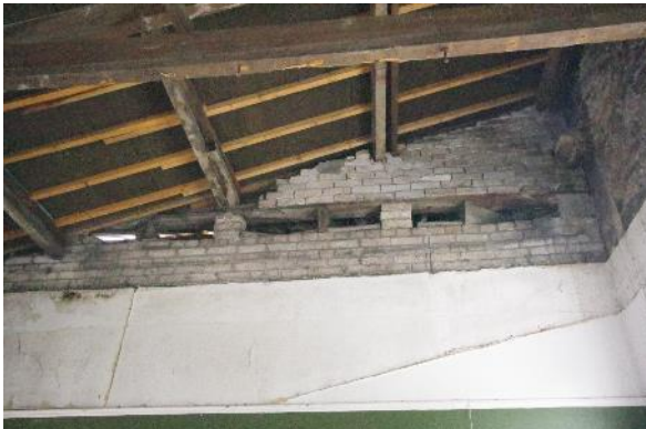
Fig 179 F17 Top of north west wall during watching brief showing cornice of mining exchange frontage upper right and void through to mining exchange roof space.
