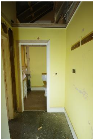
Fig 162 F12 looking south west
