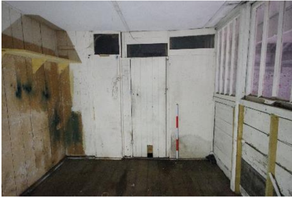
Fig 140 F5 north west wall.
