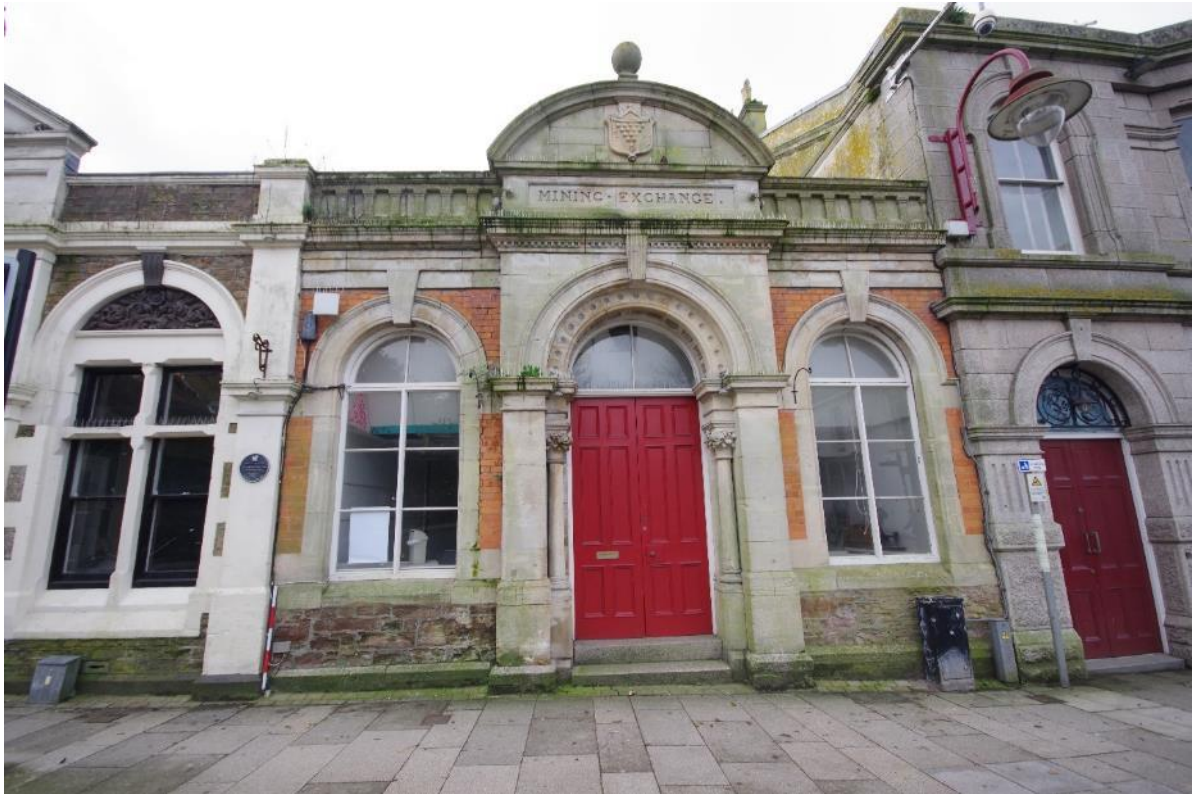
Fig 35 Frontage of the Mining Exchange on Alma Place.
