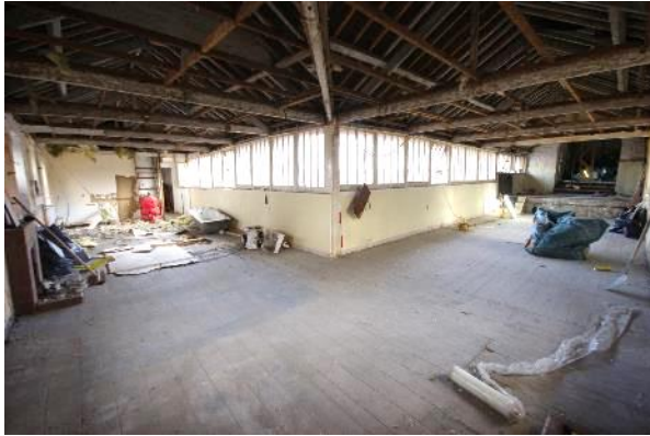
Fig 134 F3 north west and north east walls.
