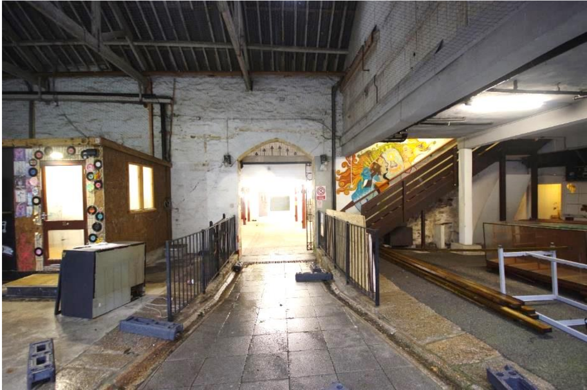
Fig 51 South east elevation under covered market area.
