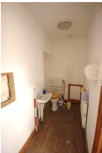
Fig 71 G6 looking north west.
