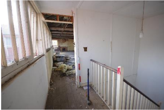
Fig 139 F4 south east wall.
