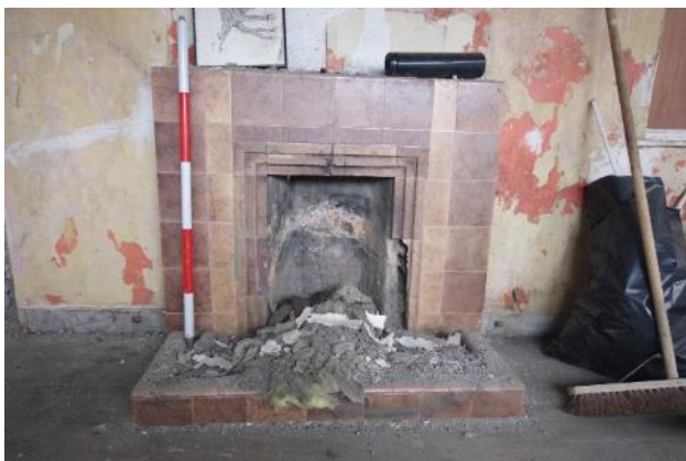
Fig 137 F3 1930s or 40s fire surround in south west wall.
