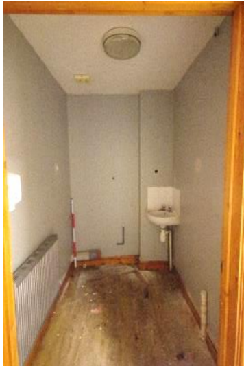
Fig 70 G5 looking north west.
