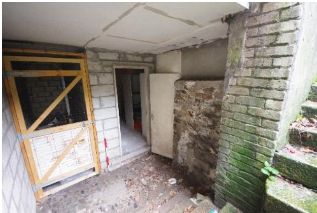
Fig 115 G27 G28 looking north.
