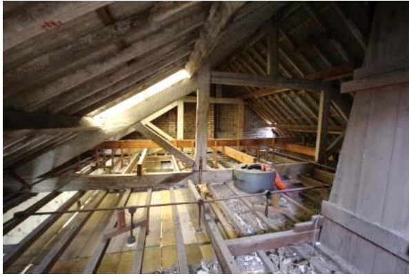
Fig 157 F5 Mining exchange roof looking south west.
