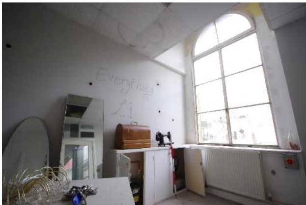
Fig 148 F8 north west and north east walls.
