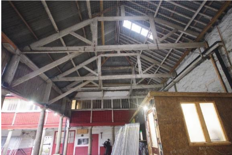
Fig 125 G31 Roof structure looking south west.
