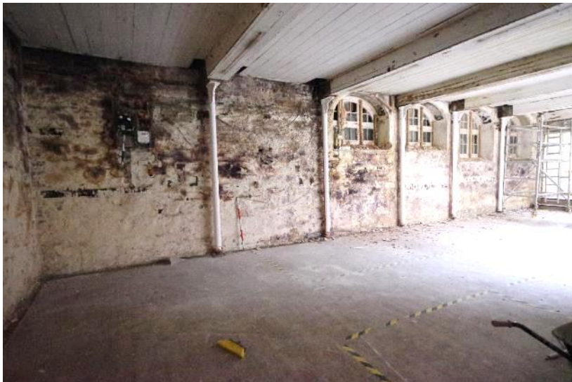
Fig 65 G1 south east wall during watching brief with modern fitting removed.
