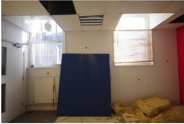
Fig 150 F8 south east wall at south west end.
