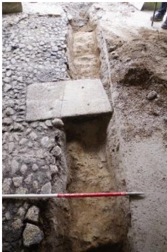
Fig 122 Stone sett surface and trench across the top of the granite lintels of the water tank, looking south east.
