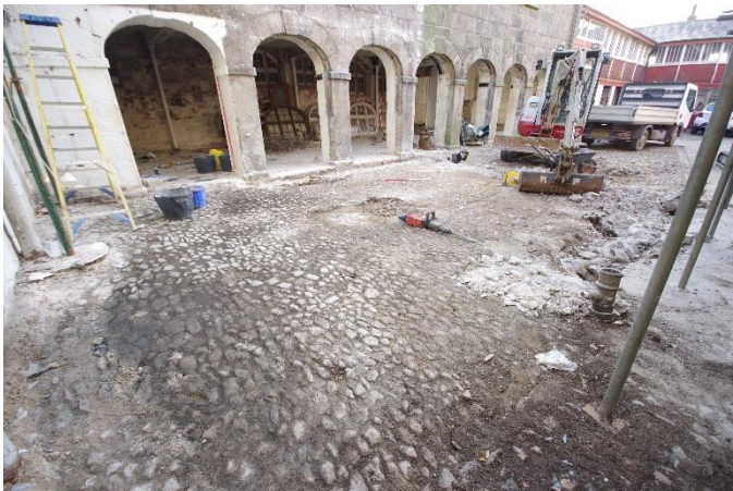
Fig 193 19th century stone sett surface below 1960s and 70s extensions to Wheal Peevor purser's office.
