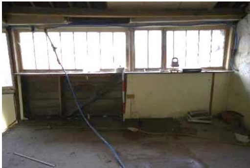
Fig 131 F2 north west wall.
