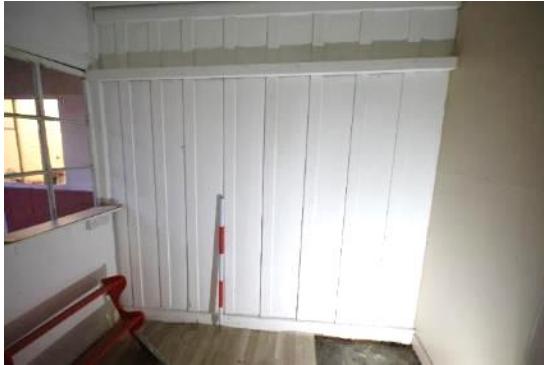
Fig 87 G15 south east wall.
