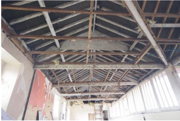
Fig 138 F3 roof structure looking north west.
