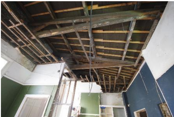
Fig 178 F17 Roof following removal of ceiling showing trusses.
