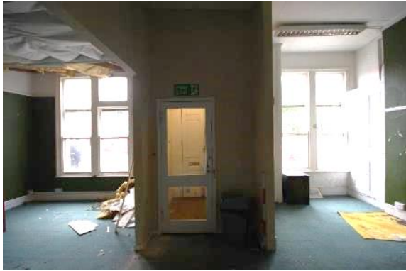
Fig 171 F17 north east wall and lobby.
