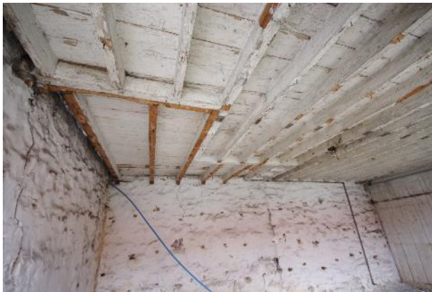
Fig 82 G12 ceiling during watching brief showing position of former staircase.
