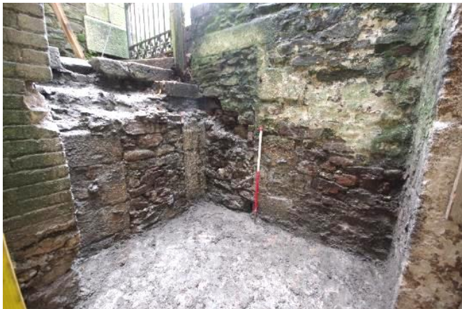
Fig 120 G29 (left) with blocked door opening. Concealed room (right) with blocked door opening. Looking east, when granite steps were removed during watching brief.
