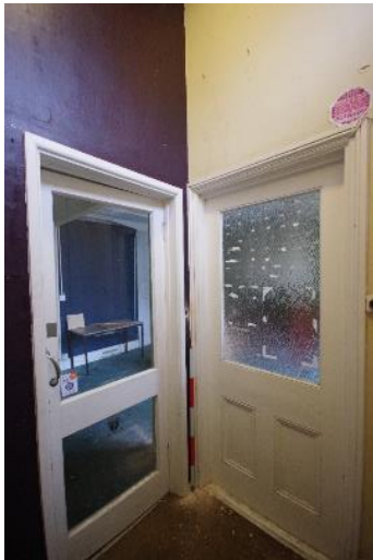
Fig 169 F16 south west and north west walls.
