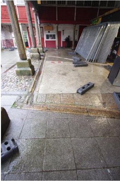
Fig 188 F17 Surface of covered market looking south west.
