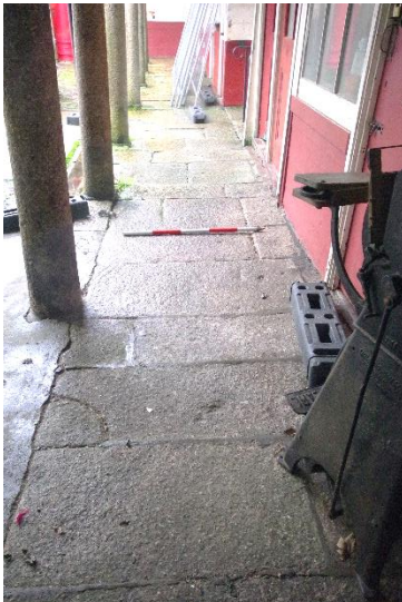
Fig 192 Mid 19th century (phase 2) granite flagstone surface below the colonnade of the south west range.
