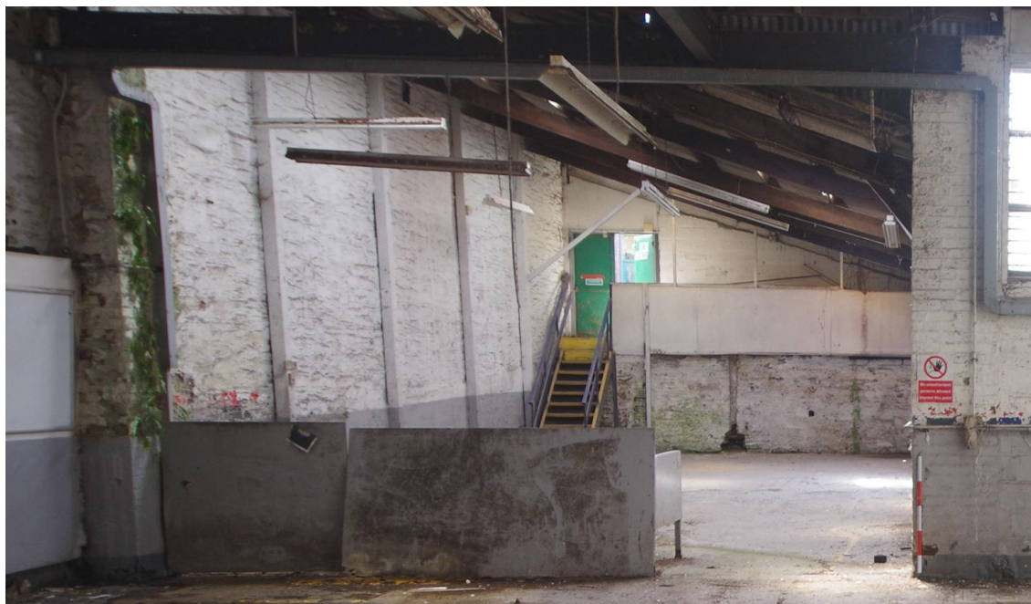
Fig 25 Interior south walls of the southern extension of Room 1 (Garage).
