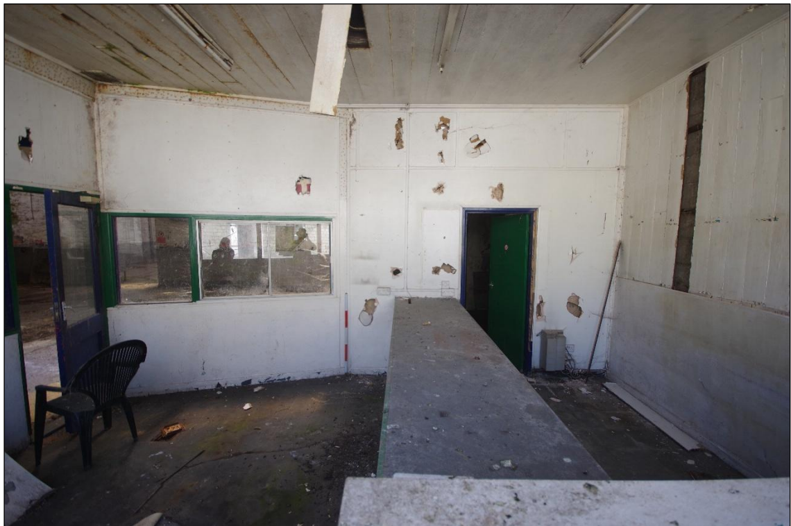
Fig 38 Interior south wall of Room 2 (customer service desk).
