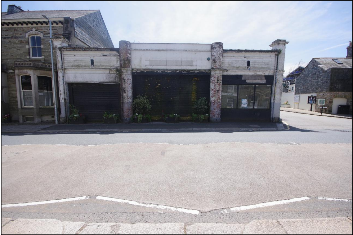
Fig 16 External north elevation of the garage.
