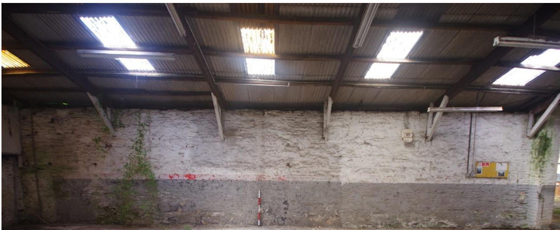
Fig 31 Roof structure in the south extension of room 1 (garage) looking west.
