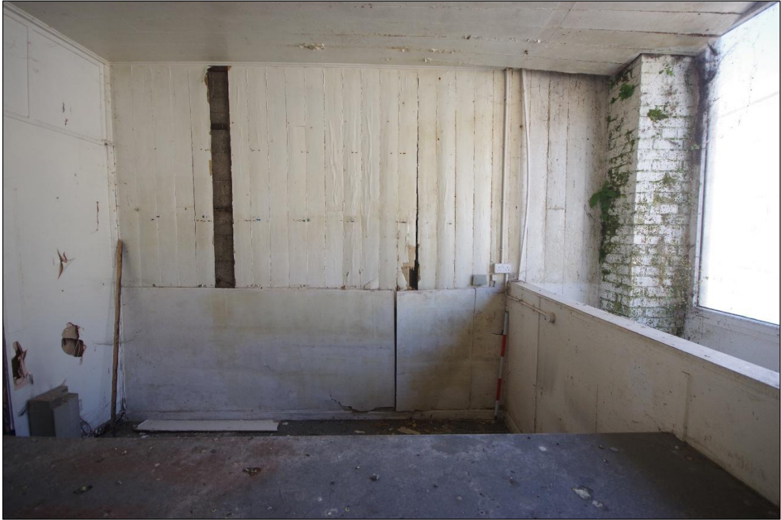
Fig 39 Interior west wall of Room 2 (customer service desk).
