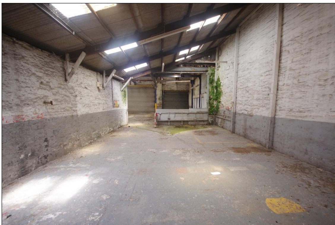
Fig 21 Interior of southern extension of Room 1 (Garage) looking north.
