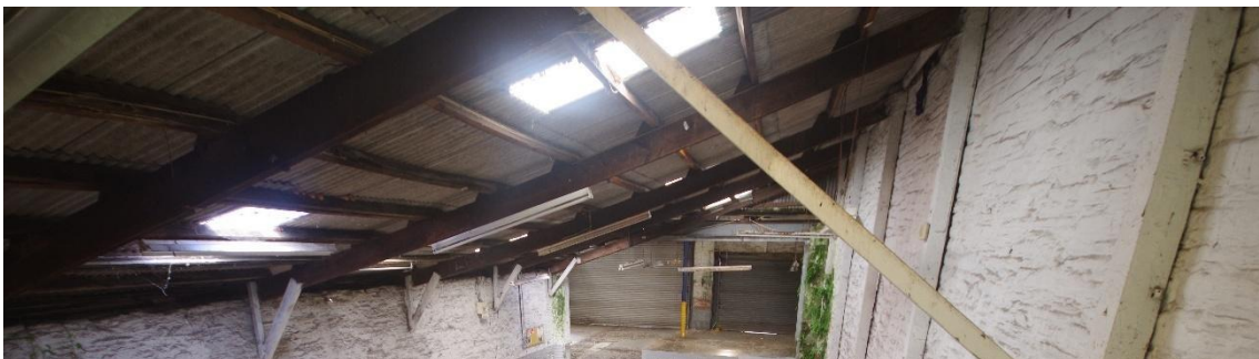
Fig 32 Roof structure in the south extension of room 1 (garage) looking north.
