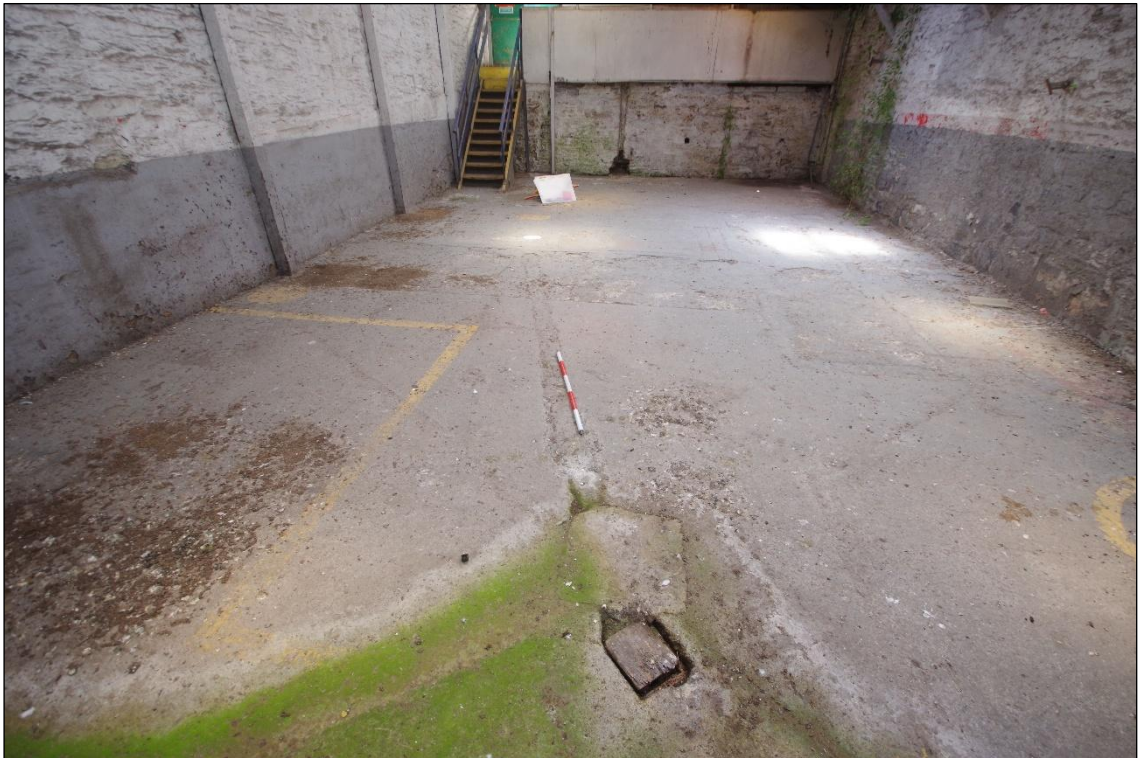
Fig 34 Floor surface in the south extension of room 1 (garage).
