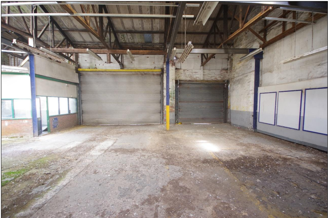
Fig 19 Interior north wall of the Room 1 (Garage).
