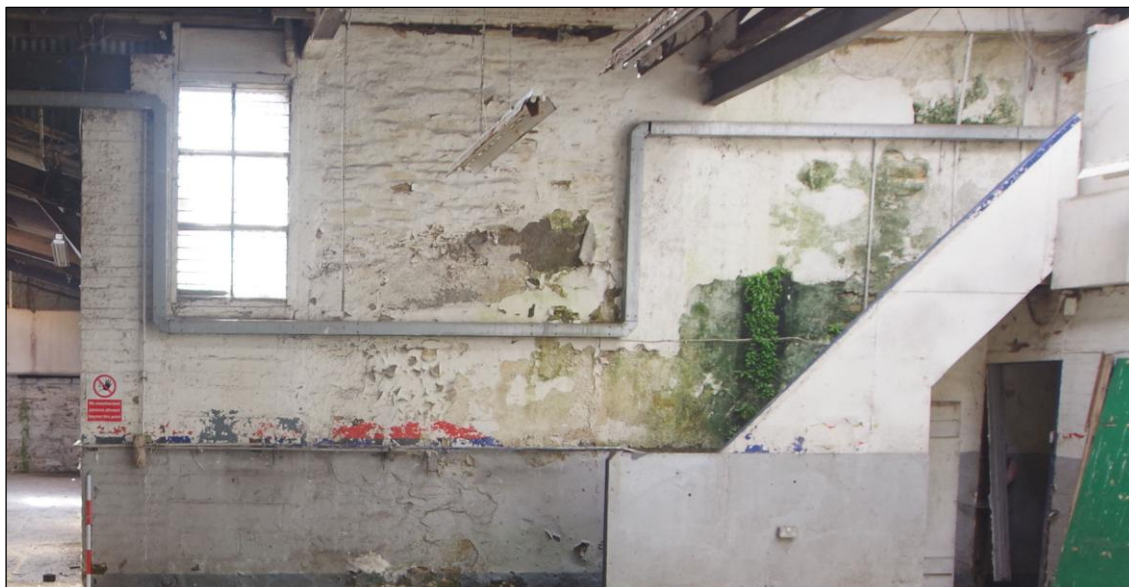
Fig 24 Interior south wall of the northern part of Room 1 (Garage).
