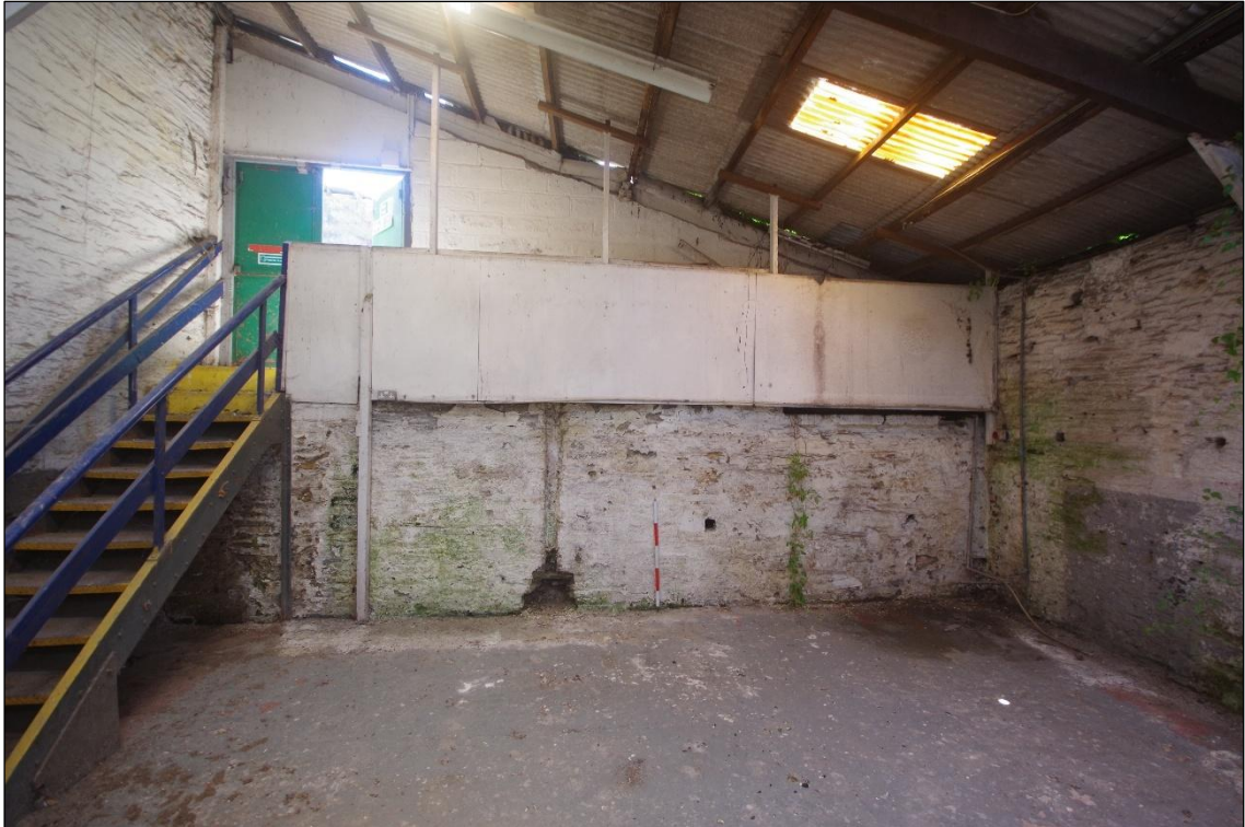
Fig 26 Interior south walls of the southern extension of Room 1 (Garage).
