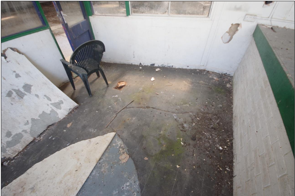
Fig 40 Floor surface of Room 2 (customer service desk).
