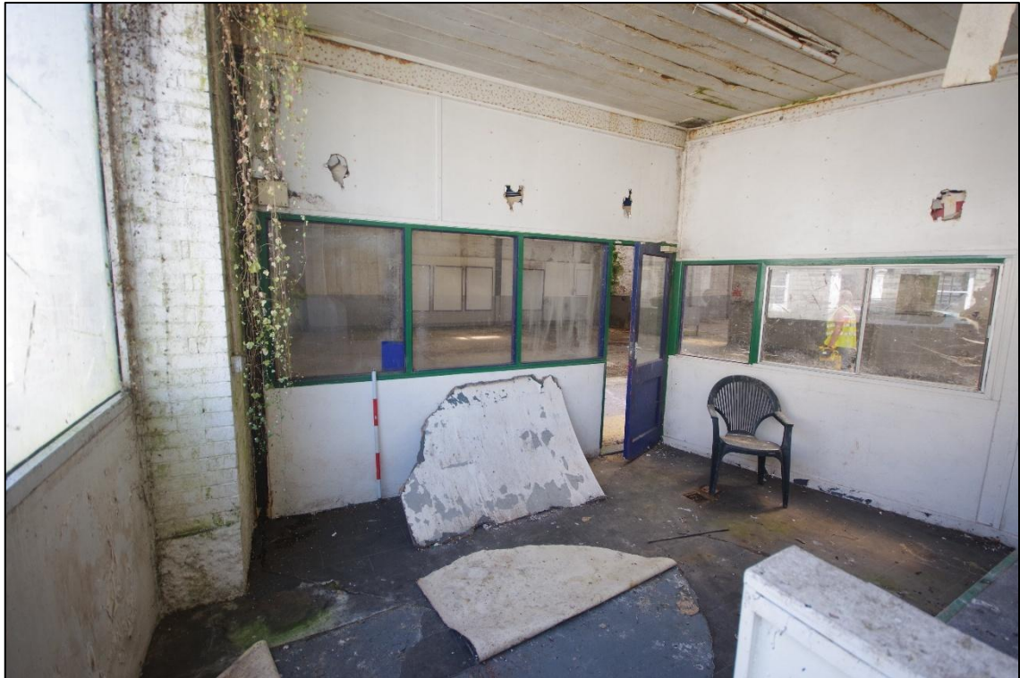
Fig 37 Interior east wall of Room 2 (customer service desk).
