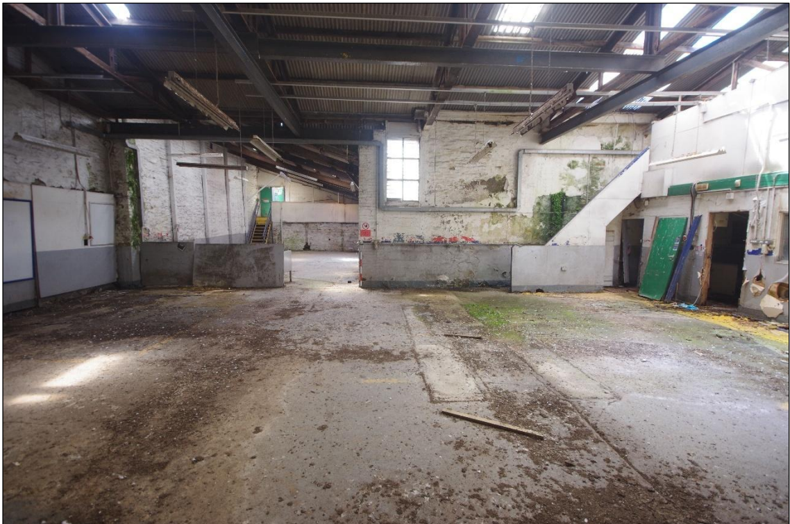
Fig 23 Interior south wall of the northern part of Room 1 (Garage).
