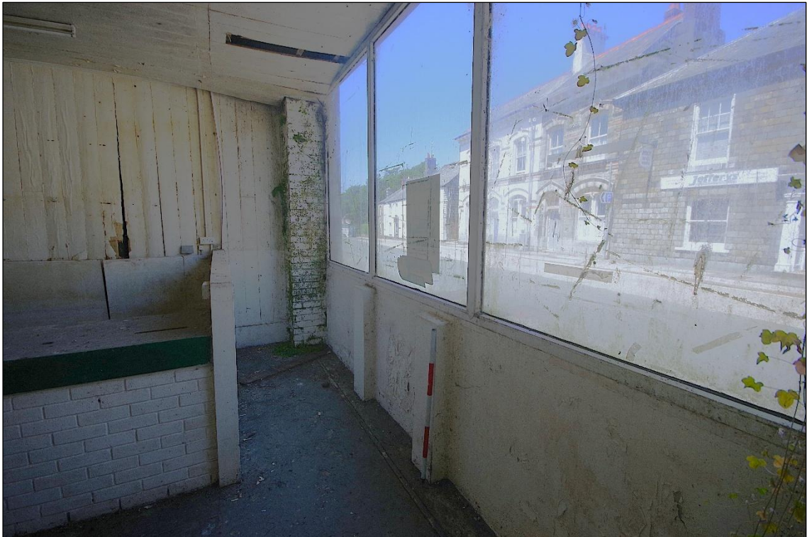
Fig 35 Interior north wall of Room 2 (customer service desk), looking north-west.
