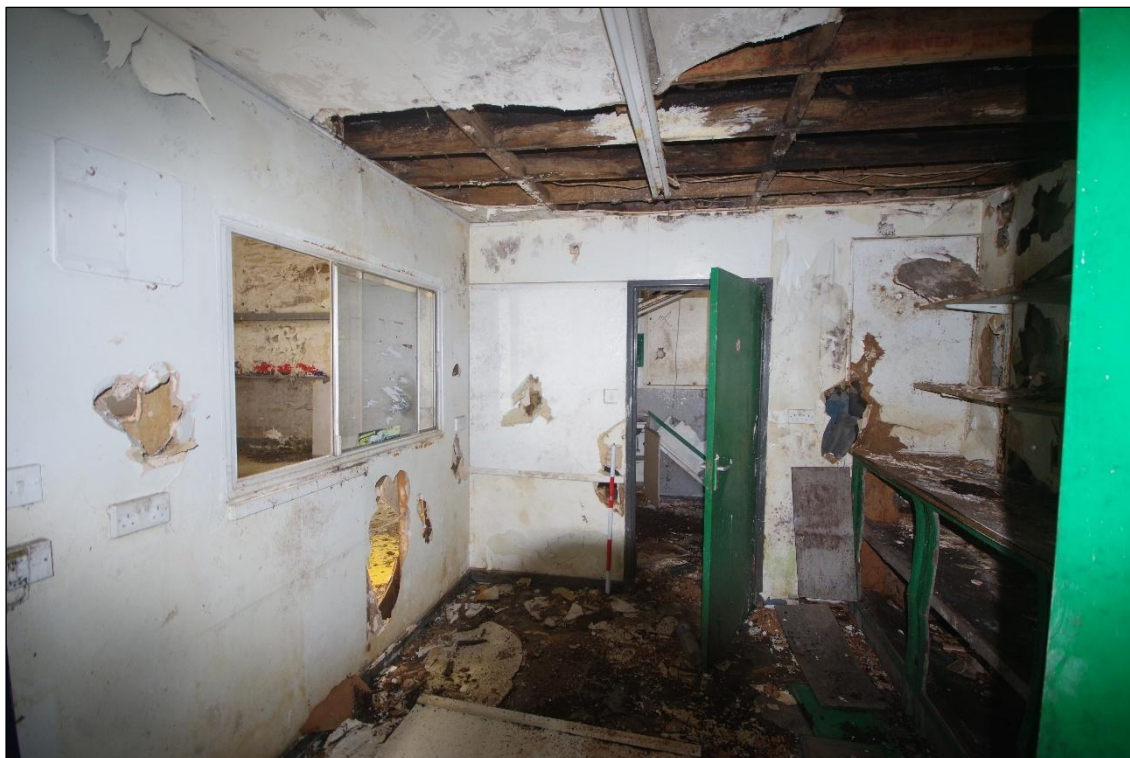
Fig 41 Room 3 (office), looking south.
