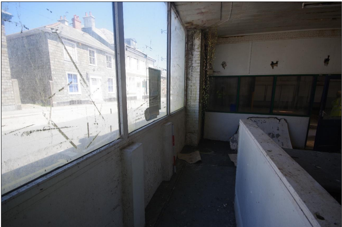
Fig 36 Interior north wall of Room 2 (customer service desk), looking north-east.
