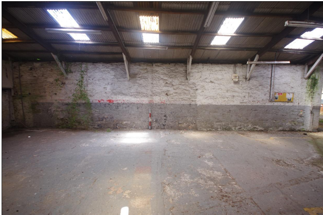
Fig 29 Interior west wall (south end) of the extension to Room 1 (Garage).
