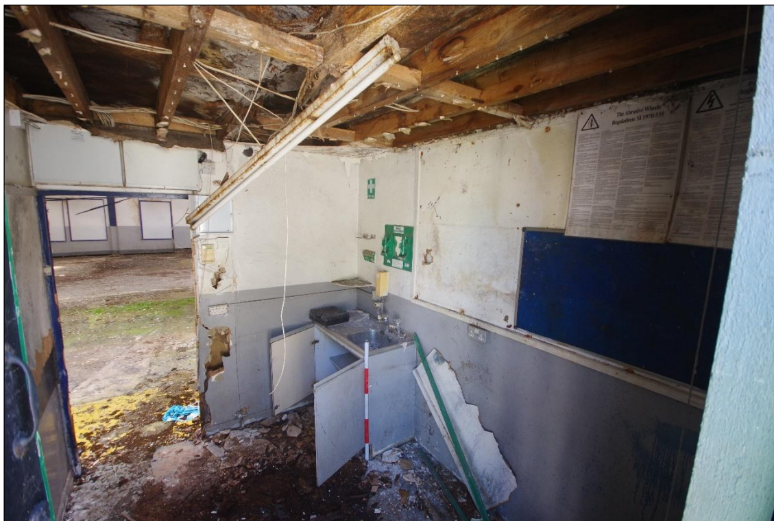
Fig 43 Room 4 (office) looking south-east.
