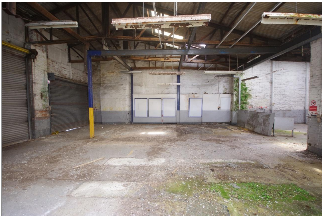
Fig 20 Interior northern part of the east wall of Room 1 (Garage).
