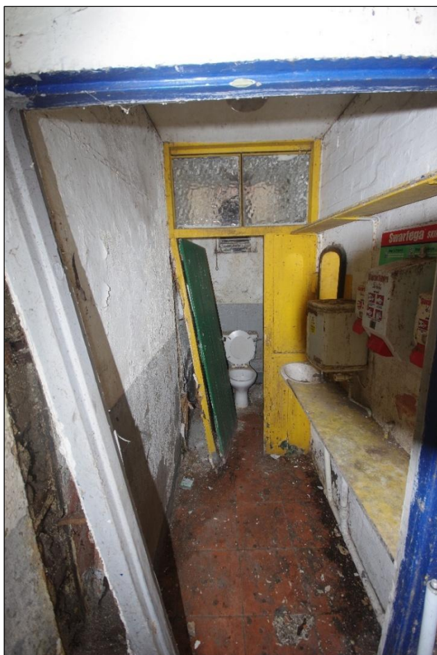
Fig 44 Room 5 (toilet), looking west.
