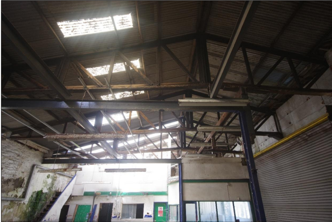
Fig 30 Roof structure at north end of room 1 (garage) looking west.
