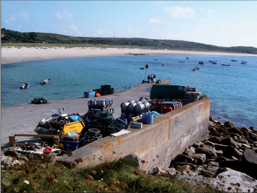
Fig 17 Higher Town Quay, St Martin's before commencement of works, September 2007 (photo: HES)
