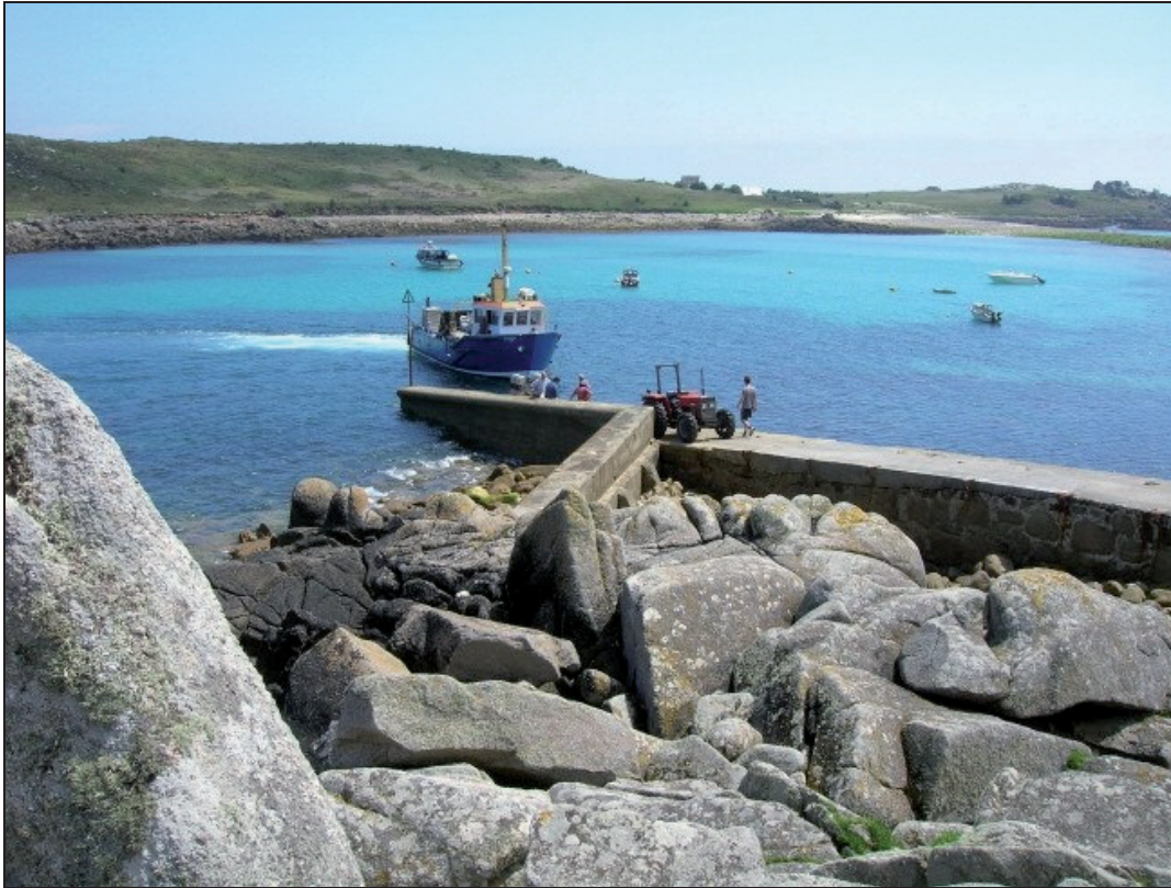
Fig 15 Porth Conger Quay, St Agnes before commencement of works, June 2007 (photo: HES)
