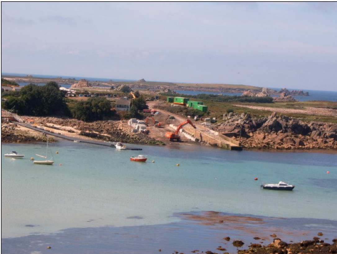
Fig 16 Porth Conger Quay, St Agnes during refurbishment work, September 2007 (photo: HES)
