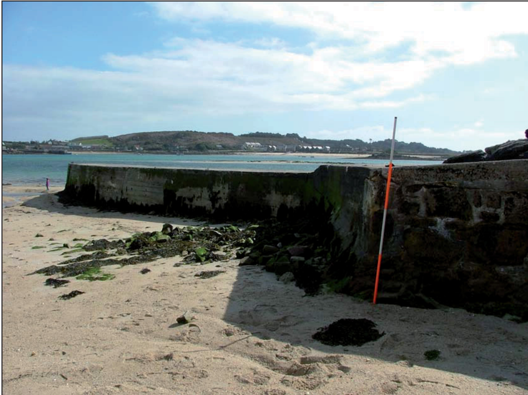
Fig 11 Church Quay, Bryher prior to works commencing, April 2007 (photo: Katharine Sawyer)
