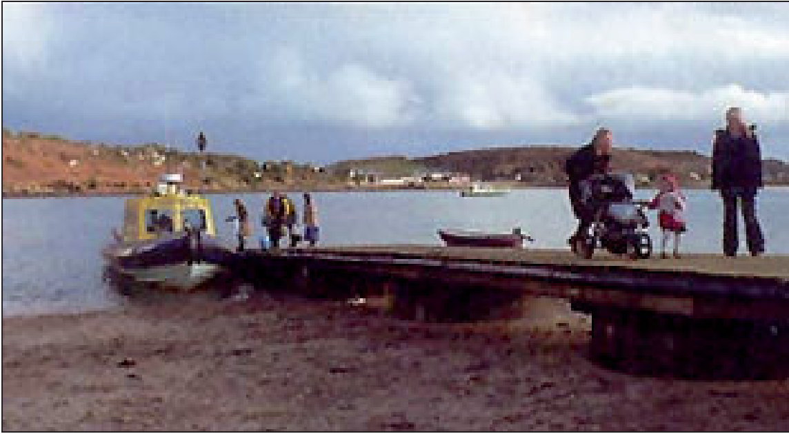
Fig 13 Anneka's Quay, Bryher, before commencement of works (photo: Edmund Nuttall Ltd)
