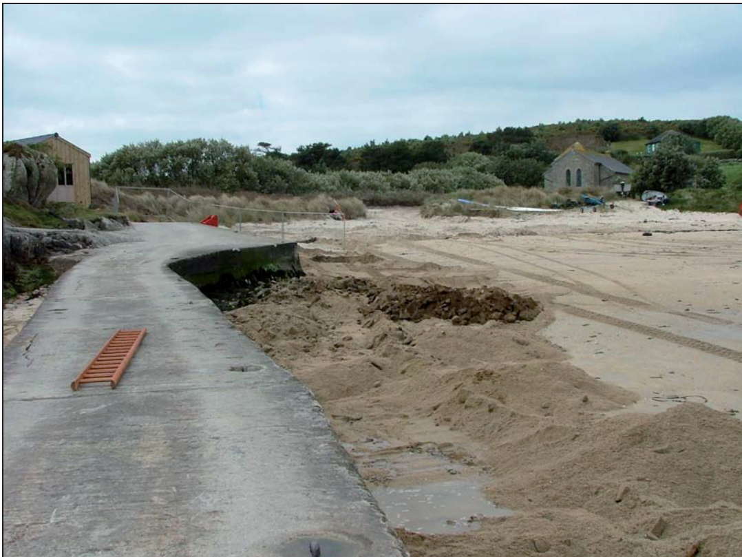
Fig 21 Excavations alongside Church Quay, April 2007 (photo: Katharine Sawyer)
