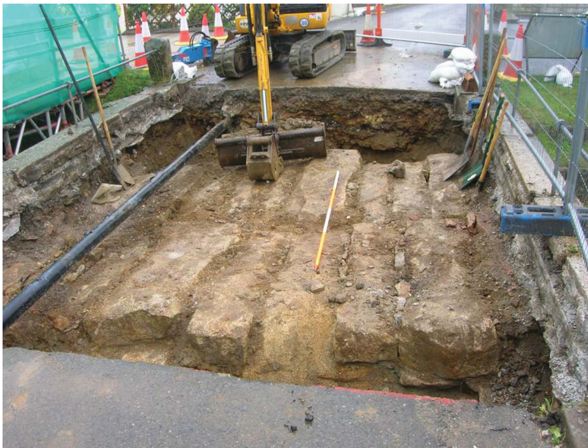
Fig 12 Overall view of bridge (from north) with roadway fill removed
