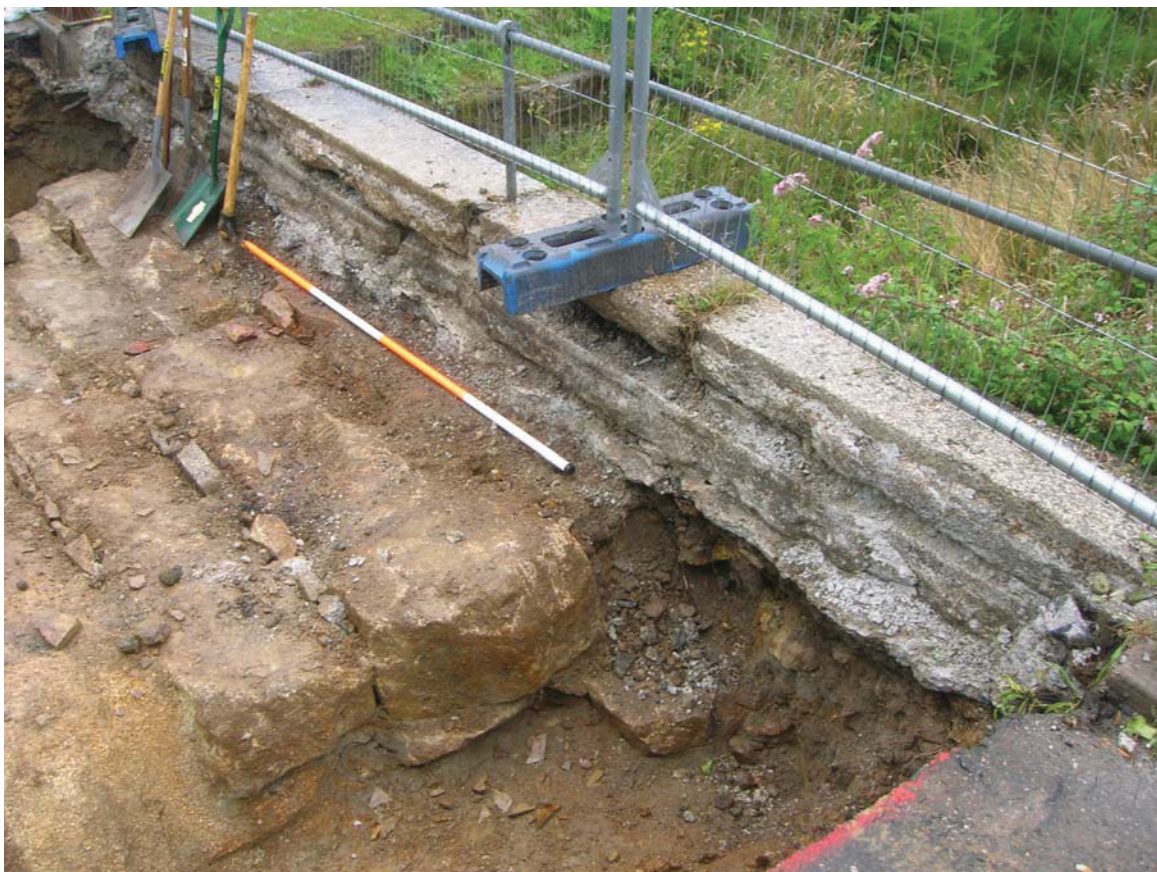
Fig 14 Rebuilt upstream side of the bridge showing 2 levels of kerbstones
