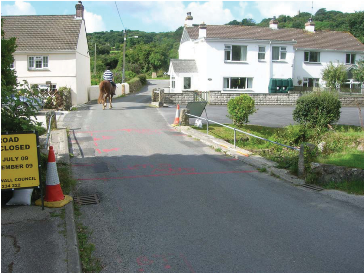
Fig 7 View of the bridge looking south
