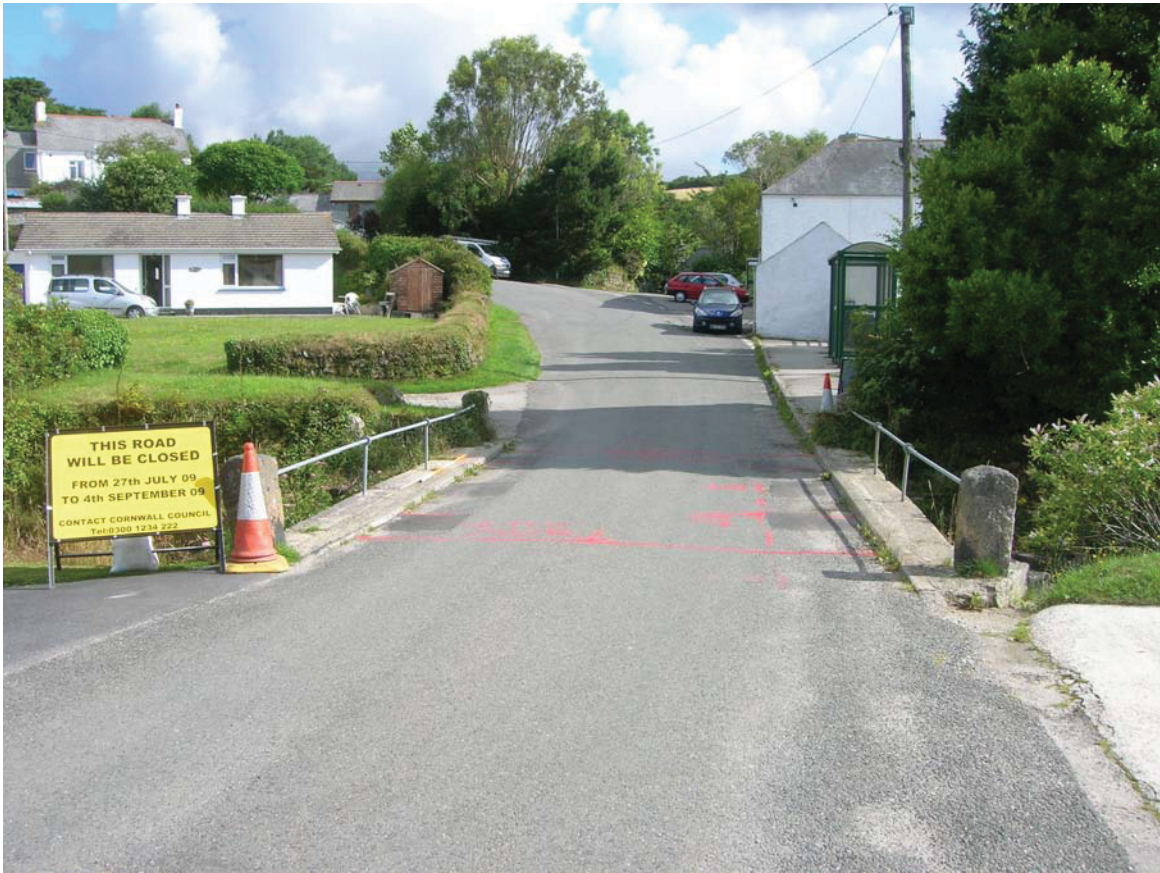
Fig 6 View of the bridge looking north
