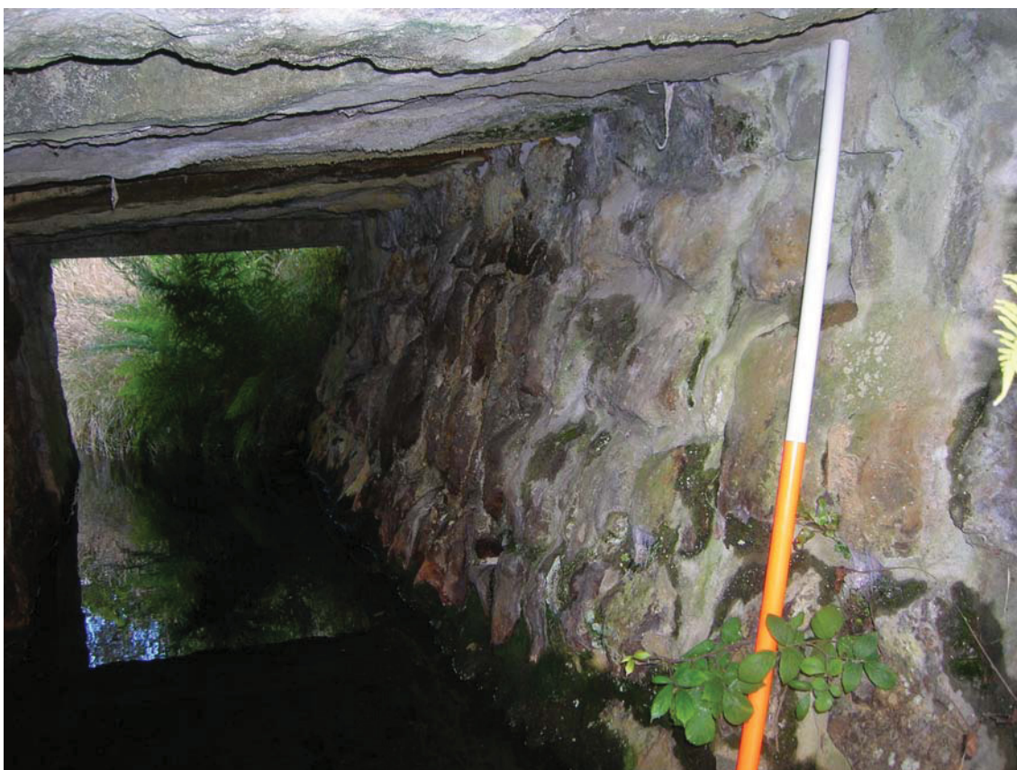
Fig 11 Northern span, showing the battered abutment face
