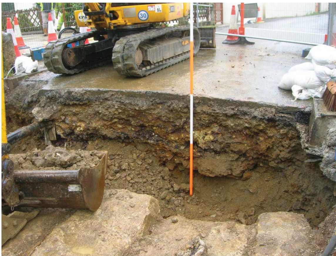
Fig 13 Roadway built up with mine waste
