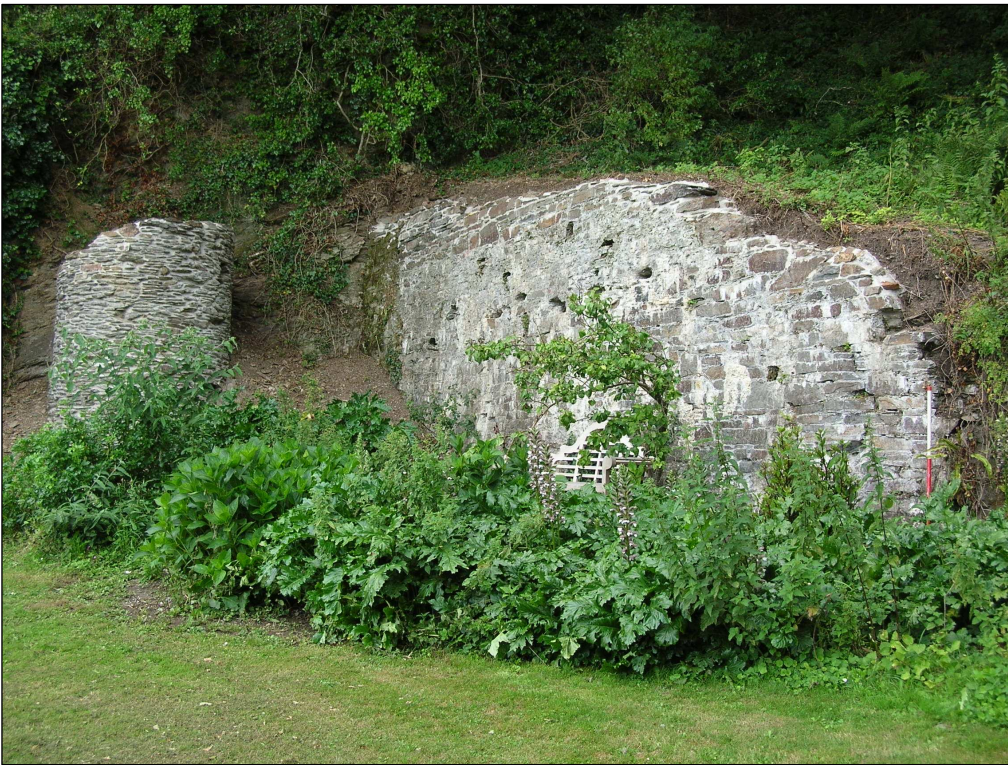
Fig 24 View of the winding engine boiler house chimney/buildings after works C Buck 2010© CC HE
