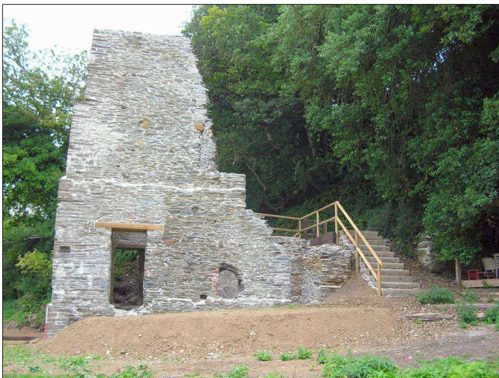
Fig 10 East side view of the Pumping Engine House after works C Buck 2010© CC HE
