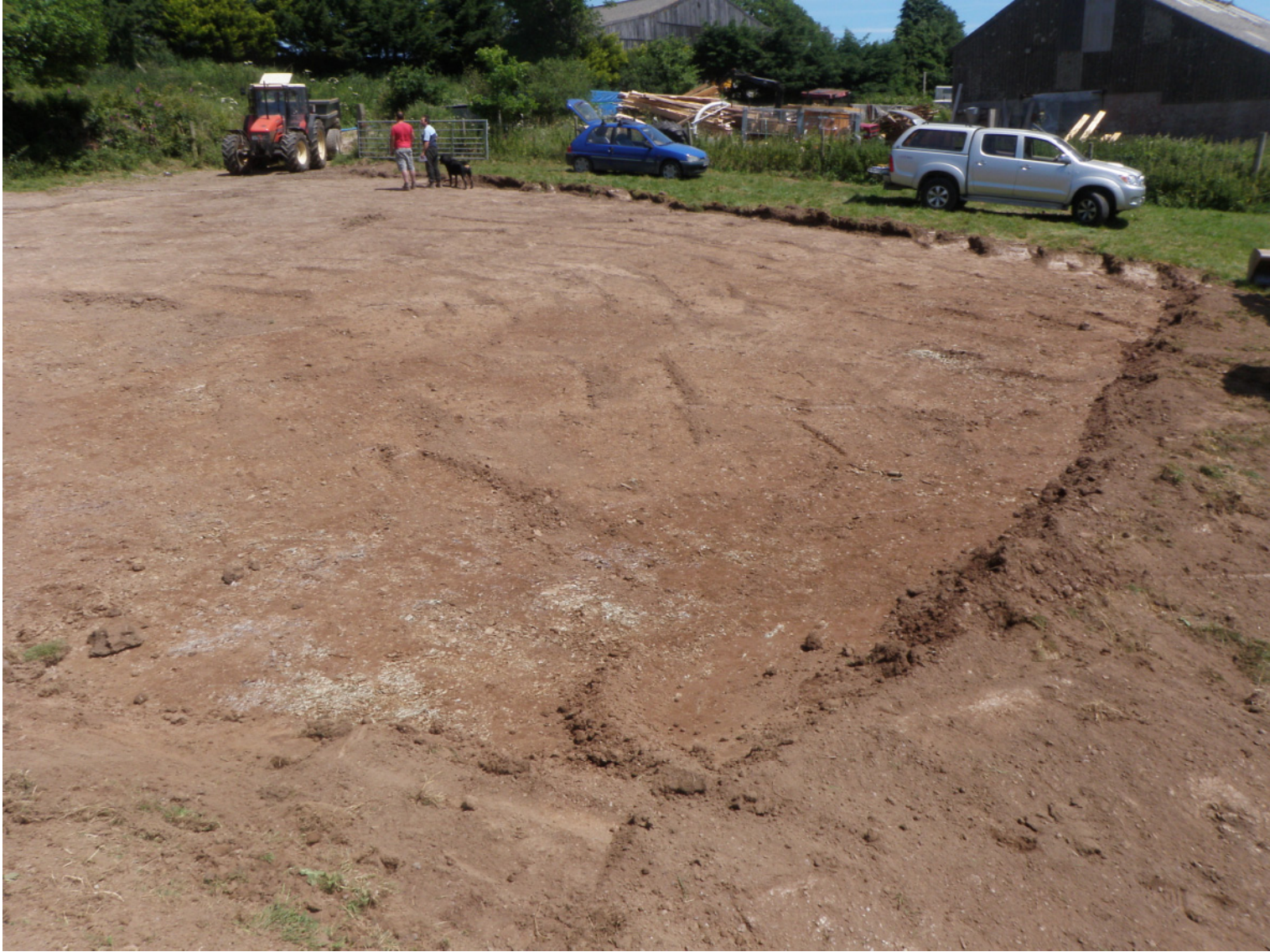
Fig 2: Stripped area looking north east
