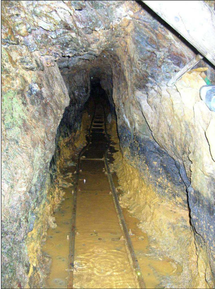
Fig 12 Middle adit (from entrance) after removal of rock/silt build up (Site 5) C Buck 2005 © HES
