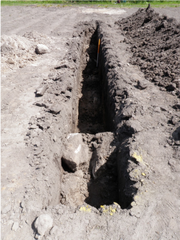
Fig 15 Trench 1 showing boundary wall (2) in foreground, looking east
