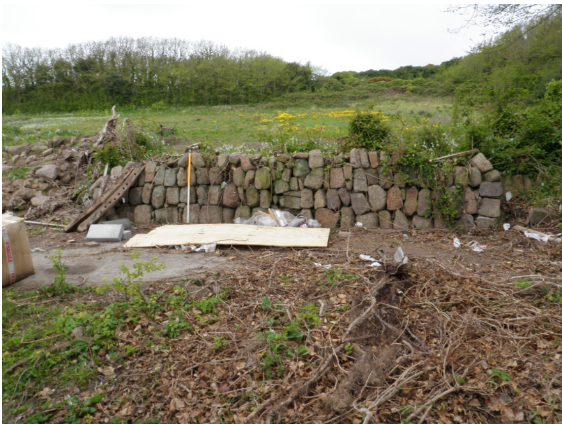
Fig 12 West wall of Building 8 looking west
