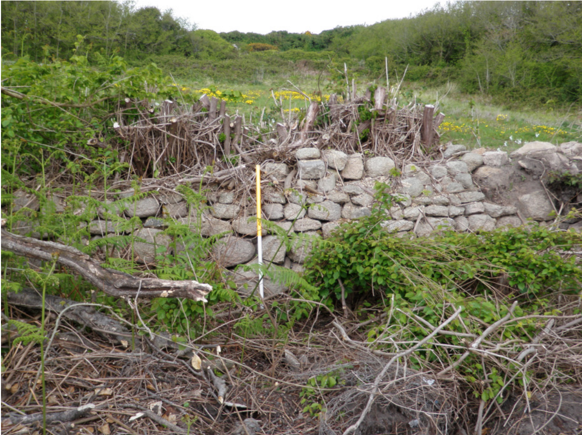
Fig 14 Retaining wall 10 looking west
