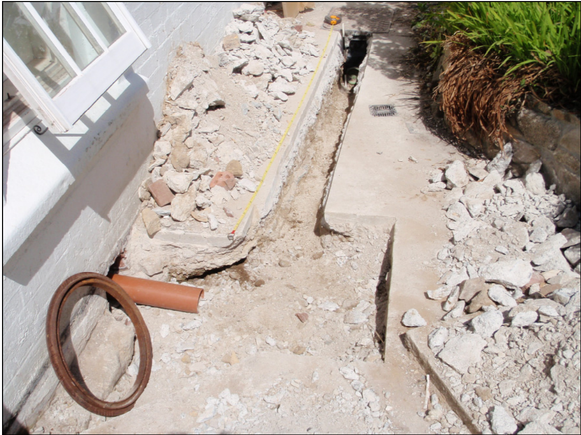
Fig 5 The excavated drain trench (photo: HE Projects)
