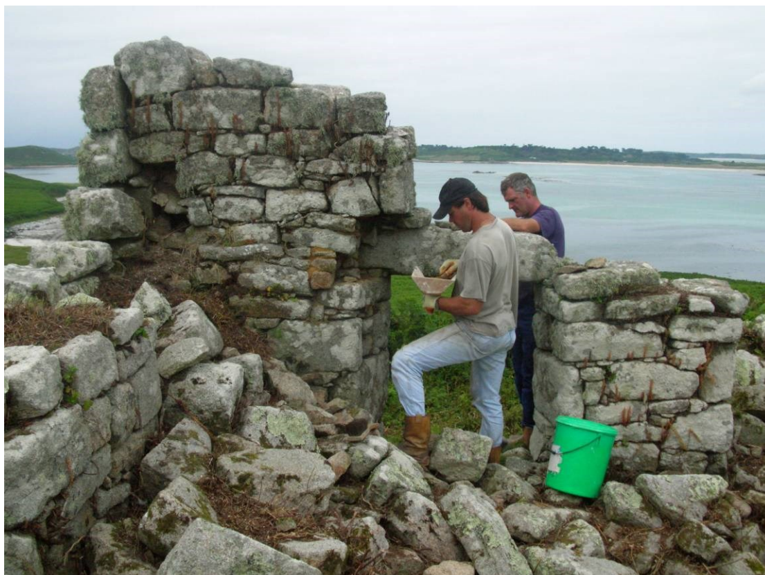
Fig 9.6 Consolidation work being carried out on House N on Samson in July 2006 (photo:Jacqui Mulville)
