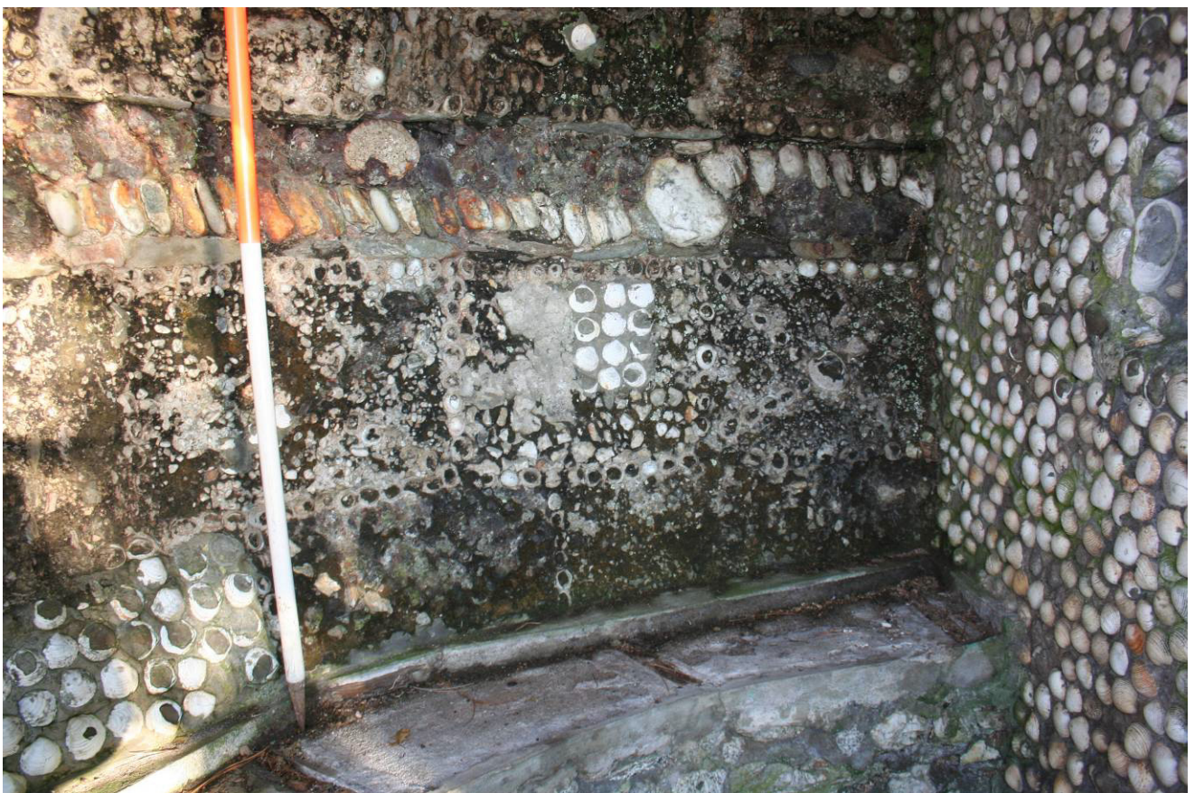
Fig 10: Back wall in western half
