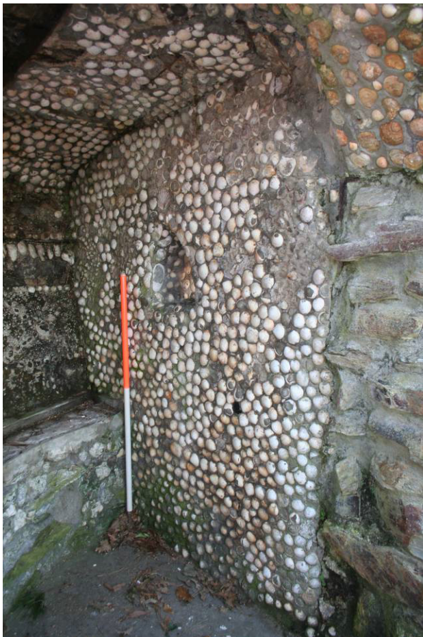
Fig 8: Interior dividing wall in western half
