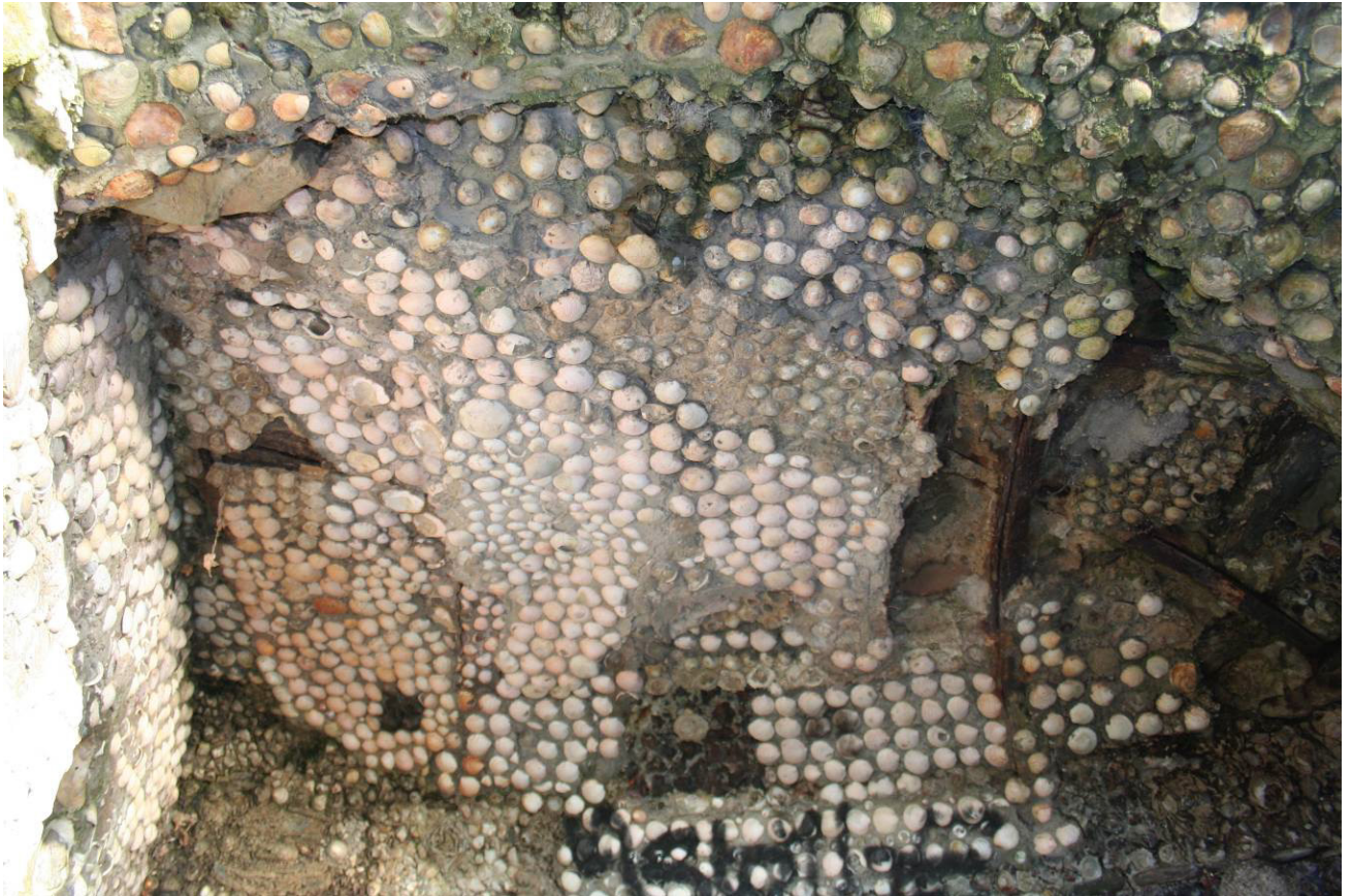
Fig 17: Ceiling in eastern half
