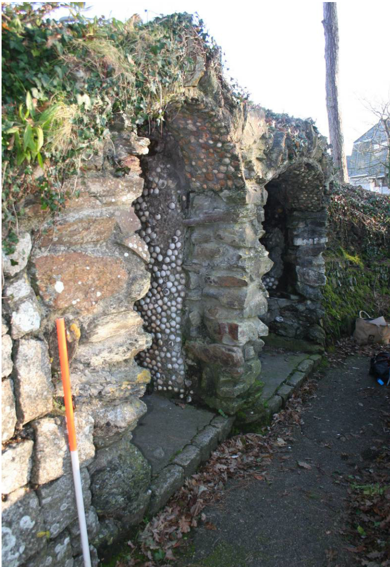
Fig 6: Present view of the front elevation looking north-east
