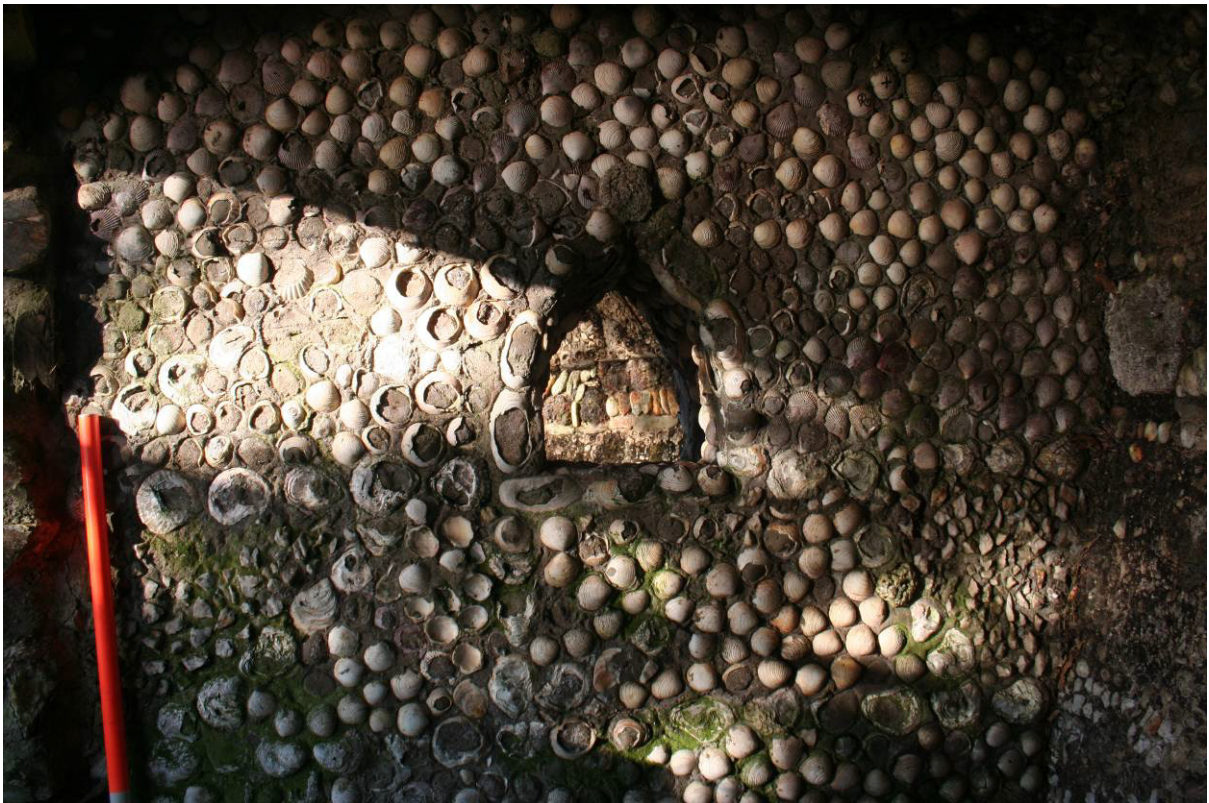
Fig 14: Interior dividing wall in eastern half
