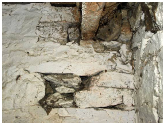
Fig 36 Building 1: rear wall detail, far right
