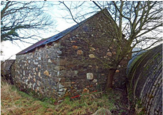
Fig 17 Building 1 from SW (rebuilt end wall)
