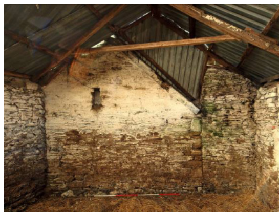
Fig 85 Building 4: W end
