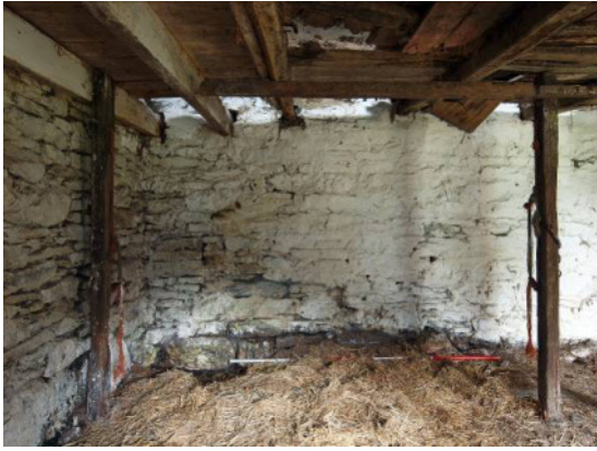
Fig 24 Building 1: rear wall, left
