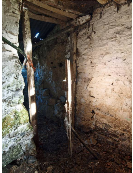
Fig 43 Building 1: NE corner, inserted doorway
