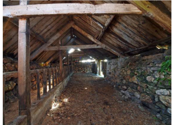
Fig 78 Building 3: shelter shed from N
