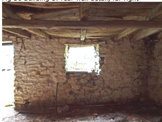
Fig 37 Building 1: E wall, right of doorway
