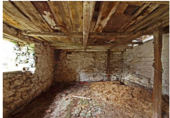
Fig 21 Building 1: S end
