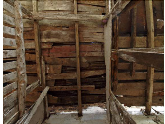
Fig 29 Building 1: ceiling, centre
