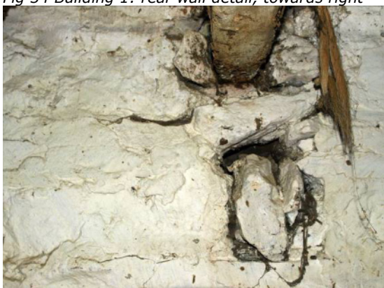
Fig 35 Building 1: rear wall detail, towards right
