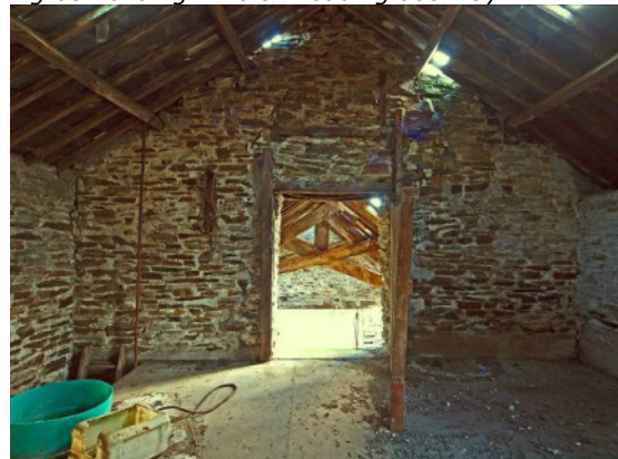
Fig 69 Building 2: loft E end
