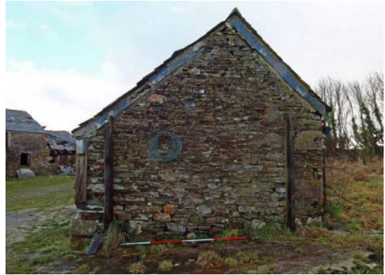
Fig 92 Building 4: W wall
