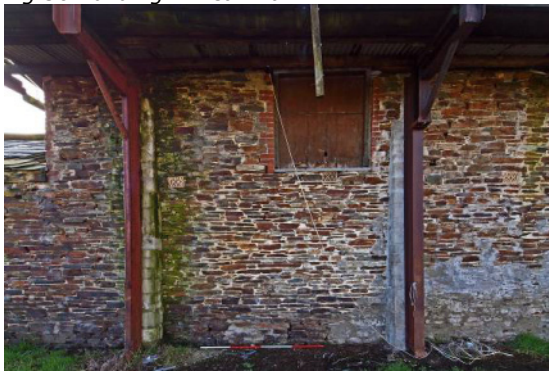
Fig 57 Building 2: rear wall loading doorway
