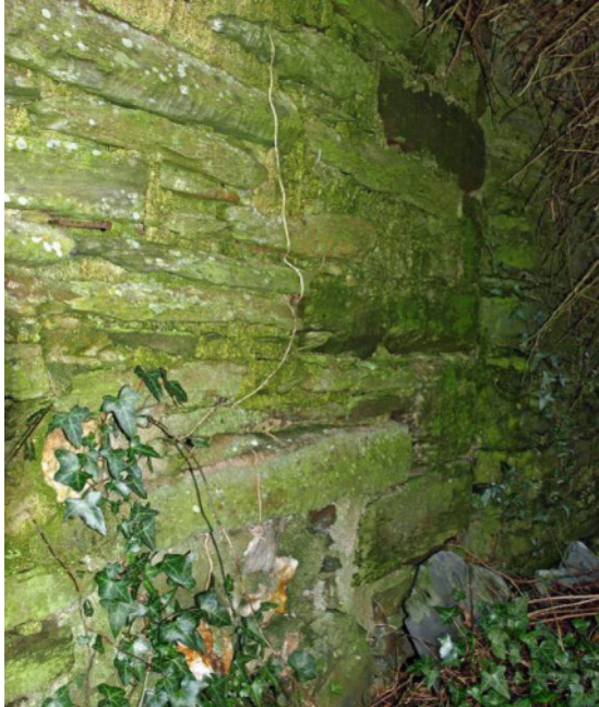
Fig 90 Building 5: rear wall phase joint
