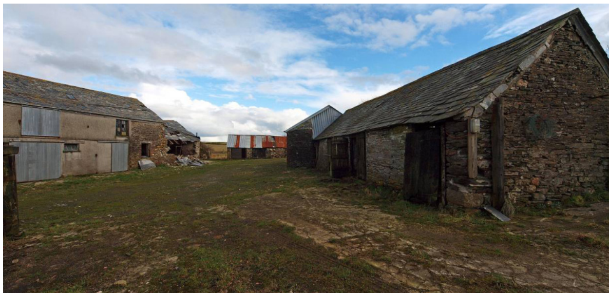
Fig 7 Context: Buildings 2, 3, 4 and 5 from west
