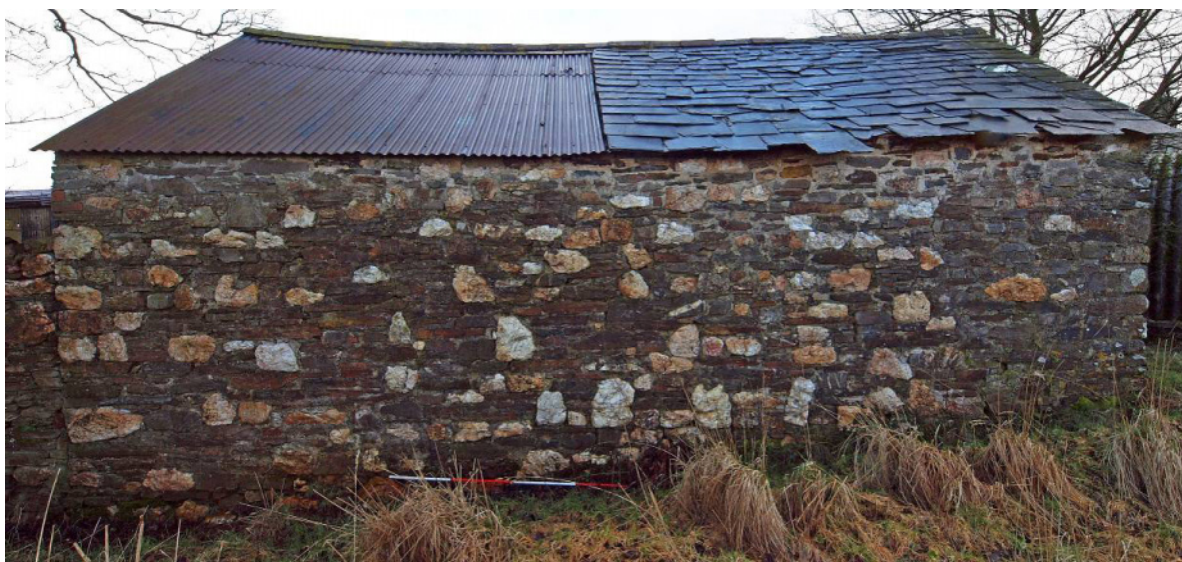
Fig 10 Building 1: rear (west) elevation (right-hand end and eaves walling rebuilt)
