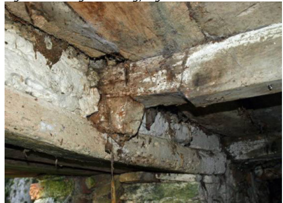
Fig 31 Building 1; E wall, joist over S window
