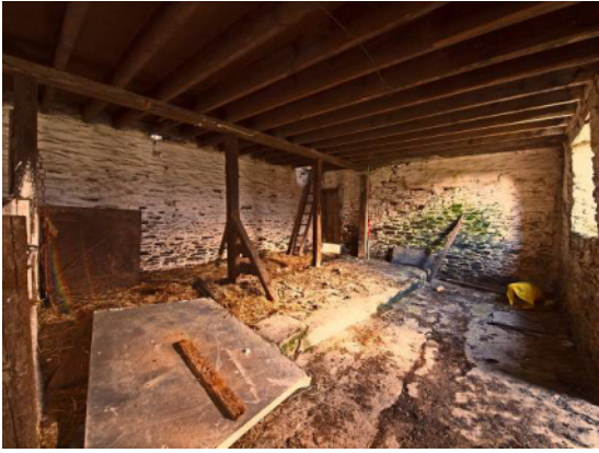
Fig 63 Building 2: NE corner
