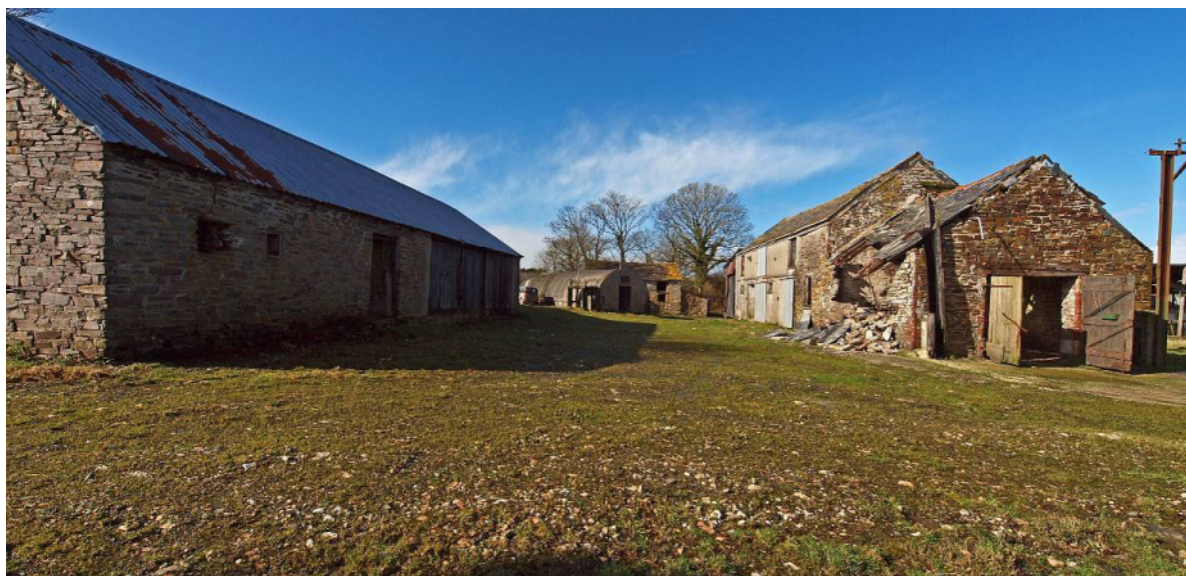
Fig 8 Context: Buildings 4, 1 and 2 from east
