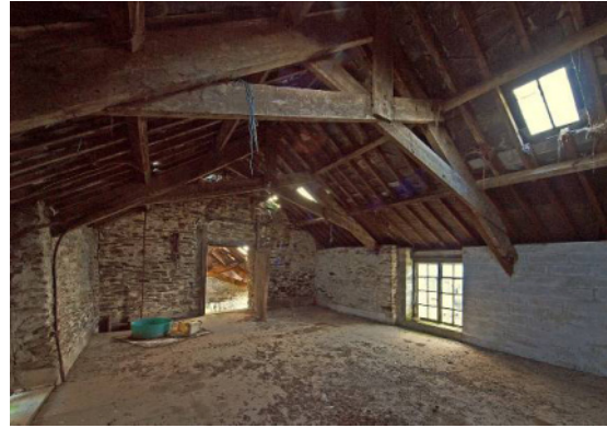
Fig 67 Building 2: loft E end
