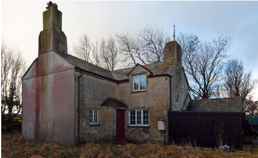
Fig 104 Hallgarden farmhouse: side view
