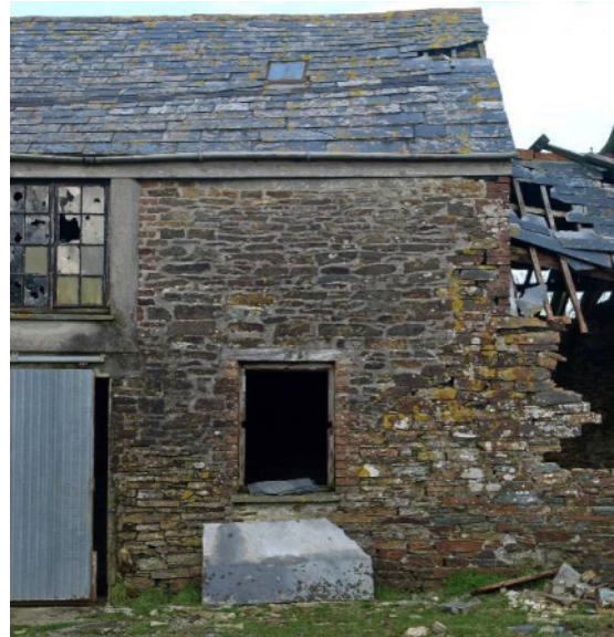
Fig 50 Building 2: front wall towards right
