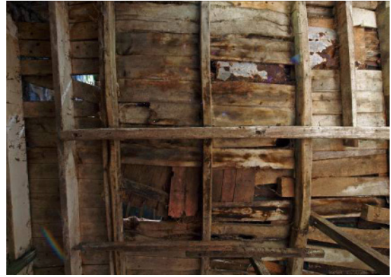
Fig 28 Building 1: ceiling, south end
