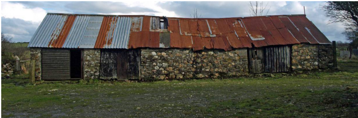
Fig 13 Building 3: cart-sheds and shippon, built in at least 2 principal phases
