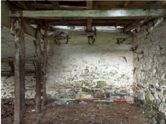
Fig 26 Building 1: rear wall, right
