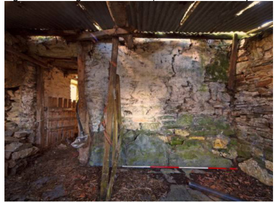
Fig 44 Building 1: lean-to from N
