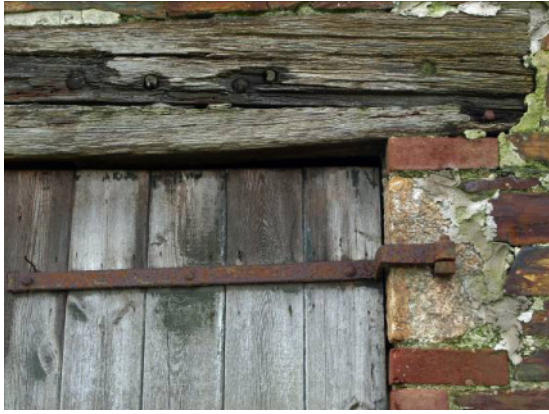
Fig 54 Building 2: E doorway (ship's timber)
