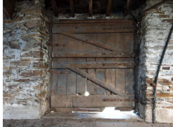
Fig 68 Building 2: loft N loading doorway
