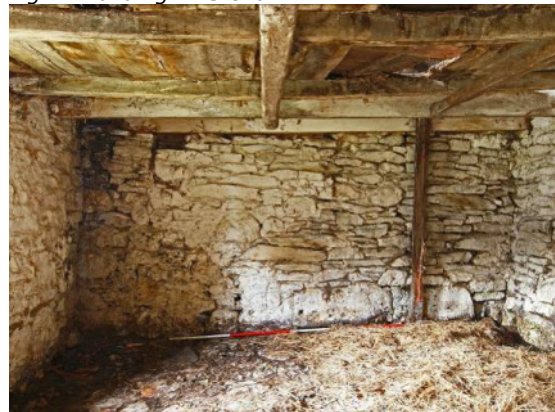
Fig 22 Building 1: S end
