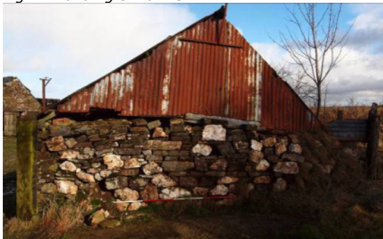
Fig 75 Building 3: S wall
