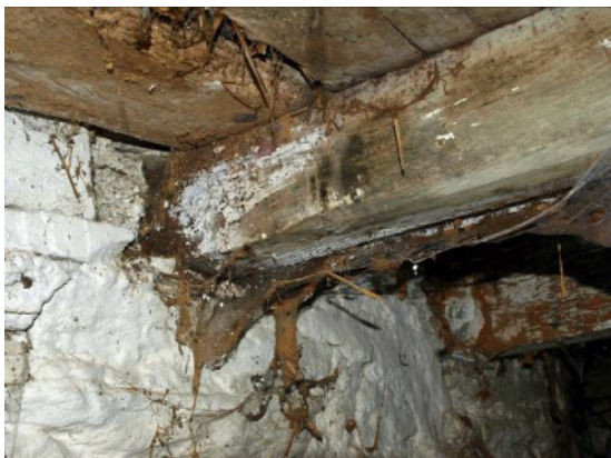
Fig 32 Building 1: E wall, joist towards right
