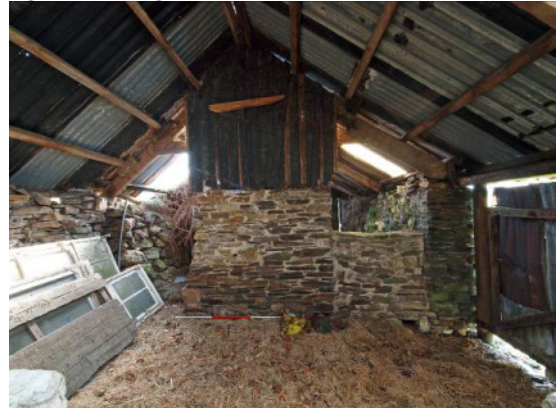
Fig 77 Building 3: cart-shed from N
