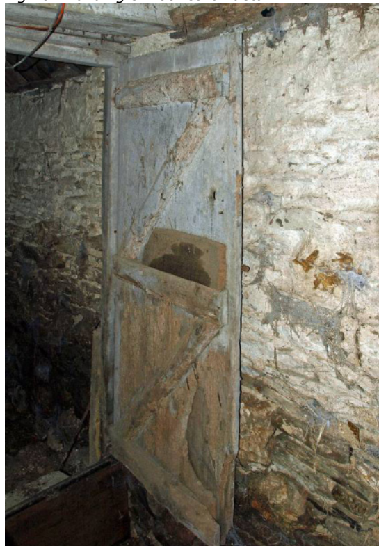
Fig 103 Building 5: doorway, E end of passage
