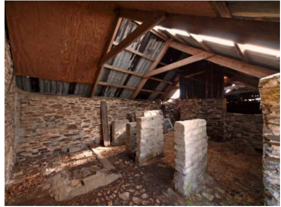
Fig 76 Building 3: cart-shed from NW
