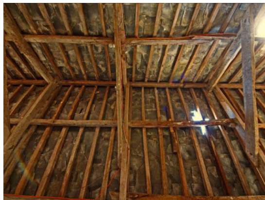
Fig 100 Building 5: roof above pigsties
