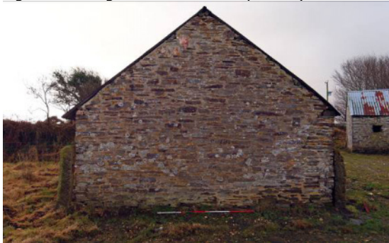
Fig 72 Building 3 N end
