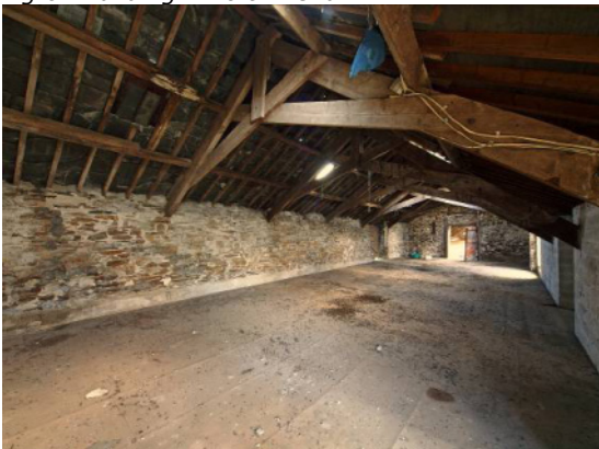
Fig 65 Building 2: loft from SW
