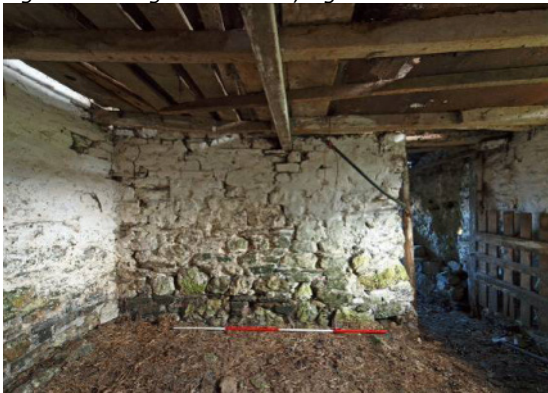
Fig 27 Building 1: north wall
