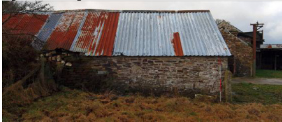
Fig 73 Building 3: E wall, right
