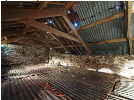
Fig 40 Building 1: loft from NE
