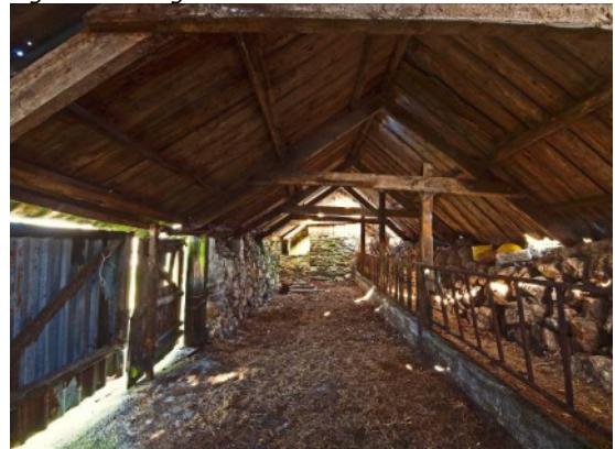
Fig 79 Building 3: shelter shed from S
