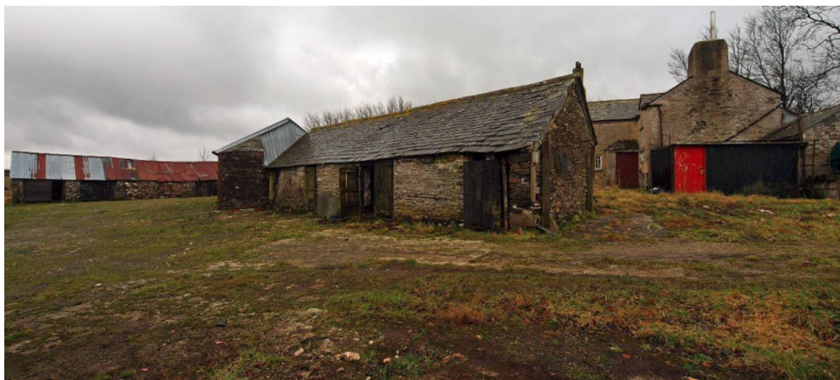
Fig 6 Context: Buildings 3,4 and 5 plus farmhouse at far right, from west
