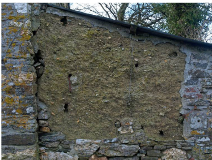
Fig 11 Building 1: lean-to E wall detail
