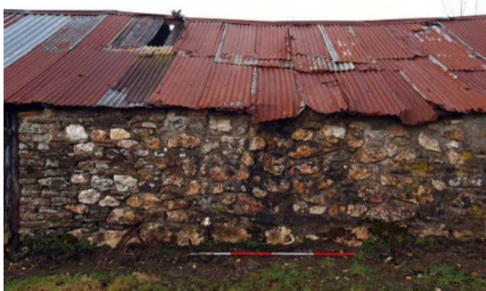
Fig 71 Building 3: W wall detail (centre)
