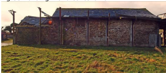
Fig 56 Building 2: rear wall
