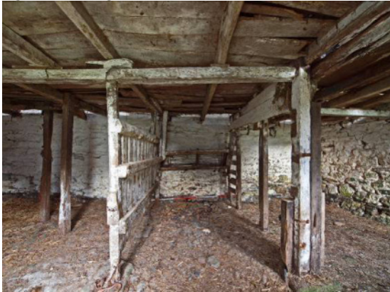
Fig 25 Building 1 from east
