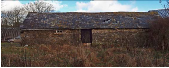
Fig 89 Building 5: rear wall
