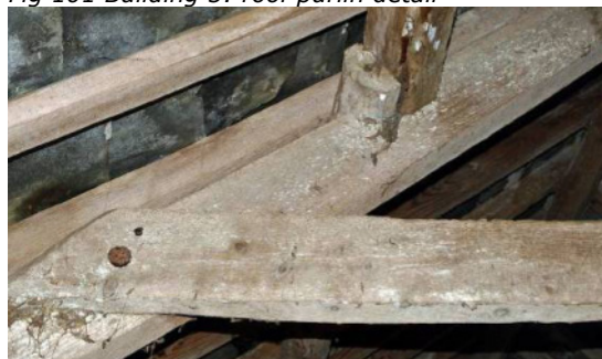
Fig 102 Building 5: roof collar detail
