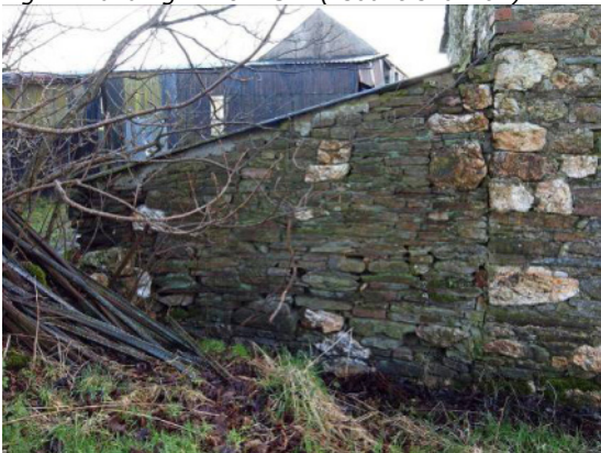
Fig 18 Building 1: lean-to (phase joint)
