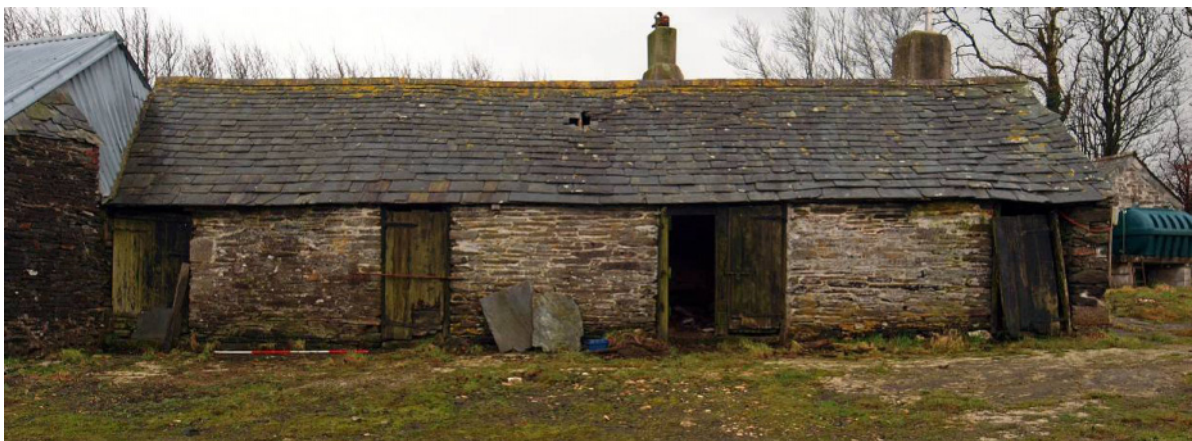
Fig 15 Building 5: north front (single-phase probable pigsties)
