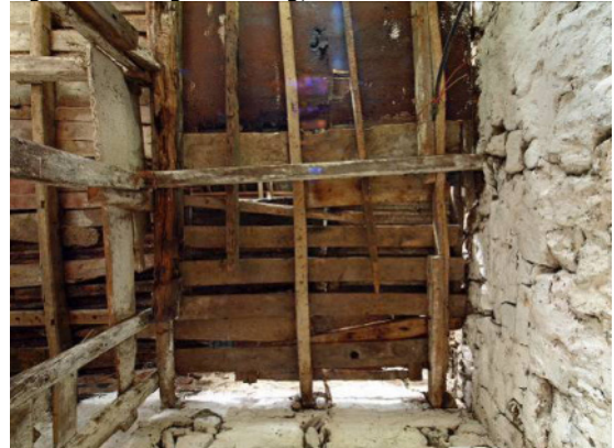
Fig 30 Building 1: ceiling, right
