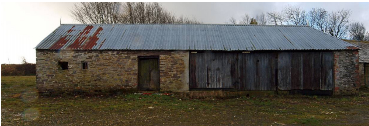
Fig 14 Building 4: shippon, built in 2 phases
