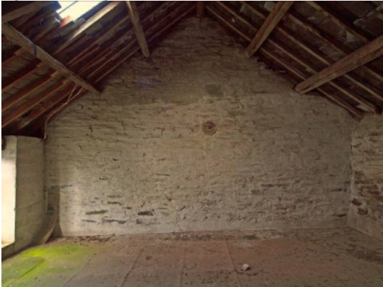
Fig 64 Building 2: loft W end
