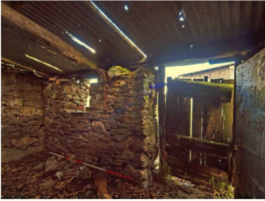
Fig 46 Building 1: lean-to from SE
