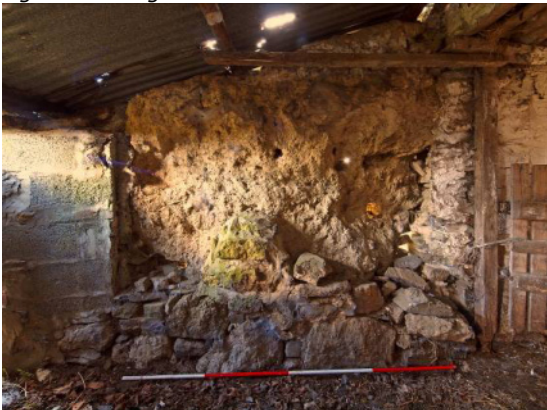
Fig 47 Building 1: lean-to E wall
