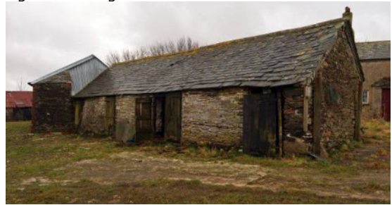
Fig 93 Building 4: from NW
