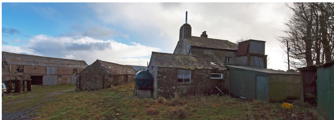
Fig 106 Rear of Hallgarden farmhouse, with buildings 2 and 5 beyond
