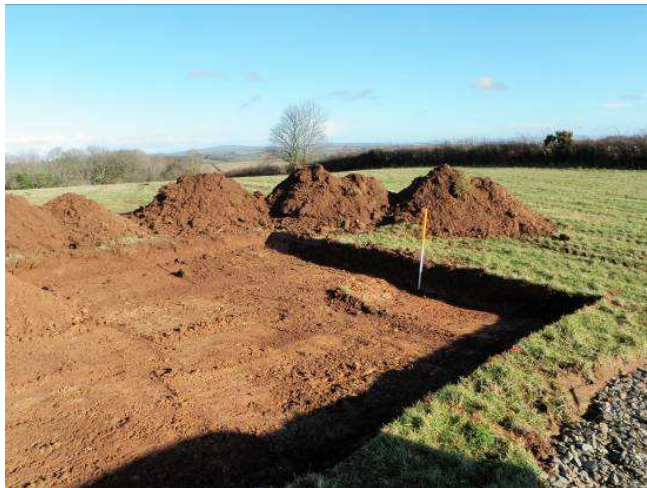
Fig 5 Excavation of the wind turbine footprint, showing ploughsoil overlying natural subsoil.
