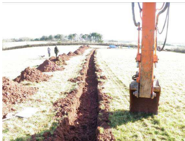
Fig 6 Excavated cable trench running east from the house towards the turbine.
