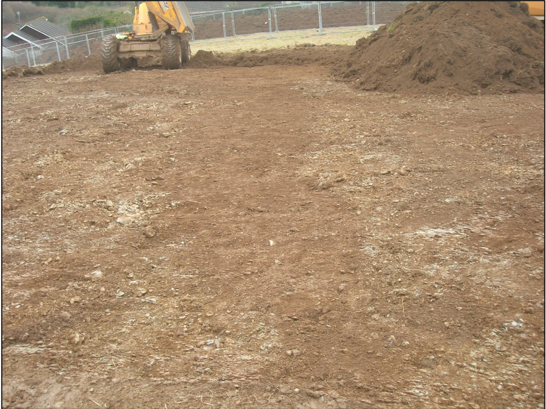
Fig 9 Ditch [05] looking east.
