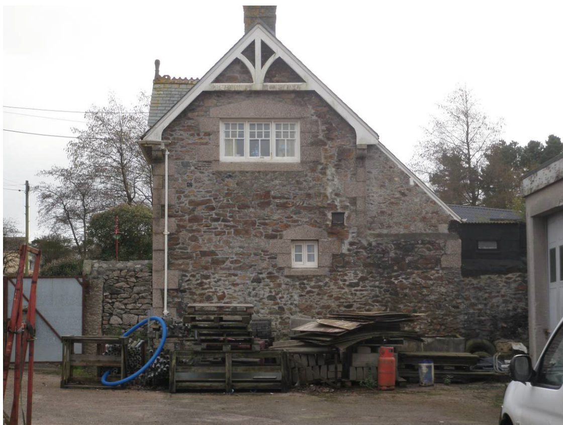
Fig 25: Site 23- Smelting works manager's office built on top of existing boundary wall
