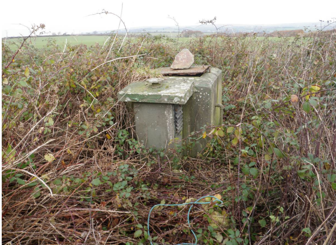
Fig 4 Surface feature of the Royal Observer Corps monitoring post HER No MCO42712
