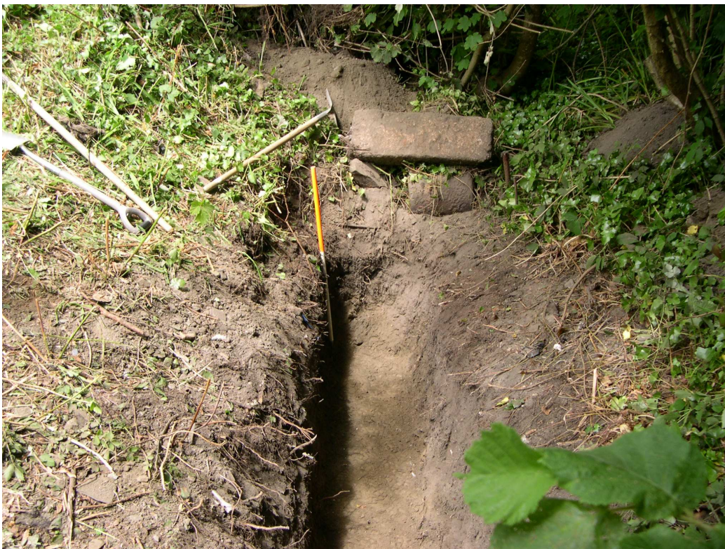
Figure 7 Looking east-north-east along the length of the soakaway (30 th June 2010). Note the stray granite block on top above the end of the trench, the rooty, dry exposed soil in section, and part of the edge of the pre-soakaway trench (see left of top of ranging rod).
