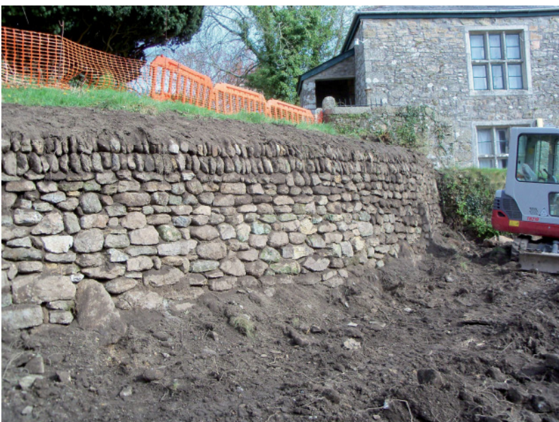
Figure 11 Looking north along the completed new walling.
