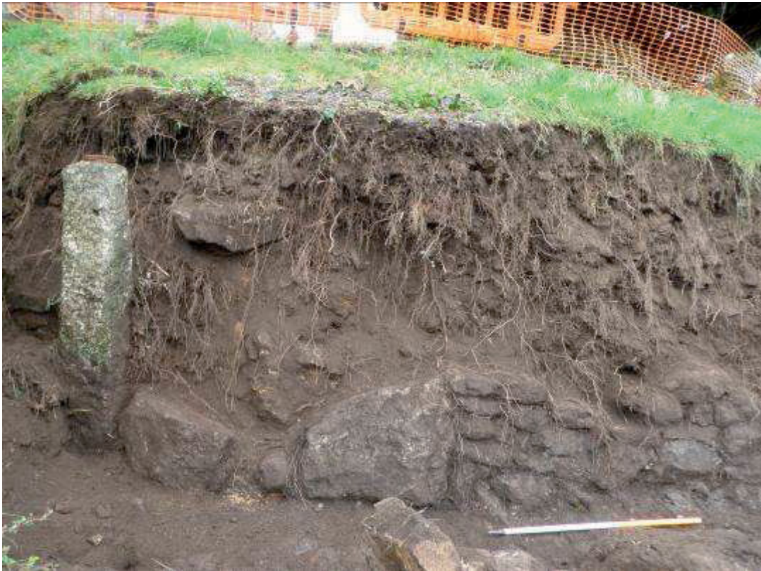
Figure 7 Looking north at the western end of the wall, showing the c19 th century granite gate post (subsequently removed) and differing wall construction techniques.
