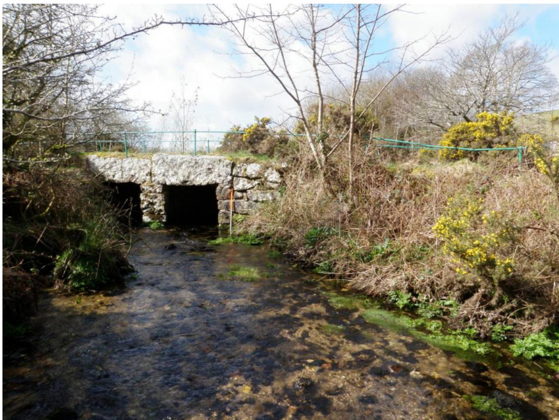
*Fig 11 Northern half of east (upstream) elevation (two spans) showing iron parapet railings*
