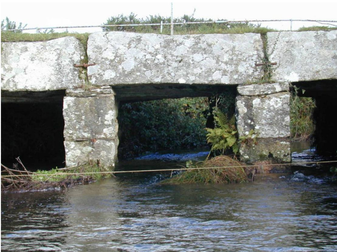
*Fig 10 West (downstream) elevation showing details of granite lintels and piers and iron ties*
