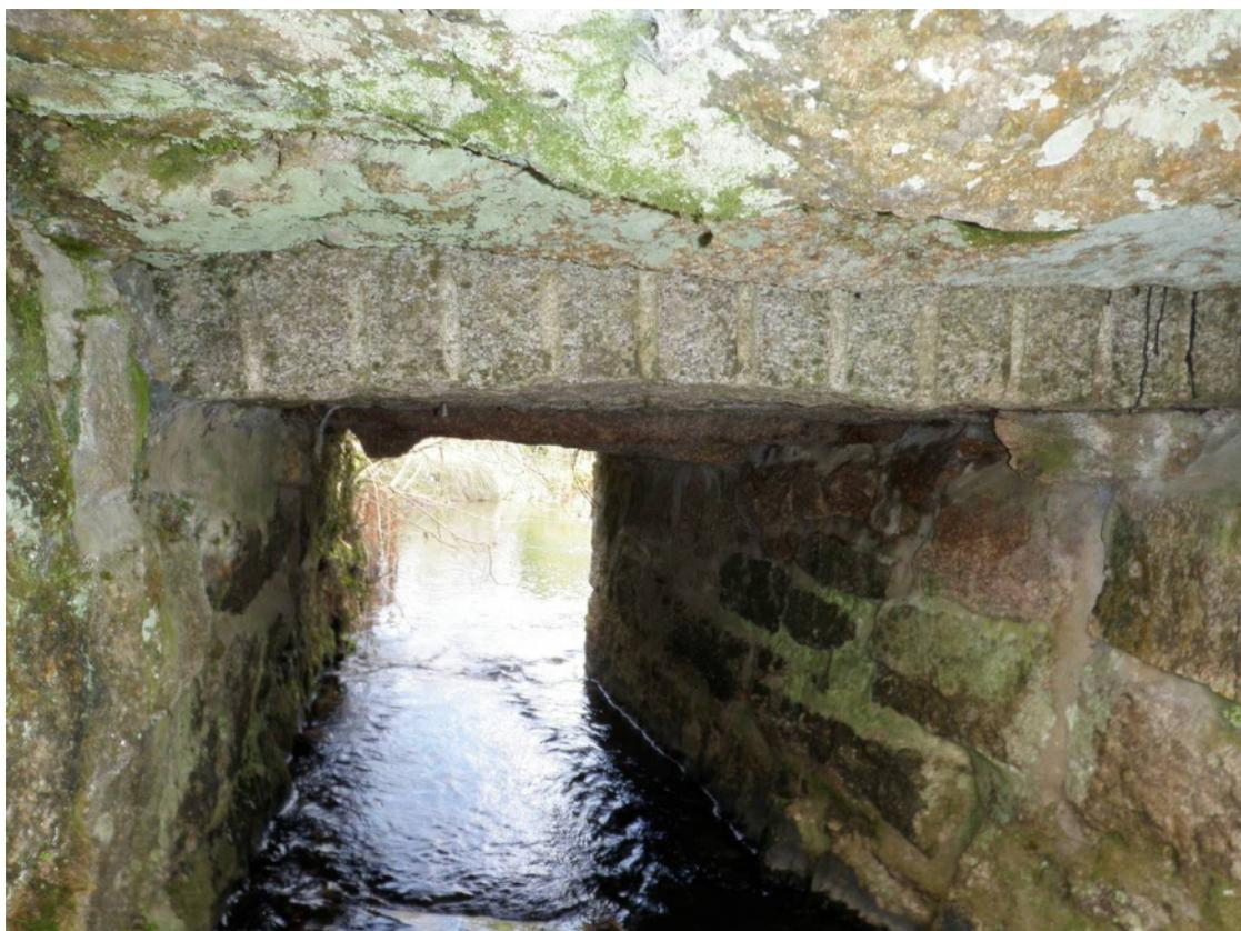
*Fig 14 View through southern span looking west and showing late 19<sup>th</sup> century quarry drill marks on one of the granite lintels*
