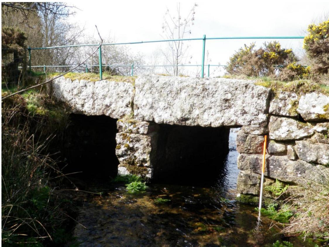
*Fig 12 Northern half of east (upstream) elevation (two spans) showing quarry drill marks on the granite lintel*
