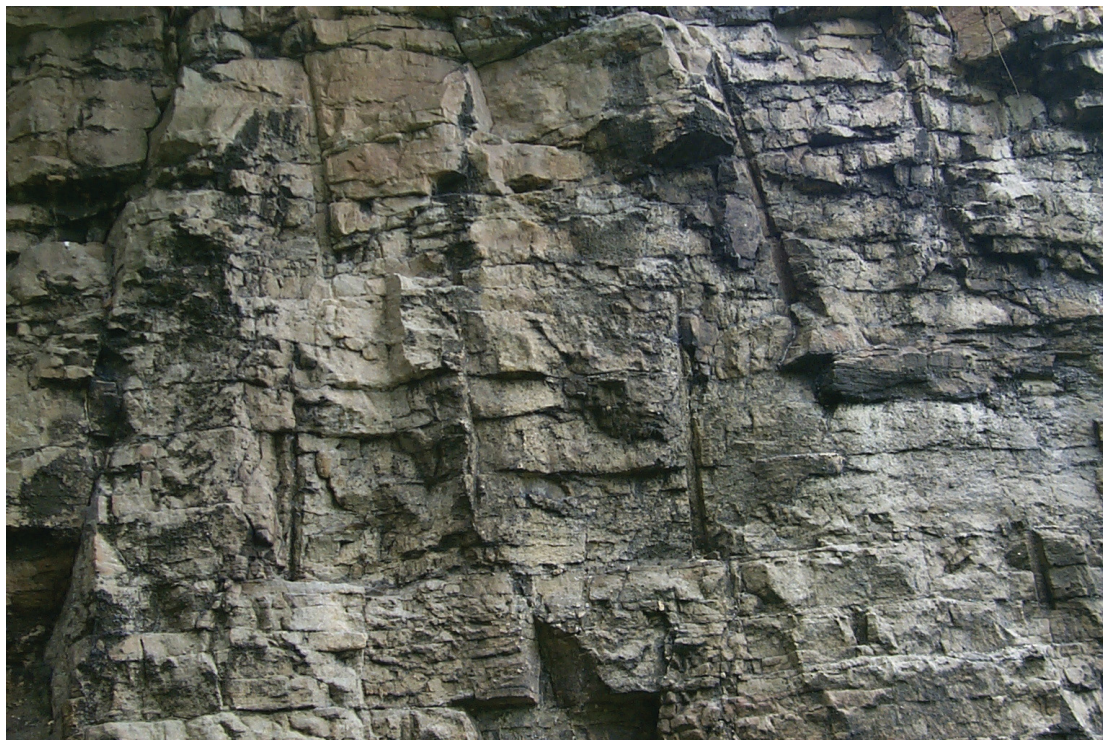
Plate 6: Drill holes for rock blasting in Pleasley Vale.
